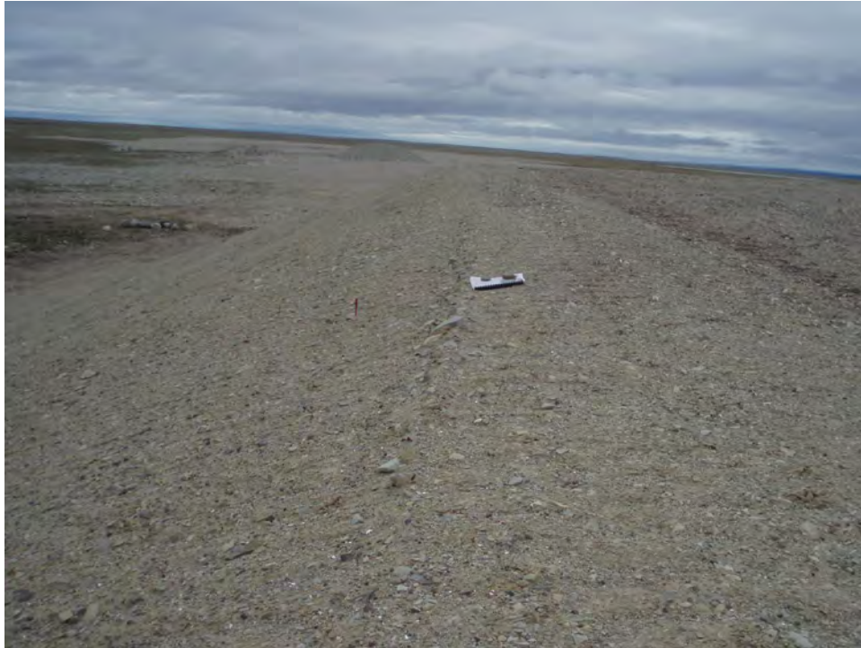
Photograph 5. West Facing Slope - Looking NE (Settlement On Slope, Approx 2m by 2m by 100 to 150mm), Not a Scarp, Could be due to Improper Grading ↑
