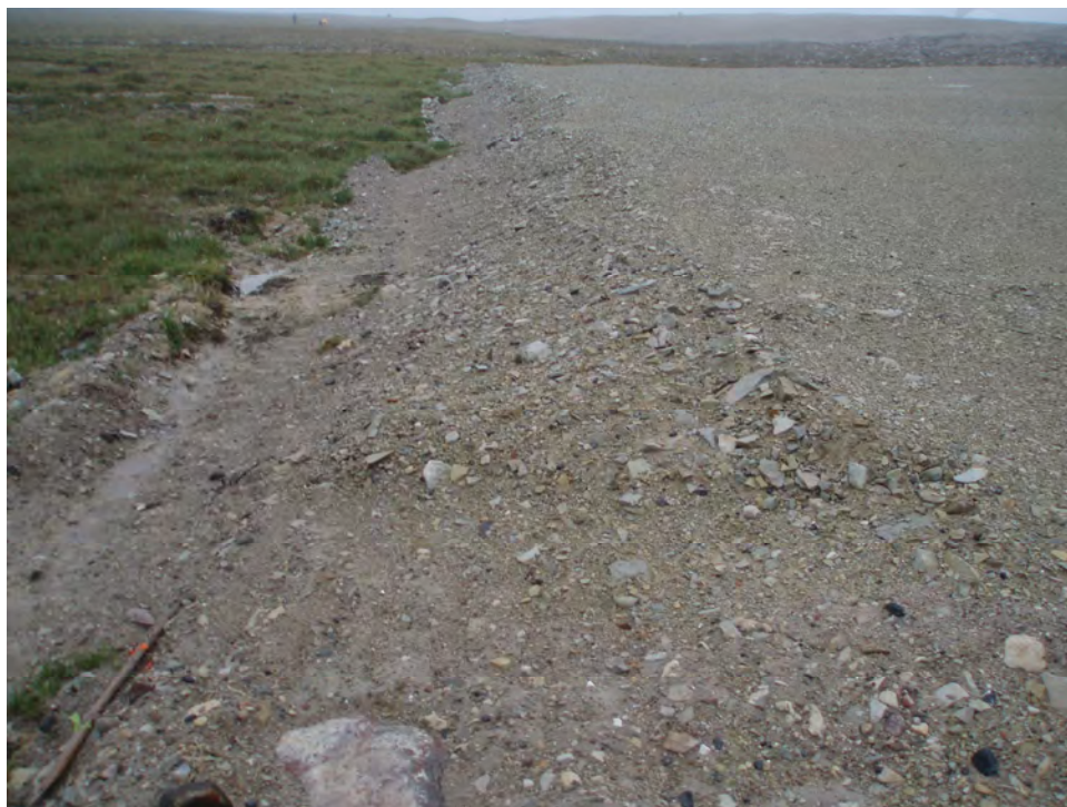
Photograph 4. Erosion on Side Slope, Looking Approximately NW, Erosion on Entire Side Slope ↑
