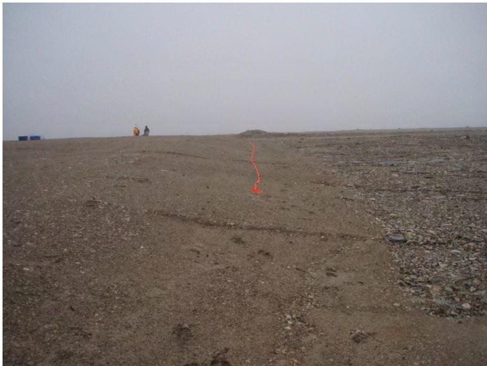
Photograph 2. Settlement on Side Slope (0.1 to 0.2 m), Looking Approximately NE Towards Shepherd Bay ↑
