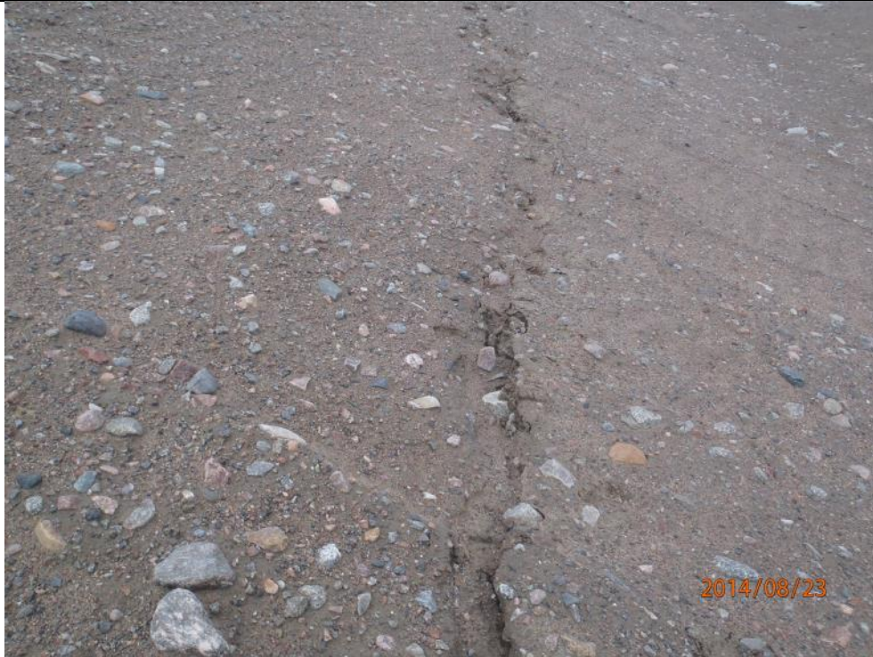
Erosion on southeast berm. Viewpoint 57 (Figure A-2; Appendix A). Photograph reference P8230057. Direction photo taken: NA
