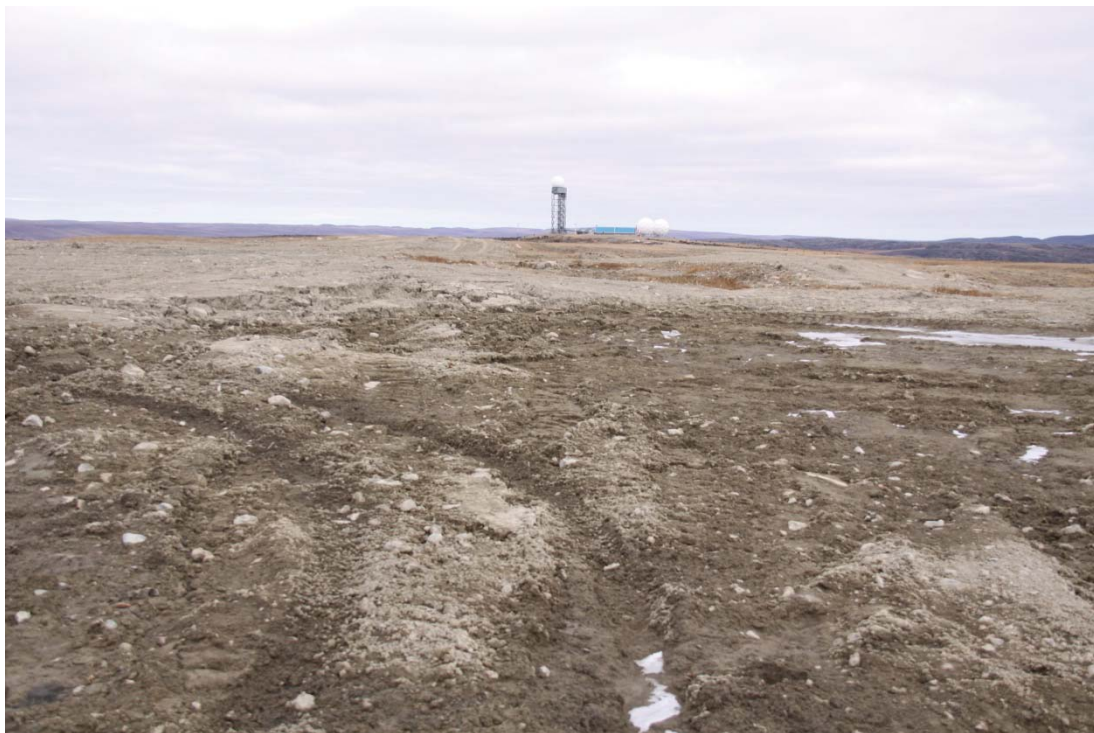
Photograph 10. After: Excavation complete; reshaped to match surrounding terrain. ↑
