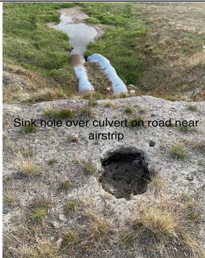
Photograph 2: Sinkhole on Road between Airstrip and Site
