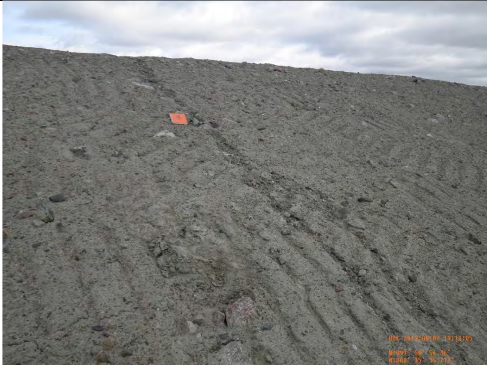
Cracking on West slope of SSDF. Viewpoint 53 (Figure A-2; Appendix A). Photograph reference RIMG0053. Direction photo taken: E
