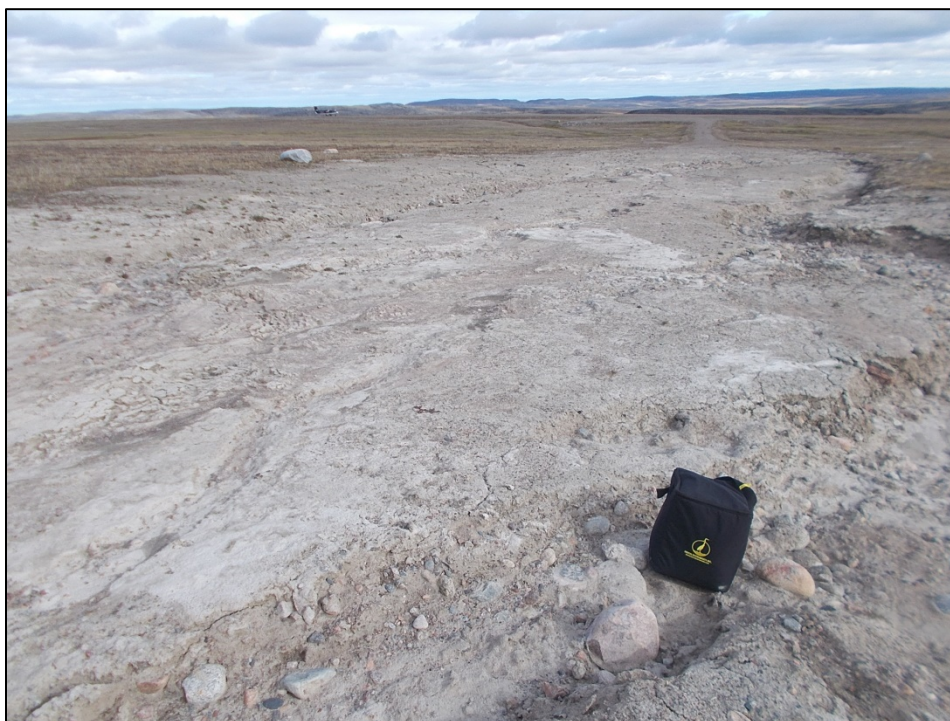
Photograph 20. Erosion on access road, facing E
