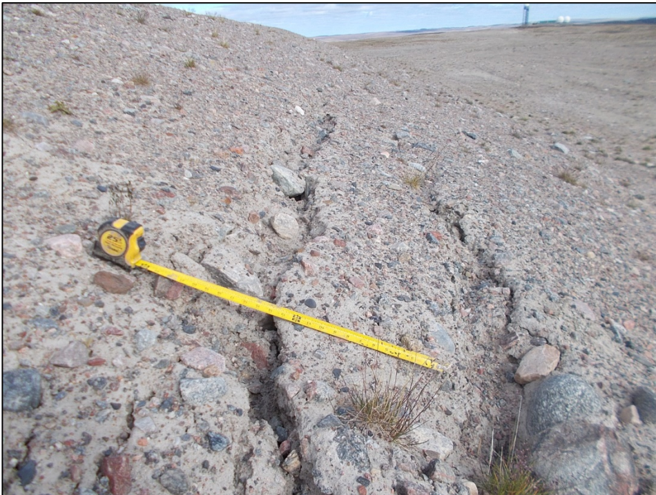
Photograph 6. Cracking on SE flank, facing NE
