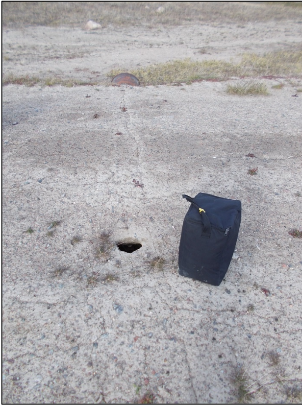
Photograph 21. Siksik burrows and cracking from culvert on access road
