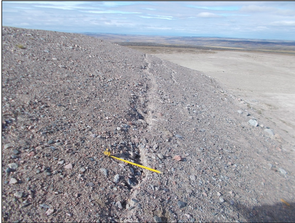
Photograph 3. Cracking on NE flank, facing NW
