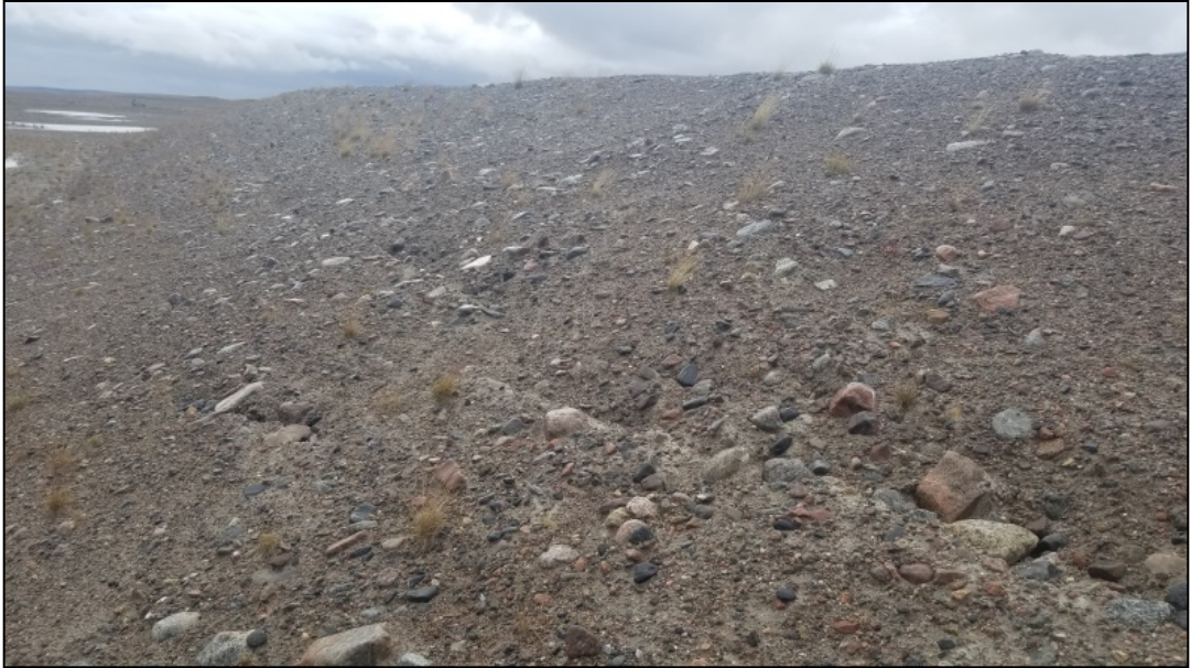
Photo 7: Frost crack looking south on the eastern side of the landfill.
