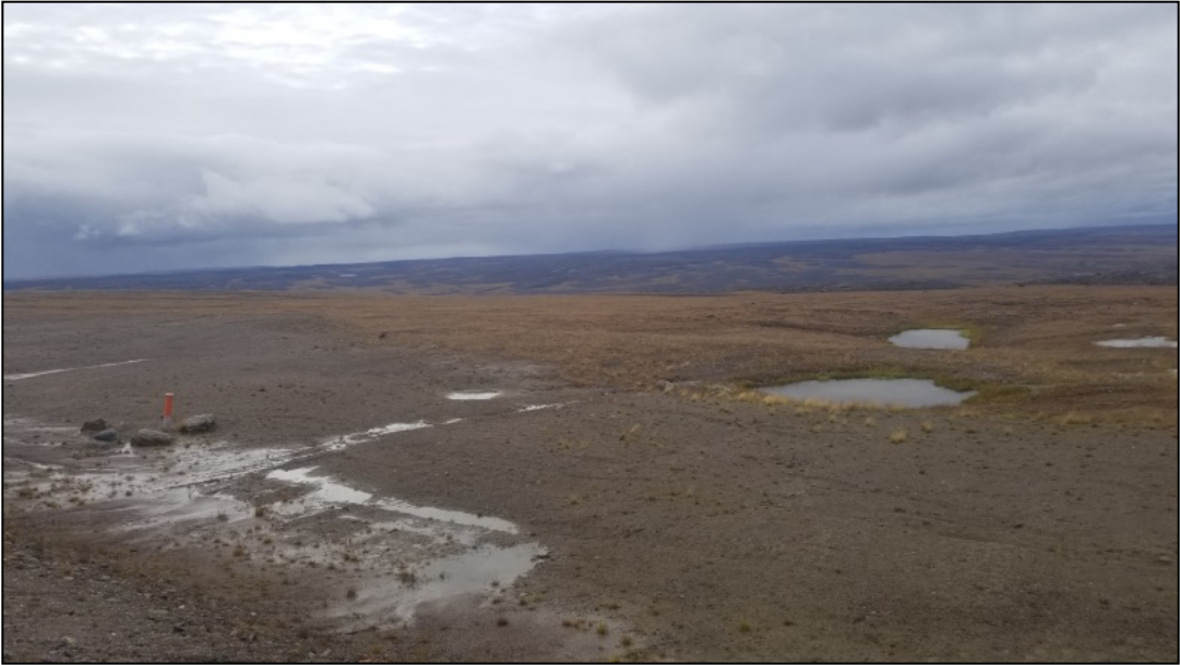
Photo 1: Drainage channel located near NE corner of landfill.
