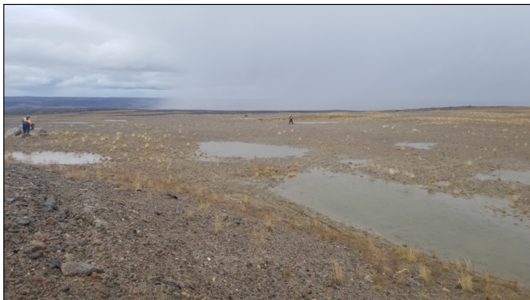
Photo 6: Frost crack on the southern side of the landfill and standing water.
