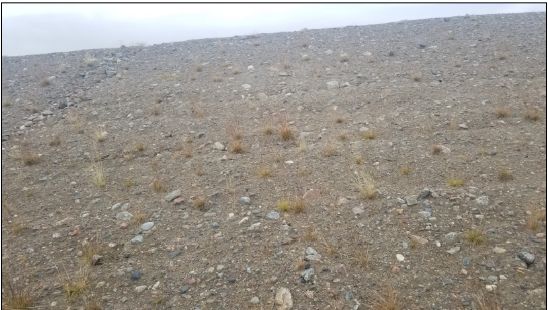
Photo 2: Erosion on NE corner of landfill.
