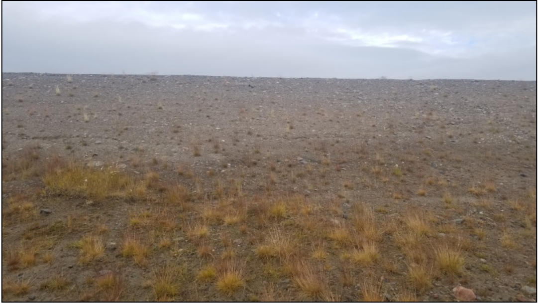
Photo 9: Frost crack on the western side of the landfill looking east.
