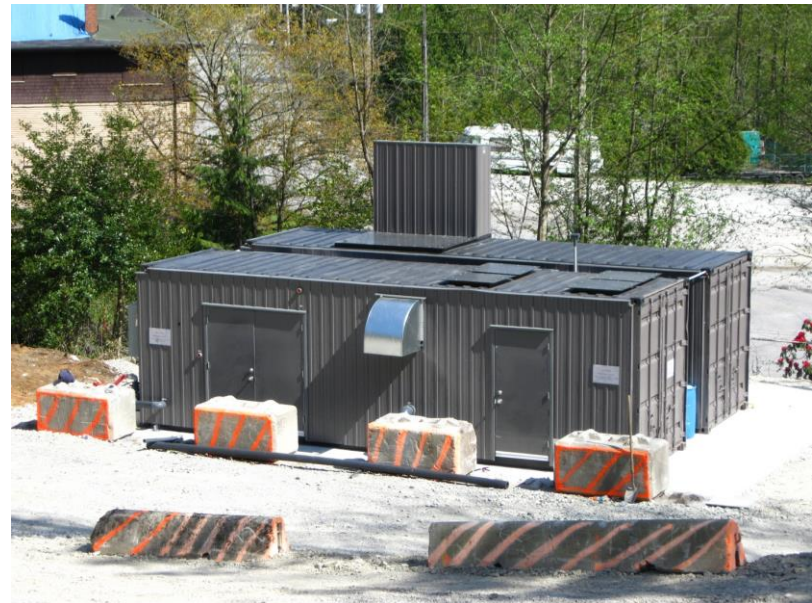
Project - Imperial Oil (IOCO) Site: Iron removal system 100 m 3 /day Contact: Linda Eastcott
