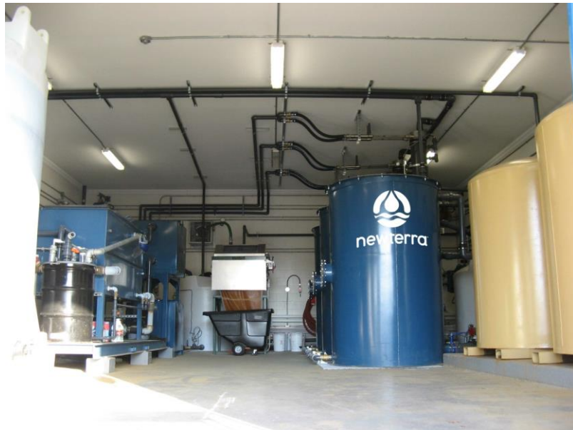
Project - City of Belleville: Iron removal system 800 m 3 /day.
