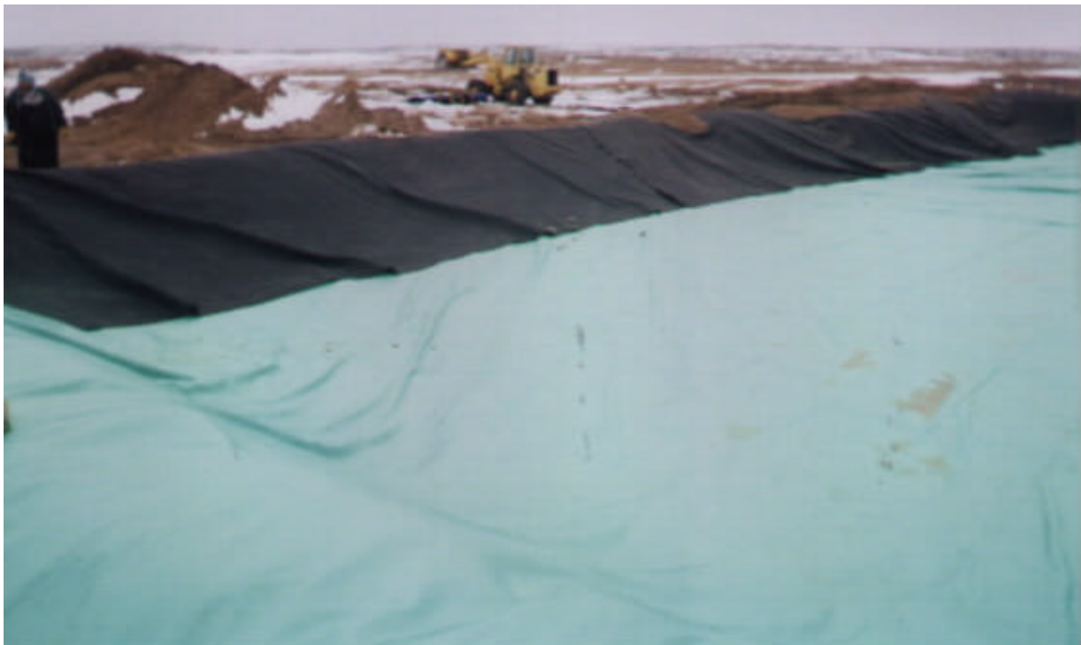
Photo 4: Installation of geotextile on top of geomembrane.
