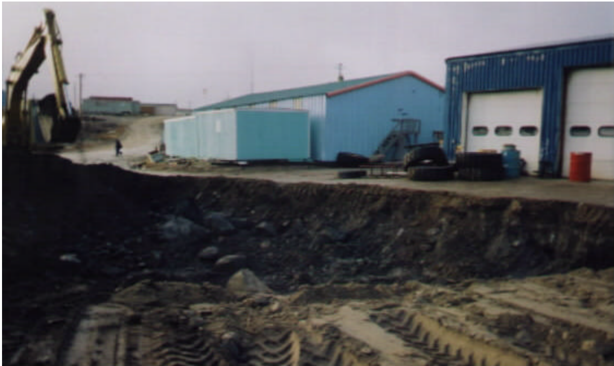
Photo 6: Excavation of contaminated material in front of garage.
