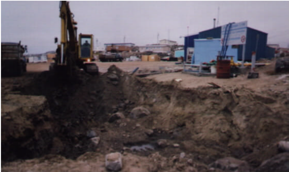
Photo 5: Excavation of contaminated material near fuel pipeline.
