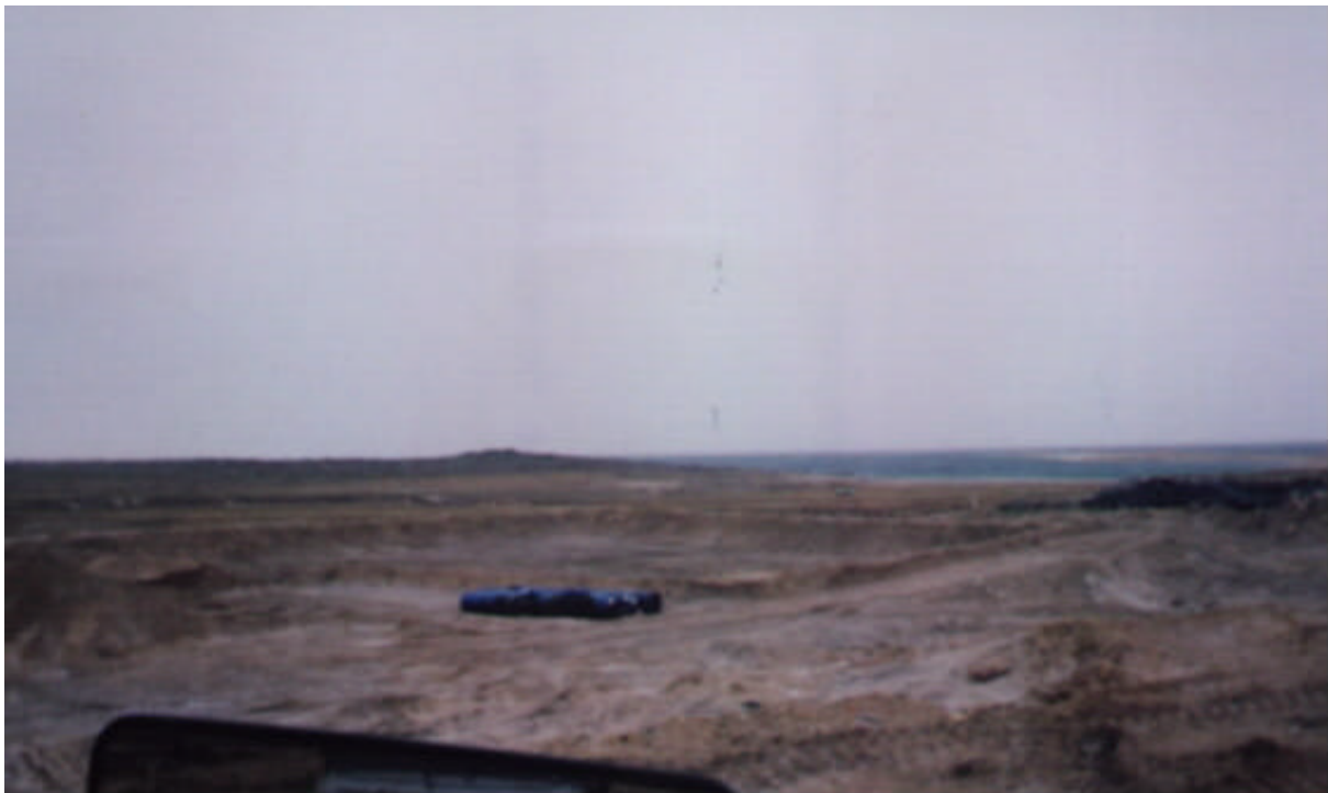
Photo 2: Berm construction complete and ready for liner.
