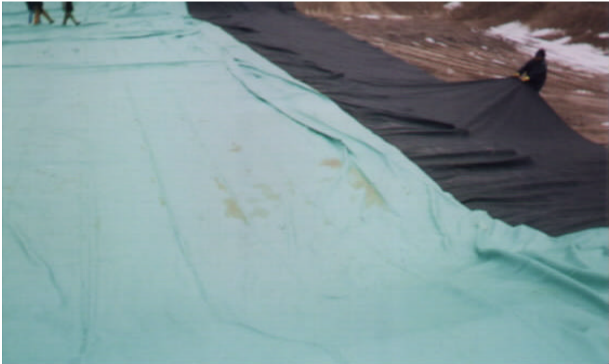
Photo 3: Installation of geomembrane on geotextile.
