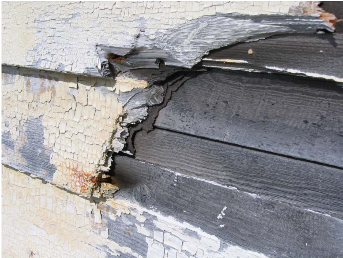
Close-up of Lead based pain on Winch Shed
