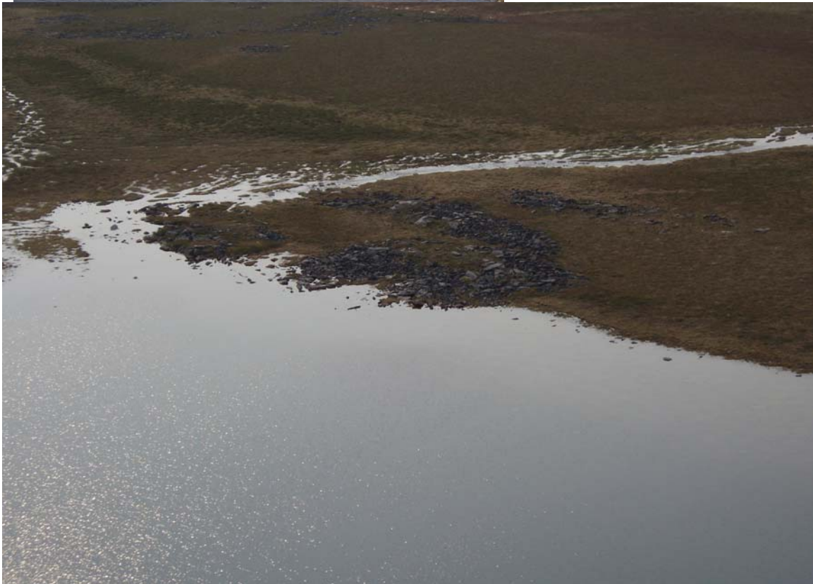
July 2 - Aerial view of crossing R12 looking south
