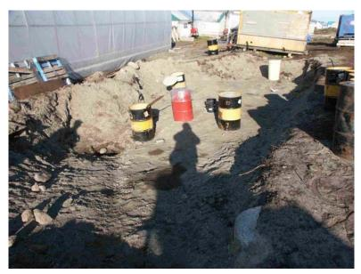
initiated. The spill had ponded between two natural berms which are probably the result of old lake shorelines in the unconsolidated beach sediments. The berms trapped the ponded product and enabled crews to recover half of the spilled material, or about 4,000 litres. The remainder had infiltrated the pore spaces in the sand and migrated into the sediments and down slope.
