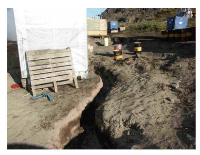
After the second phase was series completed. а monitoring pits were excavated in the main removal pit and fuel absorbent materials within them. These pits extend 1 metre below the excavation level of the main removal pit. The pits monitored are continuously and the fuel absorbent materials are replaced every 24 hours with material. The fresh soiled materials are sealed in 205 litre drums for shipment and disposal.
