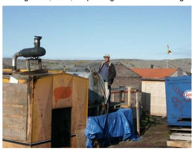
one of the storage tanks. During process of filling the generator tank, the employee left fuel flowing into the generator tank while attending to other matters in camp as there were a lot of aircraft shuttling into the site at the dock. The employee forgot that they had left the fuel flowing and it spilled approximately 3 hours, releasing approximately 8,000 litres of product onto vegetation covered beach deposits (sand, gravel, silt and clay).
