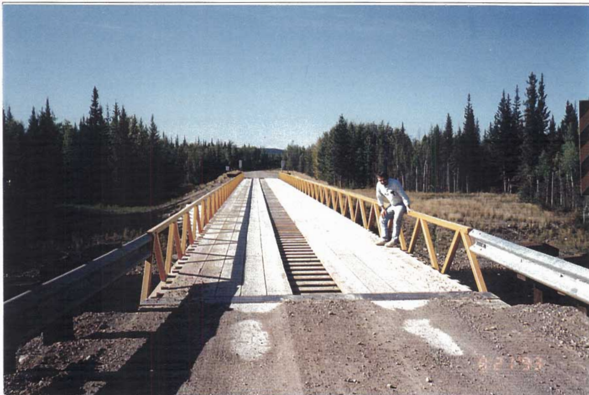
Mackenzie Winter Road km 828, Devils Canyon Bridge. Single lane timber deck
