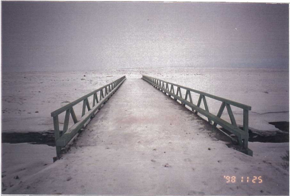
Baker Lake, Prince River Bridge, Span 48 m. Single lane timber deck
