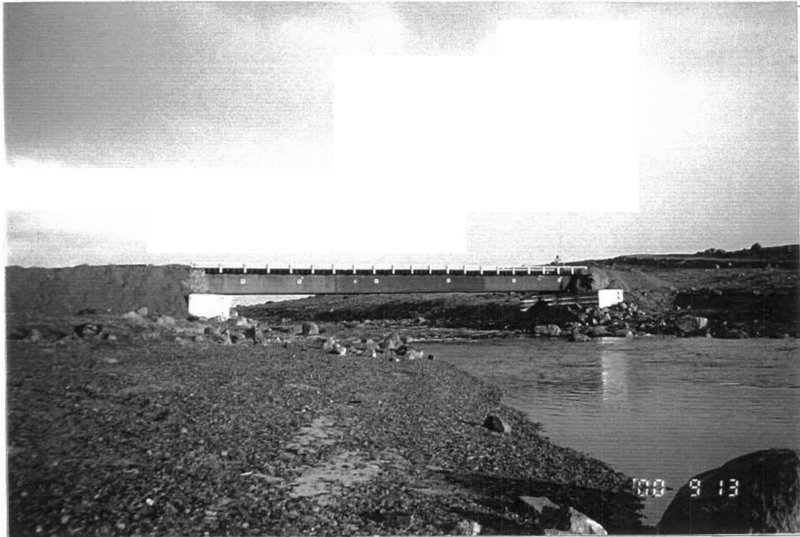
General View of the Bridge
