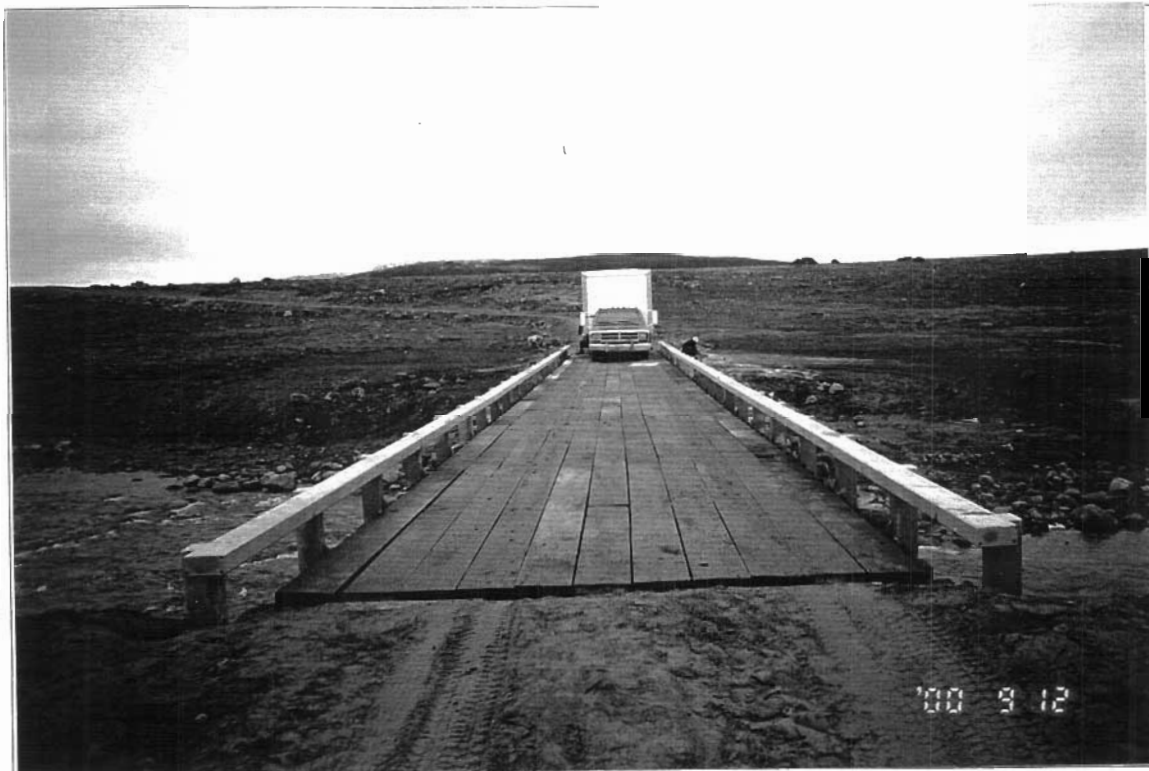
View of the Bridge Deck.
