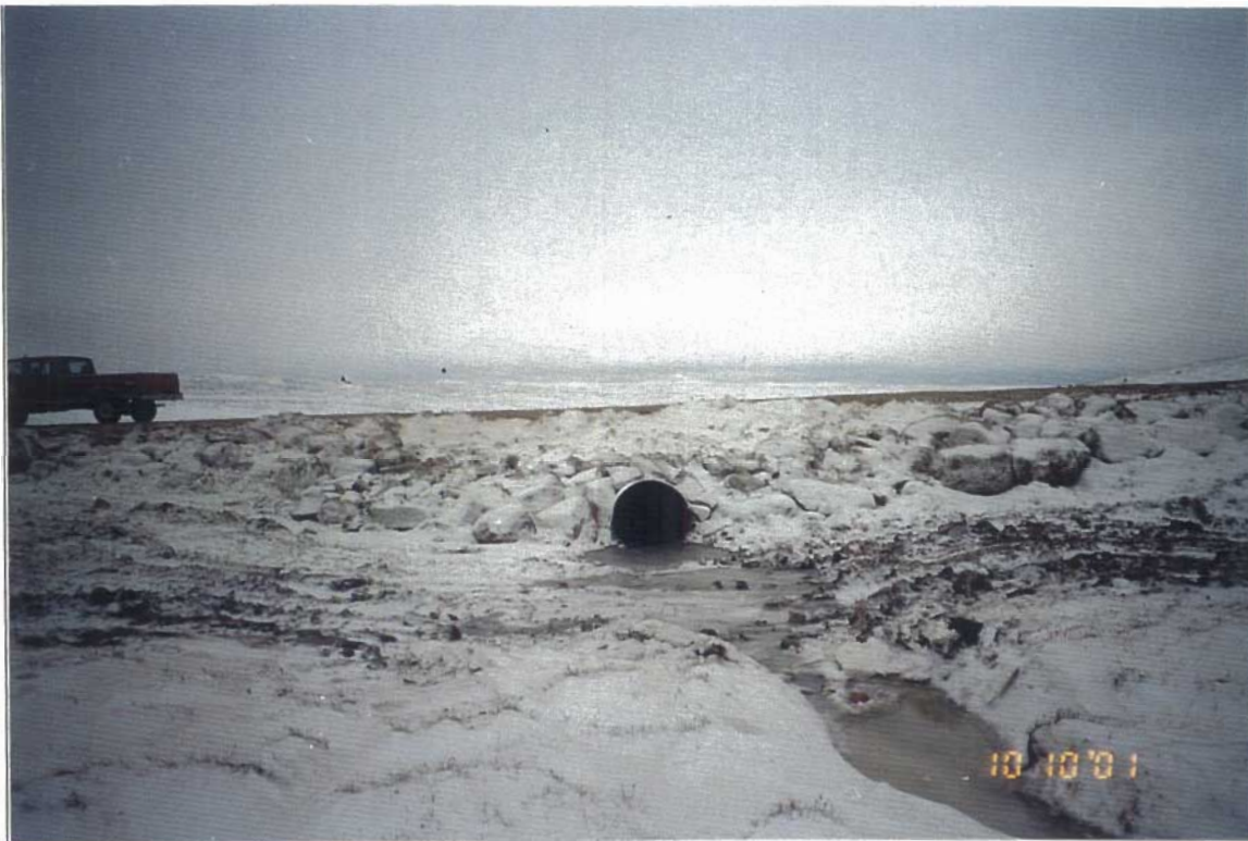
View of inlet with riprap protection. Temporary creek crossing in close plan.
