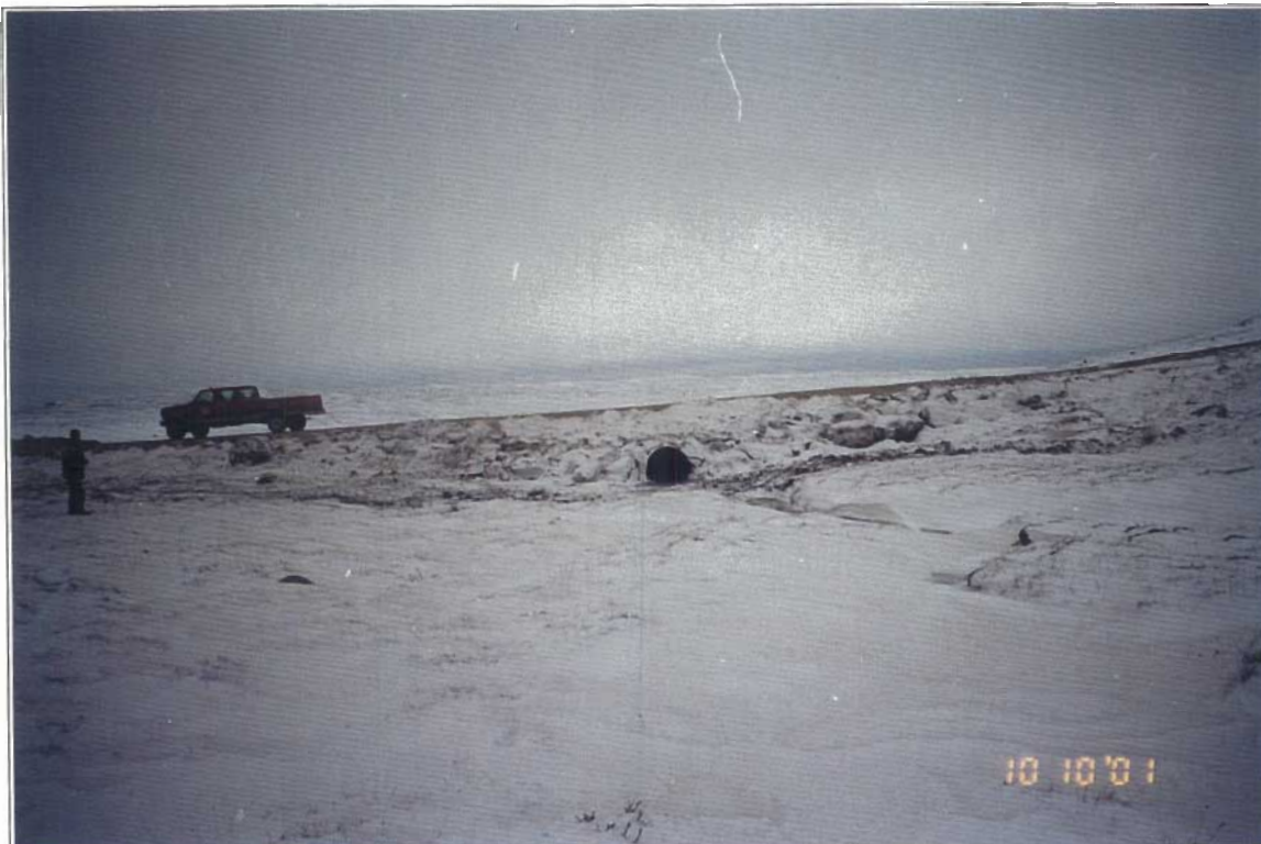
View of inlet with riprap protection.
