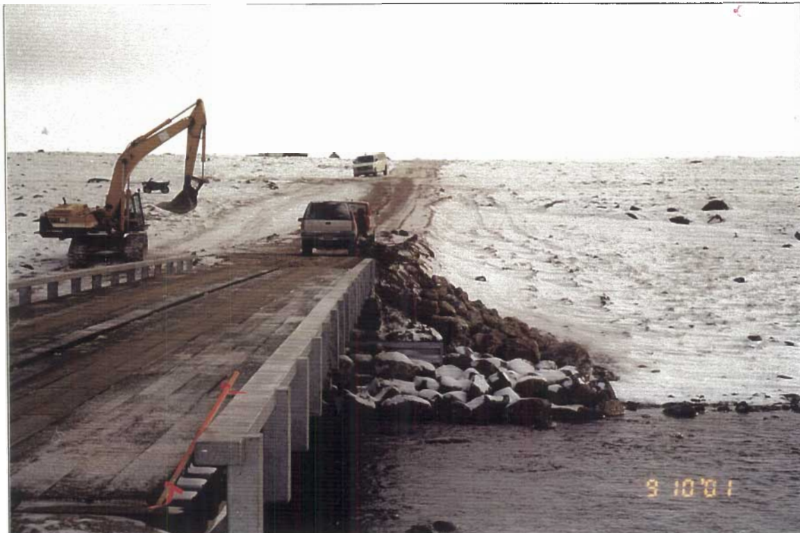
View of east abutment upstream riprap arrangement
