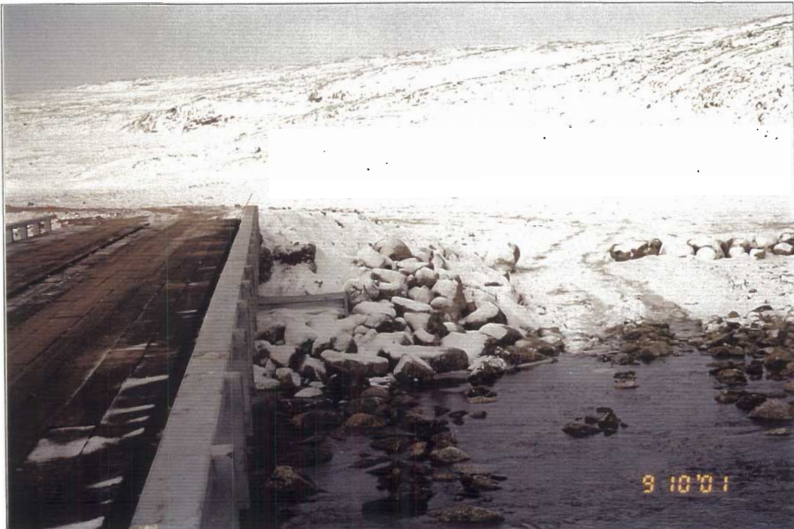
Riprap on west down stream corner of bridge.
