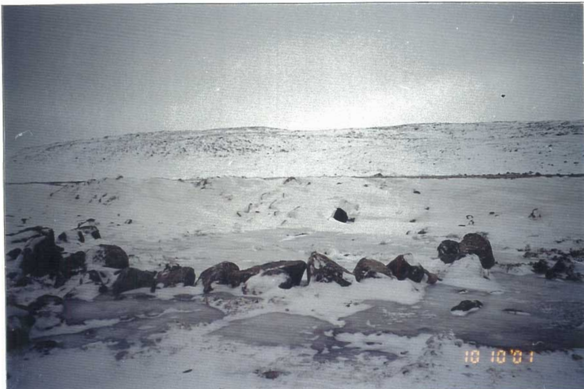
View of outlet with riprap protection and reflective dyke forming a pool.
