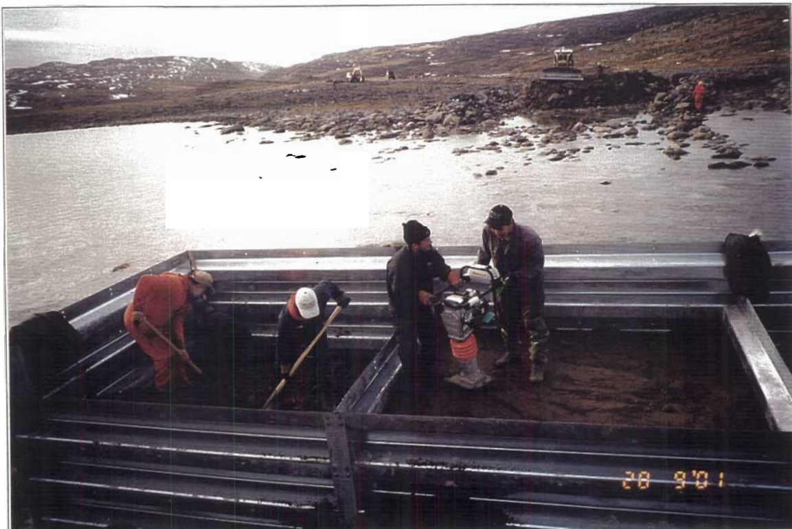
Construction of Binwall on east abutment
