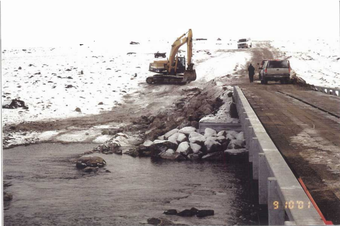
View of east abutment downstream riprap arrangement and ford
