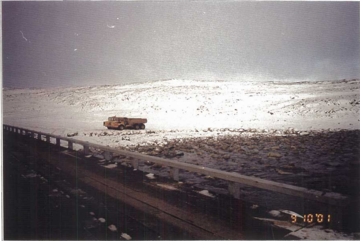
Spur dyke and riprap protection along the high water mark on east downstream abutment.
