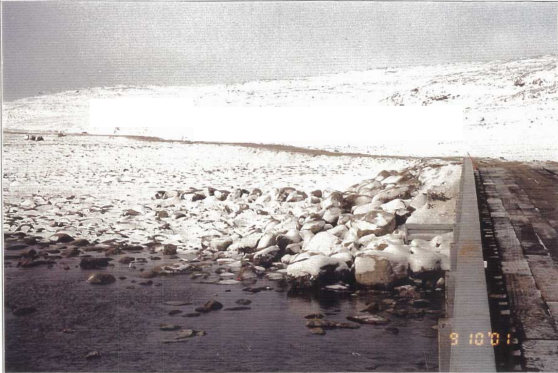
Riprap on west-up stream corner of bridge.
