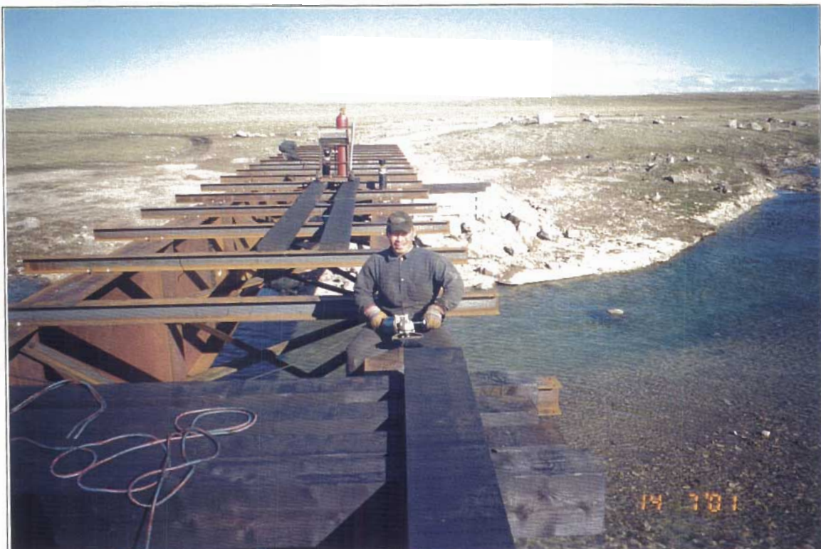
Local bridge crew working on deck installation
