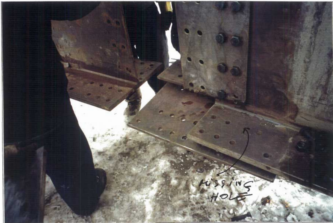
Girder splice detail.
