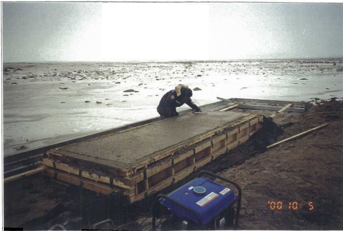
Concrete bearing seat installed on top of the binwall abutment
