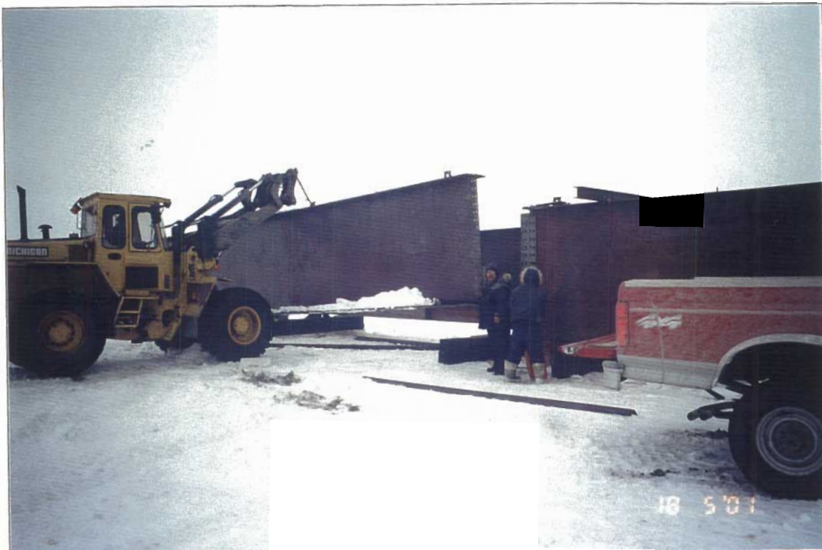
Transportation and assembly of bridge girders using local loader.
