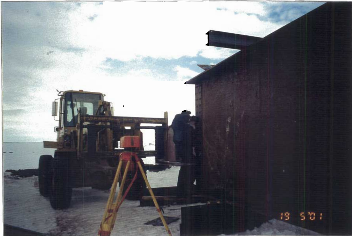
Bridge crew member working on girder splice
