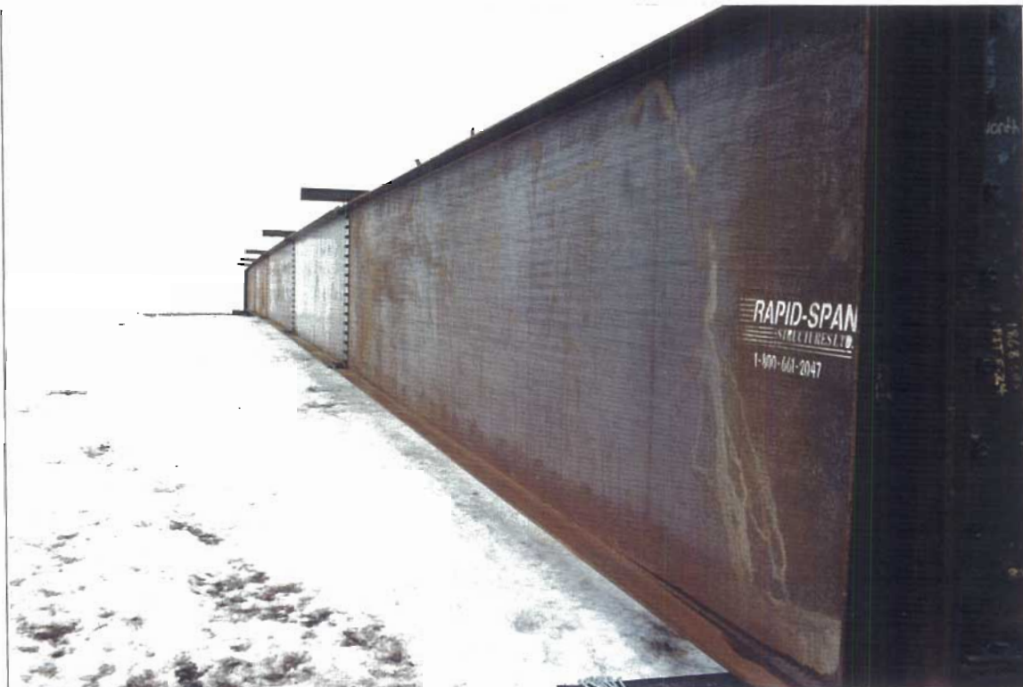
April 2001. Bridge girders installed on 3.5 m high snow berm.
