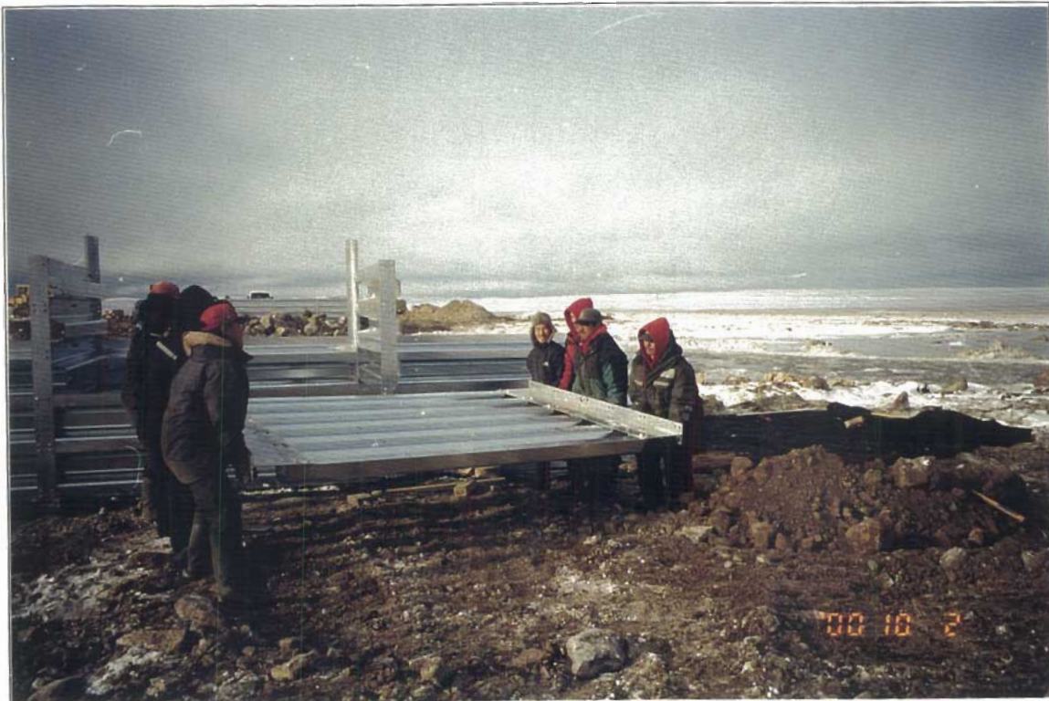
Local bridge crew carrying 900 lb. Pre-assembled binwall panel
