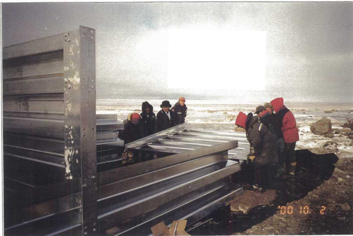
Local bridge crew assembling a binwall abutment
