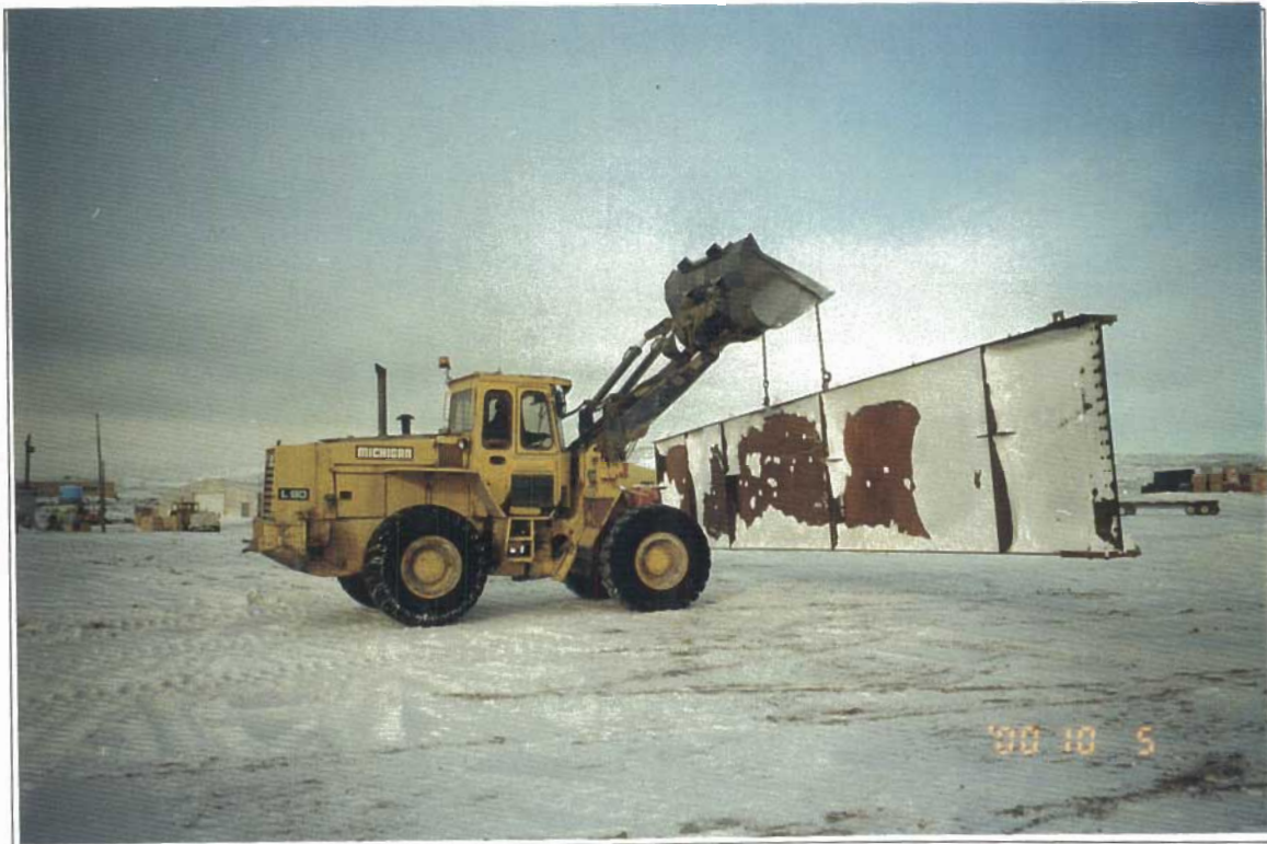
Local equipment transporting 12,000 lb. Bridge girder section
