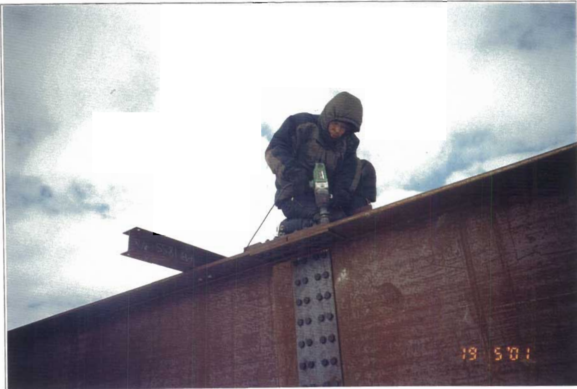
Bridge crew member working on girder splice.
