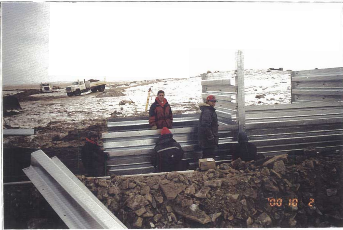
Local bridge crew assembling a binwall abutment
