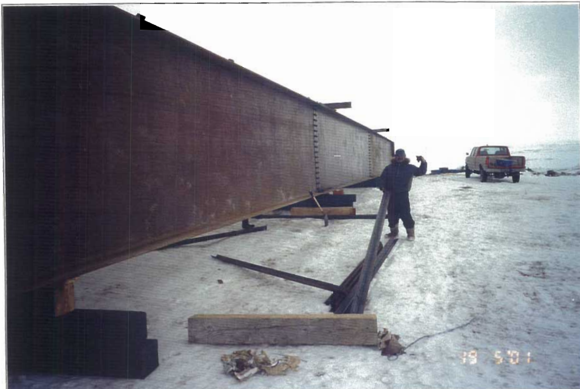
Side view of partially installed bridge. A 3.5 m high and 20.0 m wide berm constructed of snow was used as working platform
