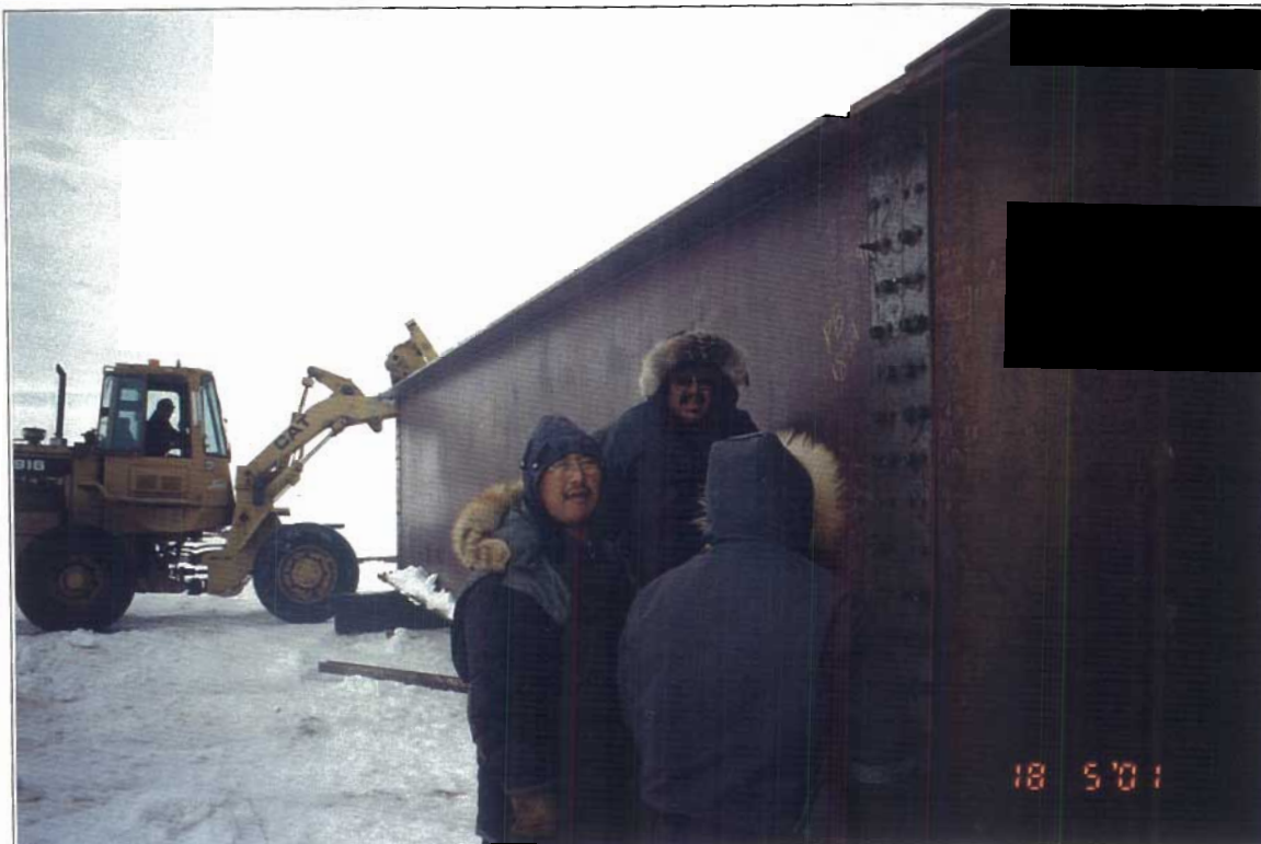
Local crew working on girder splice.
