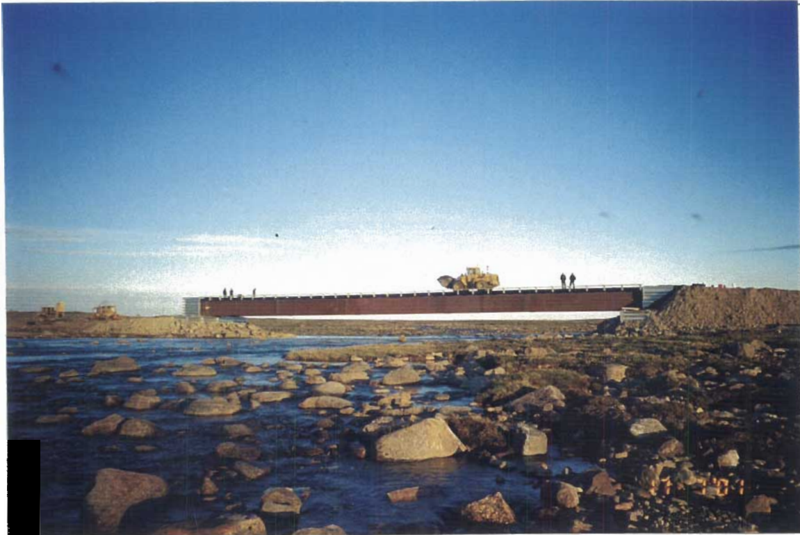
First vehicle travel on the bridge to deliver gravel for the east binwall backfill
