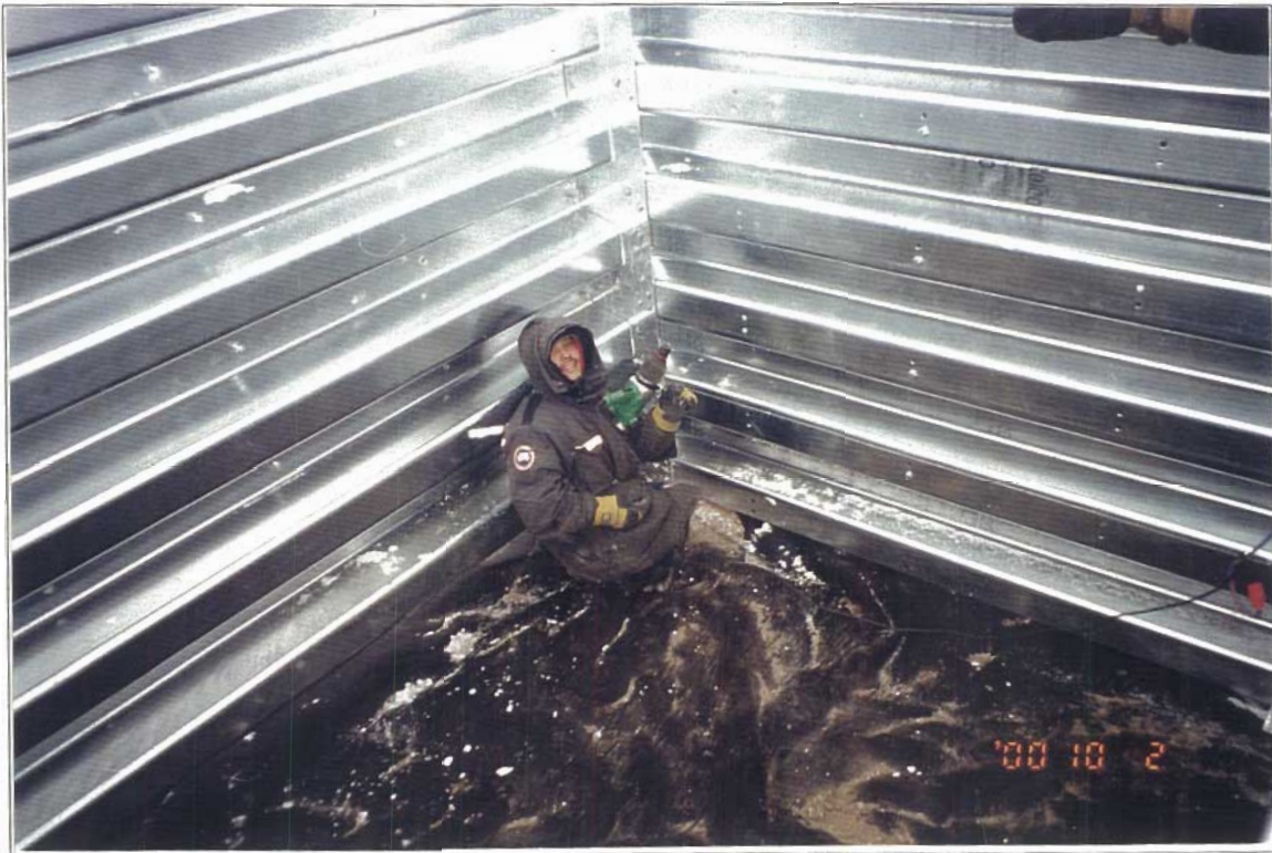
Local crew member working on binwall assembly
