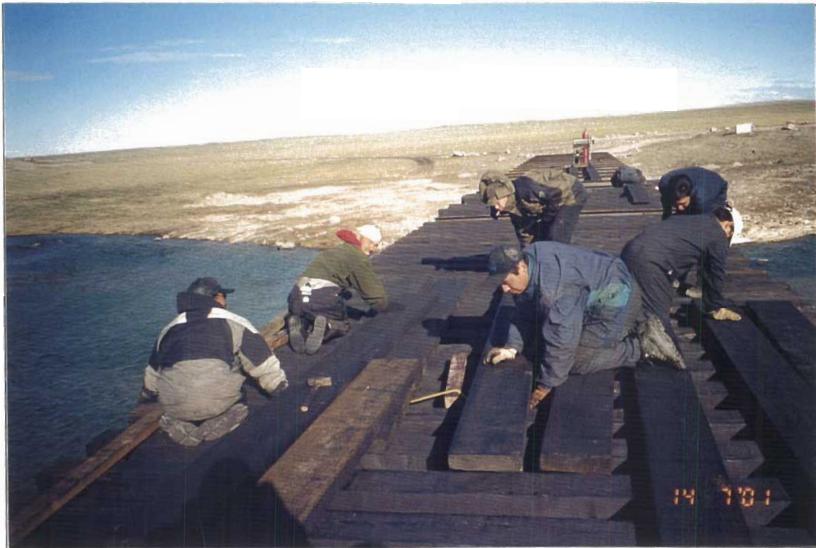
Local bridge crew working on deck installation
