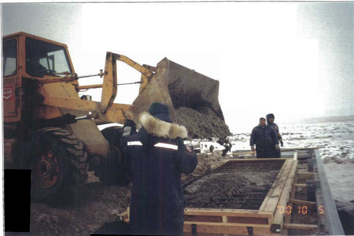
Local crew placing concrete
