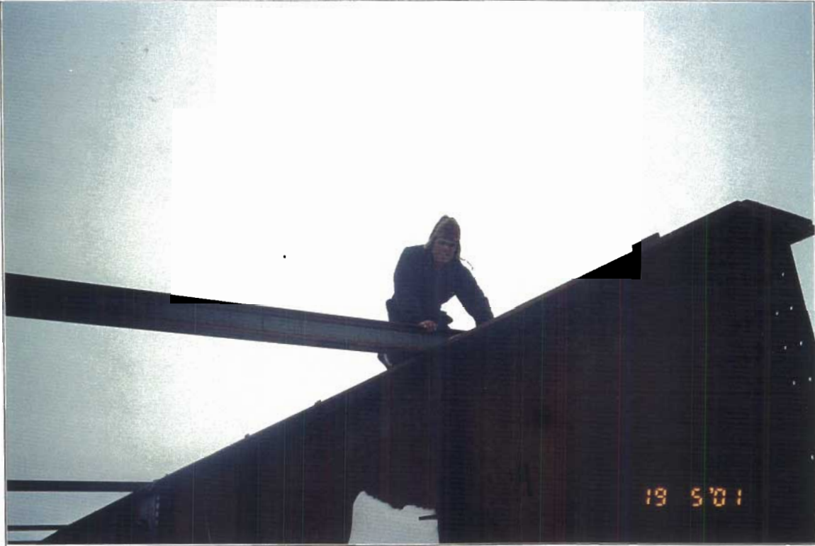
Bridge crew member installing floor beam
