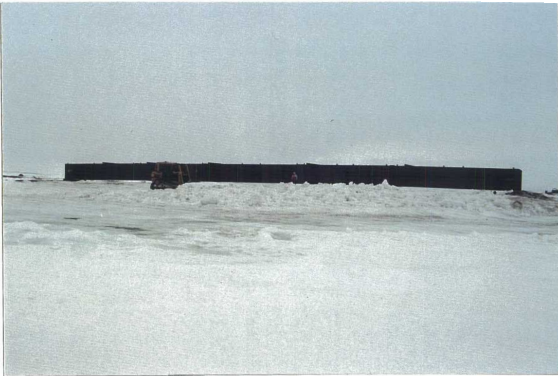
Elevation of bridge girders installed on 3.5 m high snow berm
