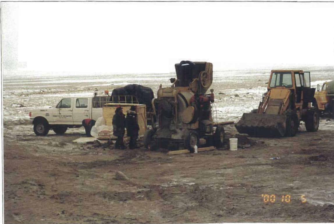
Concrete production plant, owned and operated by the local Koomiut Co-op produced the concrete for the bridge bearing seats.
