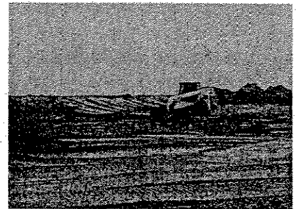
Establishing a sand bed on liner using a tracked skid steer.
