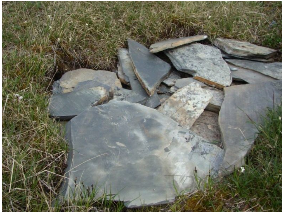
Photograph 4: Sump location. Sump has not been restored properly; material used for backfill is too large for proper contouring and compaction.
