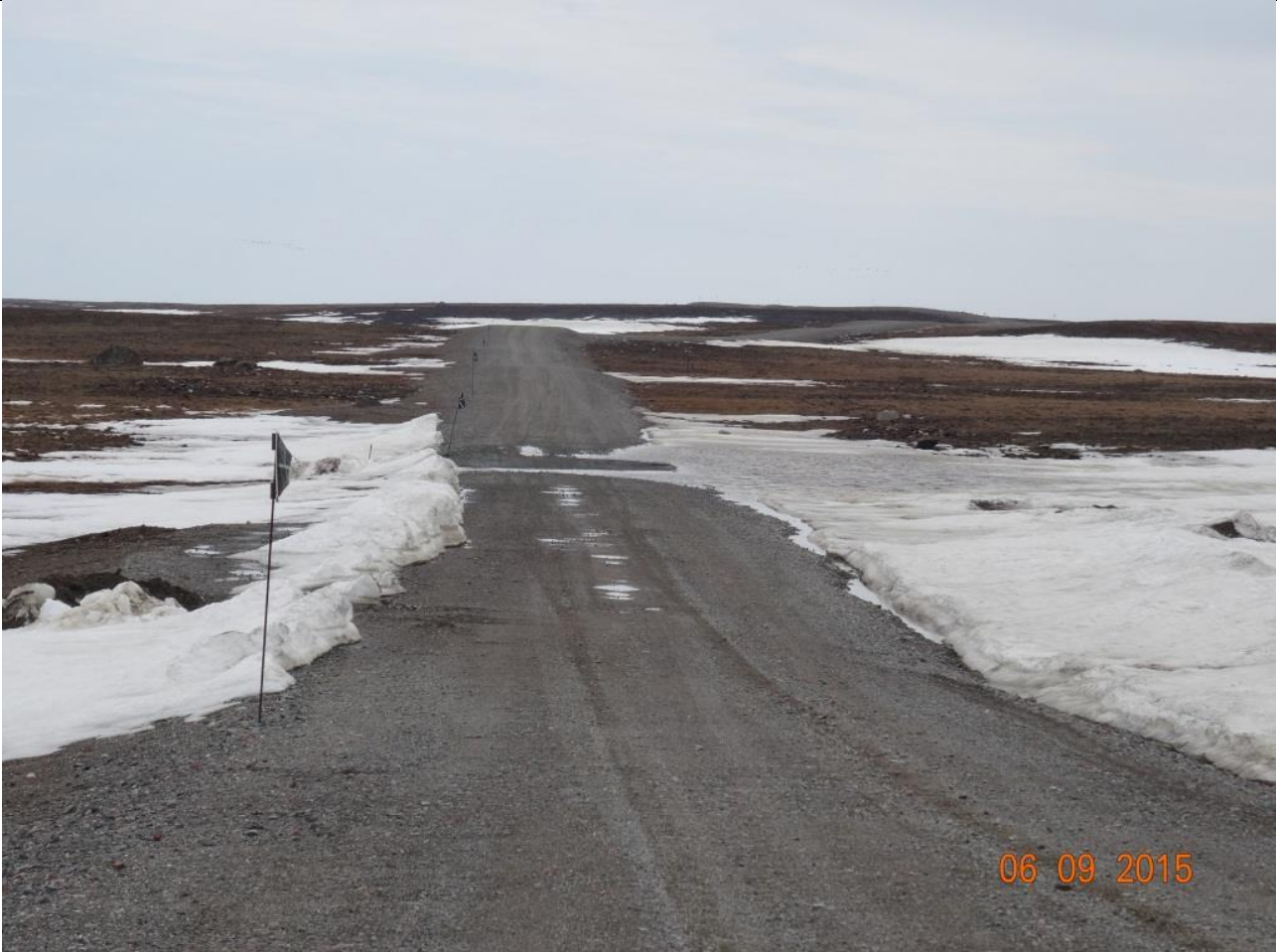
Description: Water over topping Road- Agnico Eagle’s All weather Access Road to Meliadine Project
