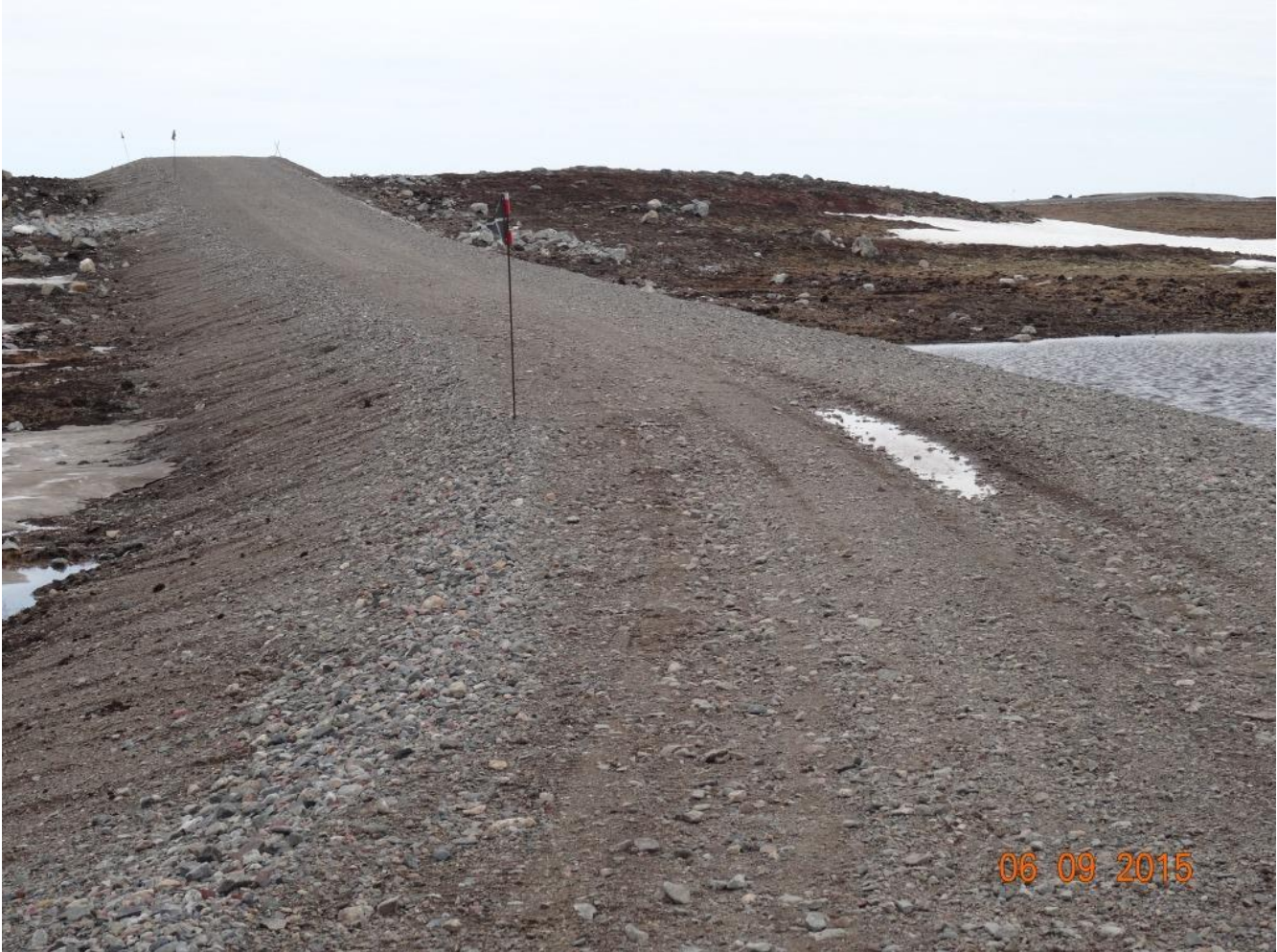
Description: Ponded water- Agnico Eagle’s All weather Access Road to Meliadine Project
