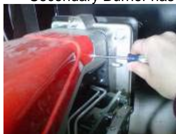
Secondary Burner has 4 screws (2 on each side)
