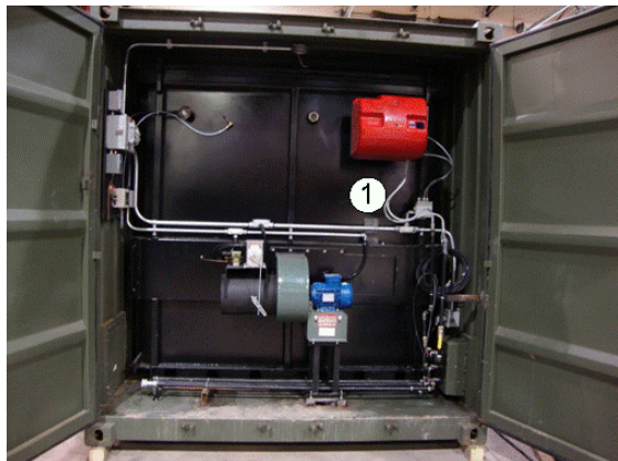
Primary Chamber Burner Flexible lines (Item # 1 Above)
