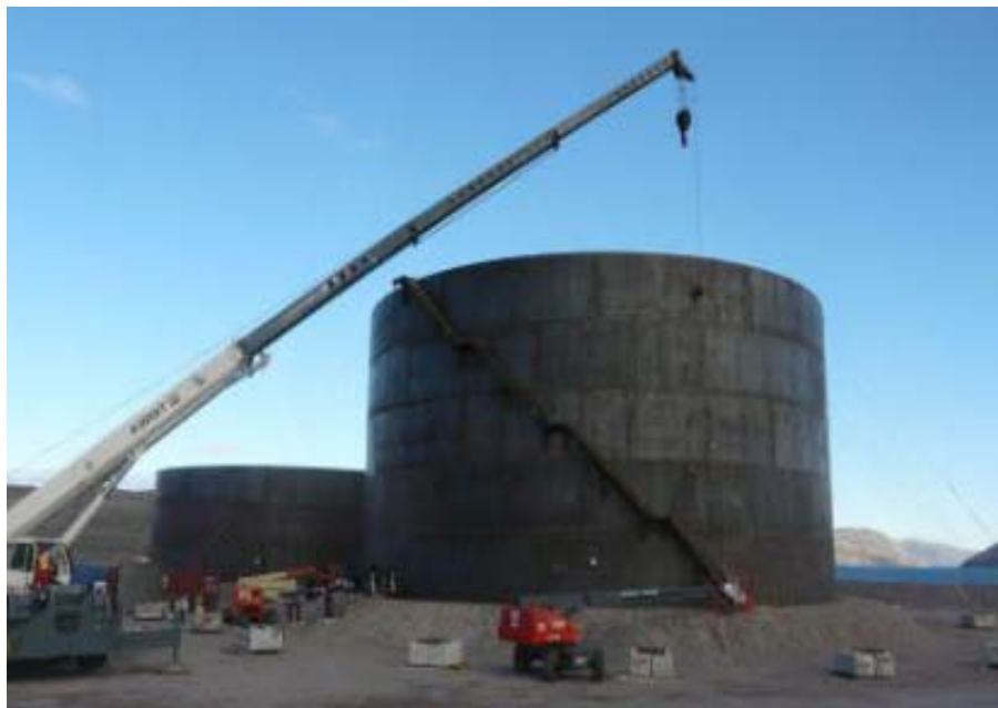
PHOTO 14 Installing roof on Tank #1 August 2013
