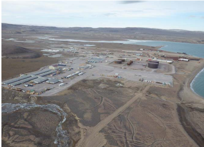
PHOTO 4 Aerial View – Infrastructure Layout September 2013
