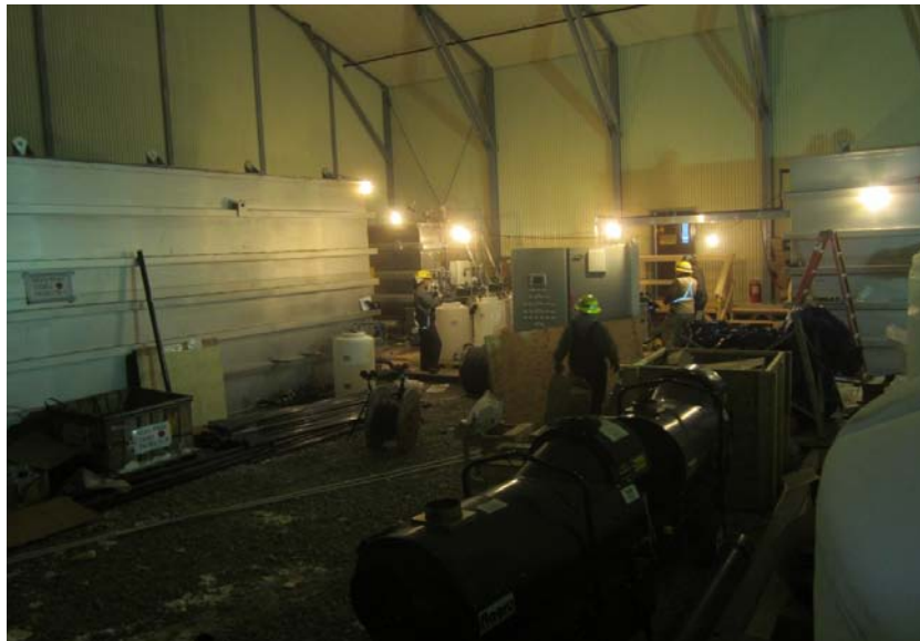
PHOTO 13 Water (Fresh) Treatment System Installation November 2013
