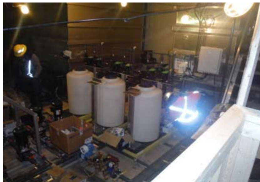
PHOTO 14 Water Building - Mechanical Installation November 2013
