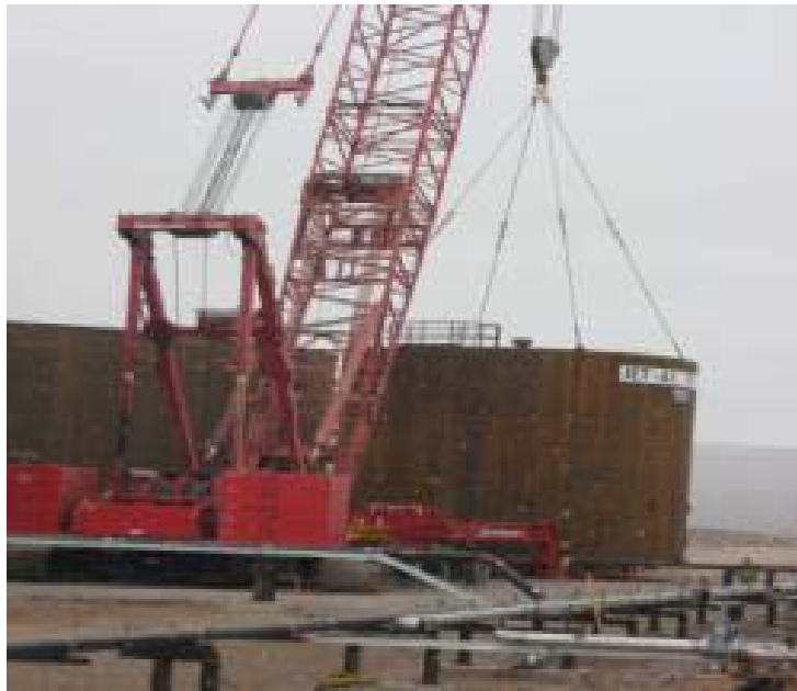
PHOTO 13 300 Ton crane placing 1 st 750,000L Jet A Tank August 2013
