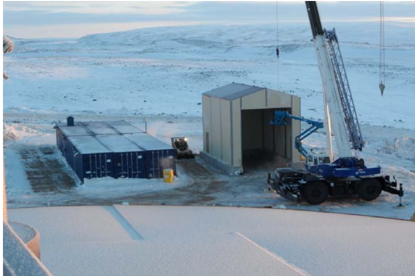
PHOTO 11 Wastewater Treatment Facility utilizing MBR Technology and adjacent Sewage Truck Building
