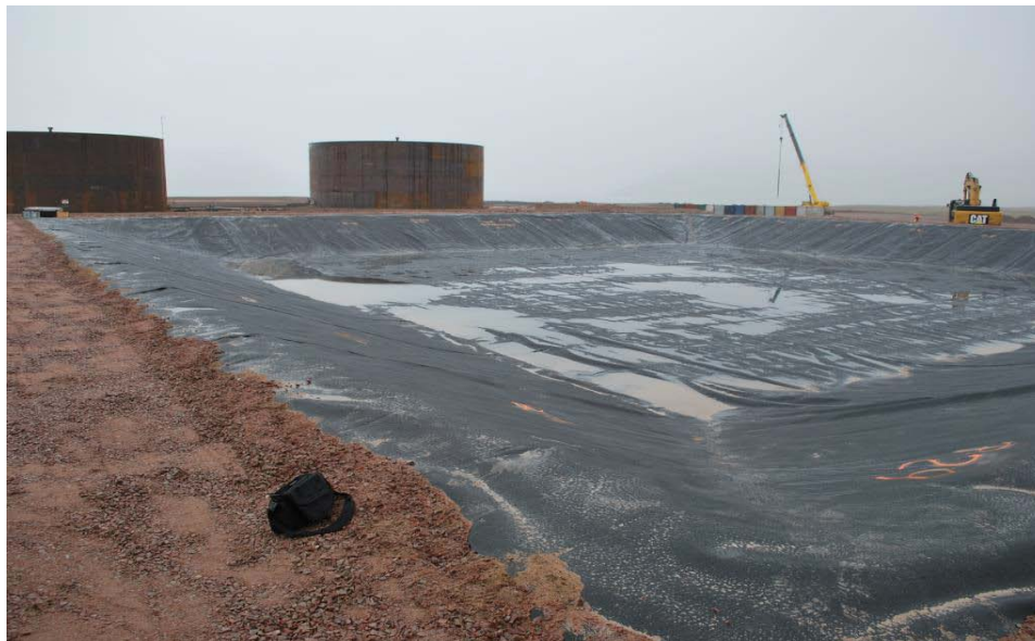
PHOTO 8 Polishing Waste Stabilization Pond (PWSP) engineered containment structure arctic liner installation July 2013
