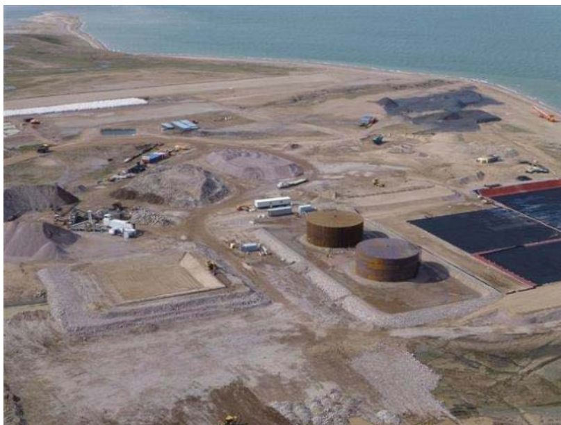
Figure 4: During – Grading of Final Layer
