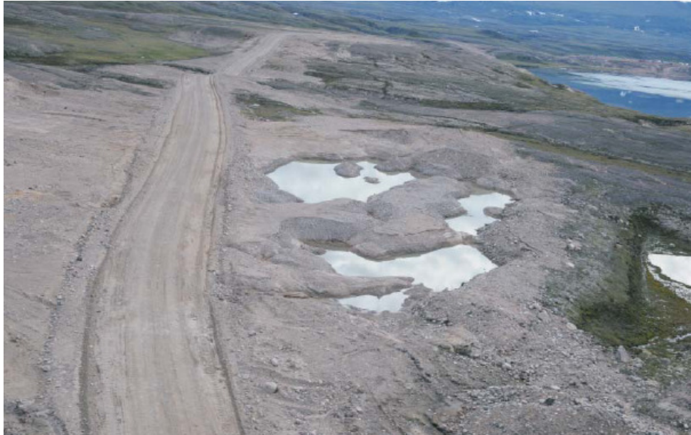
Photo 3-1: Km97 Borrow Source: Typical depression formation from thaw of massive ice
