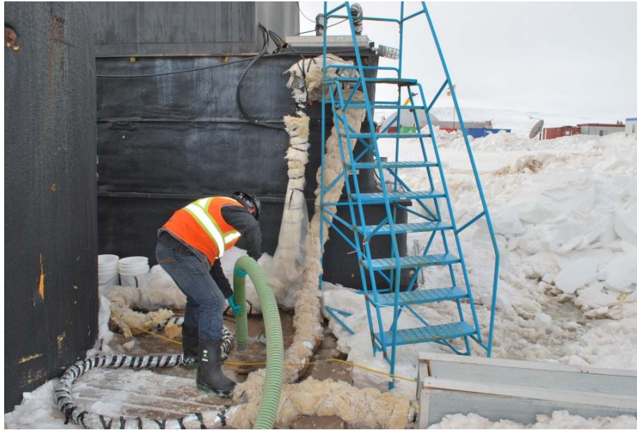
Photo 2 – Collecting Spilled Effluent with Vacuum Truck
