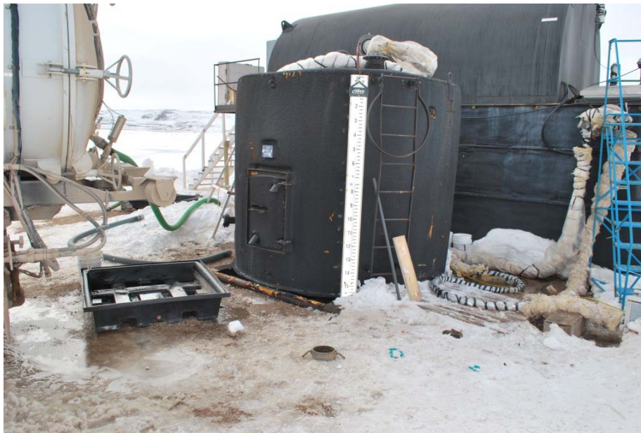
Photo 1 – Milne RBC after Access Port was Capped
