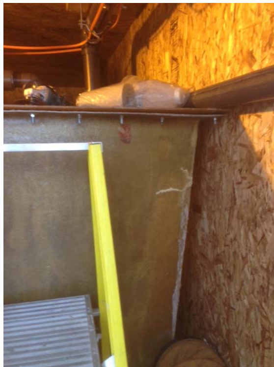
13 10 29 Tank Breach
