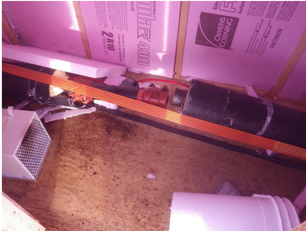
Photo 3 Failed Pressure Fit Coupler
