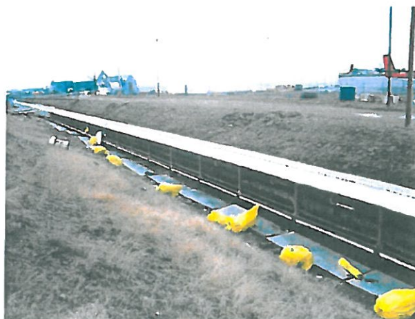
Photo 6: Glove-bagging asbestos for cutting of pipe
