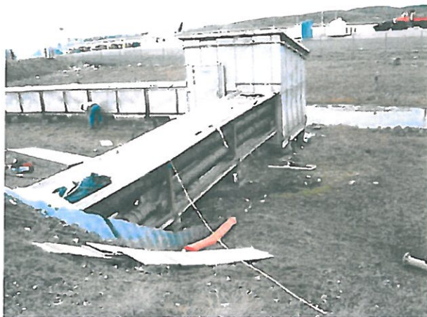
Photo 1: Starting point for asbestos abatement
