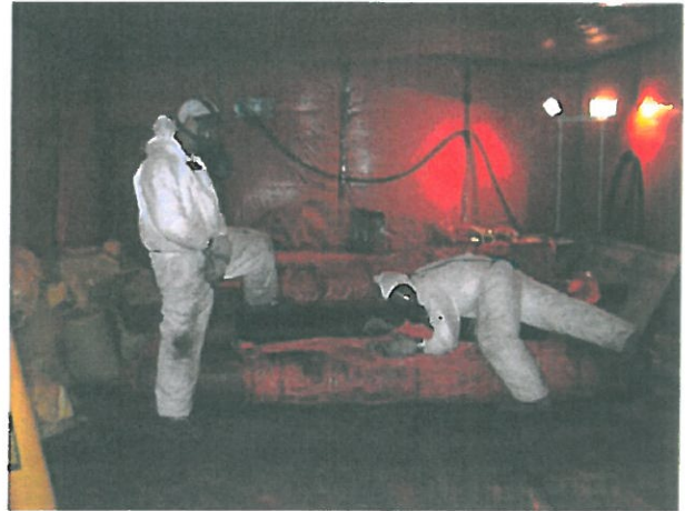
Photo 10: Asbestos pipe being decommissioned
