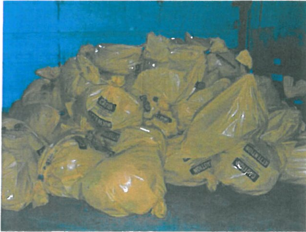
Photo 9: Asbestos to be loaded in Sea Can
