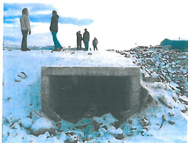
Photo 12: End of demolition under Apron1
