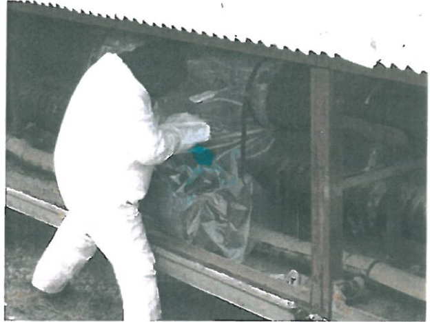
Photo 8: Asbestos pipe glove-bagging abatement
