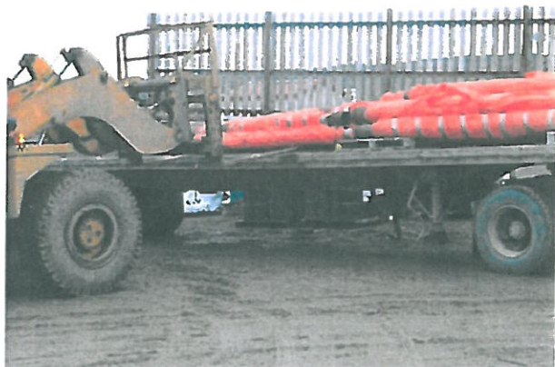
Photo 5: Loading wrapped asbestos pipe
