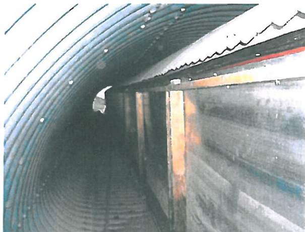
Photo 4: Utilidor running through tunnel
