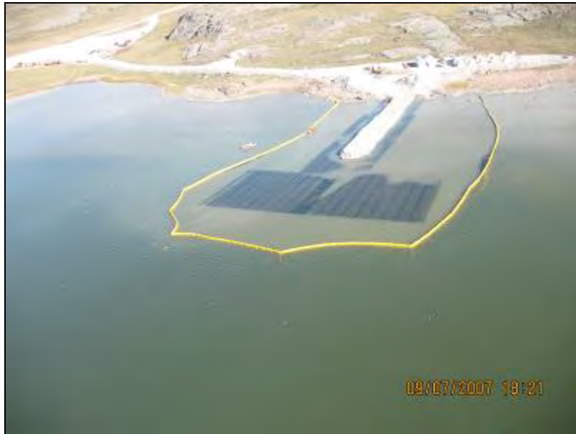
Photo 2.15 Aerial View of Geo-Grid Placement Before Fill Placement, 9 July 2007.
