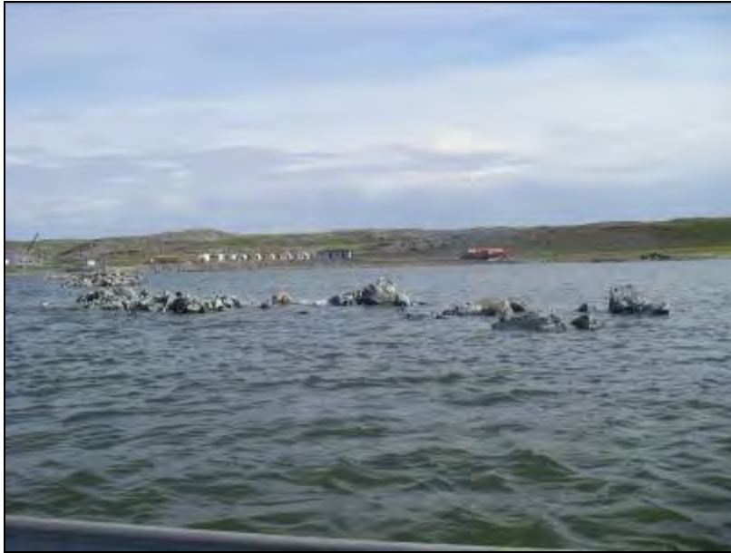
Photo 2.26 Looking South-East at Compensation Structures, 13 July 2008. Note the Structures are Settling as the Ice Below Them Melts.
