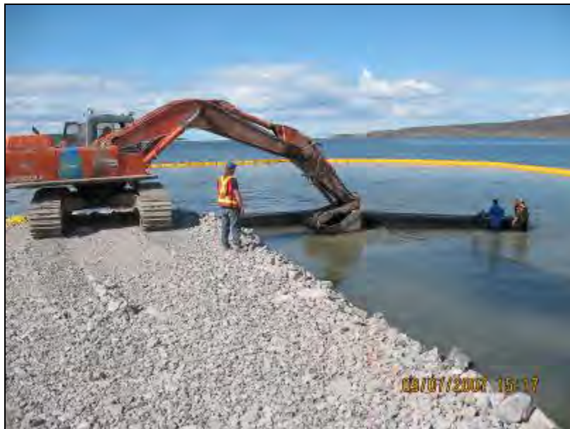
Photo 2.14 Facing North-East on Jetty as Geo-Grid is Rolled Out, 9 July 2007.
