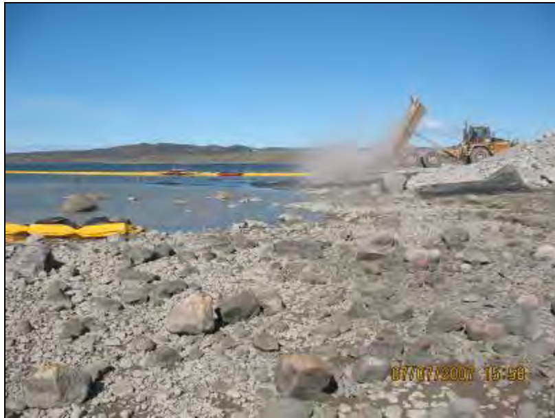
Photo 2.7 Facing East as Rock Truck Unloads Material onto the Root of the Jetty, 7 July 2007.
