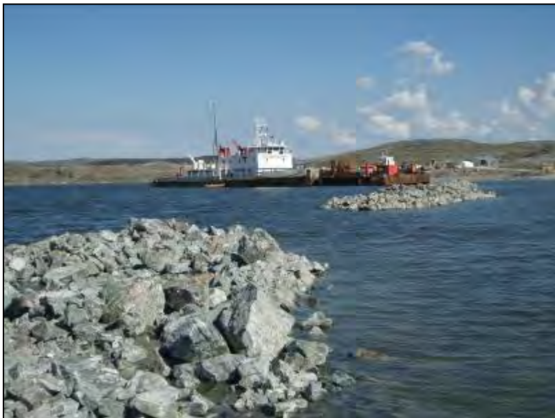
Photo 2.25 Facing South-East Along the Compensation Shoals, Showing Shoals Resting on the Frozen Substrate, 11 July 2008 (Photo: Matt Kawei, HBML).
