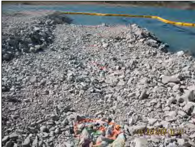
Photo 2.19 Facing West Along the Jetty Head - Note the Slope Grading and the Settlement Beacons, 16 July 2007.
