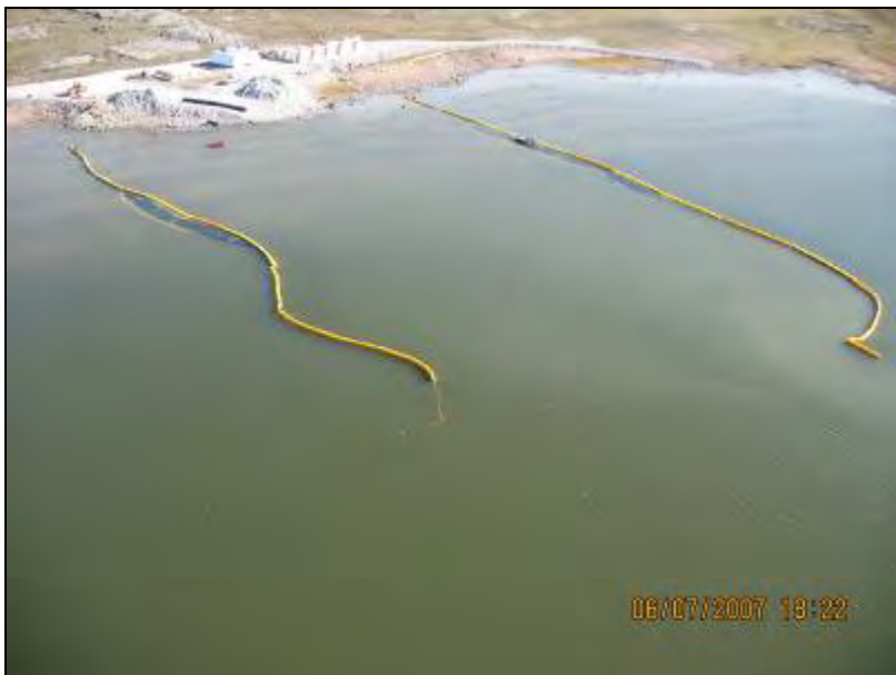
Photo 2.4 Aerial View of Silt Curtain Deployment in Roberts Bay, 6 July 2007.
