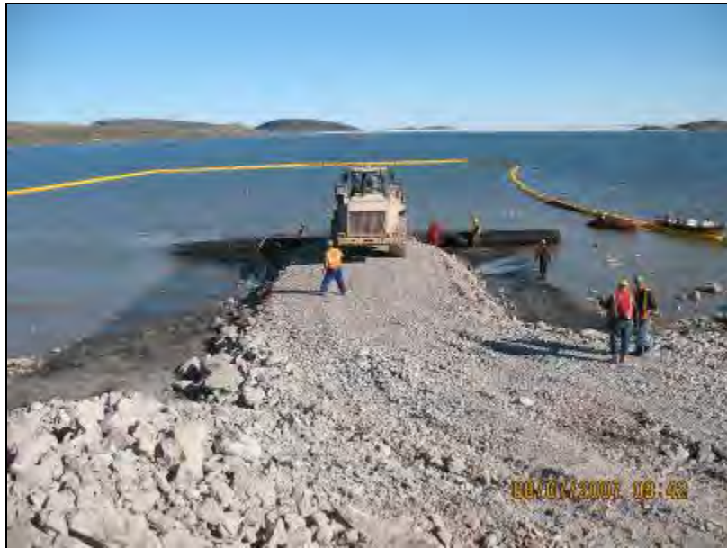
Photo 2.11 Facing North During Geo-Grid Placement, 8 July 2007.
