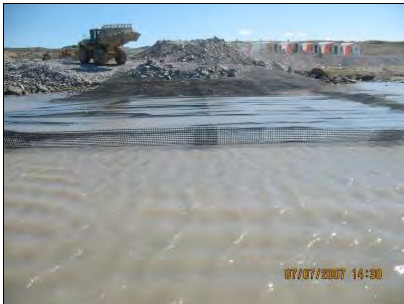
Photo 2.6 Facing South in Roberts Bay During Initial Fill Placement for the Jetty Construction, 7 July 2007.
