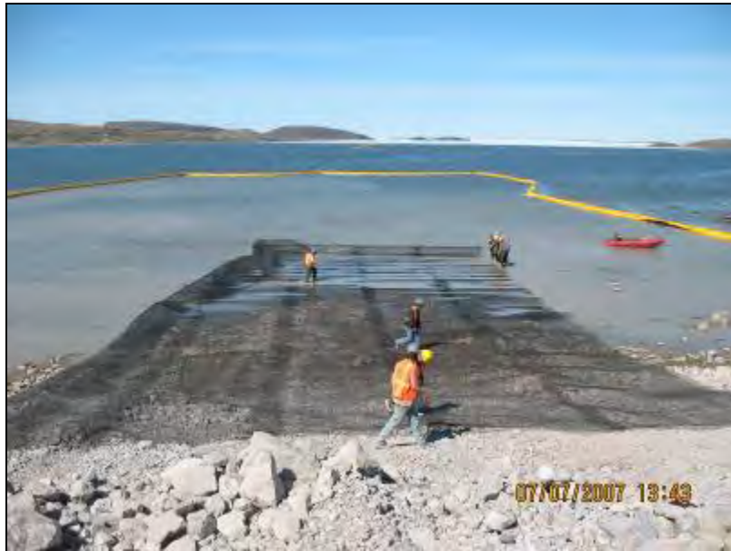
Photo 2.5 Facing North at the Jetty Location During Geo-Grid Placement in Roberts Bay, 7 July 2007. Note Silt Curtain Surrounding the In-Water Construction Area.
