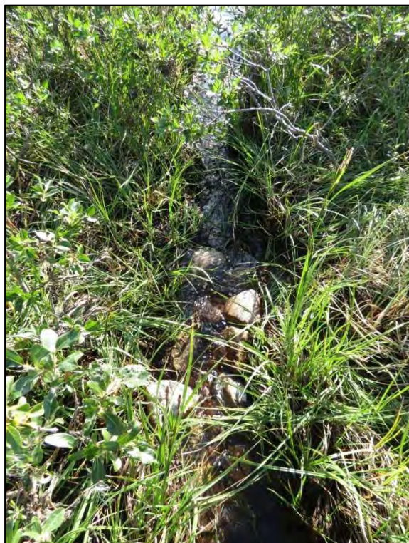
Plate 2.2-5. A small rock weir installed in the new channel will provide additional fish habitat.
