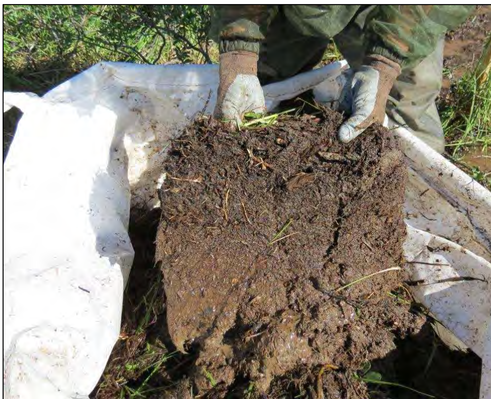
Plate 2.2-1. Dense root masses needed to be cut using hand saws, were loaded into mega bags, and removed from sites.
