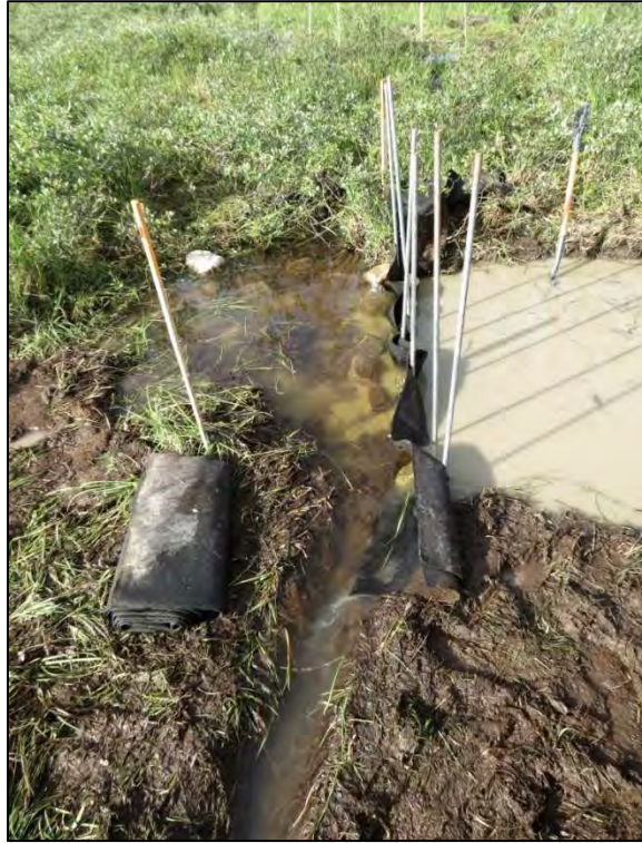
Plate 2.2-2. The work area (right) was effectively isolated from the flowing channel (left) using silt fences. This kept downstream turbidity within acceptable levels.
