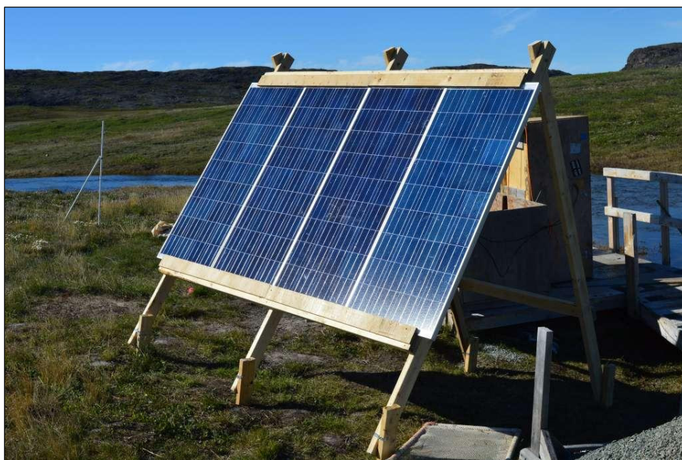
Plate 3.2-1. Solar panels providing power to the Vaki Riverwatcher downstream of the boulder garden, July 12, 2014.
