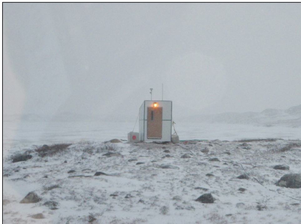
Plate 2.1-2. Temperature-controlled shelter housing the Partisol samplers, October 2011.
