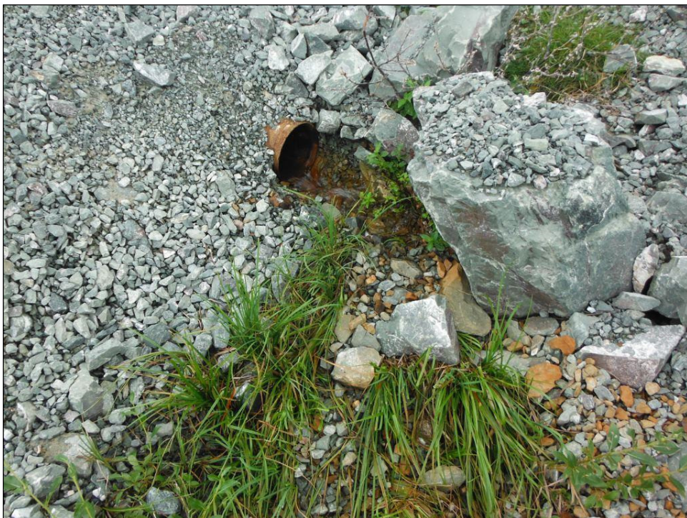
Plate 3.2-3. Discharge from the Doris Lake boat launch culvert percolates into loose gravels, August 13, 2015.
