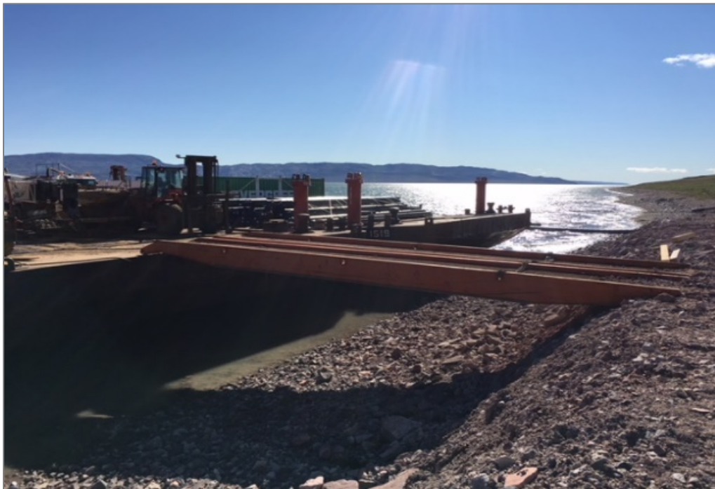
Image 5.1-1. Existing MLA Shoreline Pad Demonstrating Current Gap between Barge and Pad
