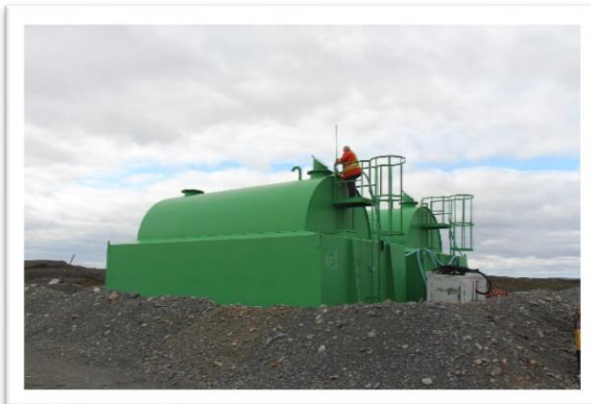
Photo 71: Fuel Tank Farm – Lined and Bermed
