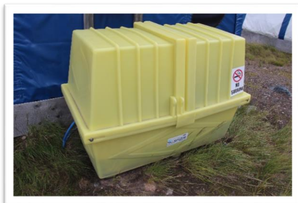
Photo 19: Heating Fuel Tank Container at Accommodations
