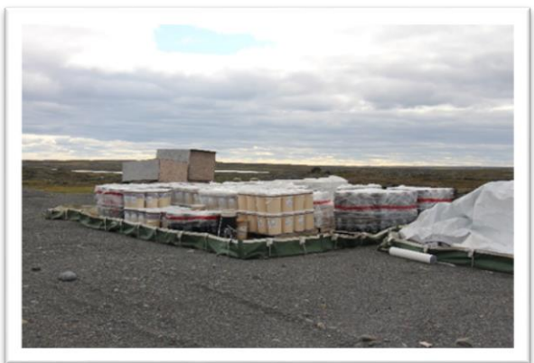
Photo 73: Insta-berm around drilling fluids
