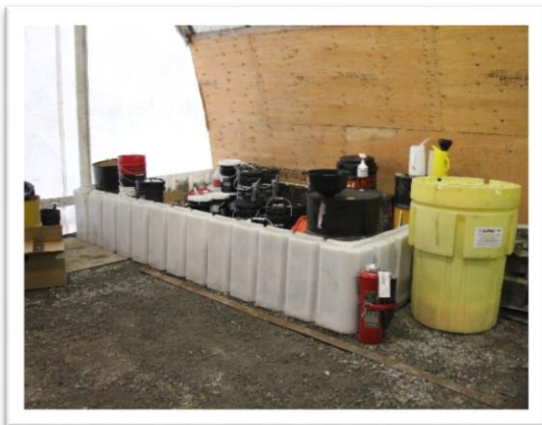
Photo 6: Oil and Fluid Containment
