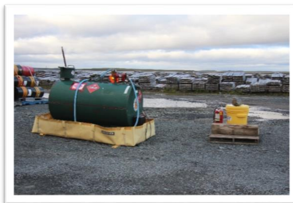
Photo 16: Insta-berm and Spill Kit
