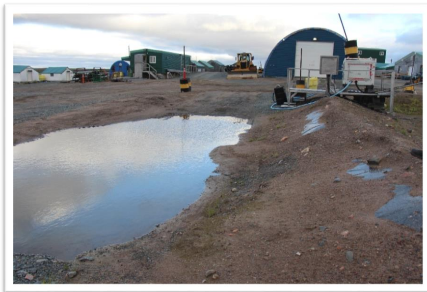
Photo 14: Ponding in Refueling Area - berm and liner
