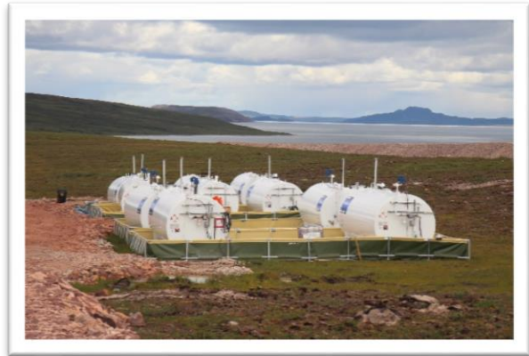
Photo 50: Fuel Tanks Contained in Insta-berm liners
