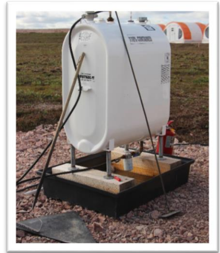
Photo 64: Spill Tray below Fuel Tank
