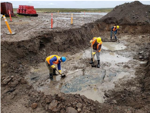
Photo 6: Exposing the bedrock in Goose Main Trench
