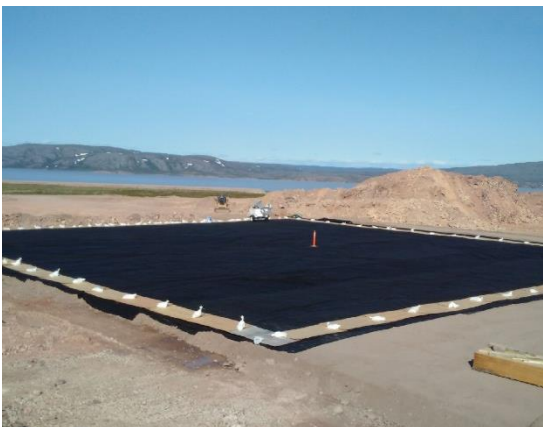
Photo 20: MLA Bulk Tank Liner
