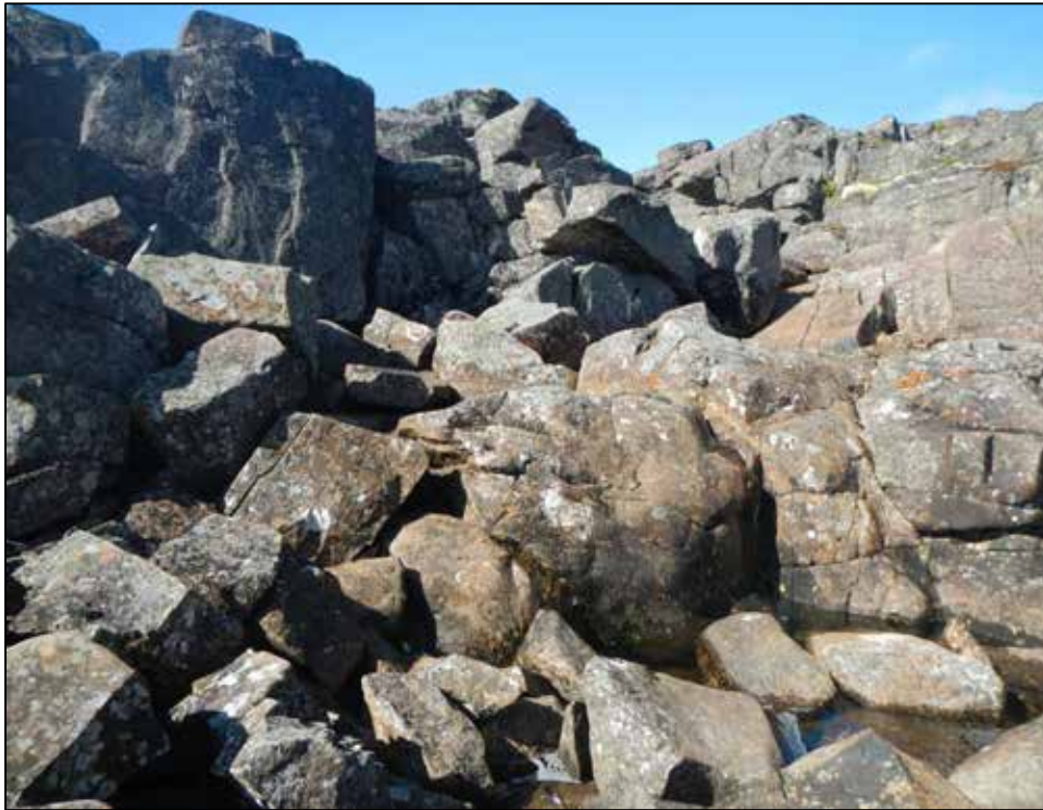
Plate 3.1-1. Rock cascade barrier on Site 101 – Umwelt Outflow, looking upstream. June 2012.
