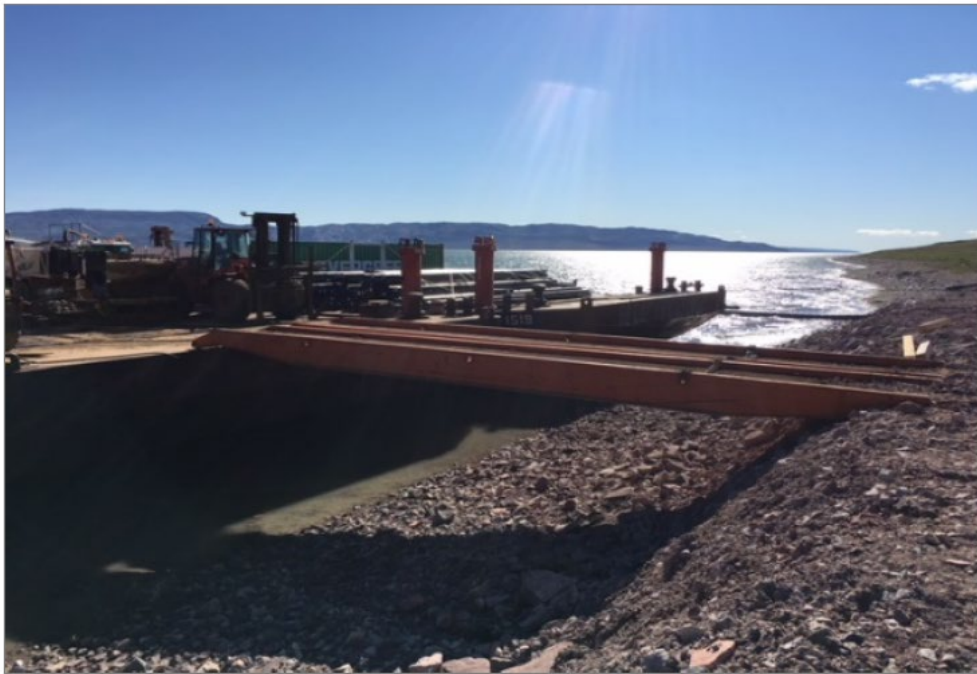
Image 5.1-1. Existing MLA Shoreline Pad Demonstrating Current Gap between Barge and Pad
