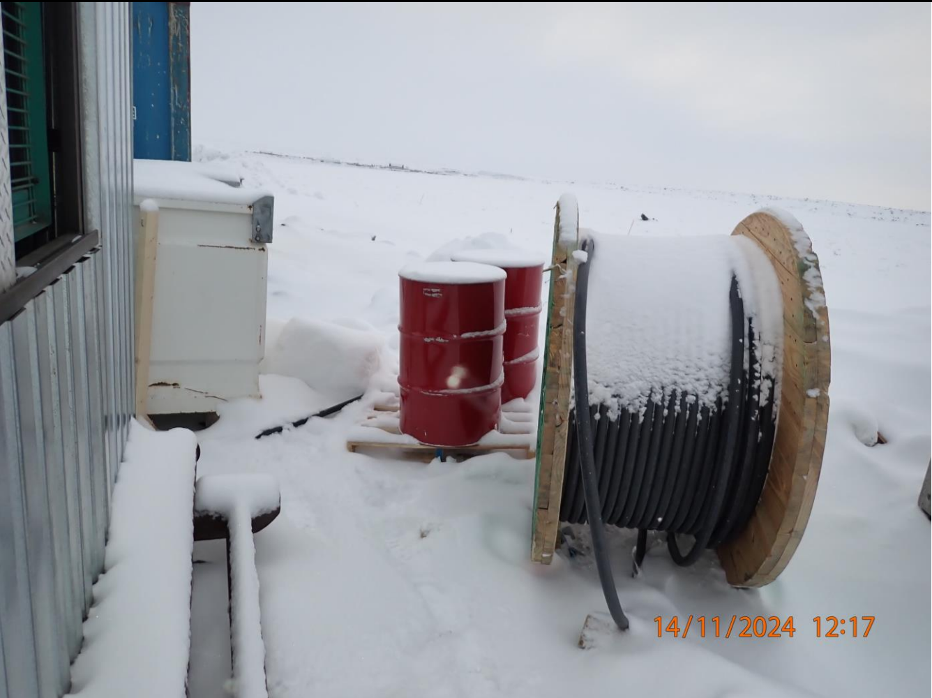
Gasoline outside of secondary containment at the emulsion plant area.
