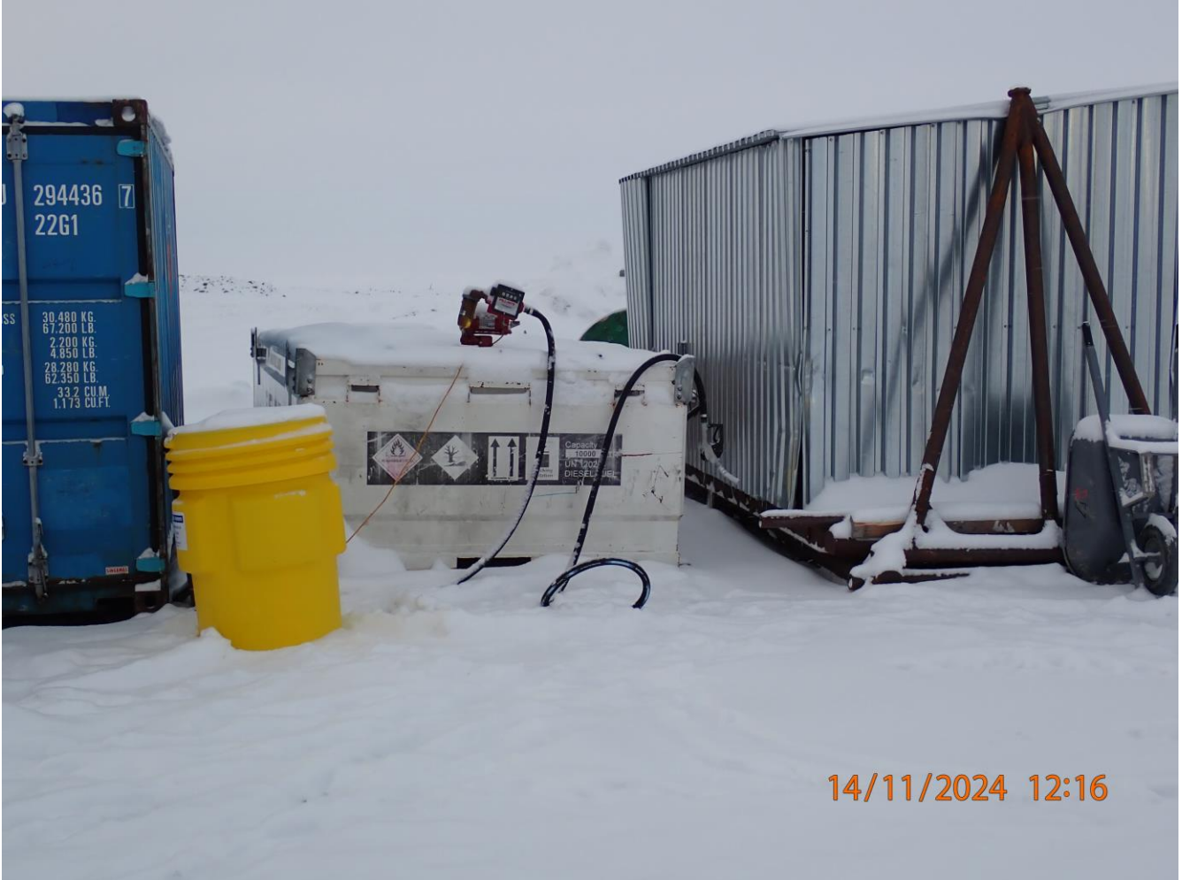
Refueling station hose and nozzle not stored in drip tray. Potential leaks can migrate from connections down the hose and onto the ground.
