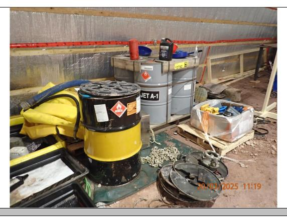
Inside the large tent truck shop at MLA showing Jet A-1 out of containment.
