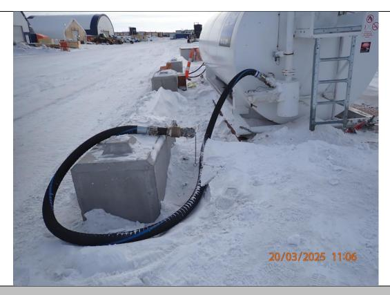
Heavy Equipment refuelling hose with no drip tray. This hose had signs of a leak at the connection to the tank.
