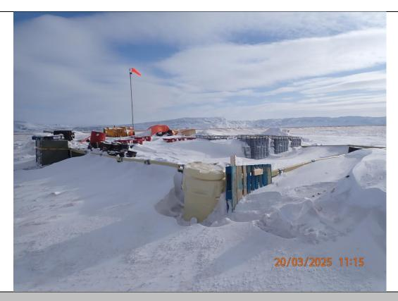
Insta-Berm beside the airstrip at MLA. Gasoline barrels and 1000L totes stored inside. A spill kit is in the foreground.
