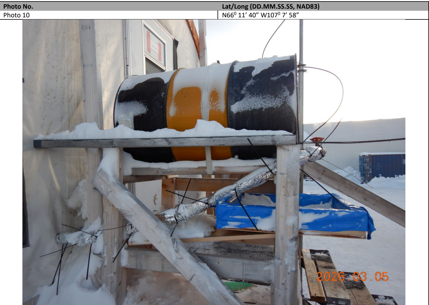
Description: Insufficient secondary containment.
