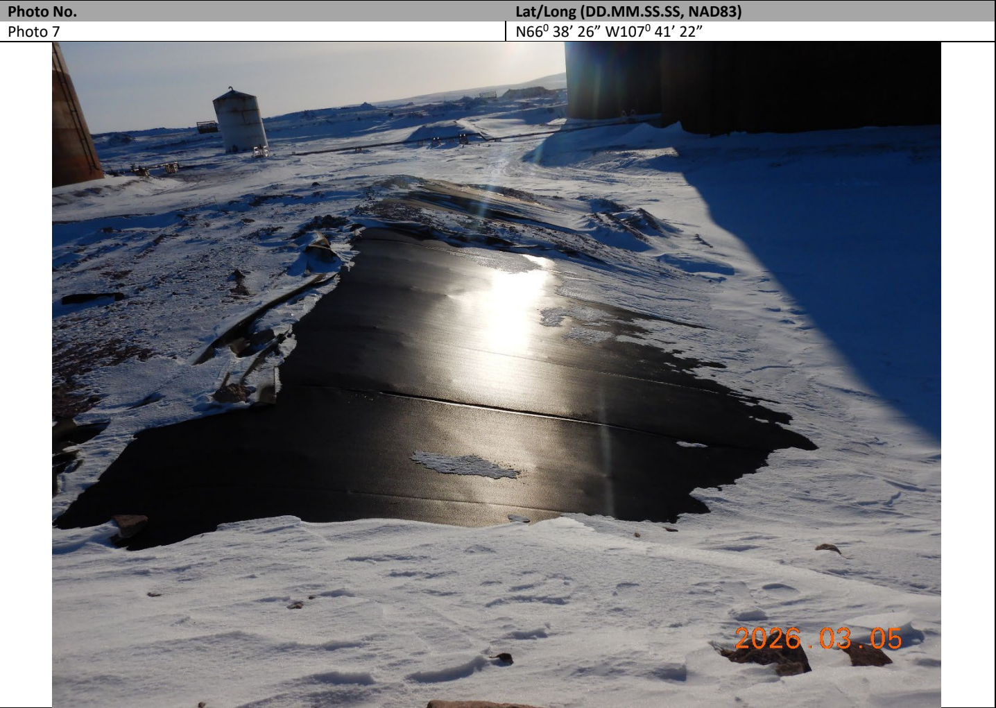
Description: Exposed HDPE Liner.
