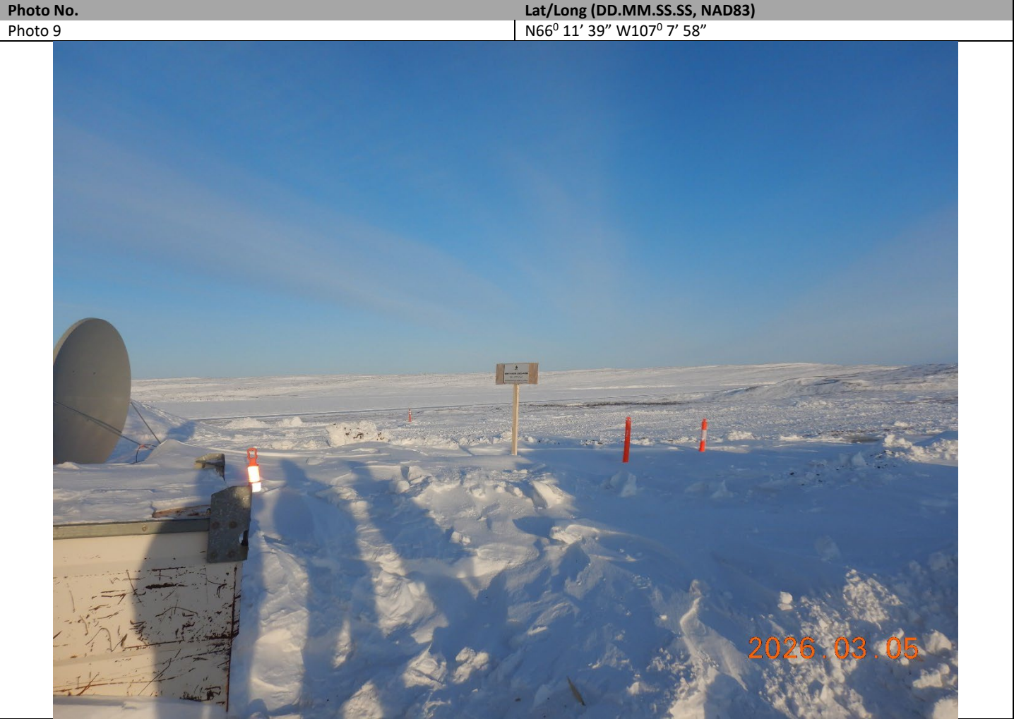
Description: Grey water discharge line at MLA forward camp.
