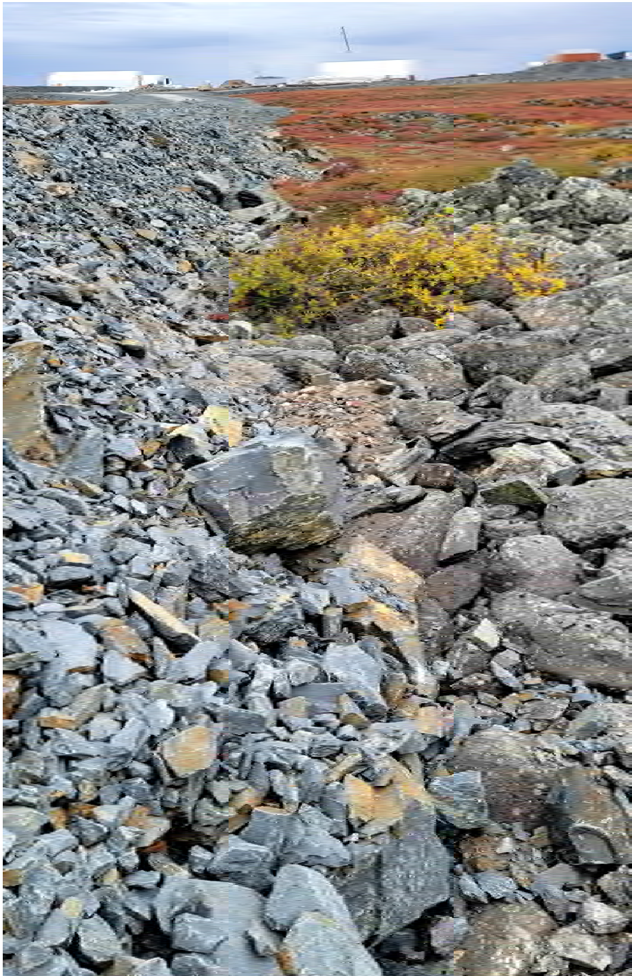
Photo G-82. - Example of the fill material used for the all-weather road construction. Some boulders greater than 0.8m in diameter are found at the toe of the embankment. Note the thickness and slope angle of the embankment. The photo was taken looking south.
