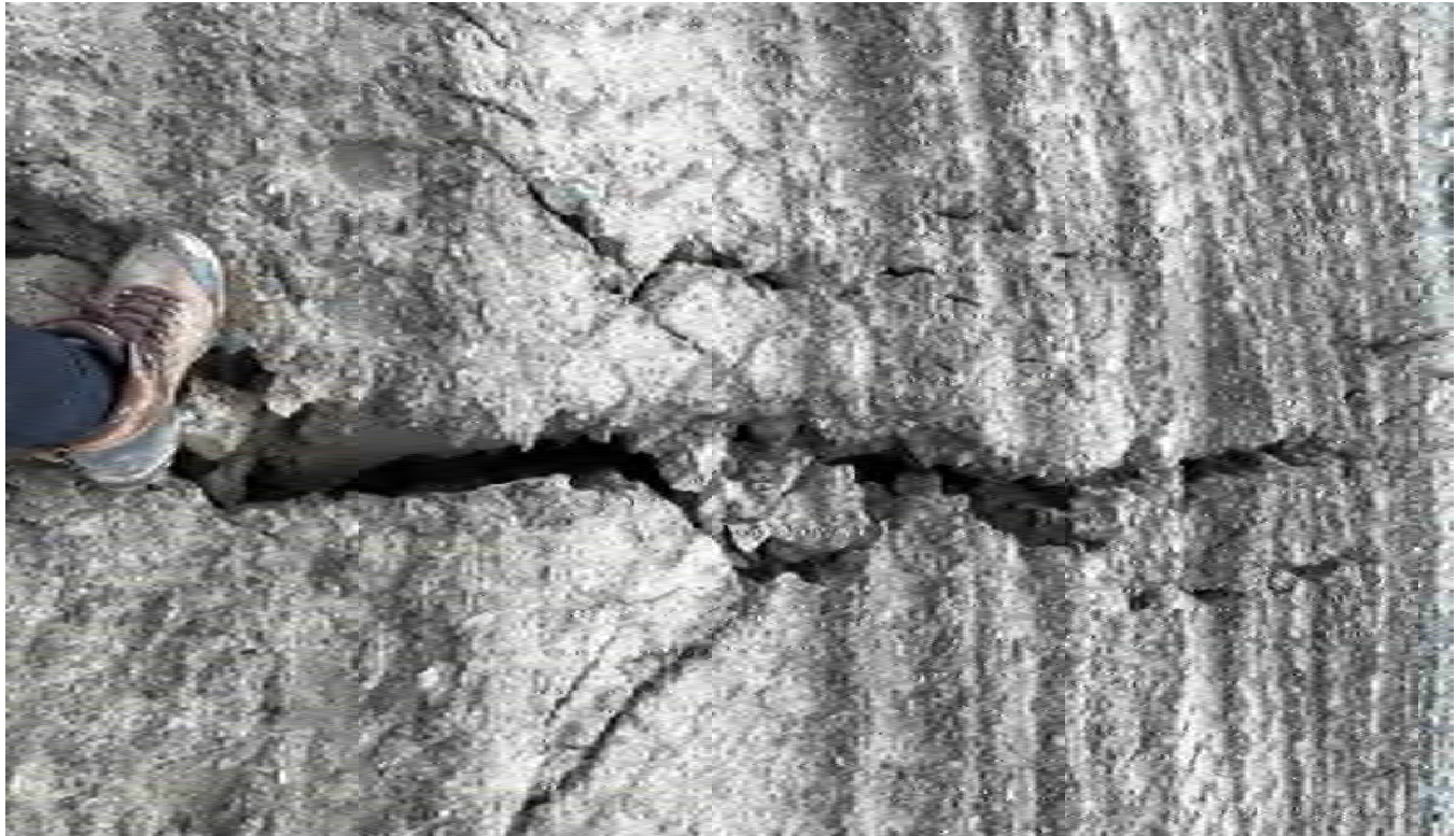
G-63. - A set of elongated cracks approx. at Sta 0+450
