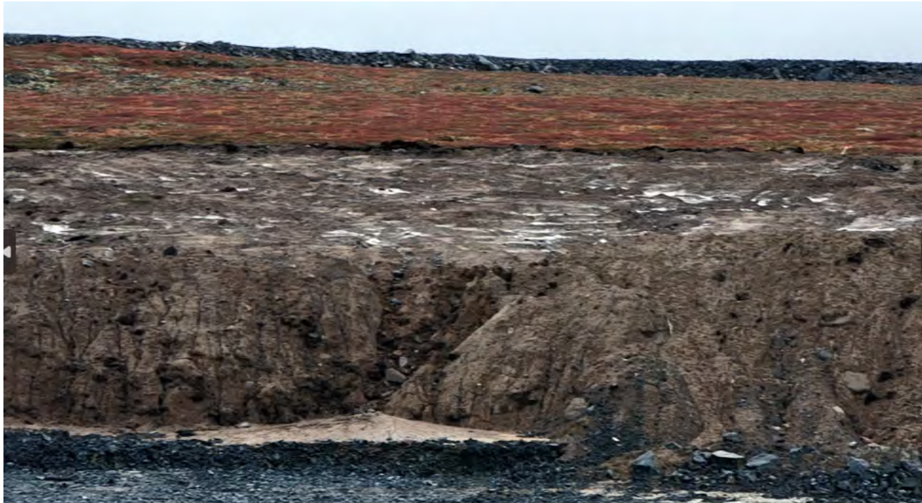
G-14. Erosion gullies at the SSW wall of Echo Pit
