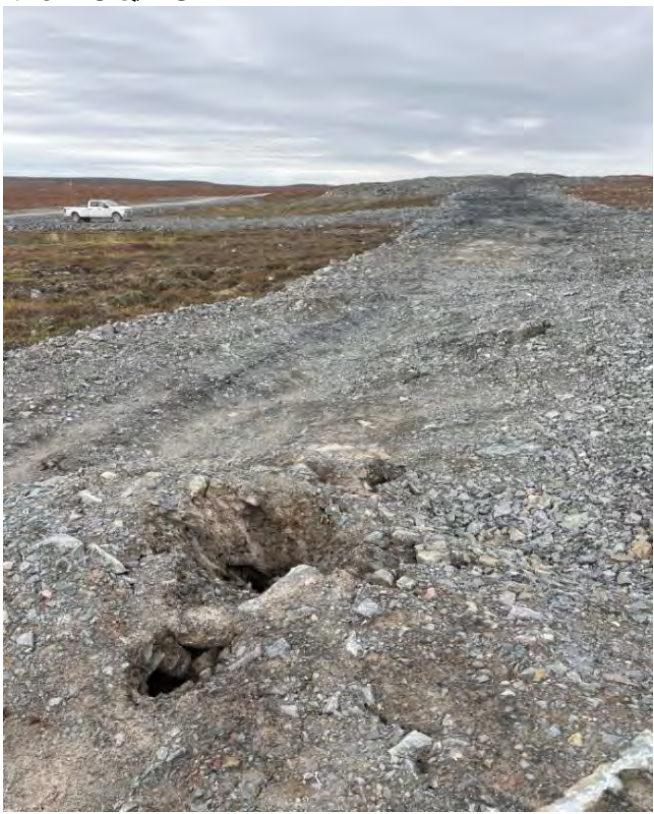
G-58 and G-59. - Embankment degradation approx. at Sta 0+260.
