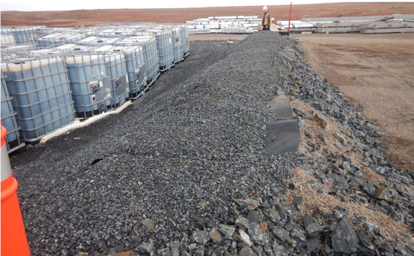
G-41. – Western berm of the secondary containment storage area, looking south. Note exposed HDPE liner
