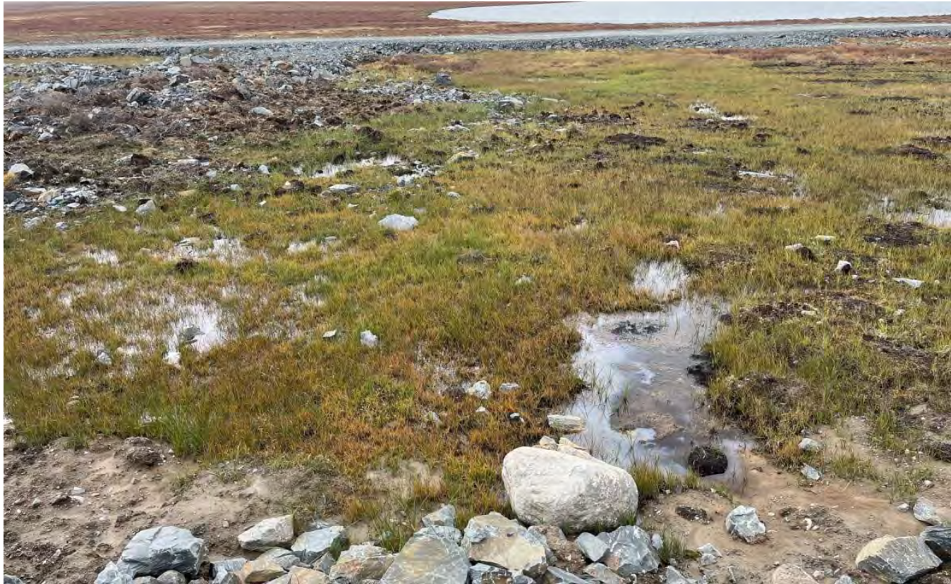
G-60. – Ponding water at the downstream side of the key trench approx. at Sta 0+270
