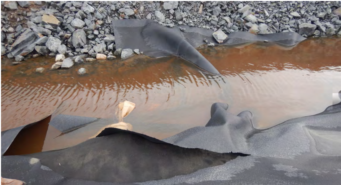
G-49. – HDPE liner is not anchored to the berm
