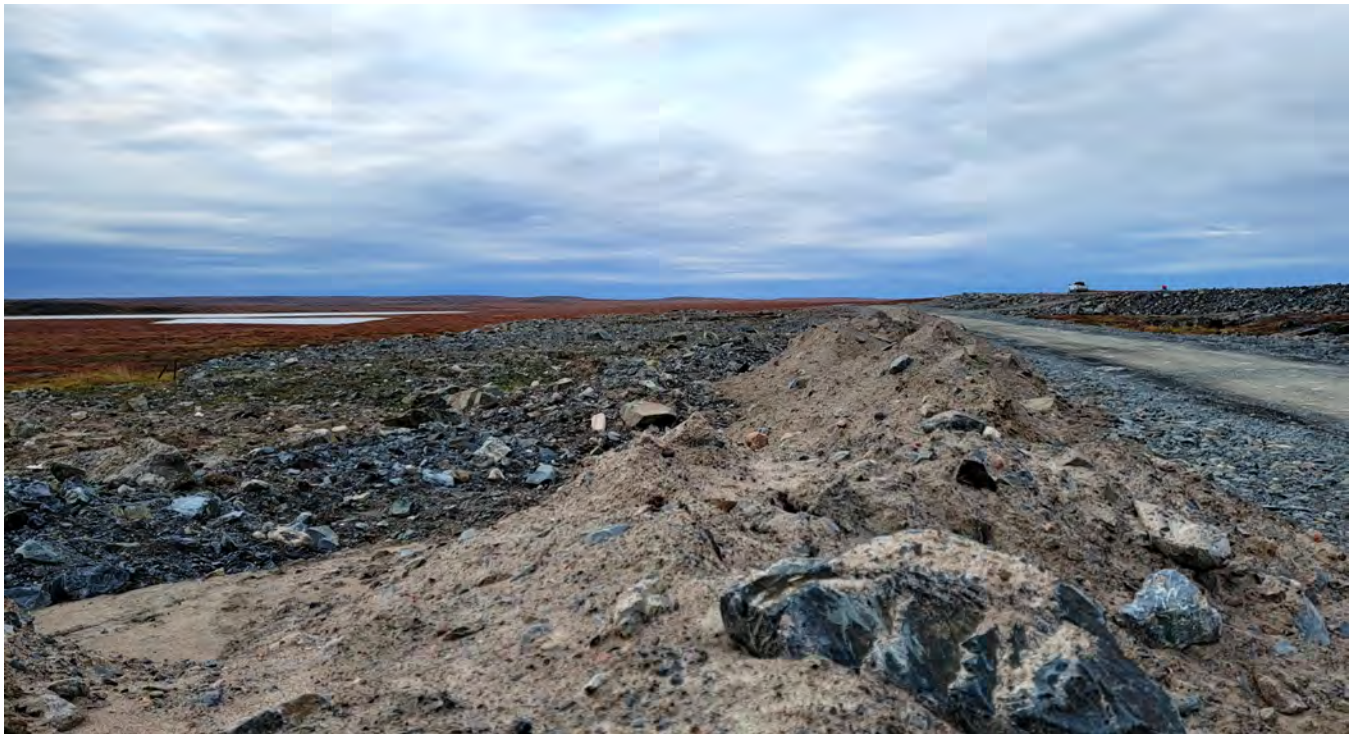
G-74. - Downstream side of the runway. Piles of the overburden material
