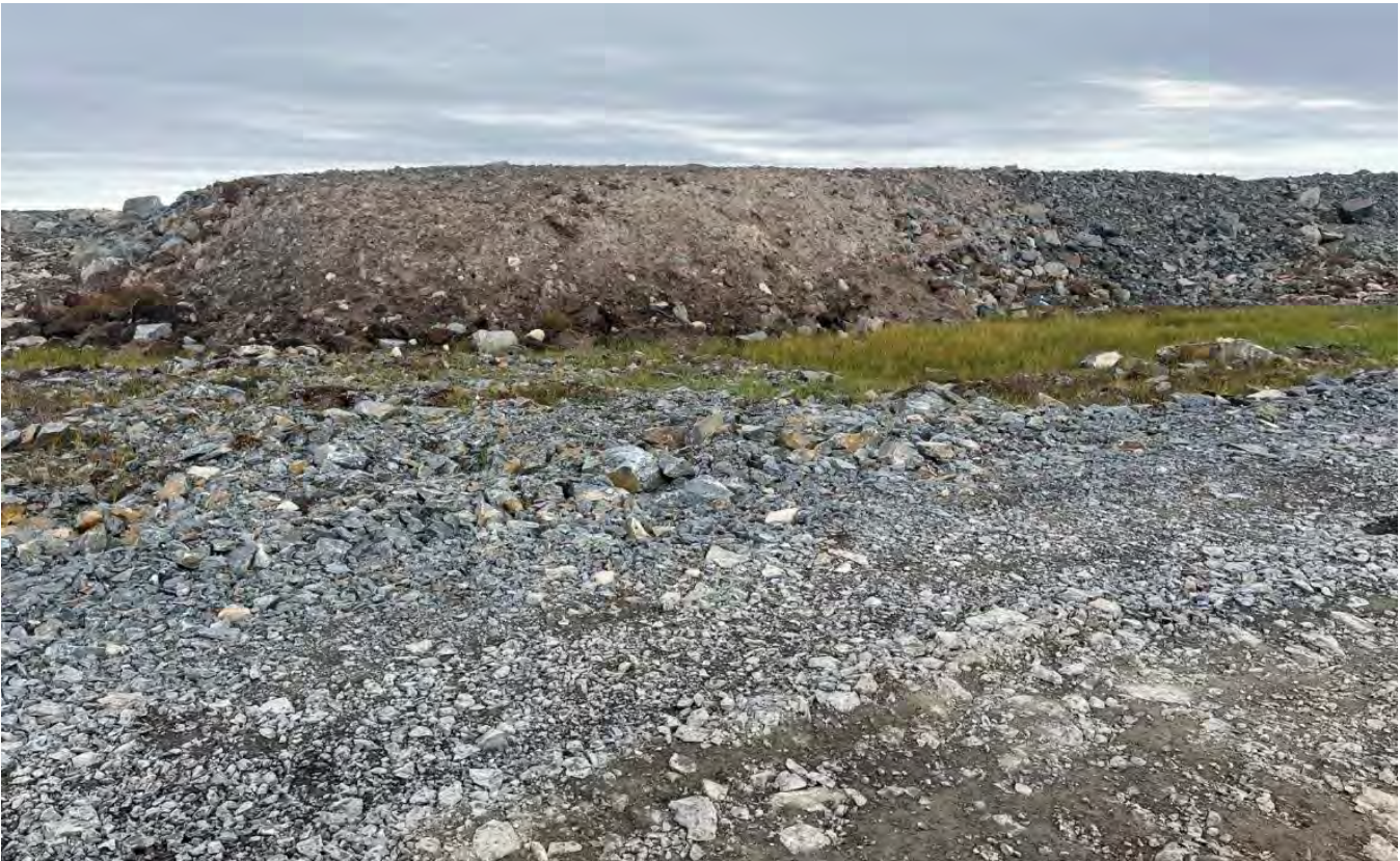
G-62. – Minimum winter cover (bulk material placed approx. at Sta 0+430)
