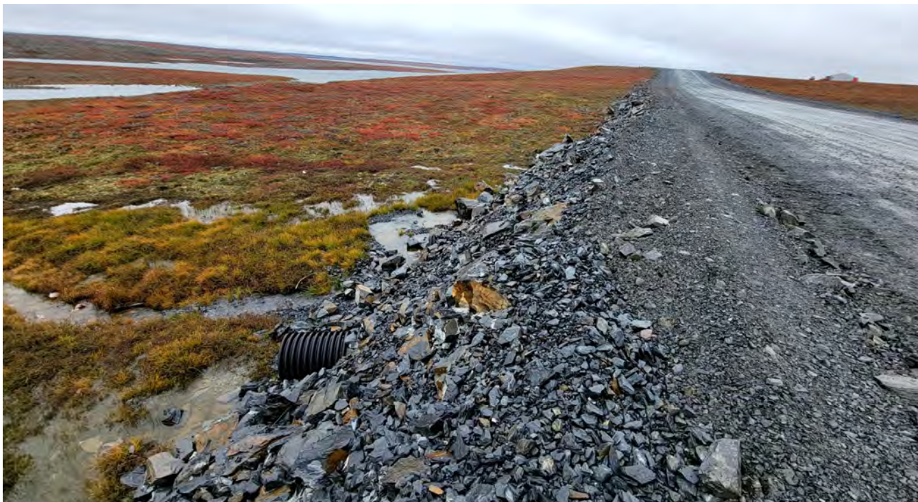
G-91. – Culvert: Inlet. Note some ponding water at the toe of the road
