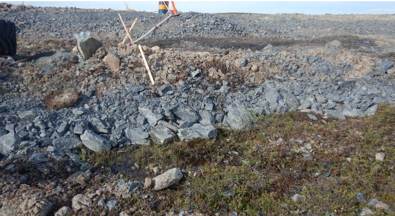
G-54. – Ponding water at the downstream side of the key trench approx. at Sta 0+550
