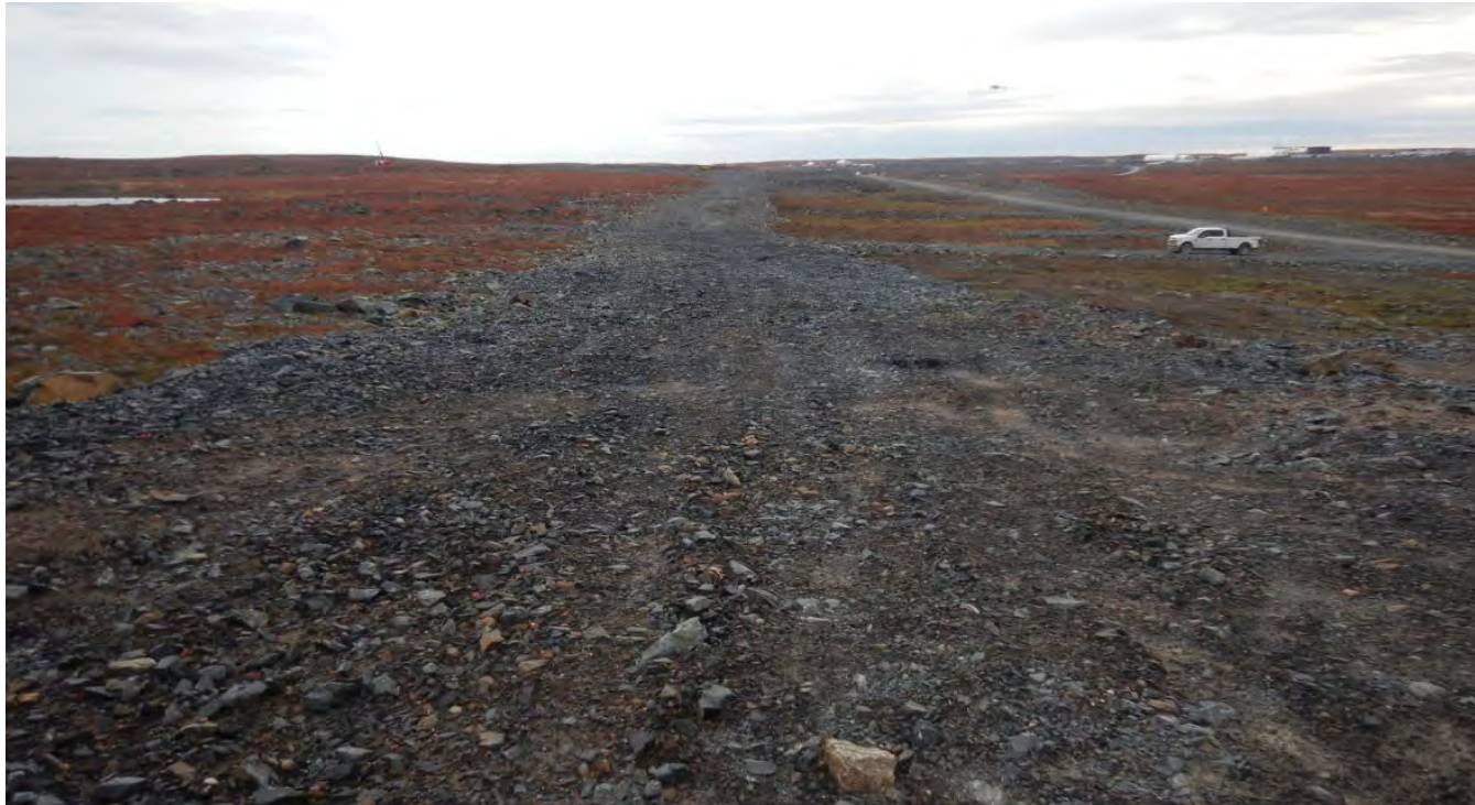
G-51. - A temporary access road at the upstream side of the key trench was built in Jan 2023, looking SE (approx. between Sta 0+50 and 0+150)
