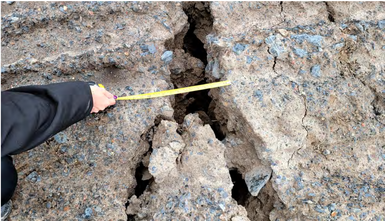
G-64. - A set of elongated cracks approx. at Sta 0+450
