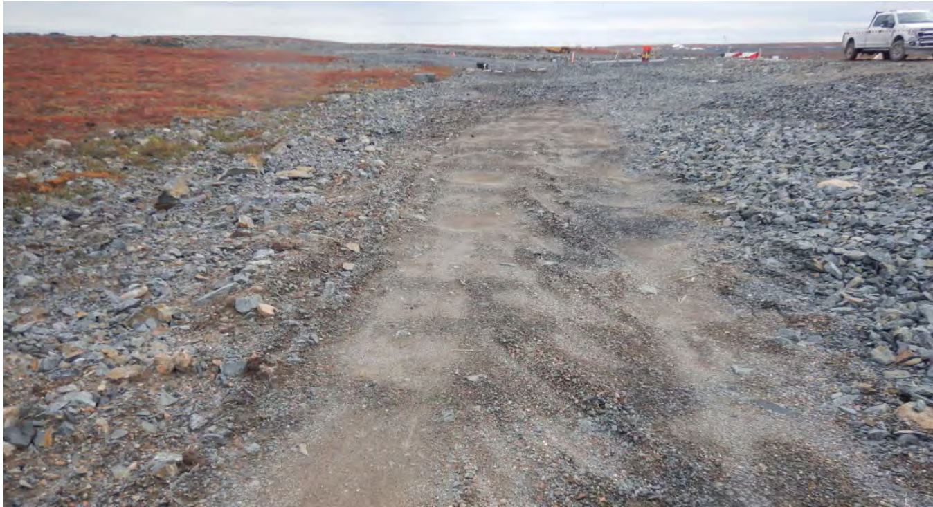
G-55. - Temporary Road along the upstream side of the key trench approx. at Sta 0+400
