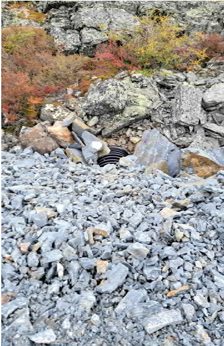
G-81. - The outlet is covered with large boulders.
