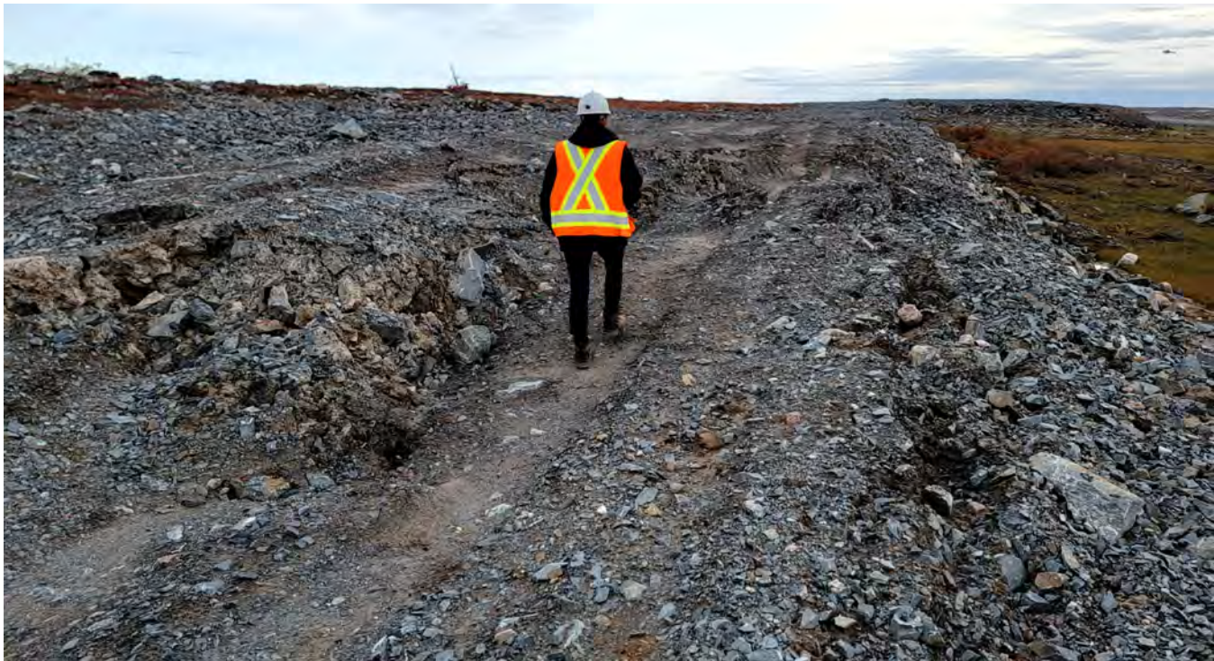
G-57. – Temporary Road along the upstream side of the key trench approx. at Sta 0+260. Note embankment degradation
