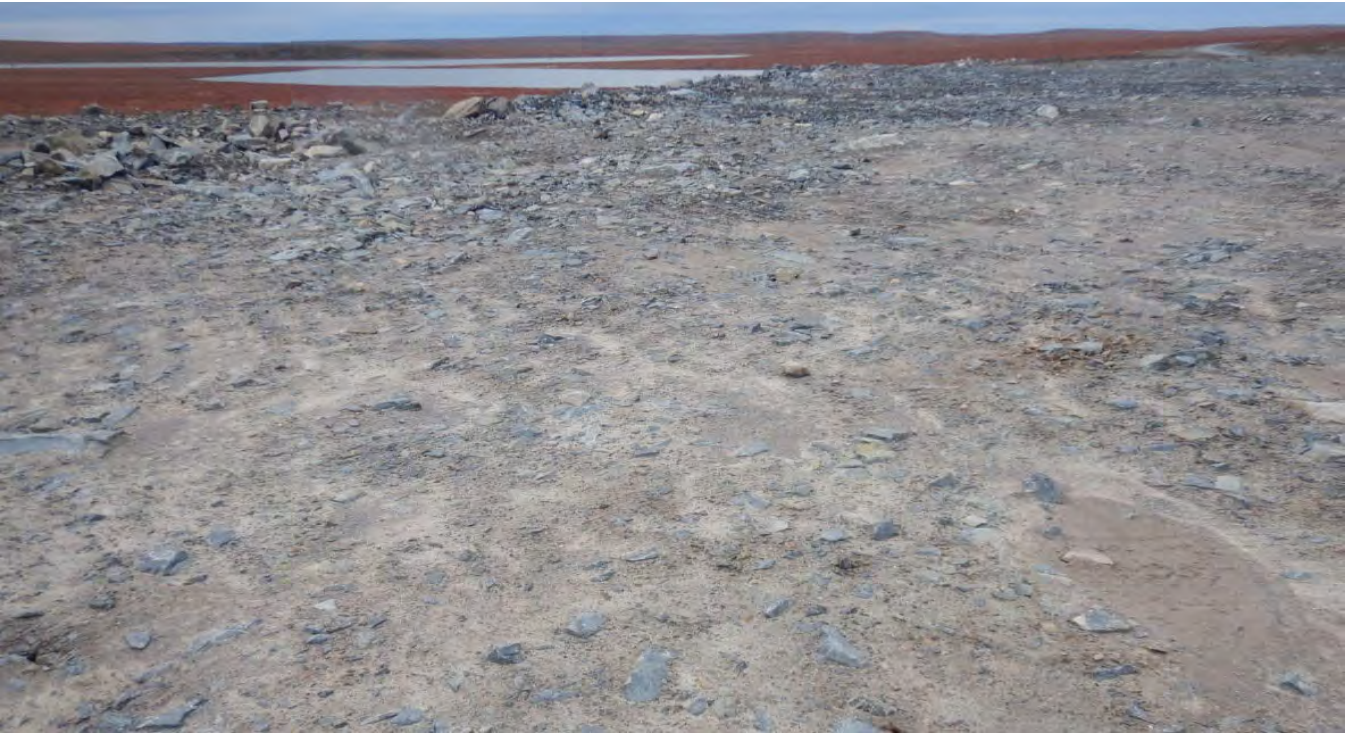
G-56. – Key trench winter cover approx. at Sta 0+410. Note the high overburden content in the ROQ/ROM
