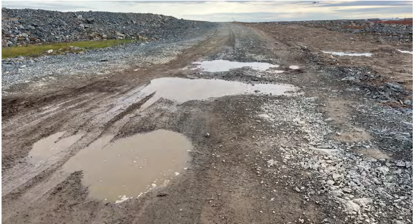
G-72. - Road embankment undulation
