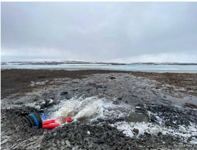
Photo 3: Dewatering pump discharge downstream of secondary culvert excavation, facing Goose Lake, 10 May 2023.
