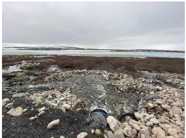
Photo 4: Temporary culverts discharging twin multiplate culvert excavation, facing Goose Lake, 10 May 2023.
