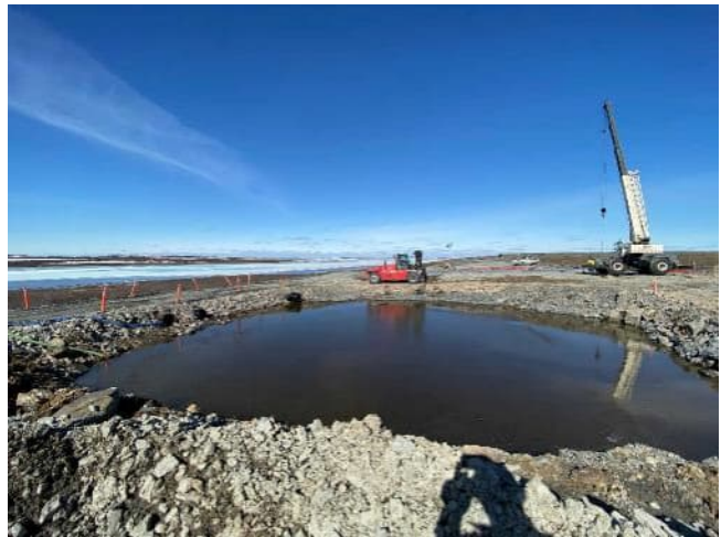
Photo 6: Twin multiplate culvert excavation, 11 May 2023.
