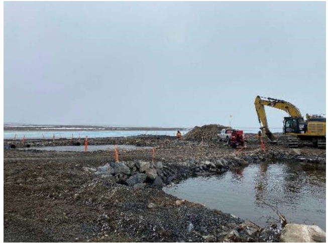
Photo 2: Lower pond seeping into twin multiplate excavation through temporary road, 10 May 2023.
