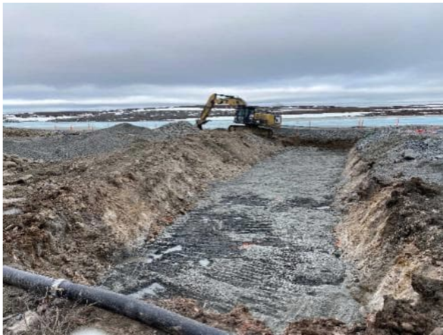
Photo 5: Secondary culvert excavation with bedding placed, looking downstream, 11 May 2023.
