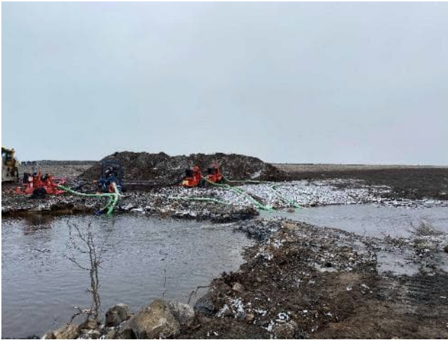
Photo 1: Dewatering pumps in upper pond and lower pond upstream of twin multiplate culvert excavation, 10 May 2023.
