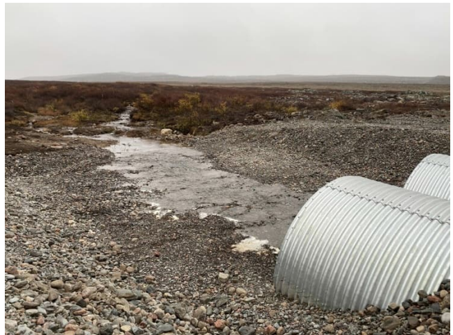
Photo 38: Completed twin steel culverts in the primary channel of RSW, facing upstream, 17 September 2023.
