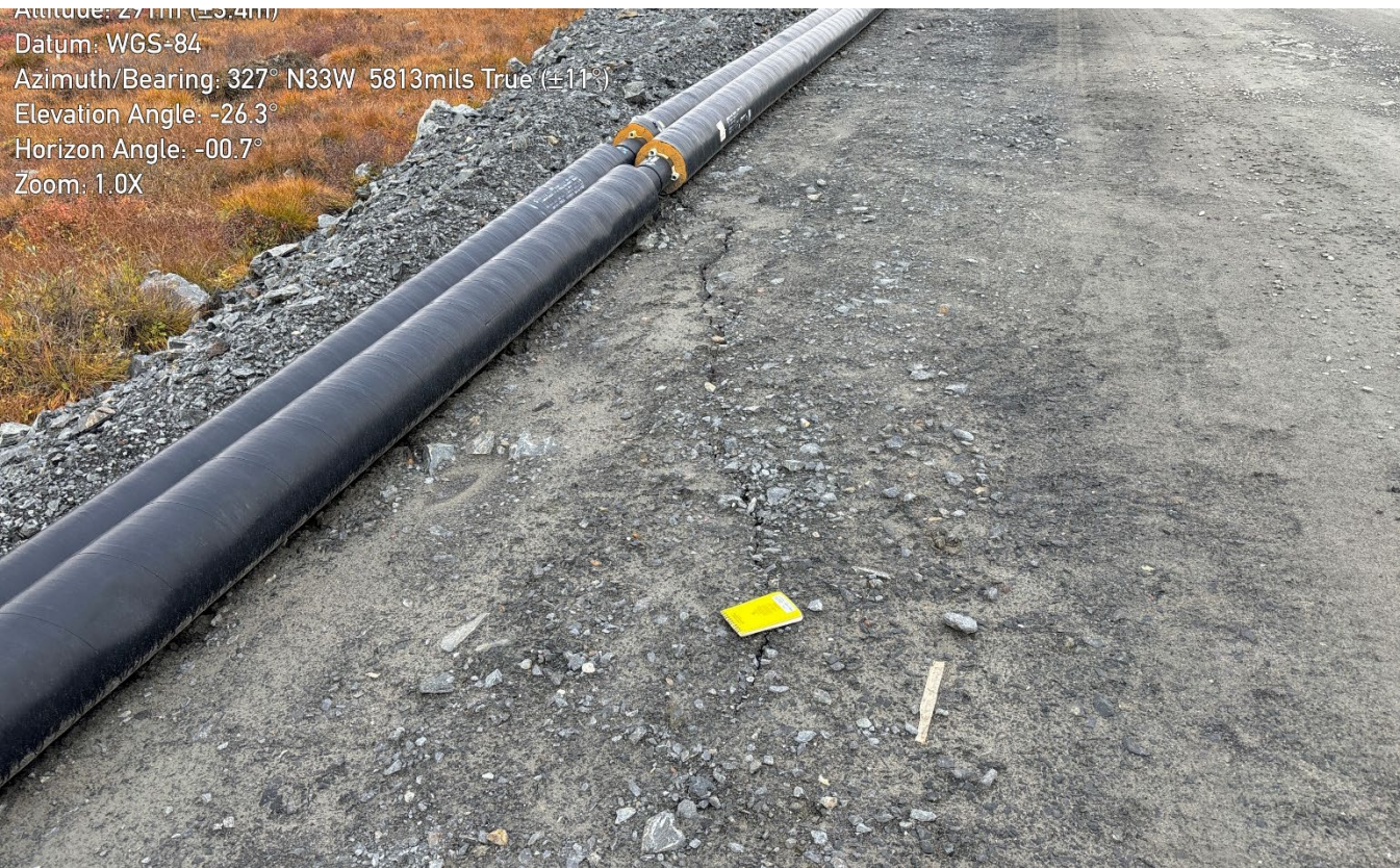
G-234: Tension crack through pipeline
