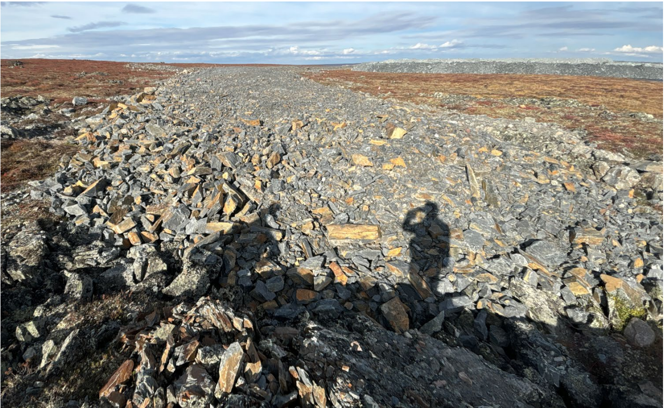
G-80: Westerly end of diversion – Note thickness below 1m
