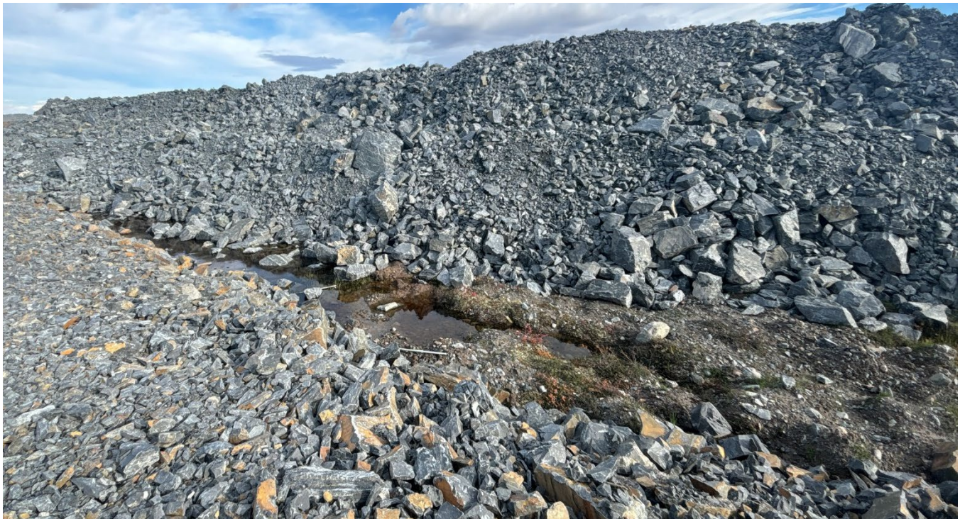
G-73: Diversion, facing west – Note that dump is built on overburden rich sections at the toe
