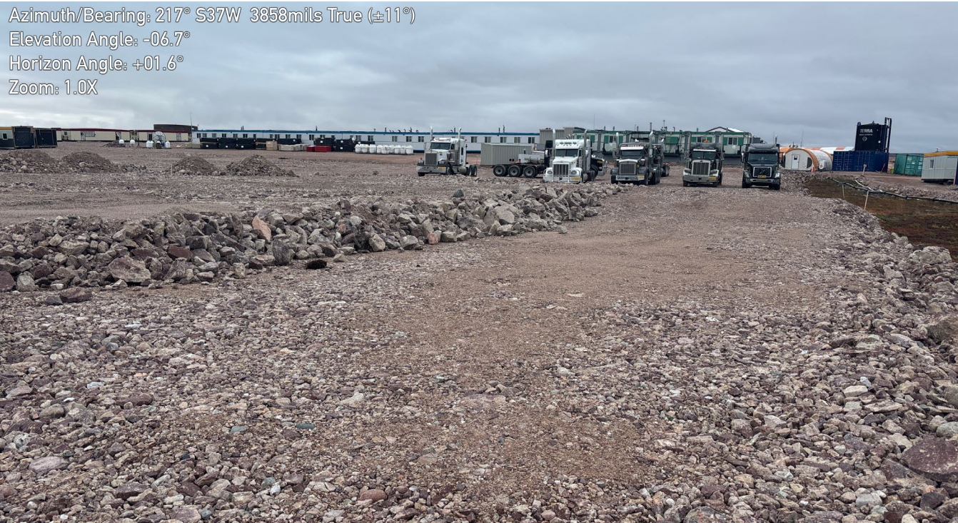
M-1: North end of pad – Note fill material is placed in lifts
