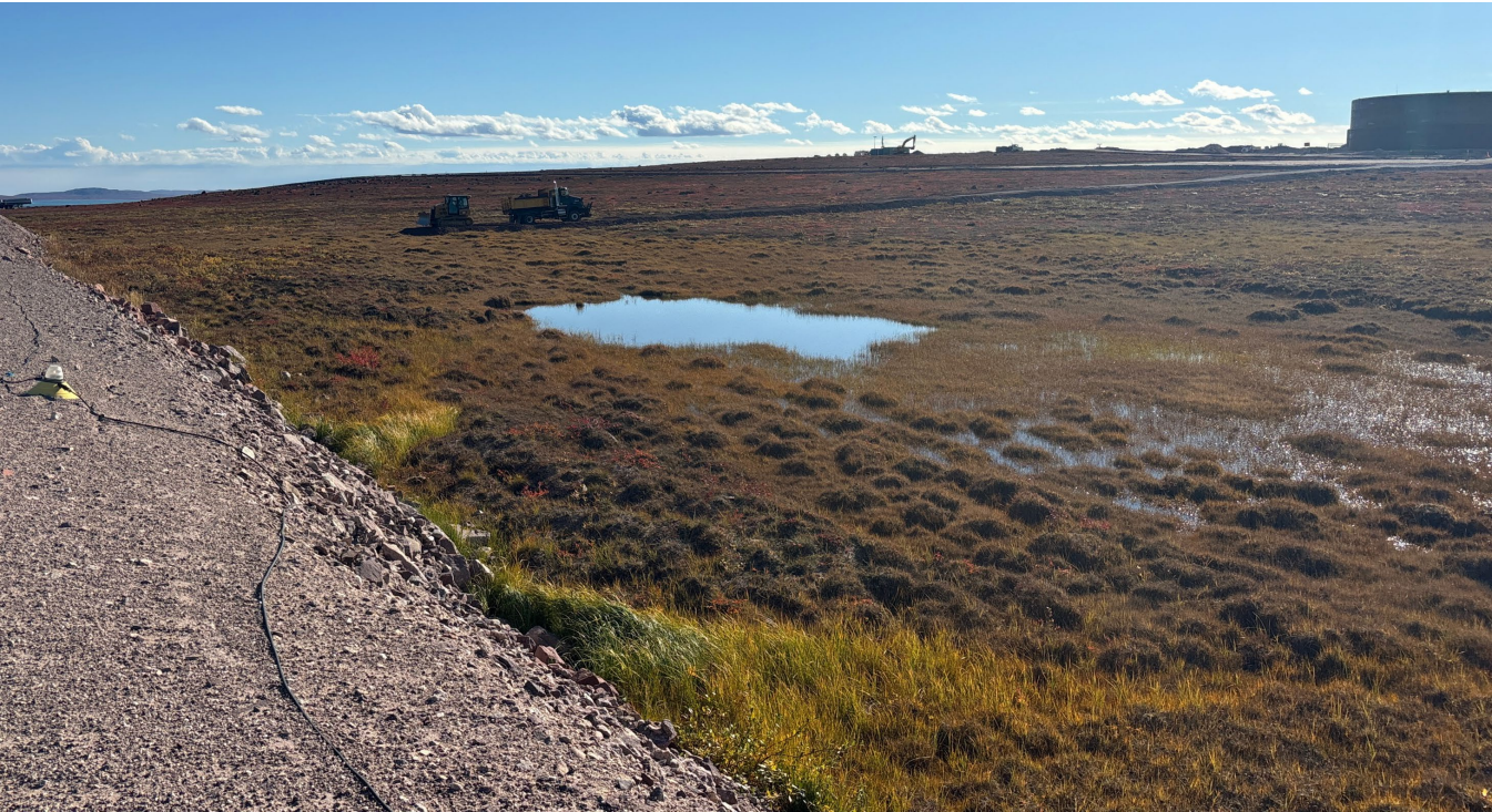
M-25: South end – Note Ponding water at the toe of the embankment
