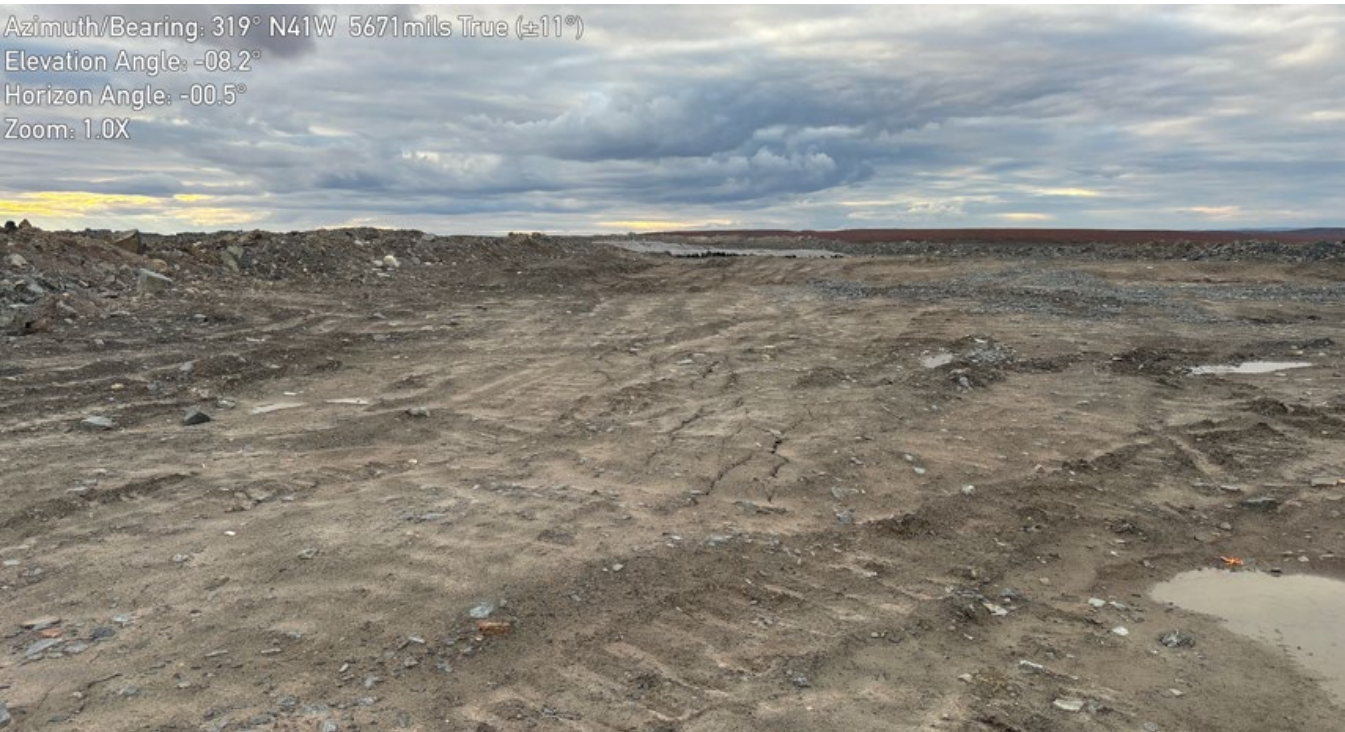
G-113: General Stockpile surface condition, facing NW – Note tension cracks
