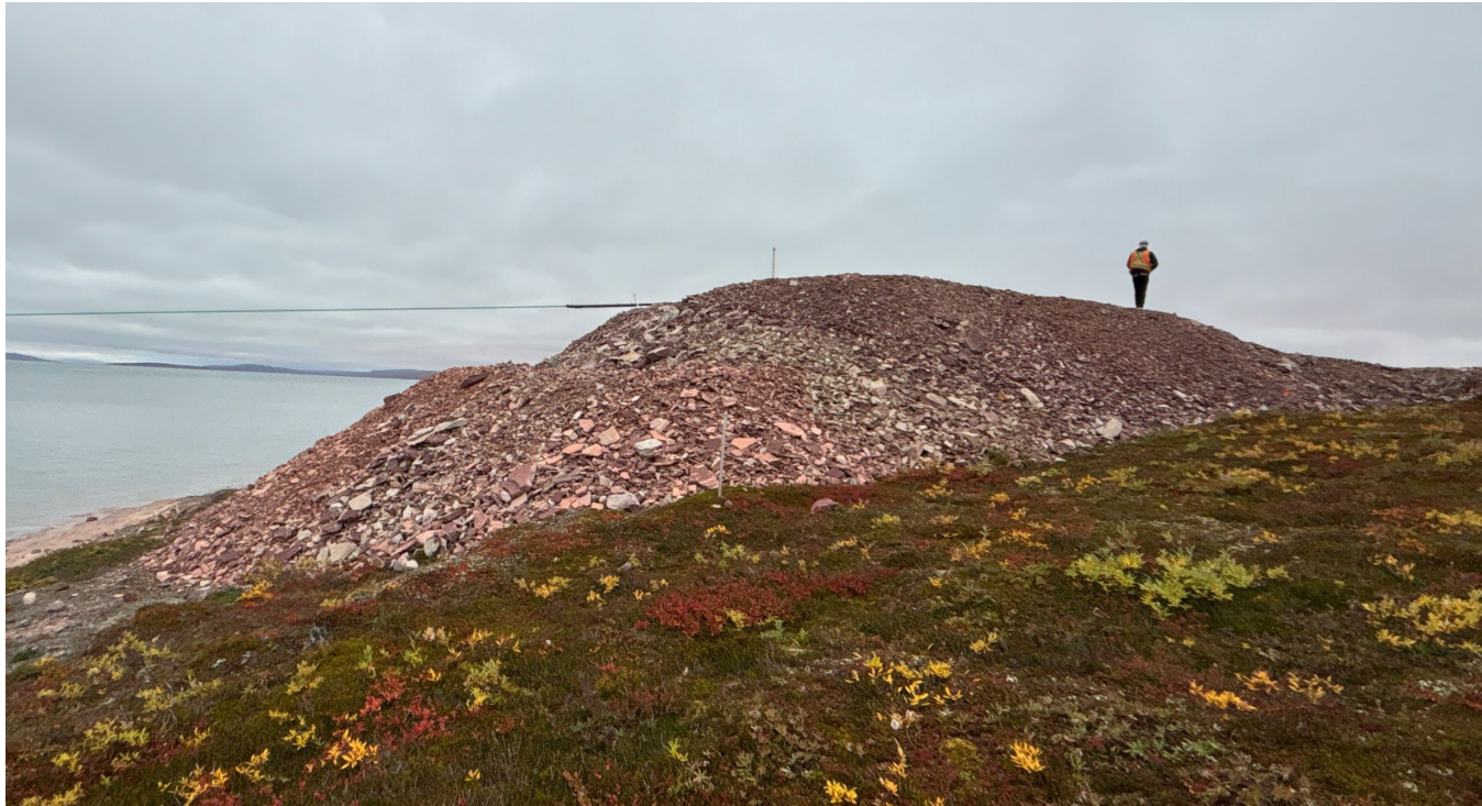
M-56: South anchor pad, facing south – Note shore erosion
