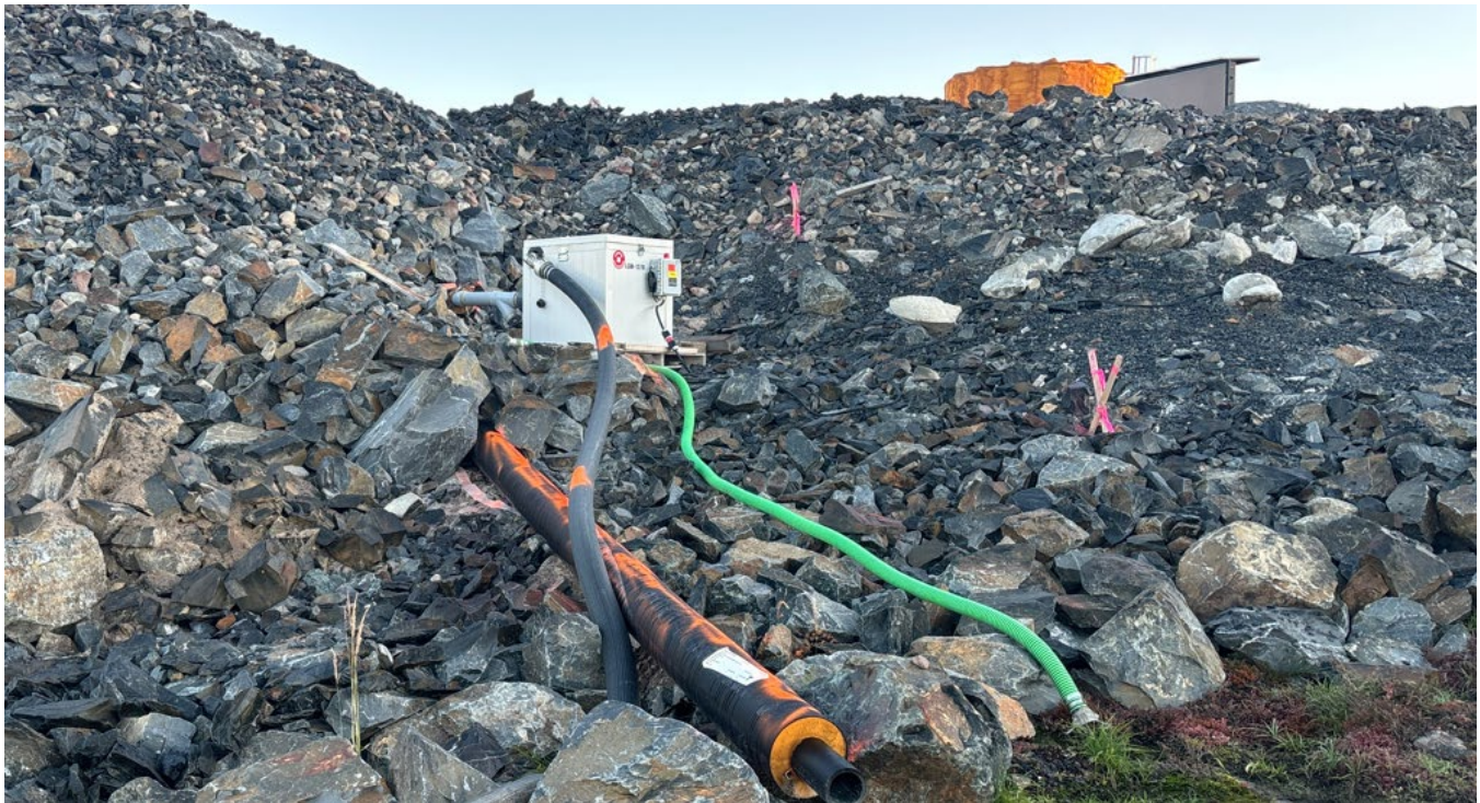
G-181: Discharge area – Note Oversteepened slope, equipment can be damaged by falling rocks
