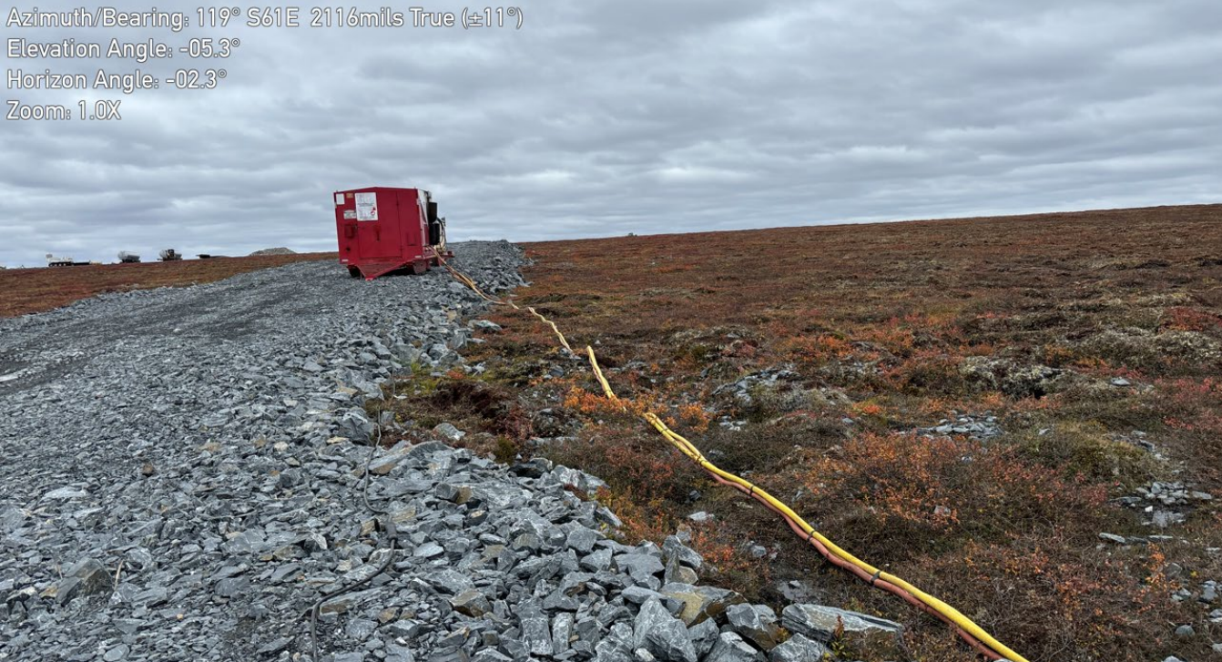
G-254: Pond access road, facing east – Note road is underbuilt
