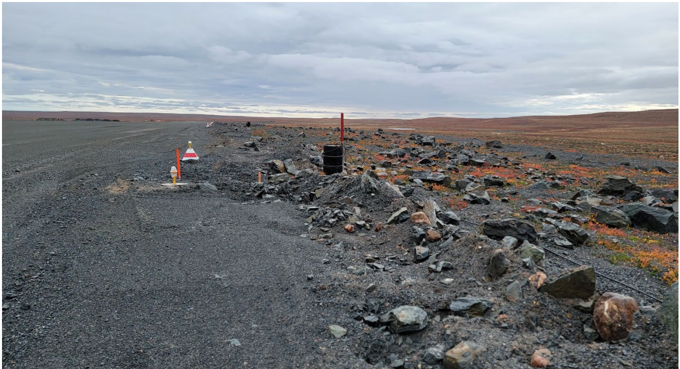
G-37: SW side of airstrip, facing SW – Note no distinct edge of runway
