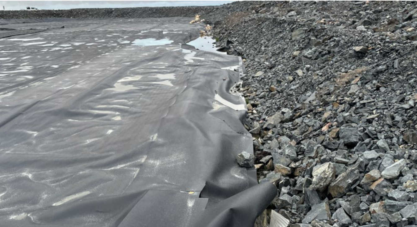
G-152: Western slope, facing east – Note no liner tie-in and varying crest of liner
