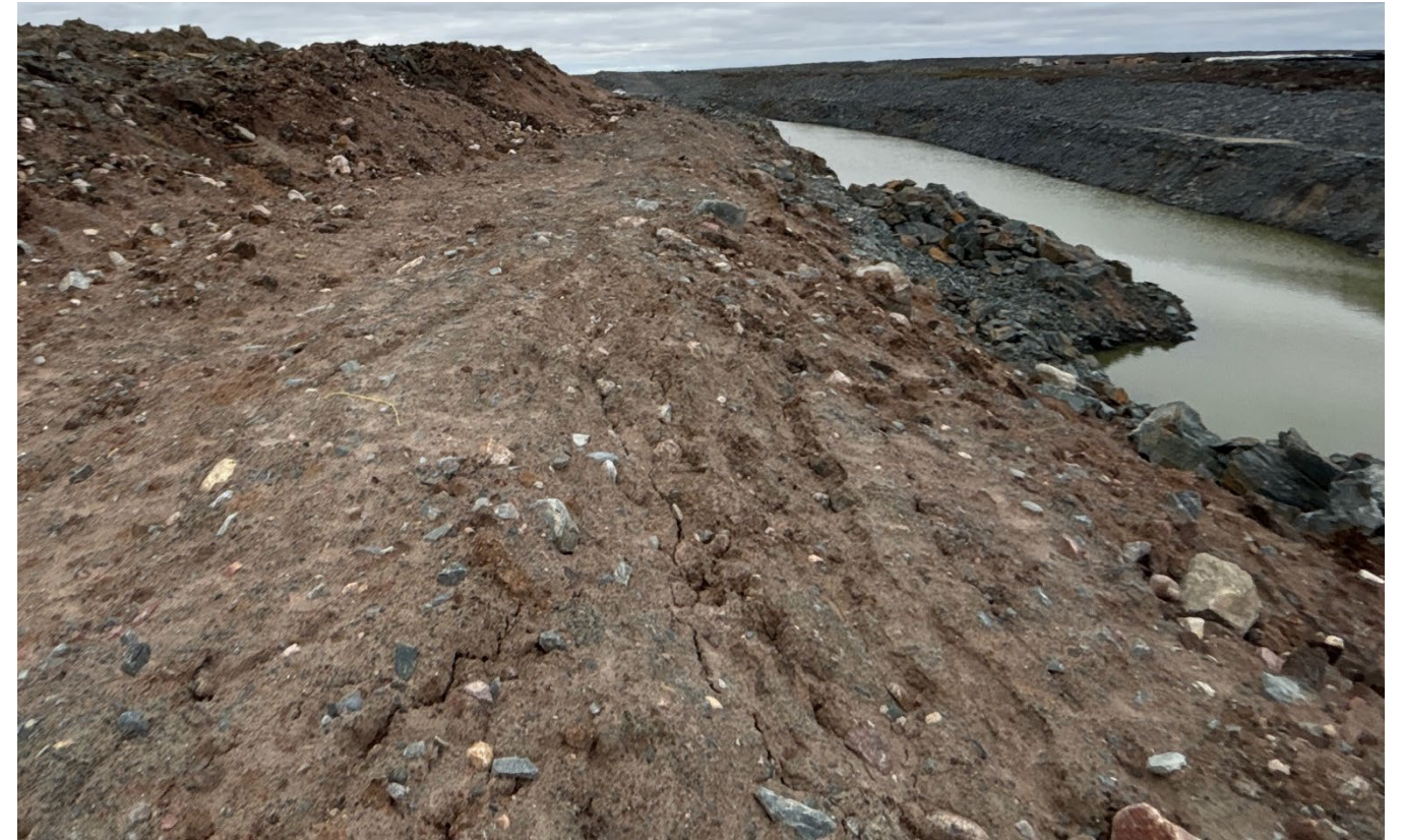
G-211: Southern end of SW slope – Note tension cracking
