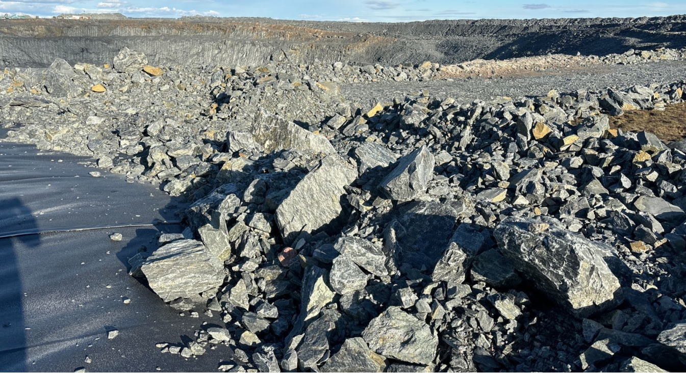
G-90: Pond tie-in – Inappropriate over-liner material (4" plus blasted rock)
