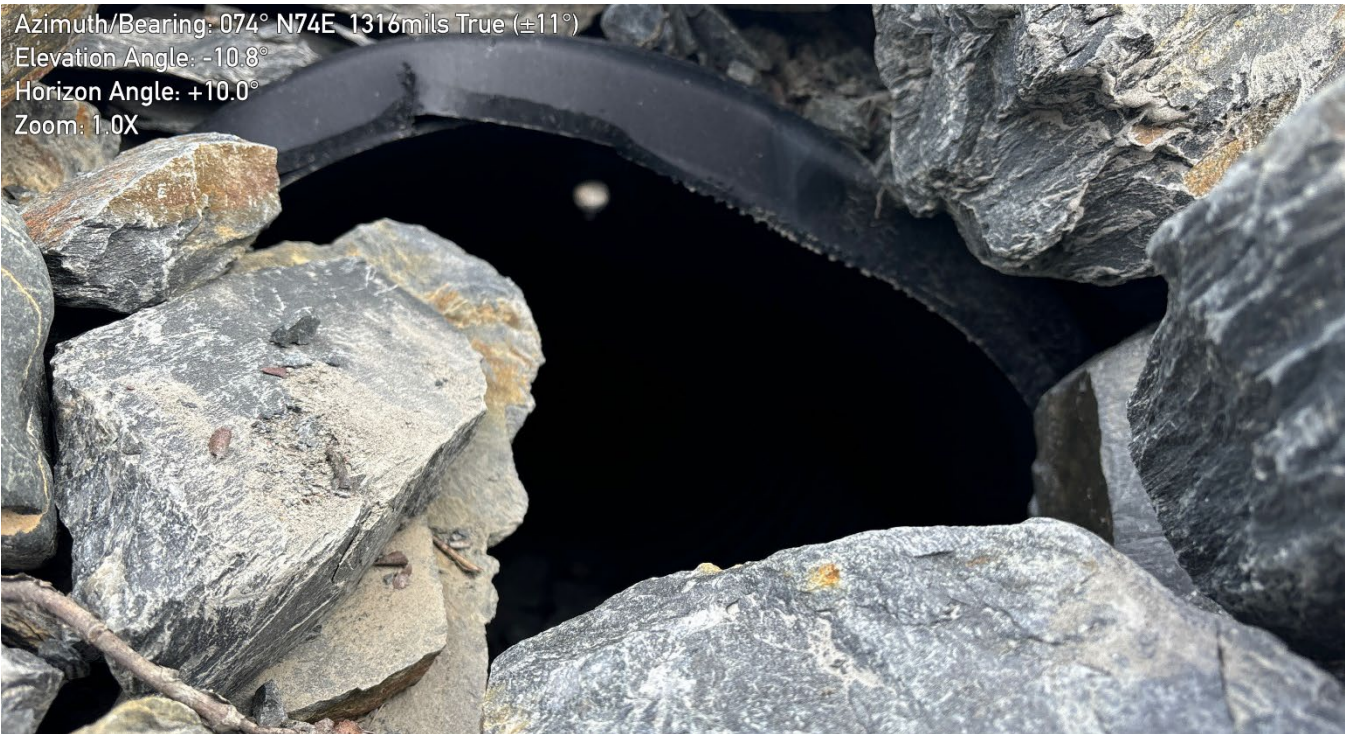
G-231: Culvert inlet partially blocked
