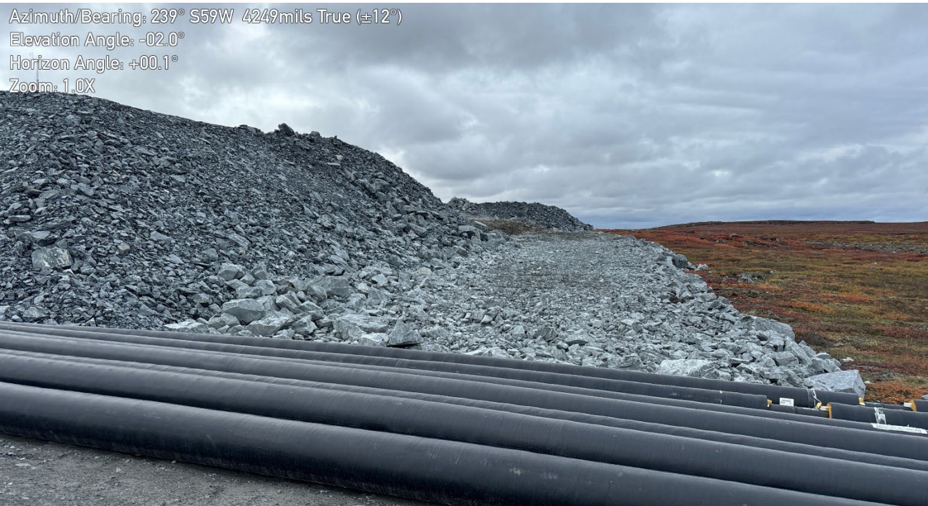
G-200: Extension from all-weather road. Facing west – Note oversteepend slopes
