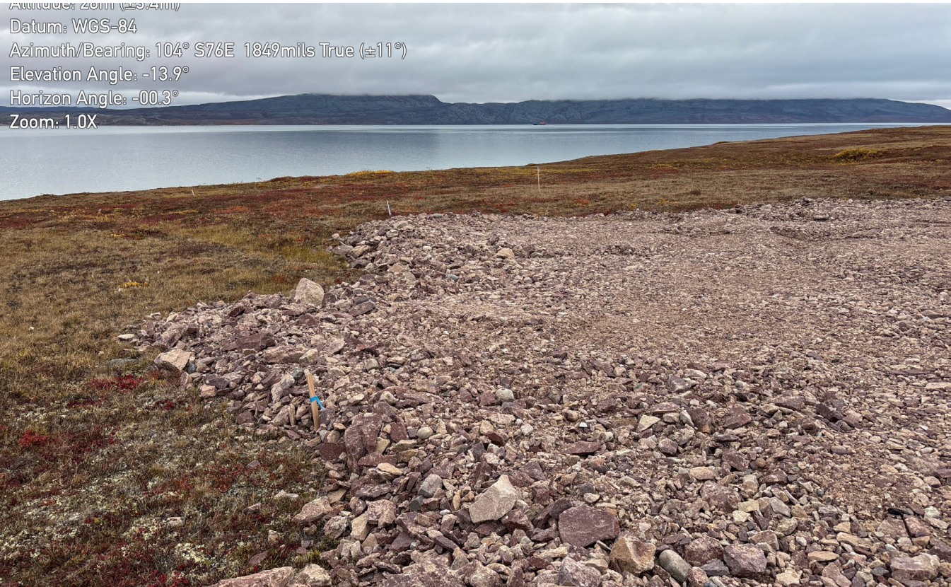
M-9: SE end of pad – Note fill is too thin
