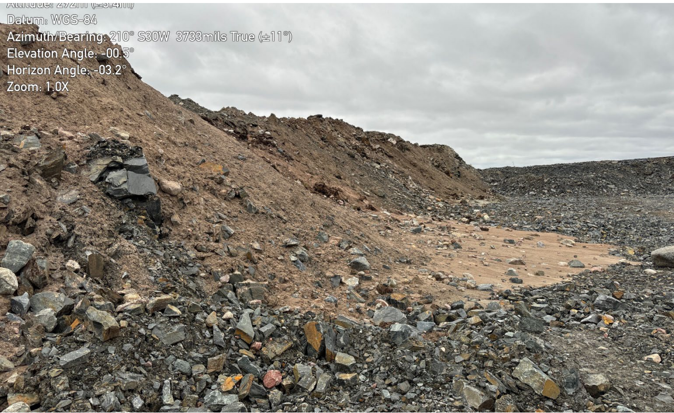
G-213: Umwelt slope. First bench on SW side, facing north – Note thermal erosion
