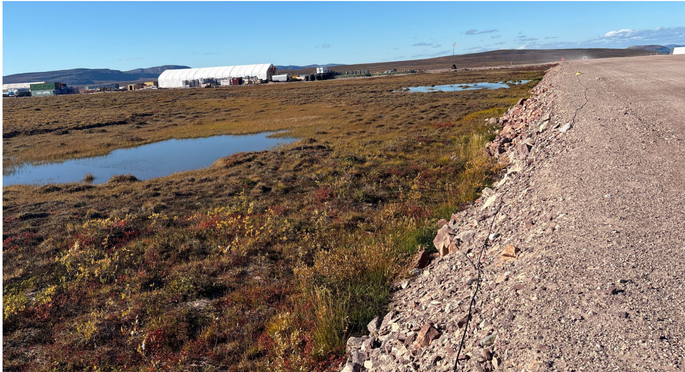
M-24: South end – Note ponding water at the toe of the embankment
