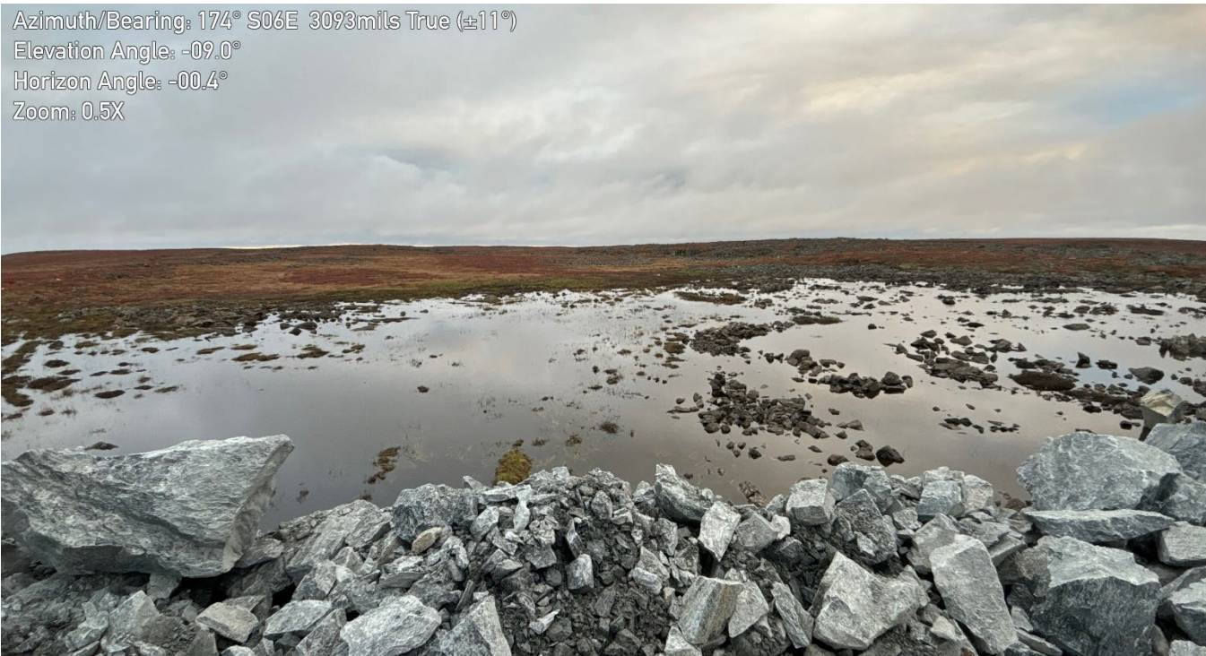
G-241: Southern slope – Note previous ponding water
