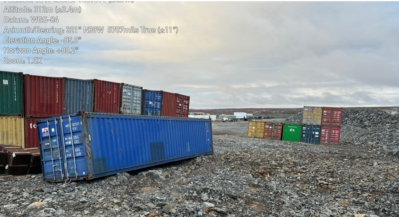
G-249: Large settlement present – Potential for seacans toppling (Hazardous & Toxic)
