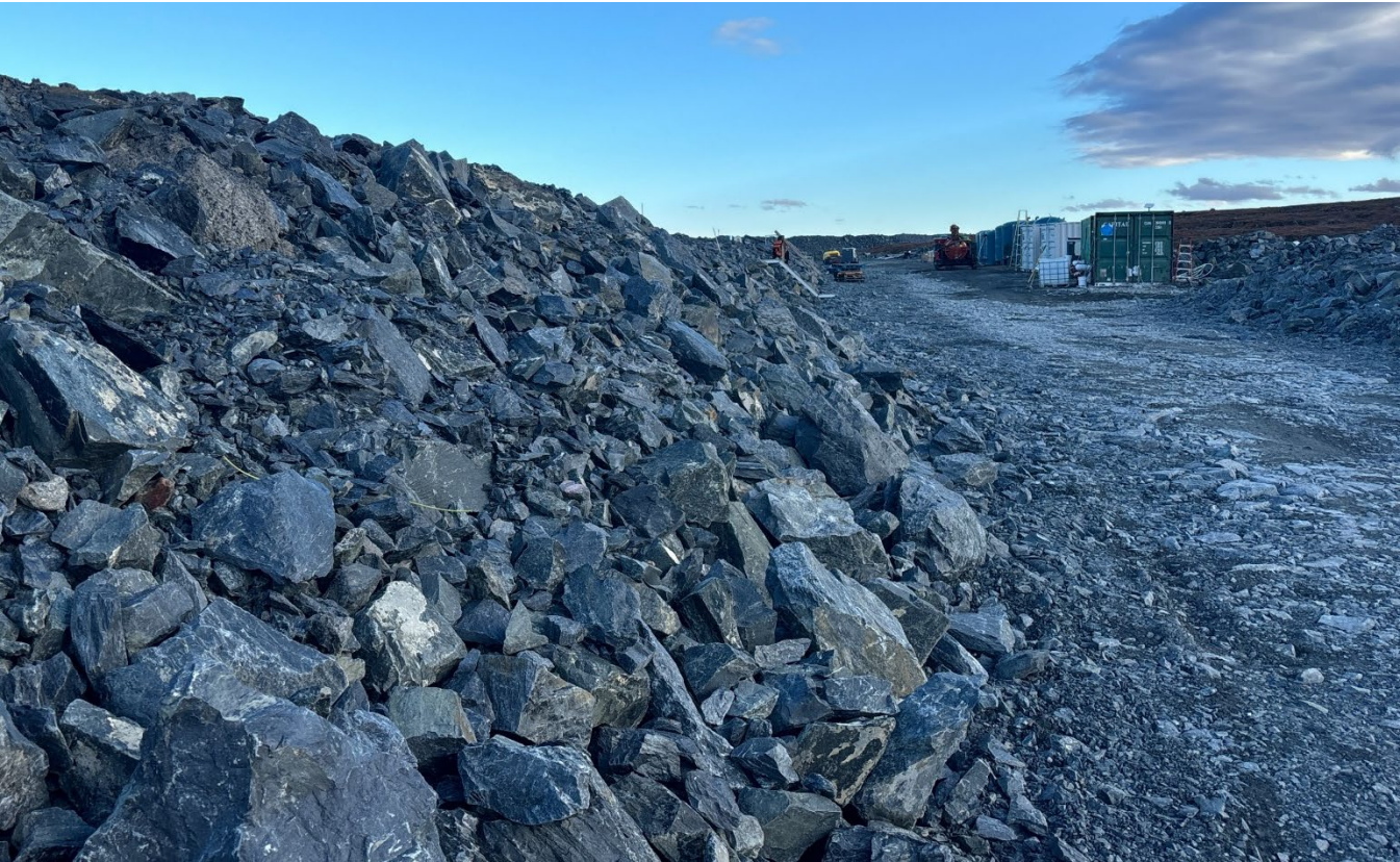
G-97: Northern most treatment pond slope – Note pond slope is oversteepended
