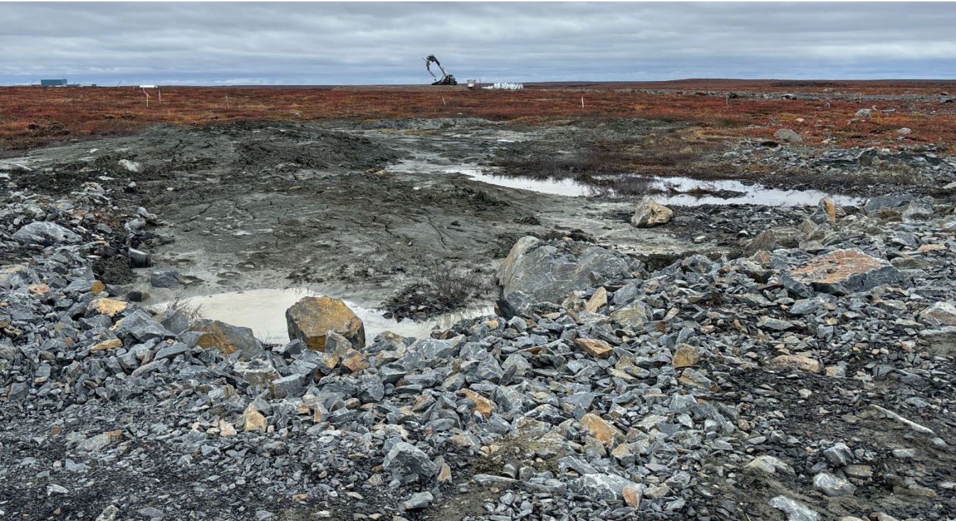
G-258: Camp pad – Note Erosion, ponding and lack of aggregate material
