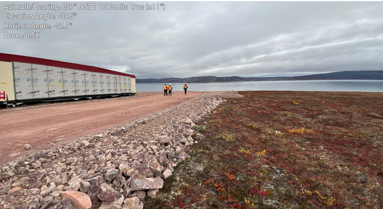
M-4: Access road under construction – Note fill is too thin
