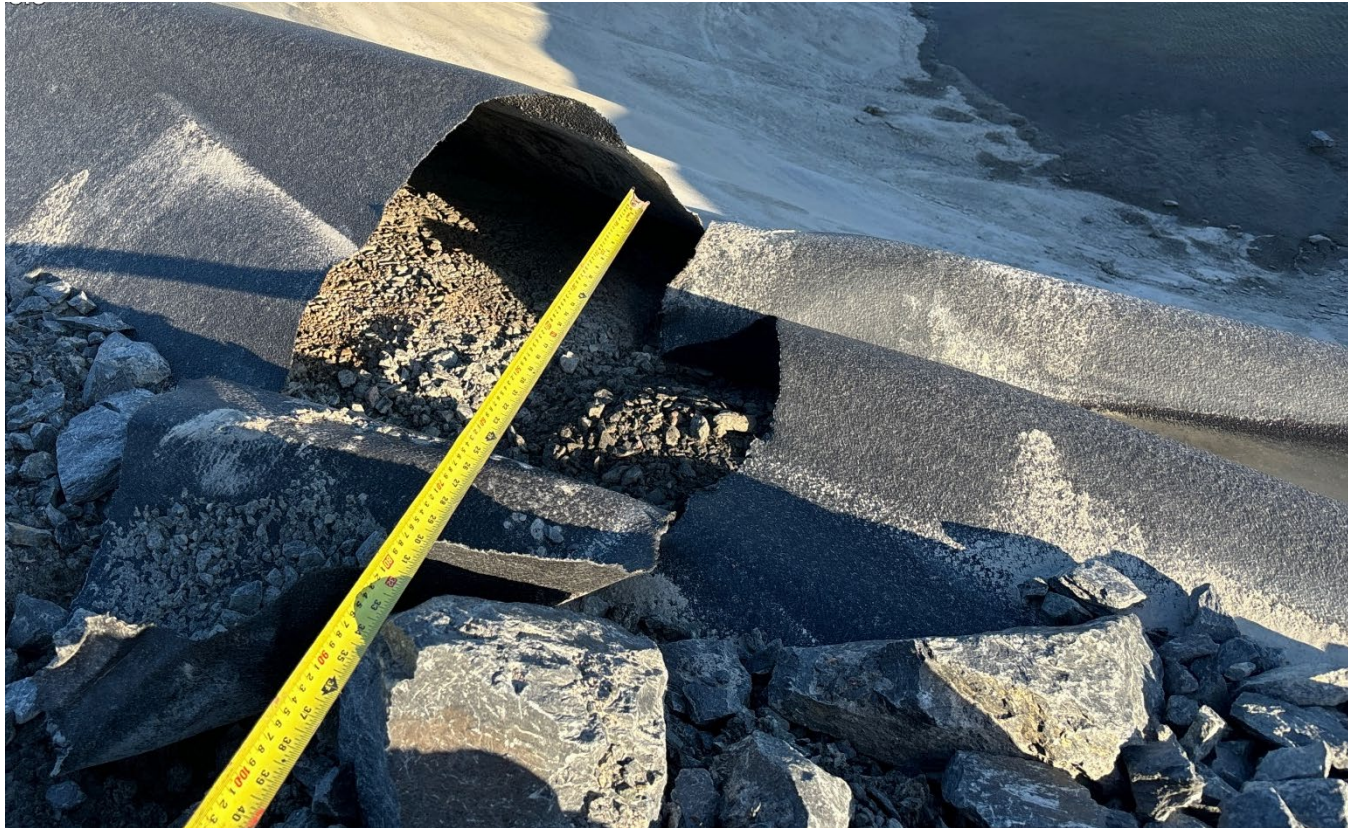
G-93: Liner tie-in damage
