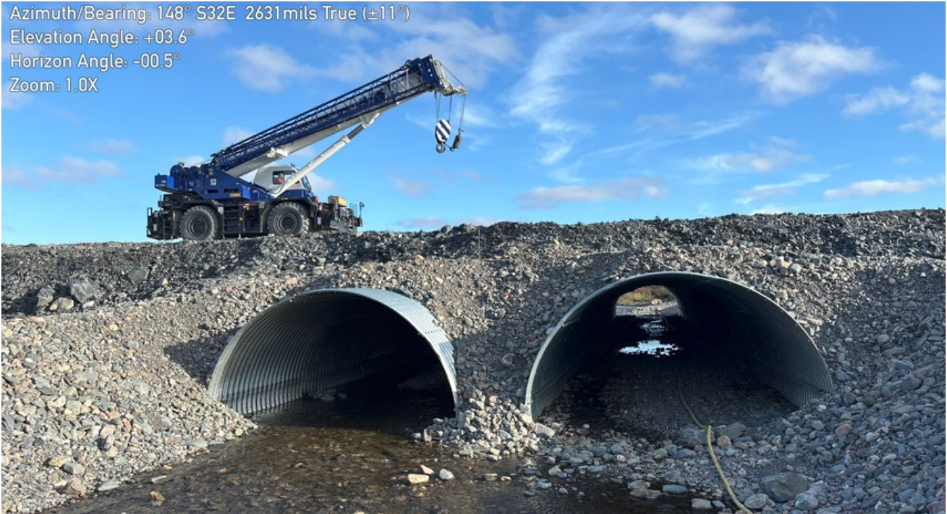
G-118: Gander Crossing Large Culverts, facing South - Note Flow into Arches
