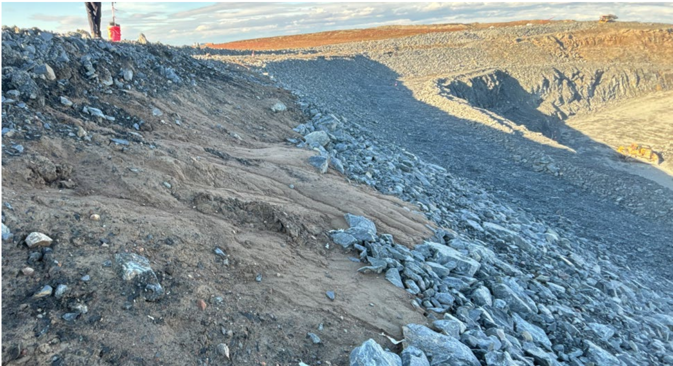
G-88: Crest of western wall, facing north – Note thermal erosion and erosion gulleys
