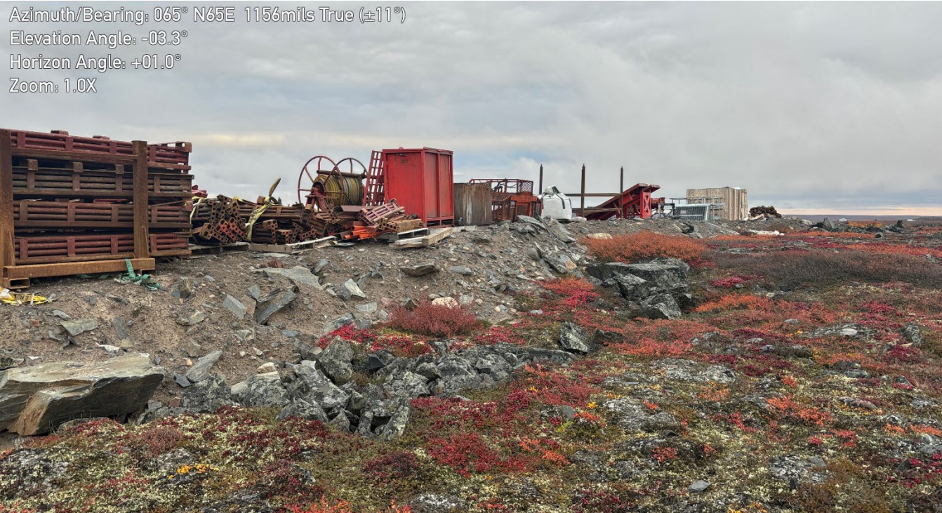
G-178: Western most laydown area, facing NW – Note equipment to close to pad edge
