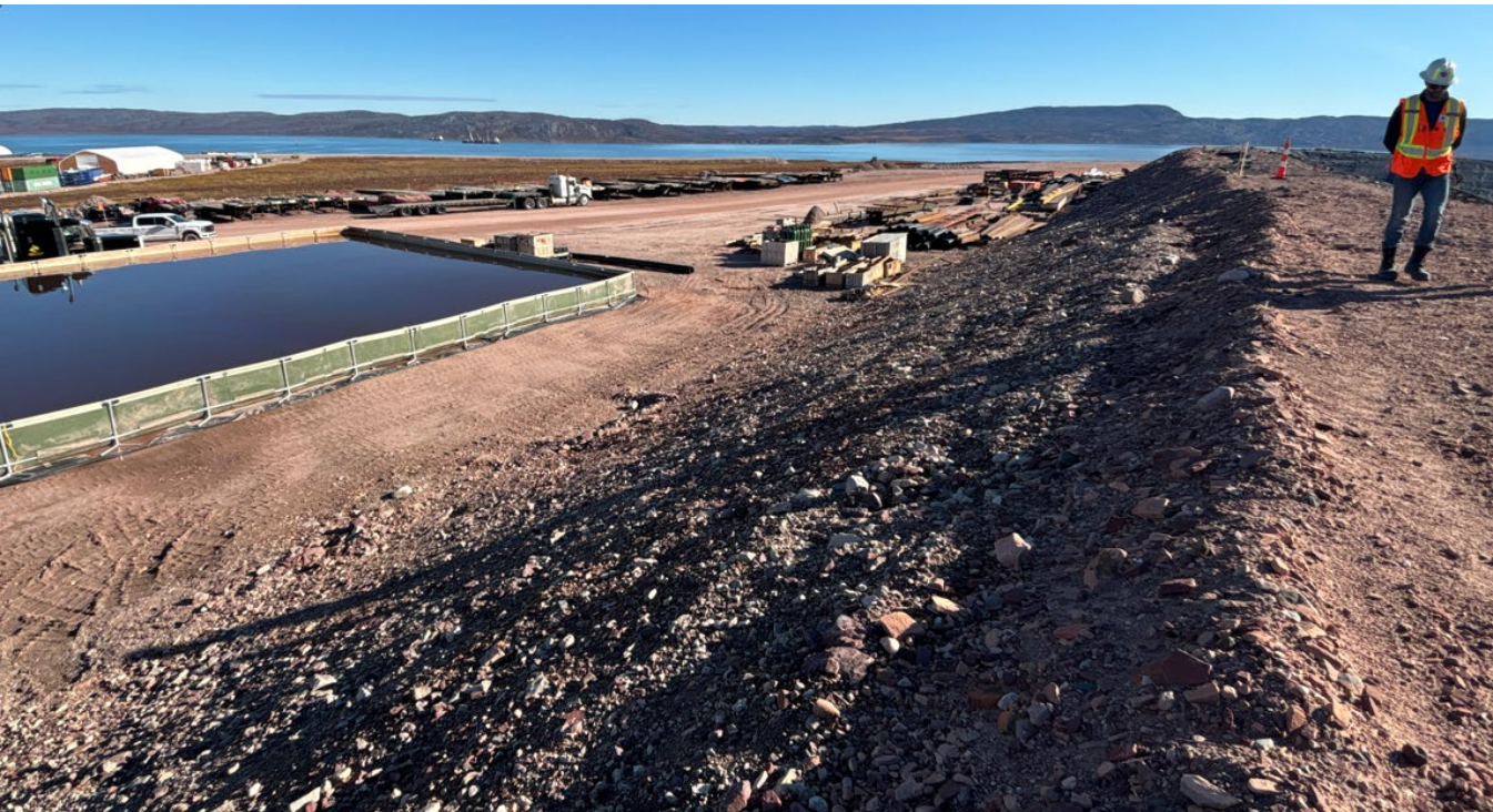
M-31: Berm slopes are too steep
