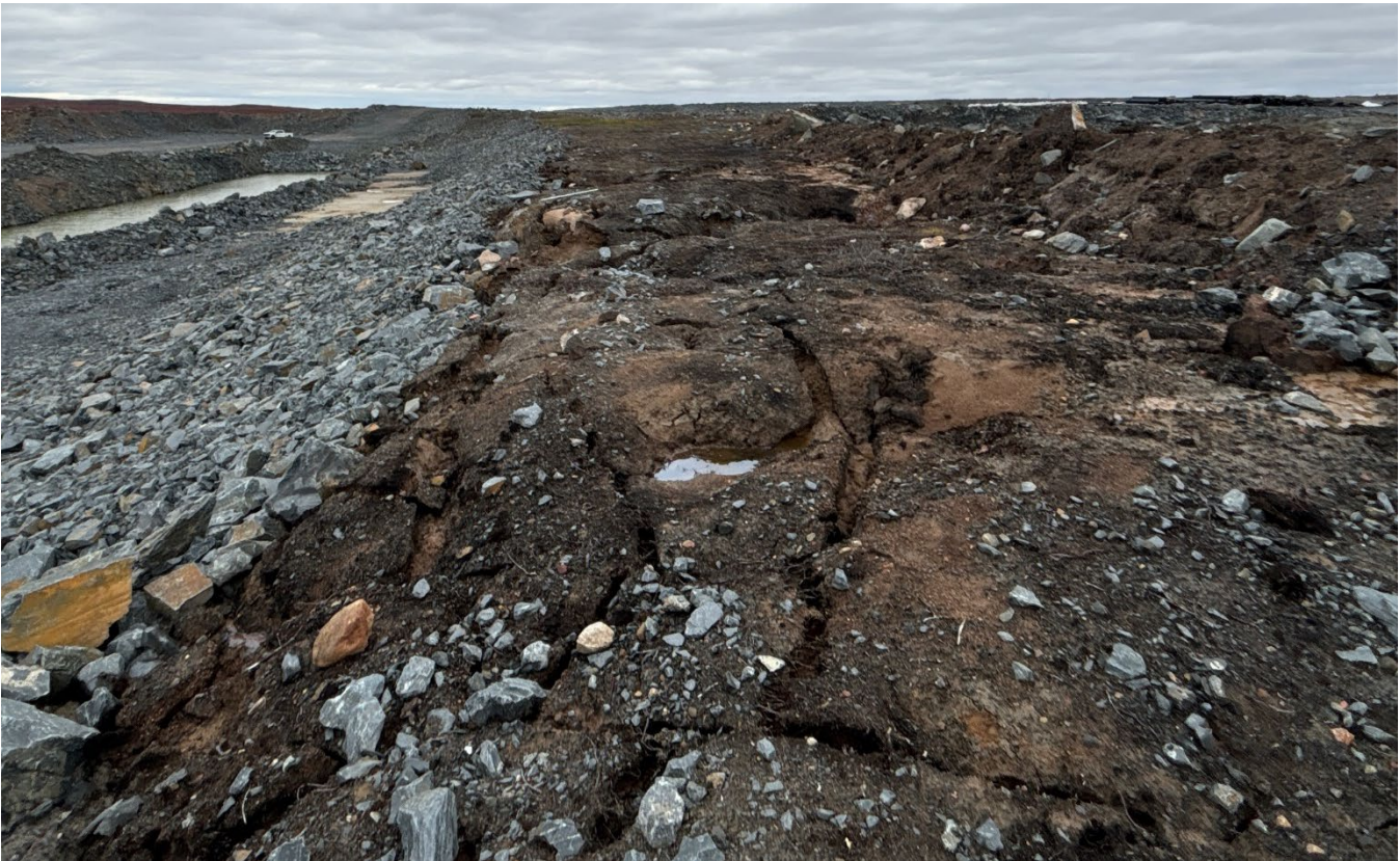
G-209: NE slope, facing NW – Note tension cracking
