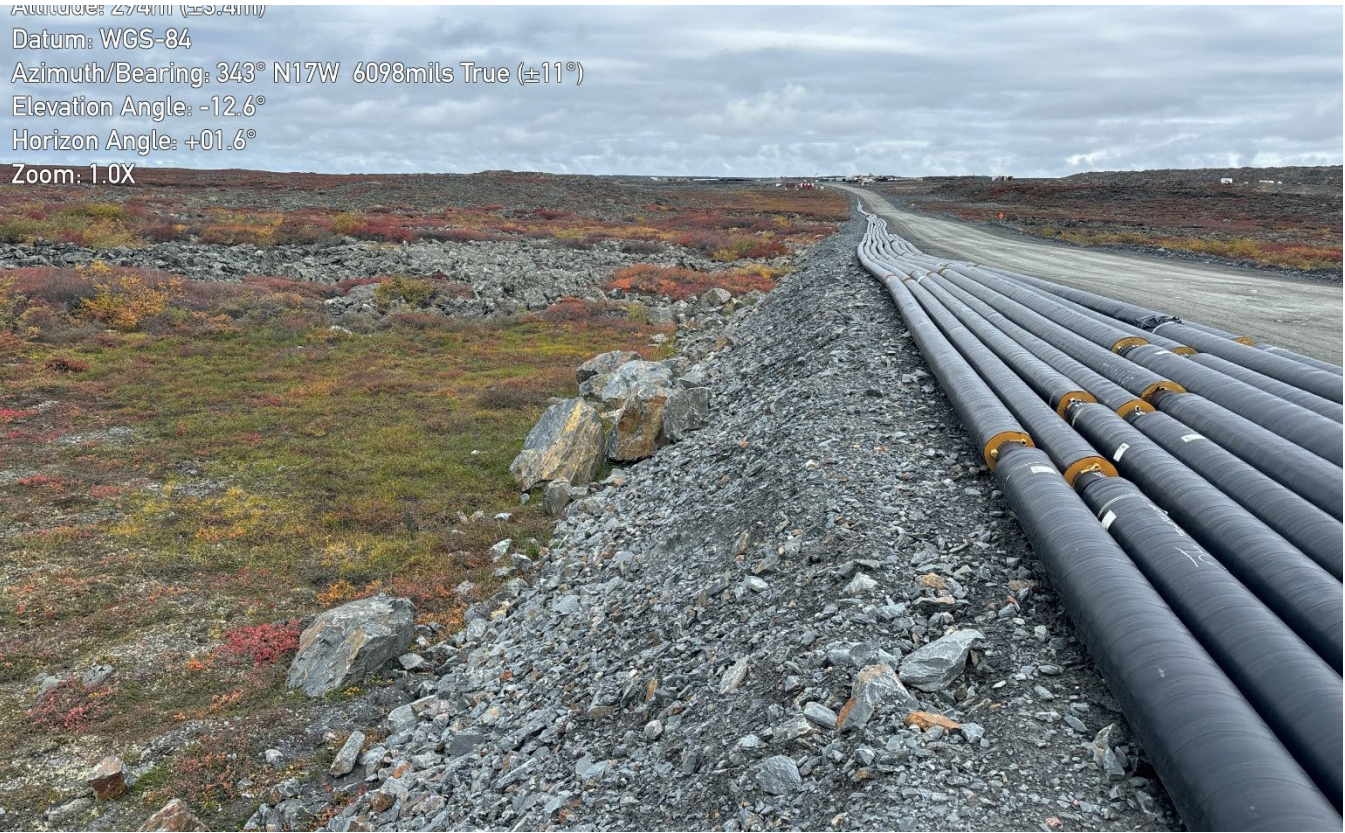
G-235: General pipe layout – Note large blast rock at toe
