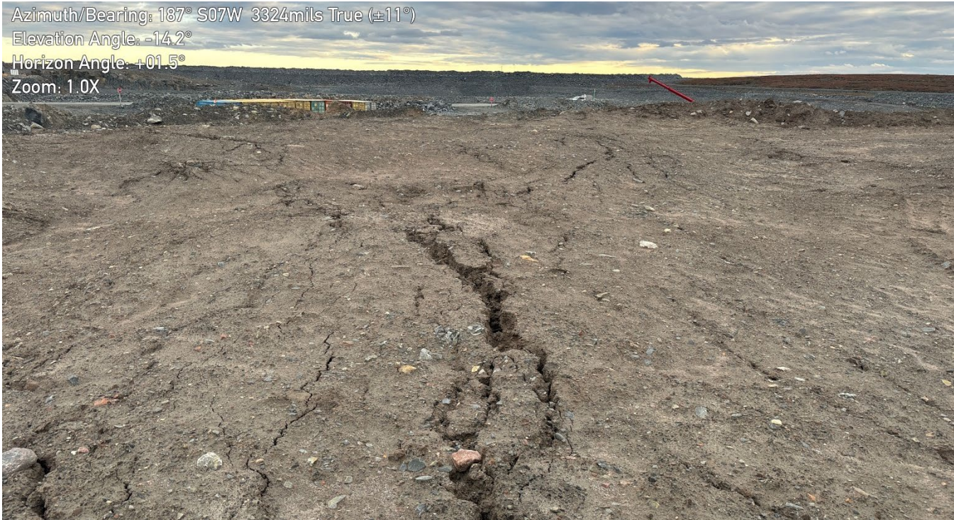
G-115: Stockpile, facing south – Note tension cracks
