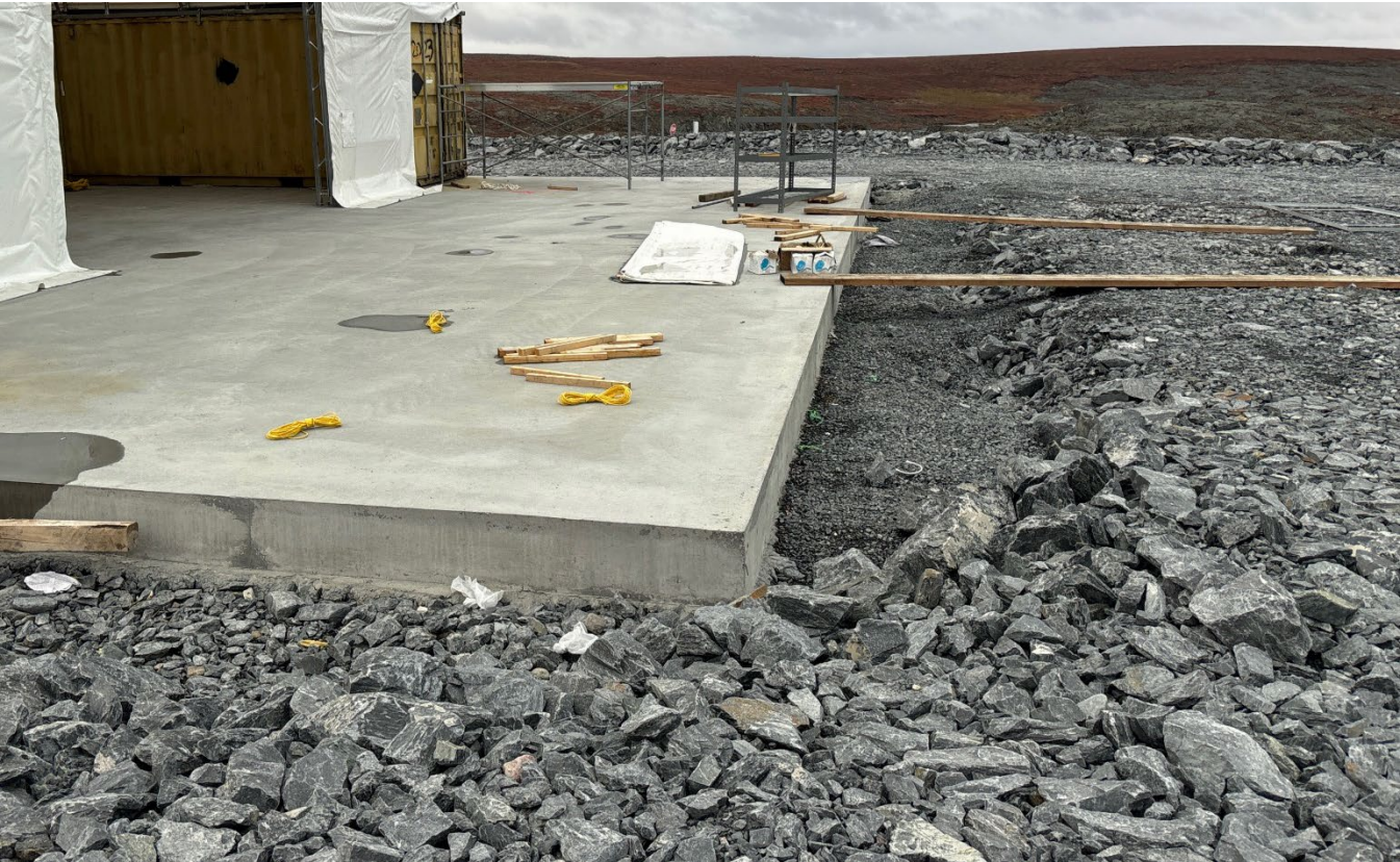
G-167: Concrete slab construction
