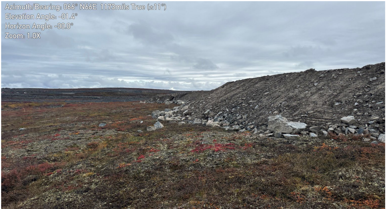
G-195: Looking East – Note oversteepened slopes
