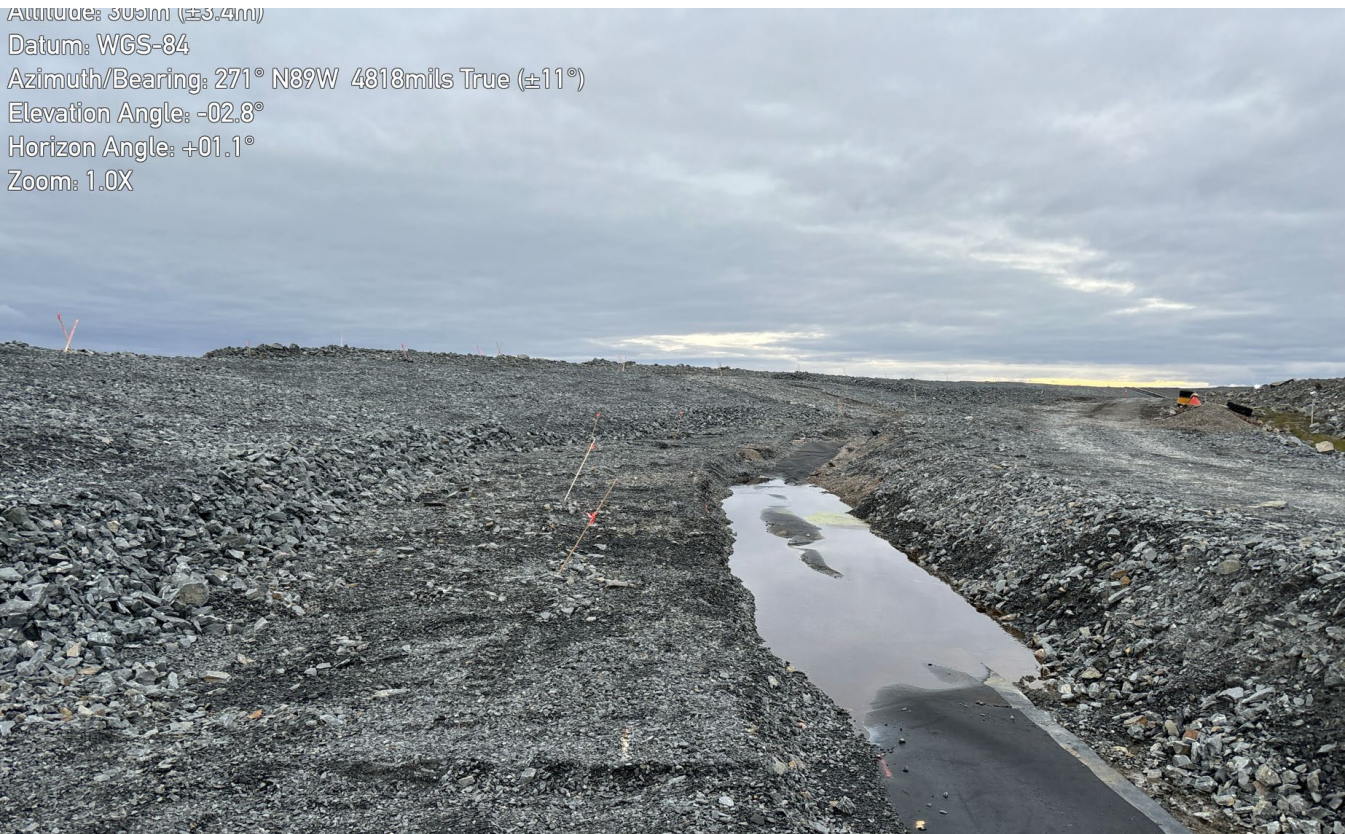
G-227: SE end, facing west – Note ponding water over liner
