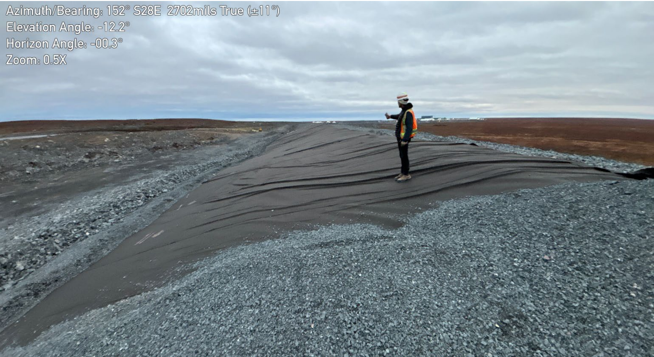
G-219: Upstream face. Previous liner fix. Looking SE (between Sta 0+150 and 0+200)
