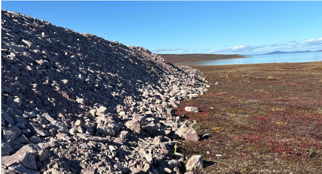
M-16: Airstrip extension, northern end – Slopes are too steep
