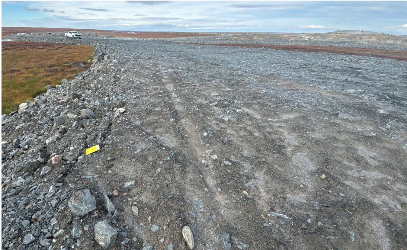
G-78: Diversion, facing north – Note thickness below 1m
