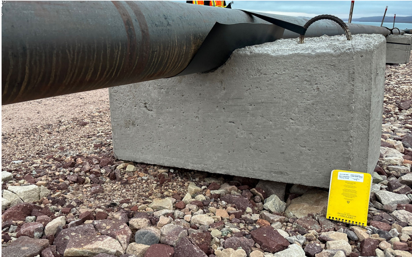
M-72: Typical bracing
