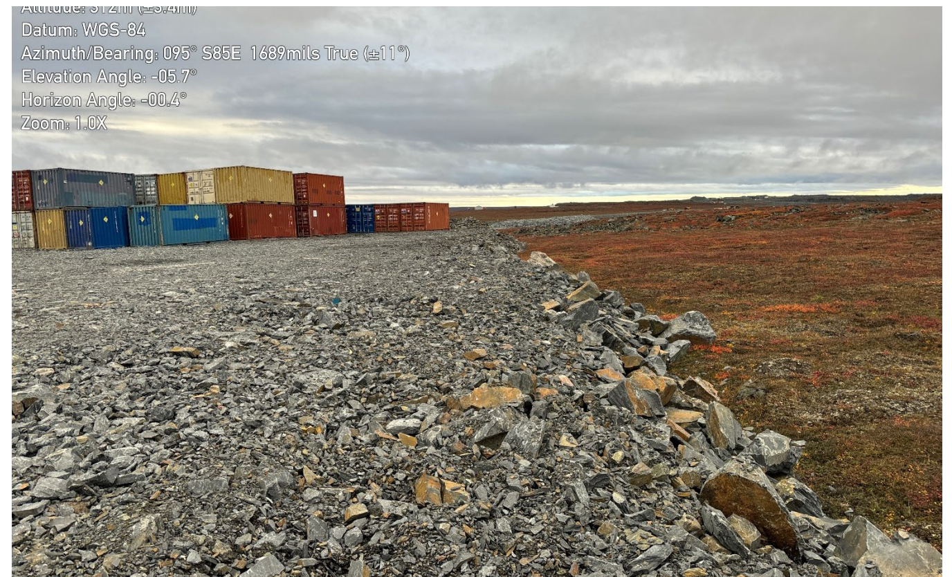
G-173: Laydown area at the northern side of the all-weather road – Note oversteepend slopes
