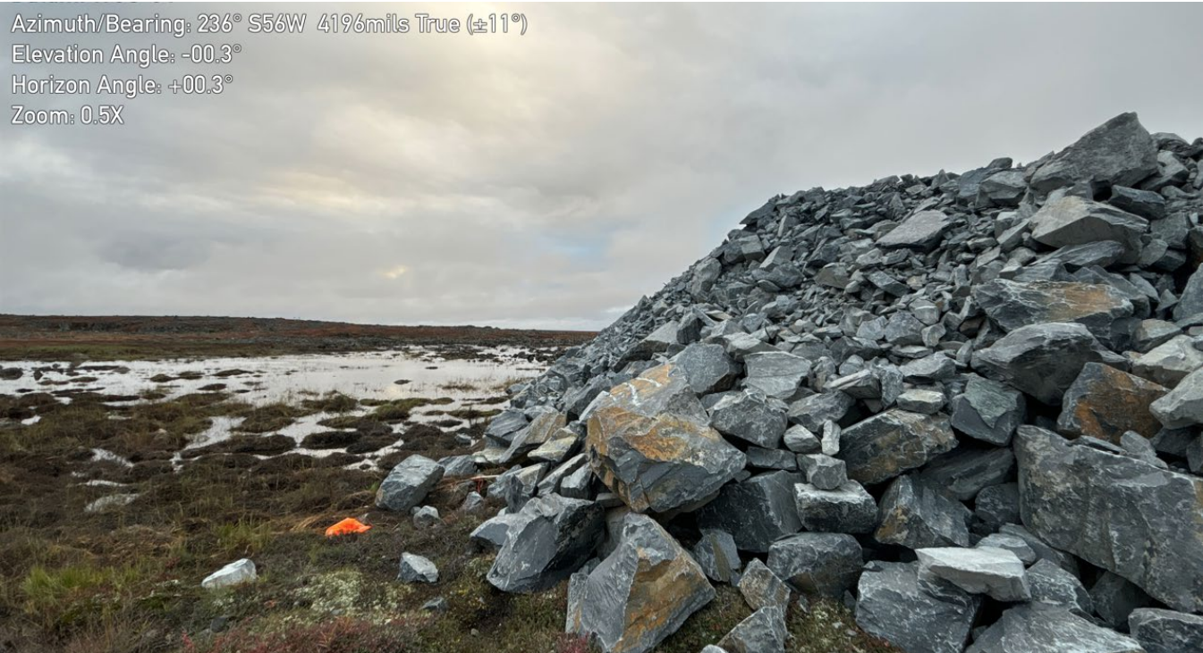
G-240: Eastern slope - Oversteepened
