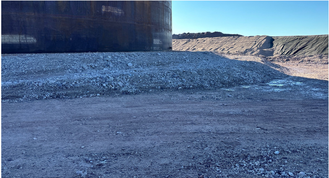
M-36: Typical tank pad
