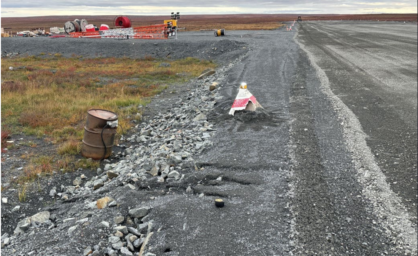
G-47: Eastern laydown area, facing SE – Note erosion pathways
