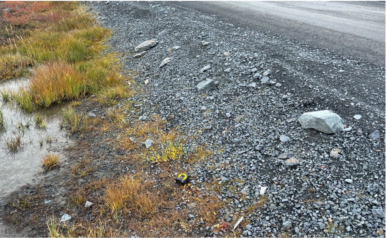
G-61: Typical thickness of the airstrip access road embankment, facing exploration camp
