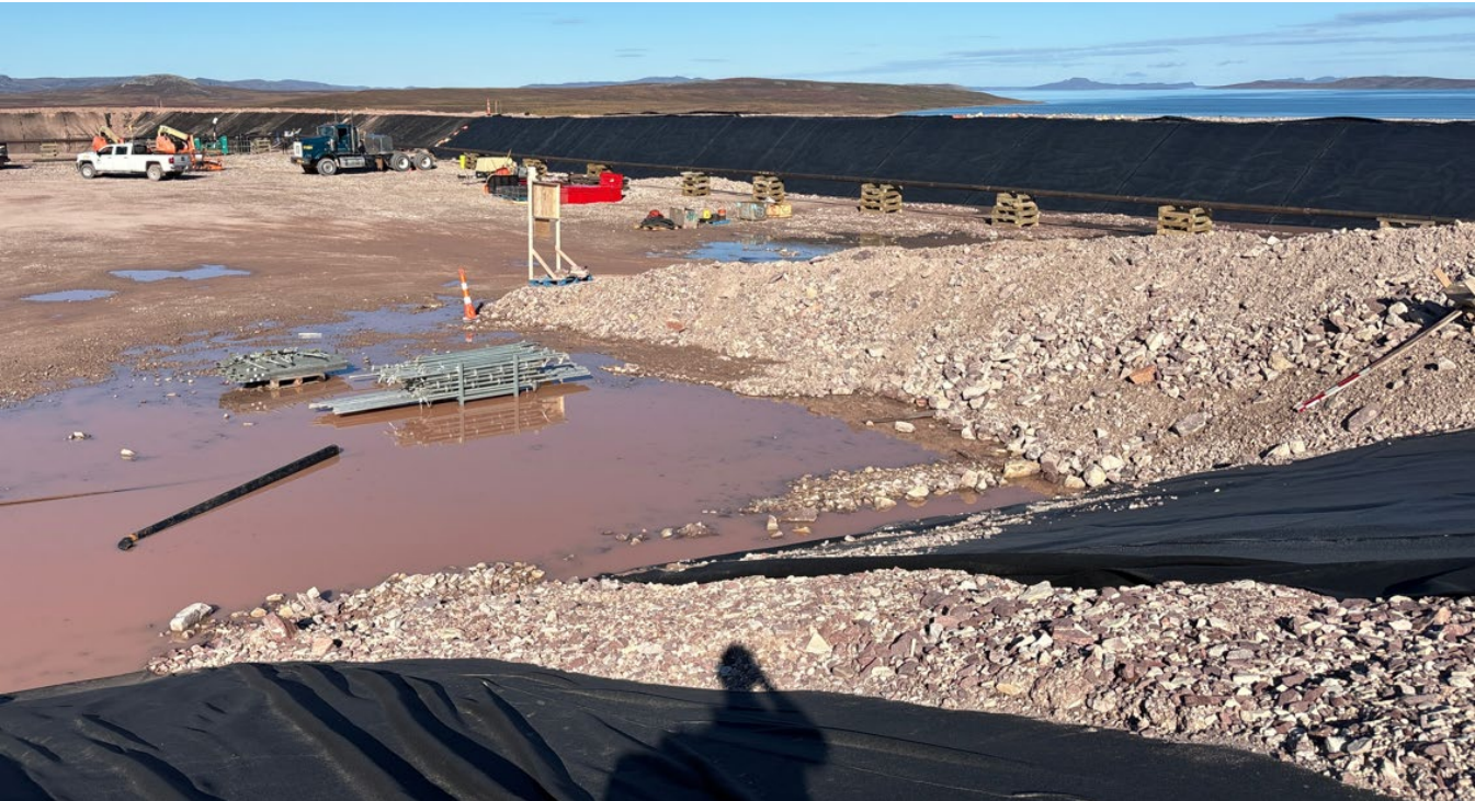
M-29: Ponding water due to the ramp access
