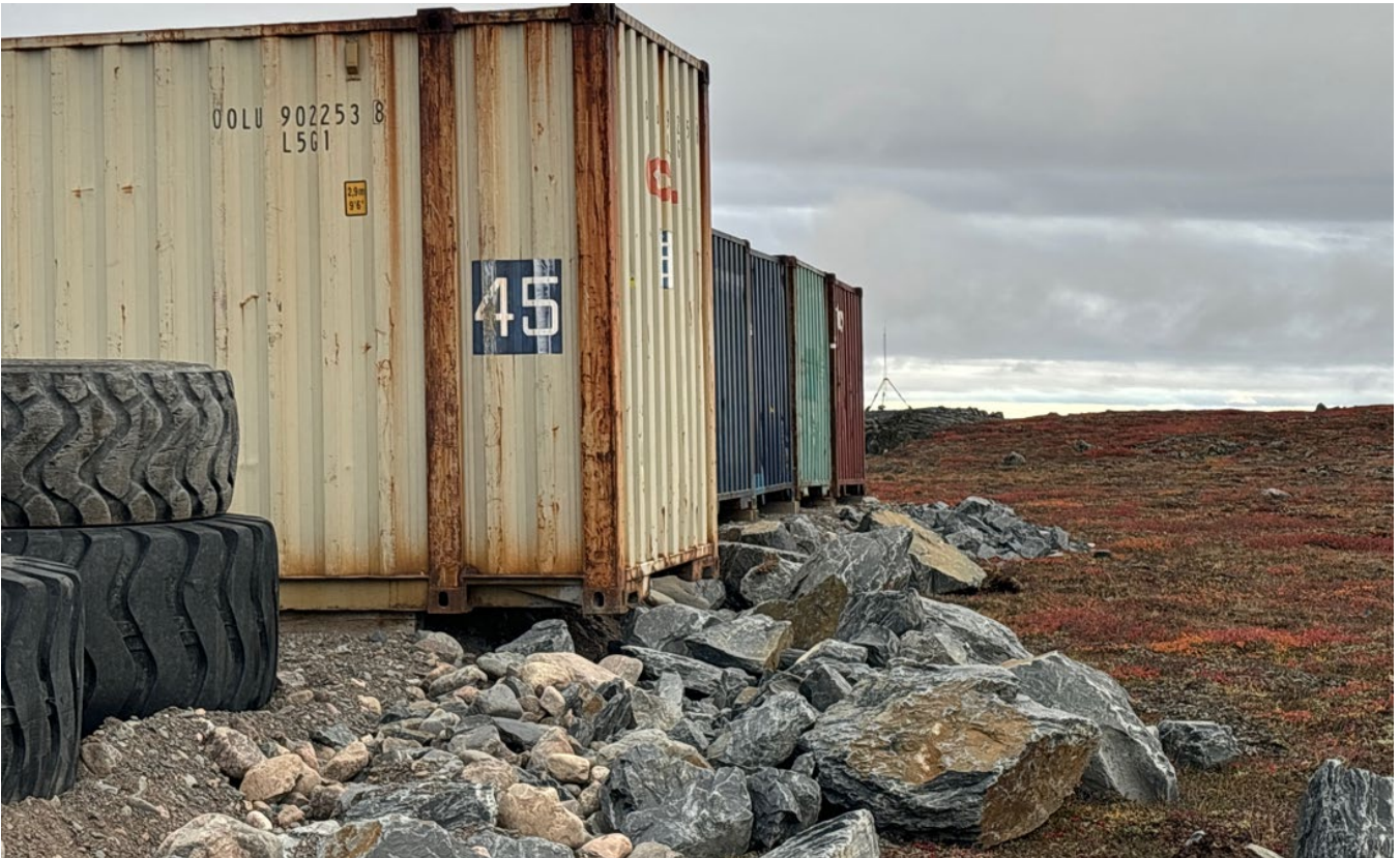
G-171: Western side of pad – Note Seacans and materials close to pad edge. Pad less than 0.5m in some areas
