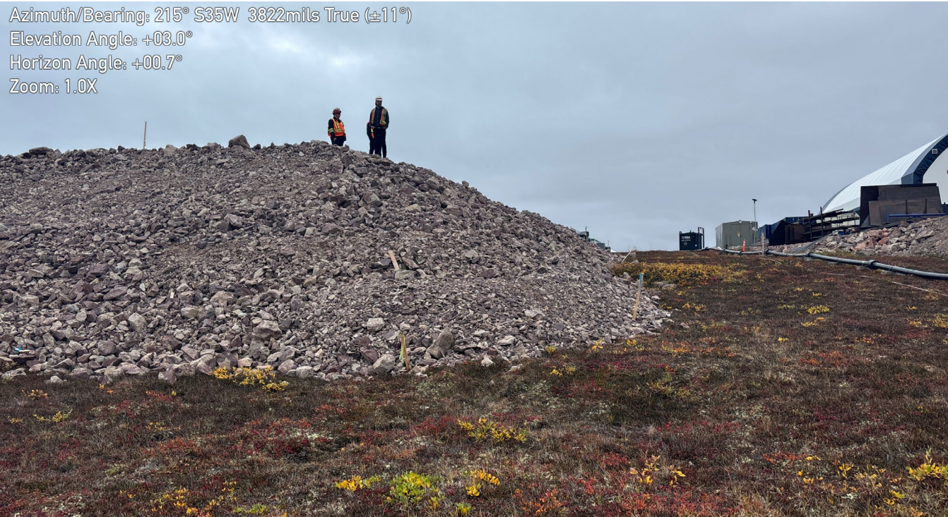
M-2: North slope – Note fill slopes are too steep
