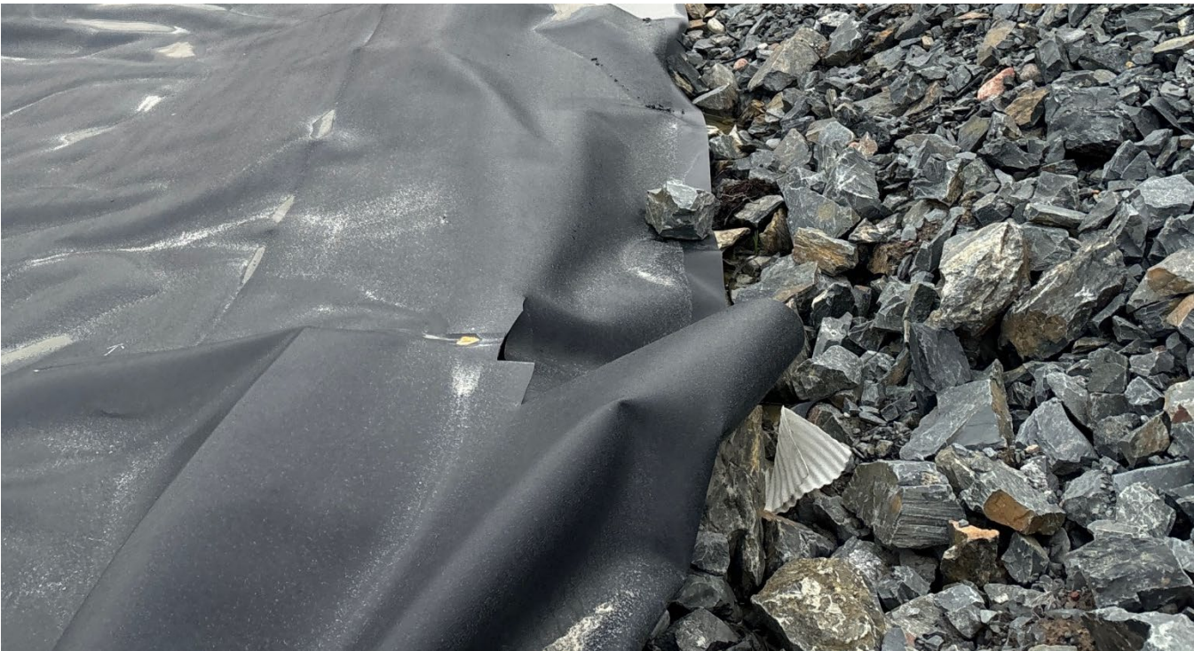
G-153: Zoomed in, No tie in and liner damage
