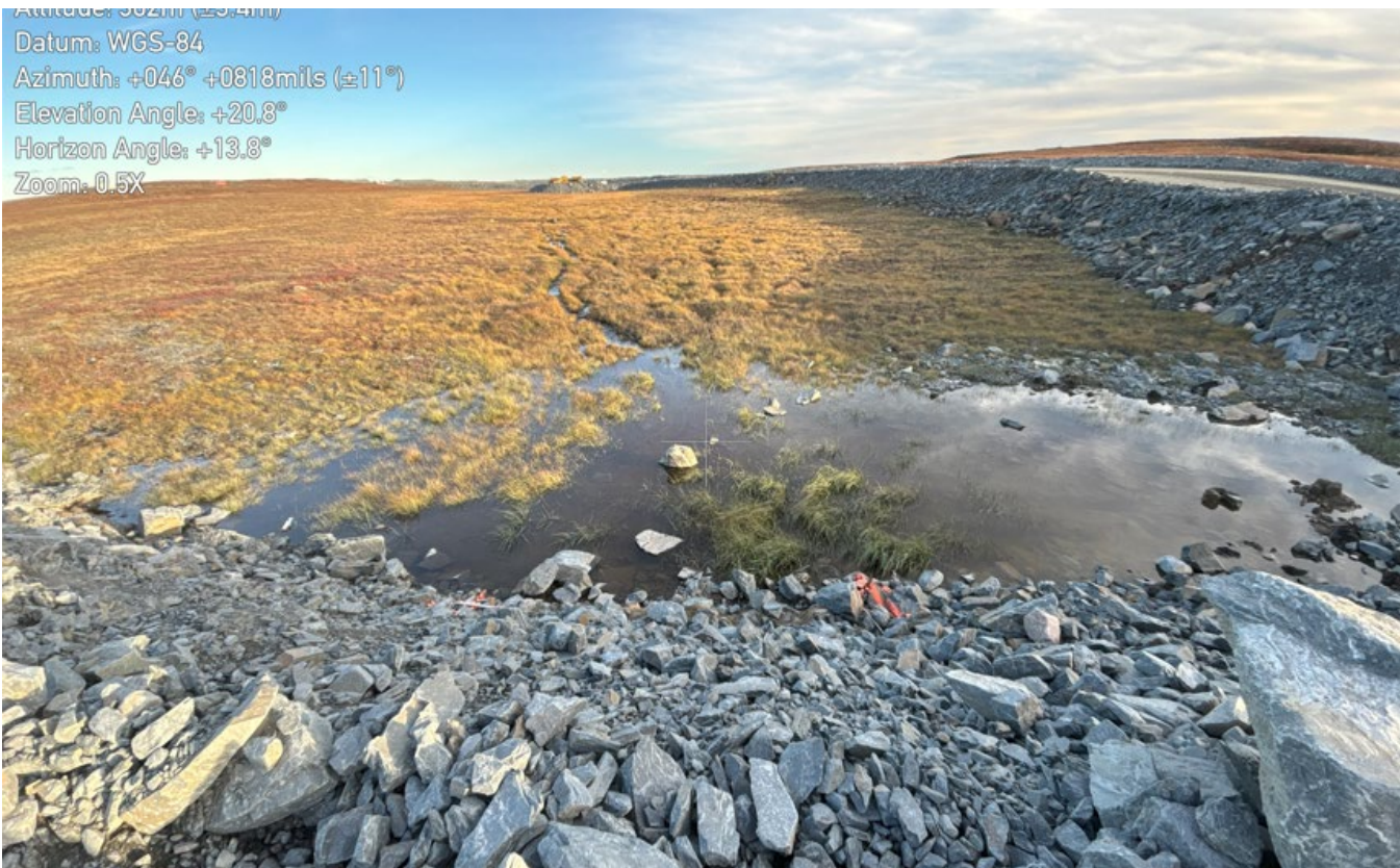
G-65: Eastern Side of Echo Pit Access Road Looking South – Note Culverts are Blocked. Ponding Water
