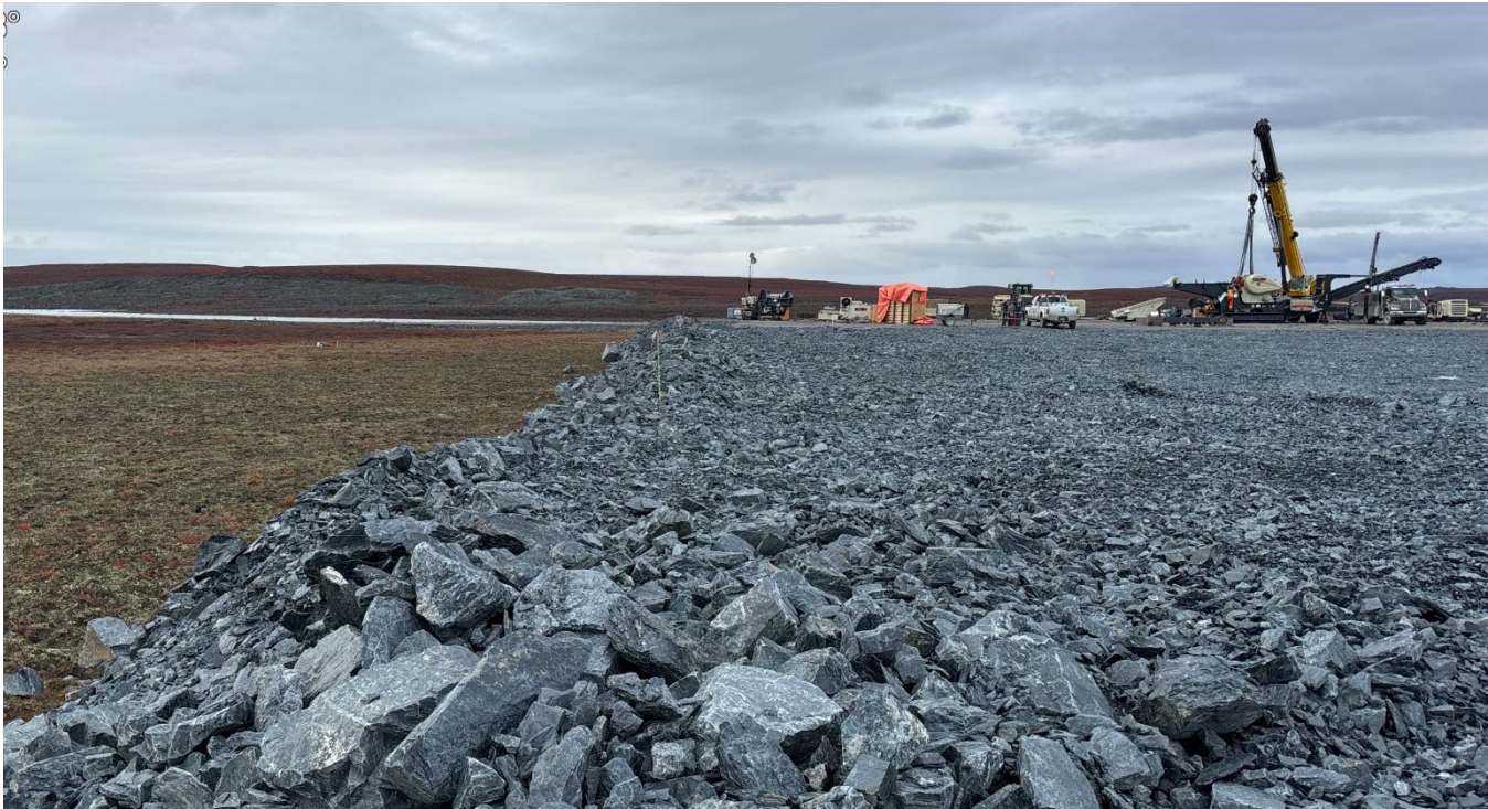
G-32: NW Apron, facing NE – Note thickness of pad less than 0.6m
