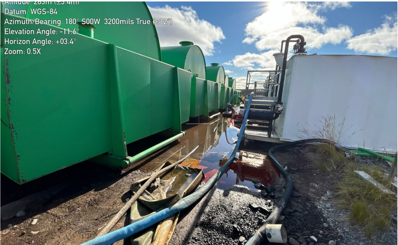
G-11: Fuel tank containment. Ponding water
