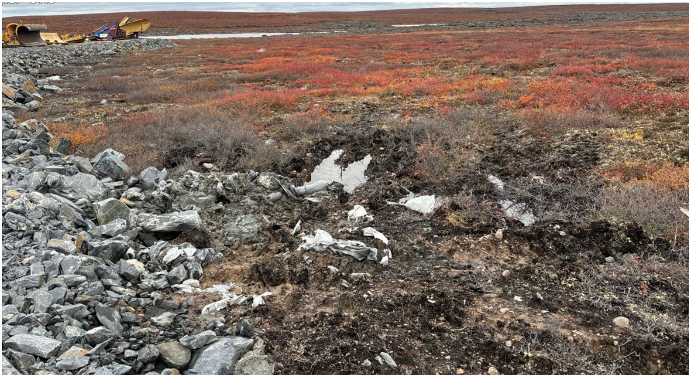
G-259: Camp pad edge, facing east – Note tundra around the pad is disturbed and degraded
