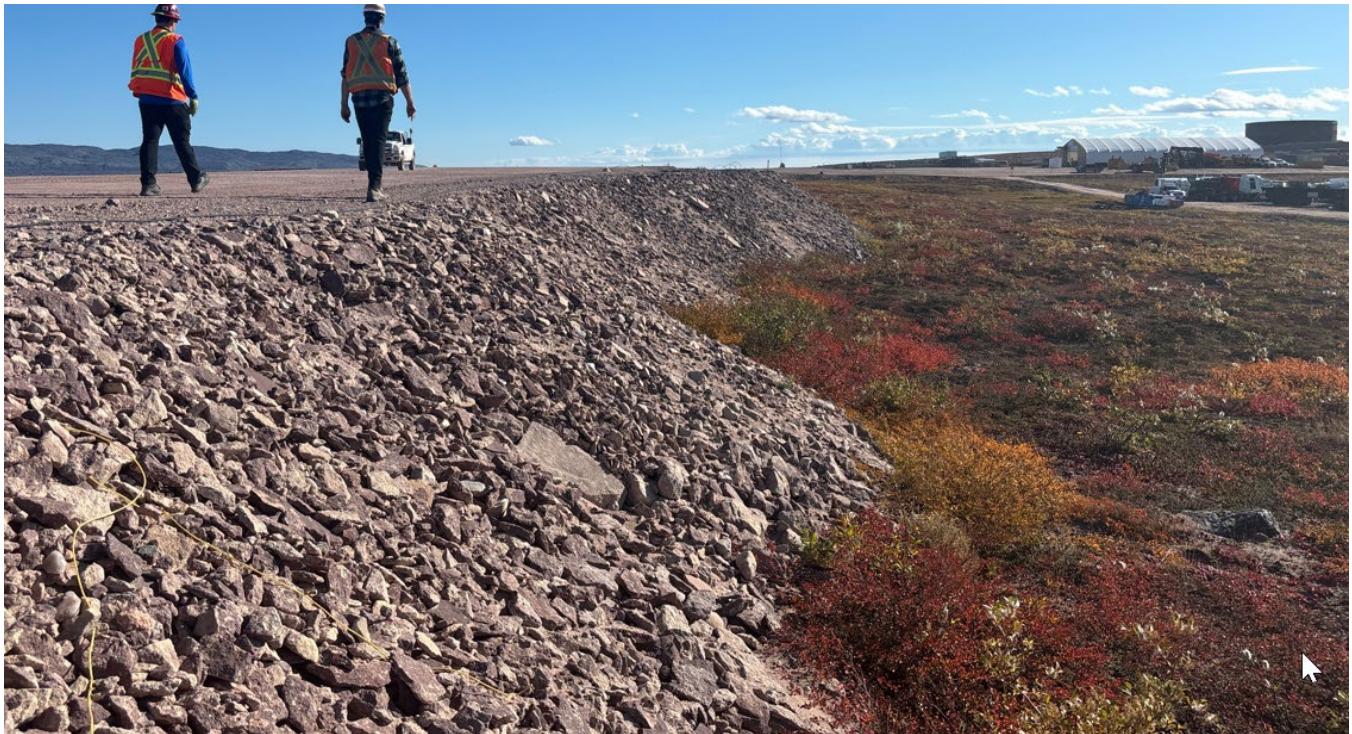
M-14: Airstrip, western side – Typical slope of the embankment - some sections are too steep
