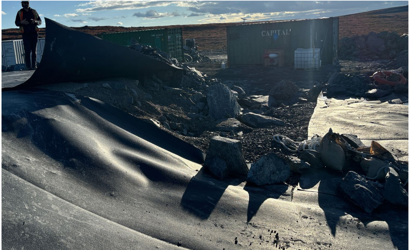
G-96: Pond slope – Note inappropriate material on liner
