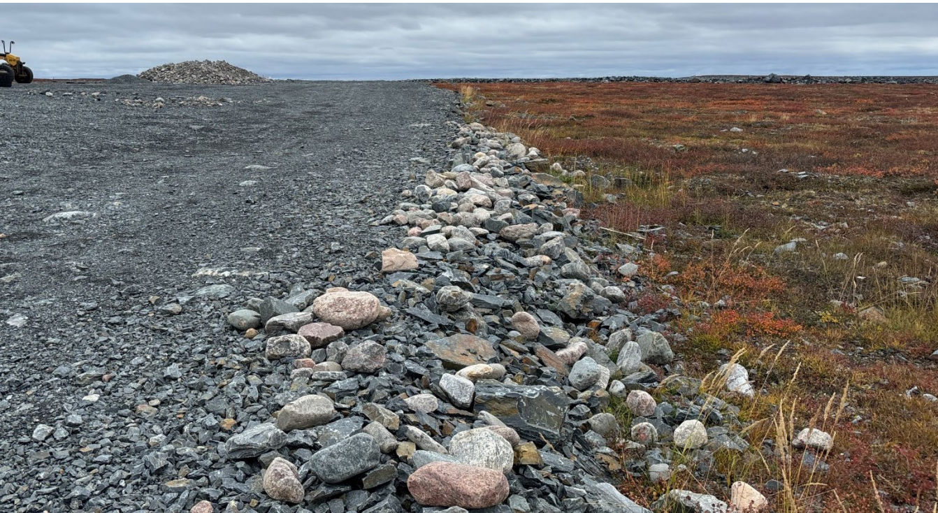
G-256: Edge of road opposite camp pad – Note thickness
