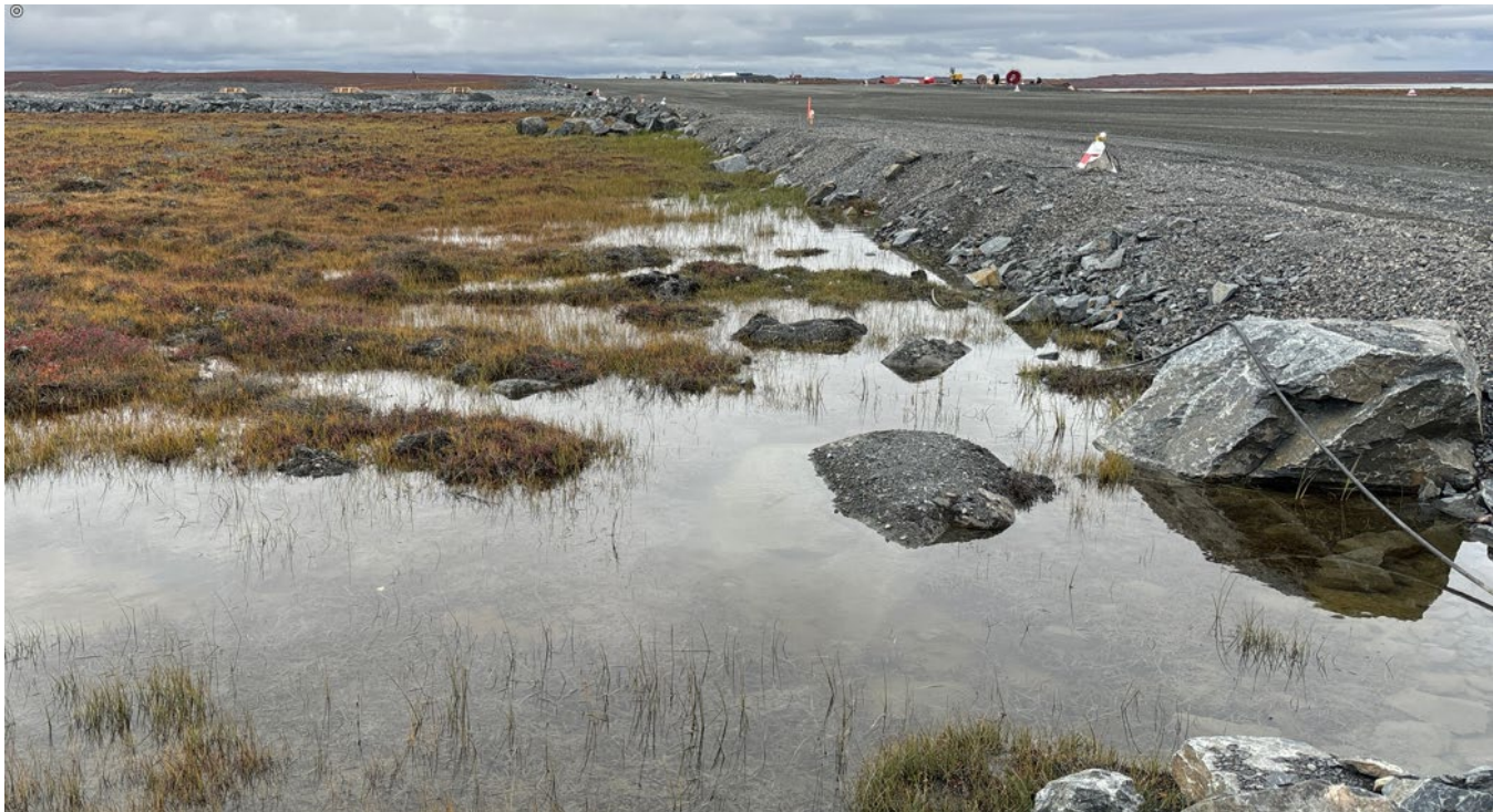
G-41: Toe of airstrip, looking NW – Note ponding water
