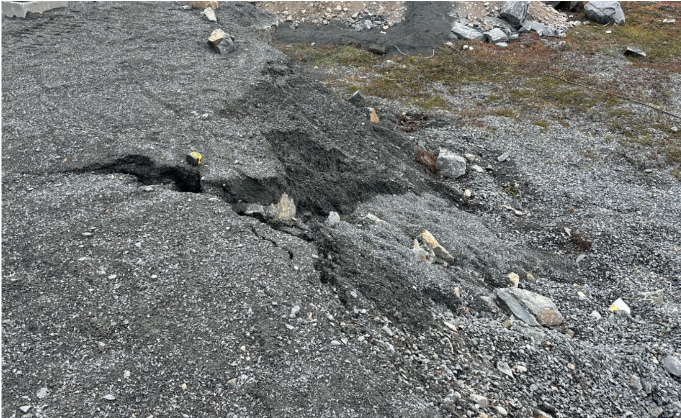
G-57: Laydown area erosion gullies
