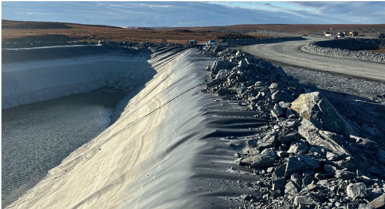
G-91: Pond Slopes are oversteepend and no spillway present
