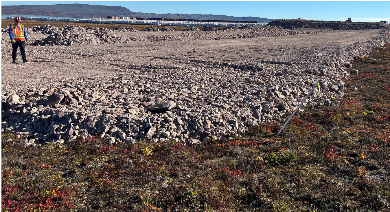
M-18: Northernmost end of airstrip extension – 0.8m lifts
