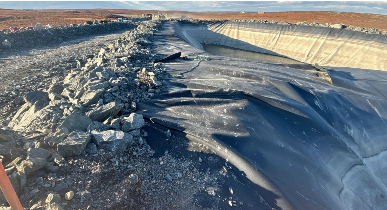
G-92: Pond tie-in – Inappropriate over-liner material (4" plus blasted rock) and no spillway present
