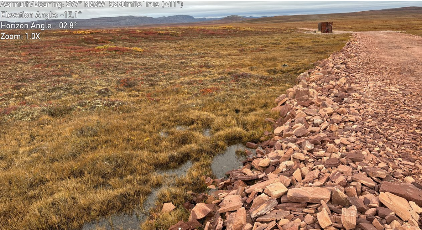
M-86: Embankment of the former explosives storage access road, facing W – Note ponding water at the western toe
