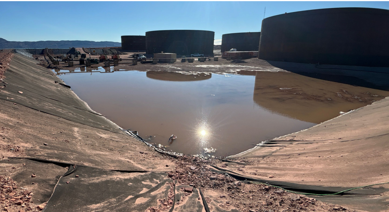
M-39: NW end of tank farm, facing south – Note ponding water
