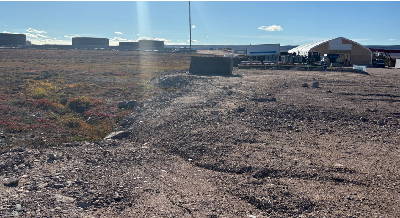
M-15: Airstrip, western side – Note erosion gullies
