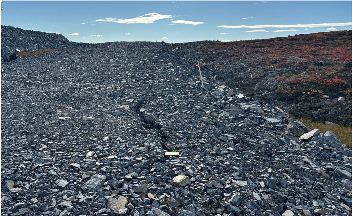
G-75: Diversion, facing SW – Note tension cracks
