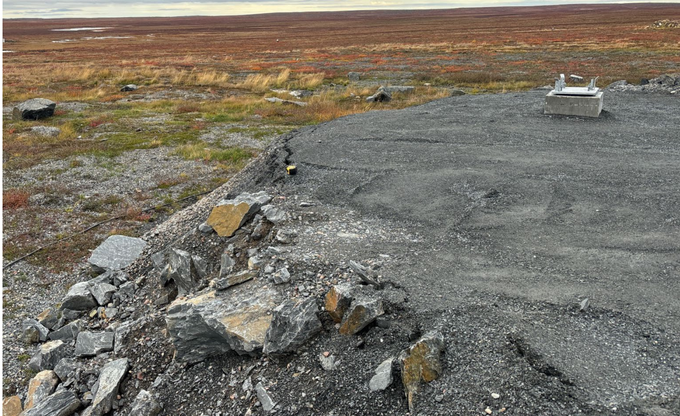
G-49: Eastern side apron, facing NW – Note tension cracking
