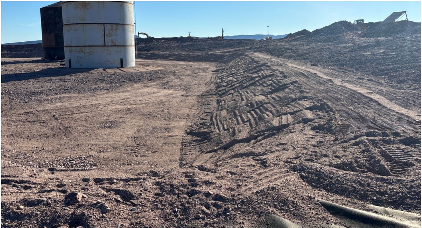
M-30: Liner fill is presented by sand, that is prone to the erosion – need to be buttressed with courser material
