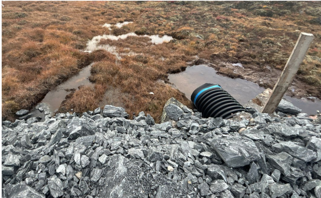
G-172: Damaged culvert causing water ponding at inlet
