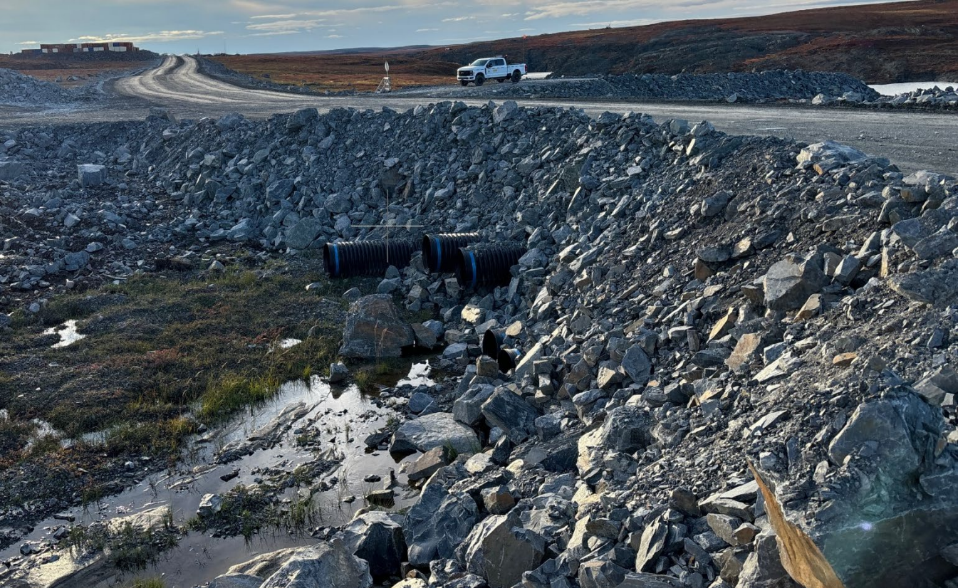
G-69: Haul road slope, facing west to crossing culverts
