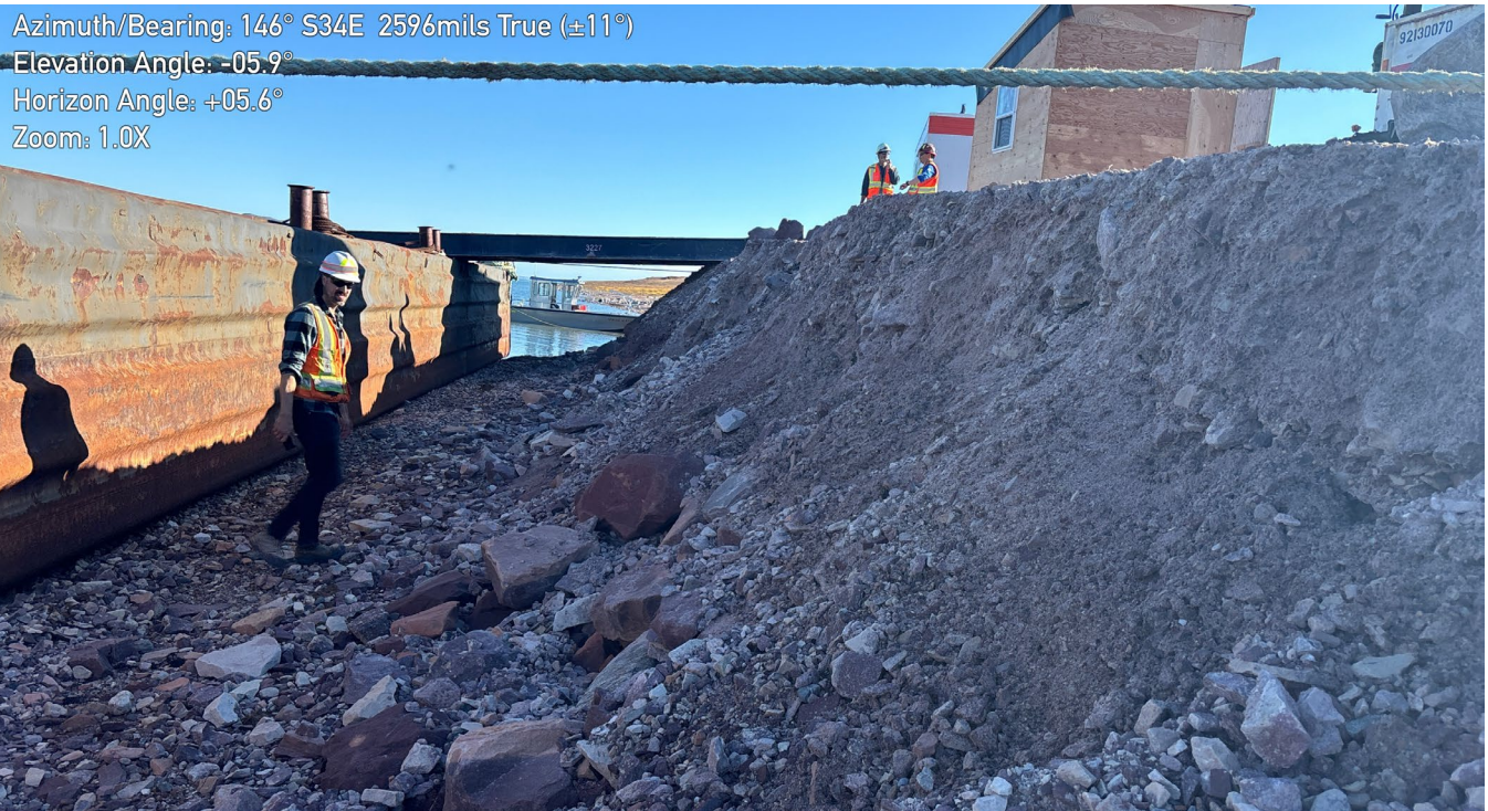
M-62: Embankment face - Note oversteepened slope
