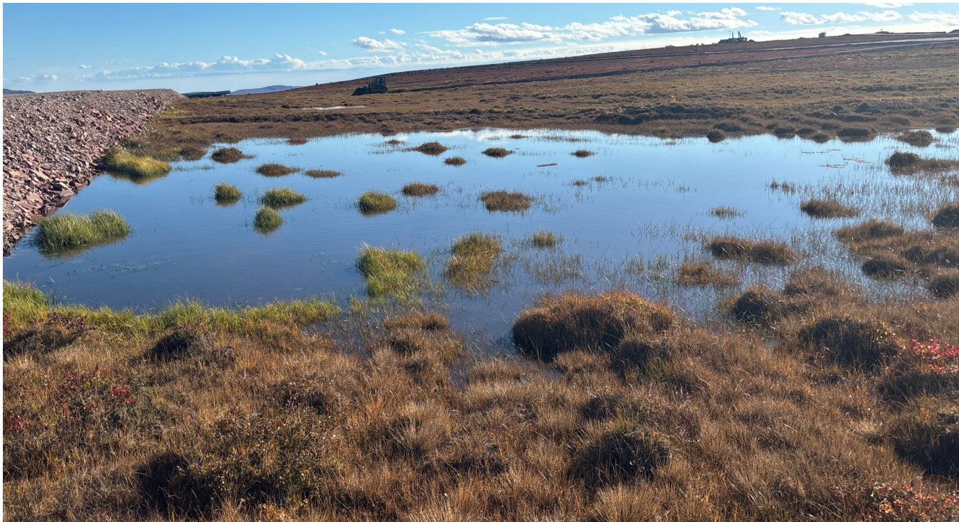
M-26: South end – Note ponding water at the toe of the embankment
