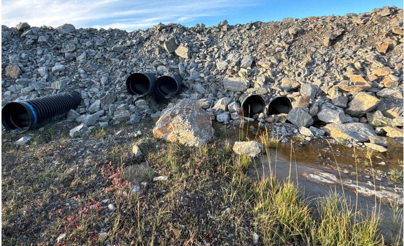
G-68: Southern Side of Echo Pit Haul Road – Note two Culverts are elevated approx. 0.5m from toe of embankment. Culverts partially blocked
