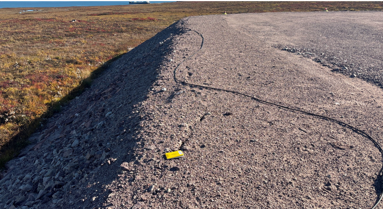
M-23: Southern end, facing SE – Note tension cracks
