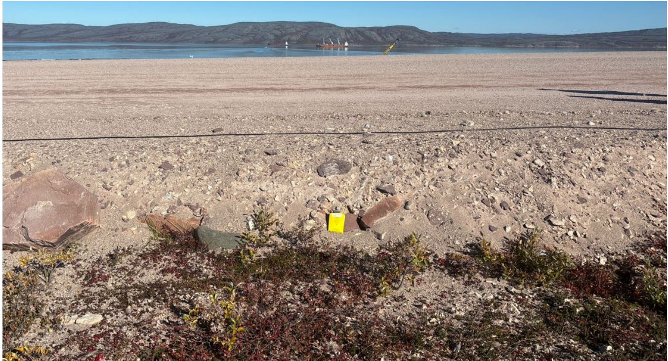
M-12: Airstrip, western side, facing East – Typical thickness of the embankment - some sections are too thin
