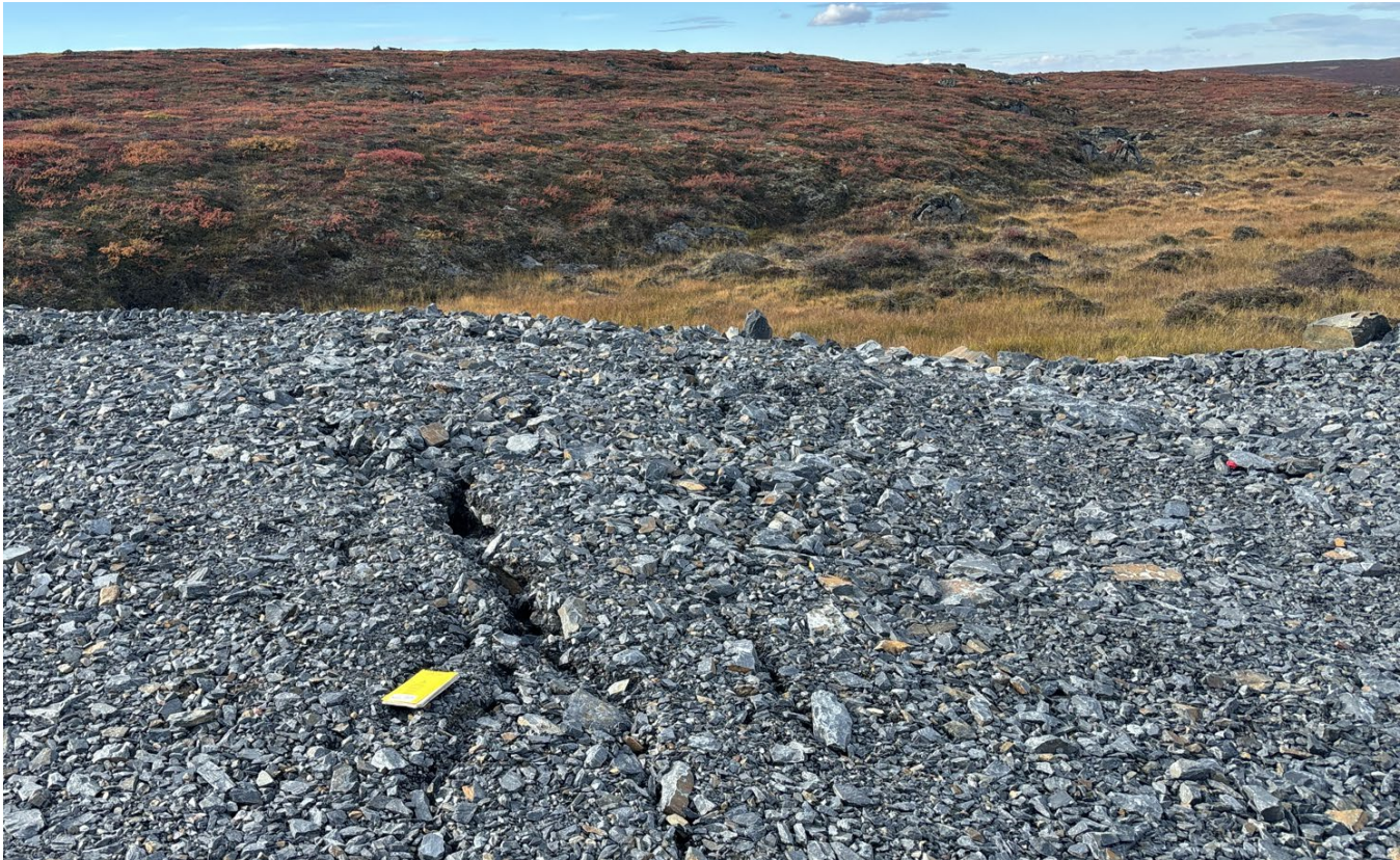
G-76: Diversion, facing north – Note tension crack
