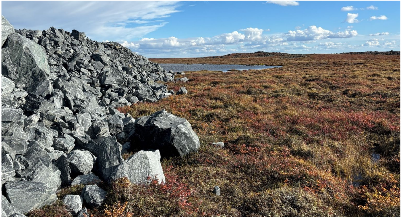
G-99: Southern end of WRSA, facing SE – Note oversteepened slopes
