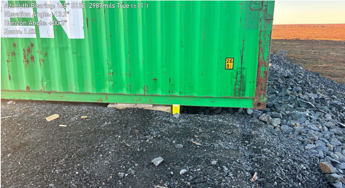
G-190: Western slope seacan – Note gap beneath seacan
