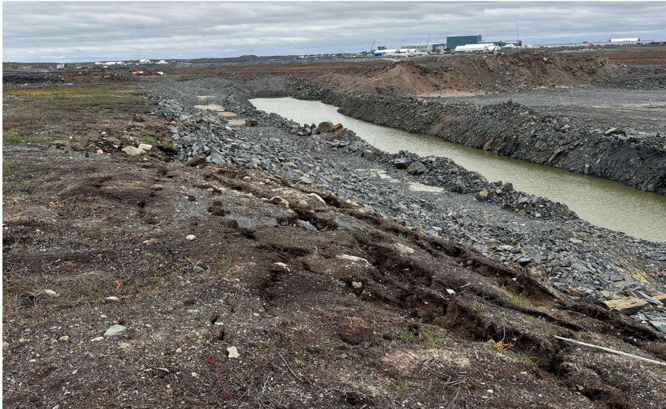
G-207: NE slope, facing south – Note thermal erosion and tension cracking due to lack of rockfill layer
