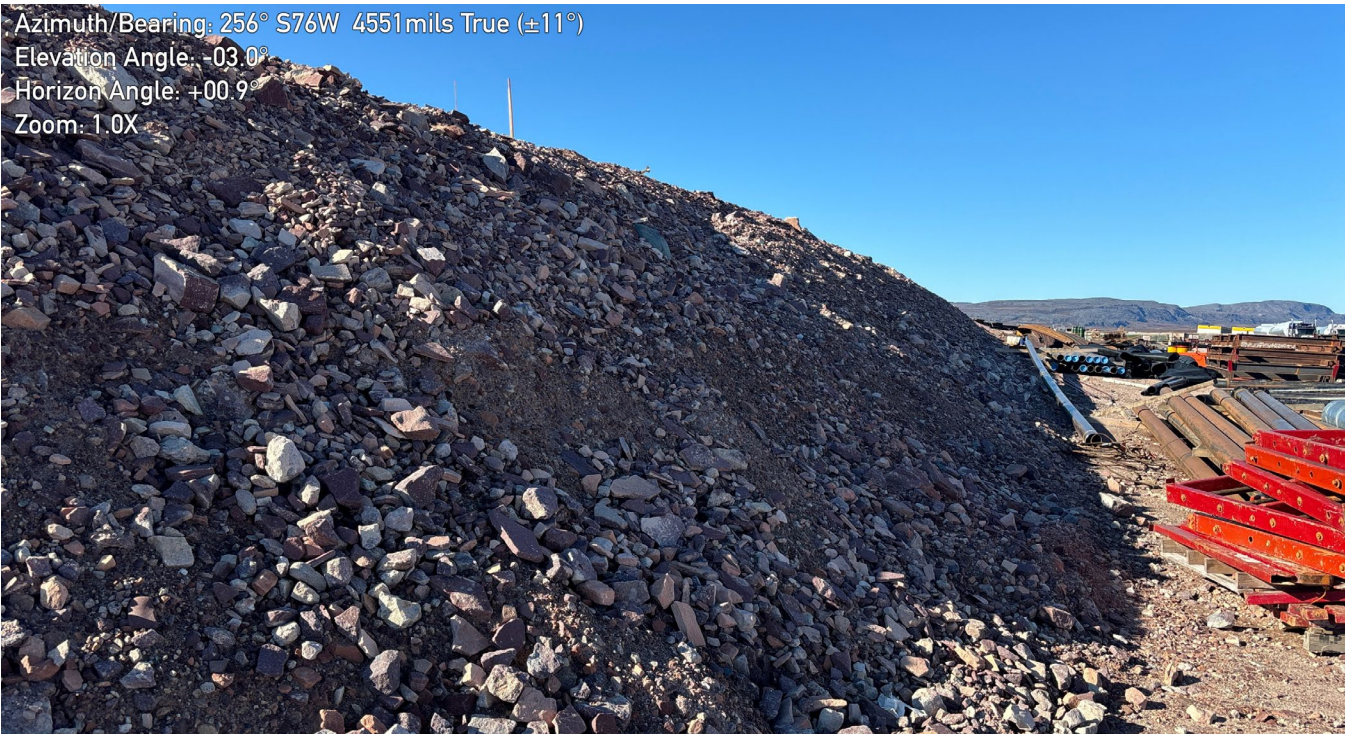
M-46: Tank farm laydown area – Note slopes oversteepened
