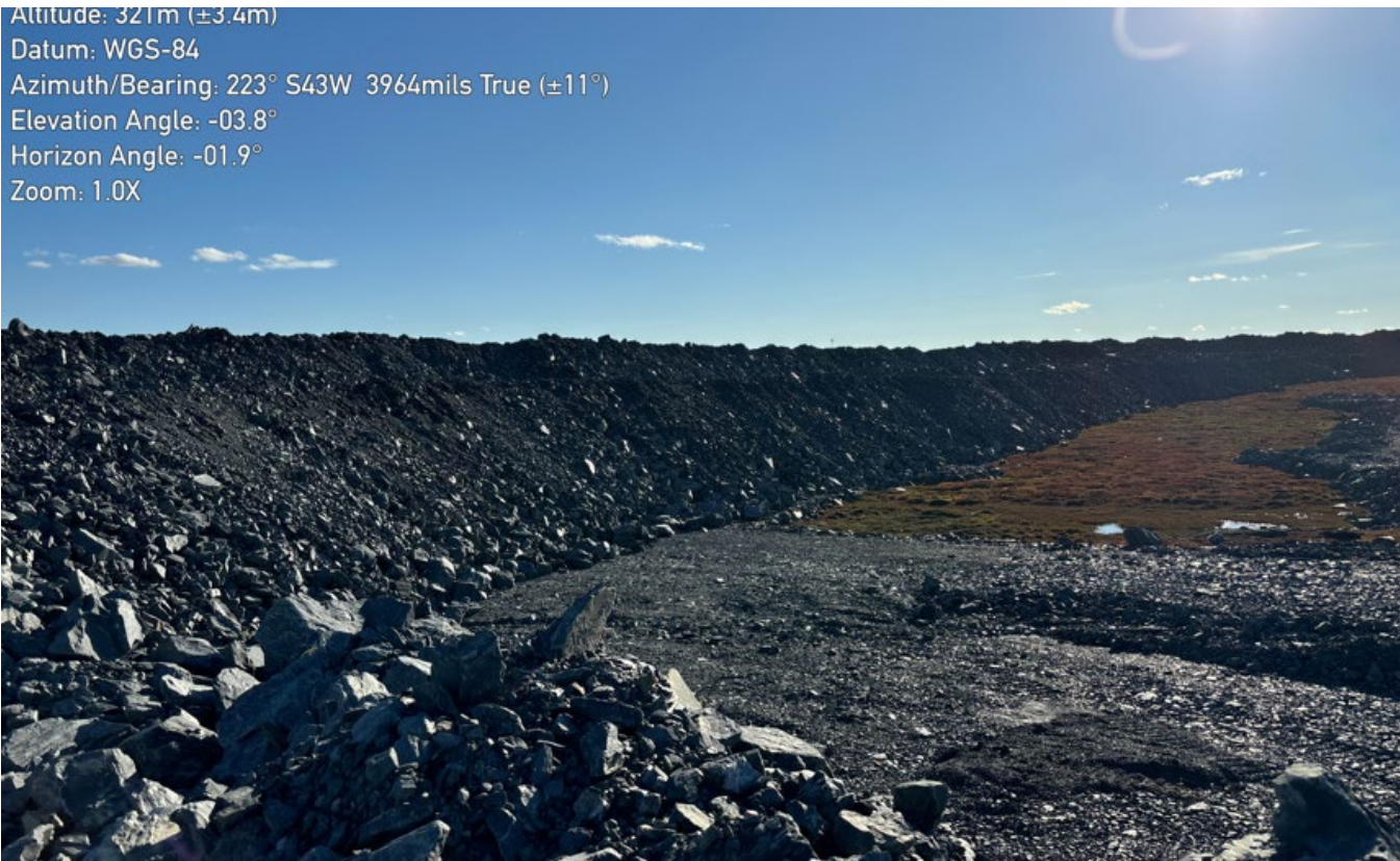
G-104: Northern face of WRSA, facing SW – Note oversteepened slopes
