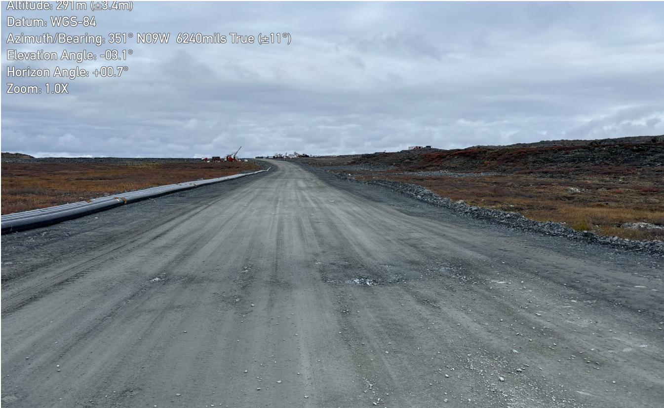
G-236: Haul Road Looking North – Note Road is underbuilt
