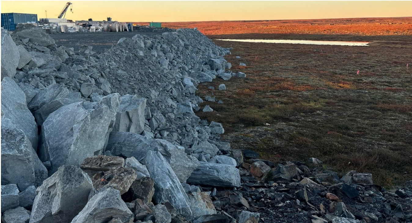
G-180: South facing slope – Note oversteepened, rockfall evident
