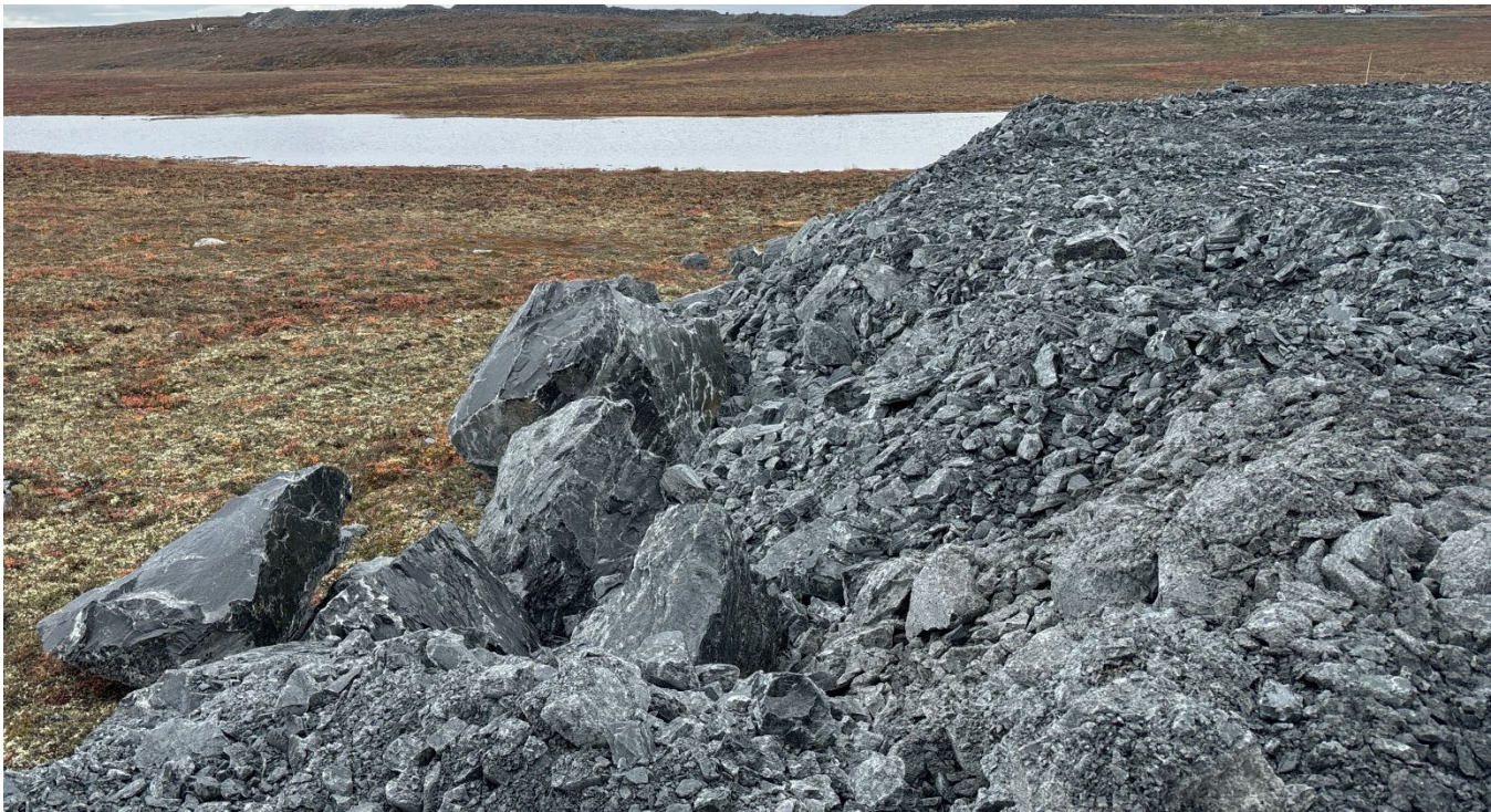
G-34: South end of NW apron, facing SW – Note irregular slope face
