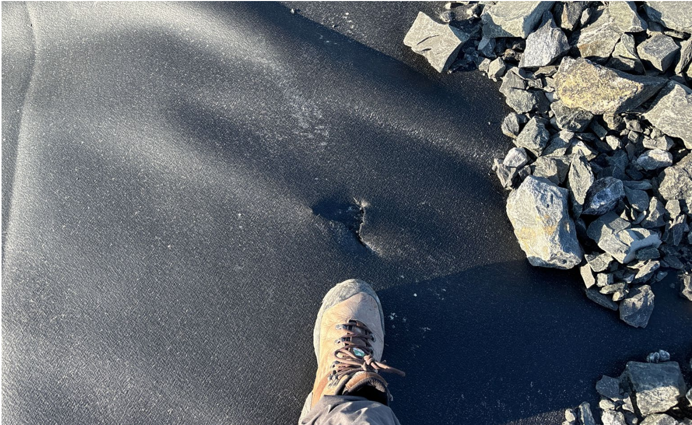
G-94: Liner damage
