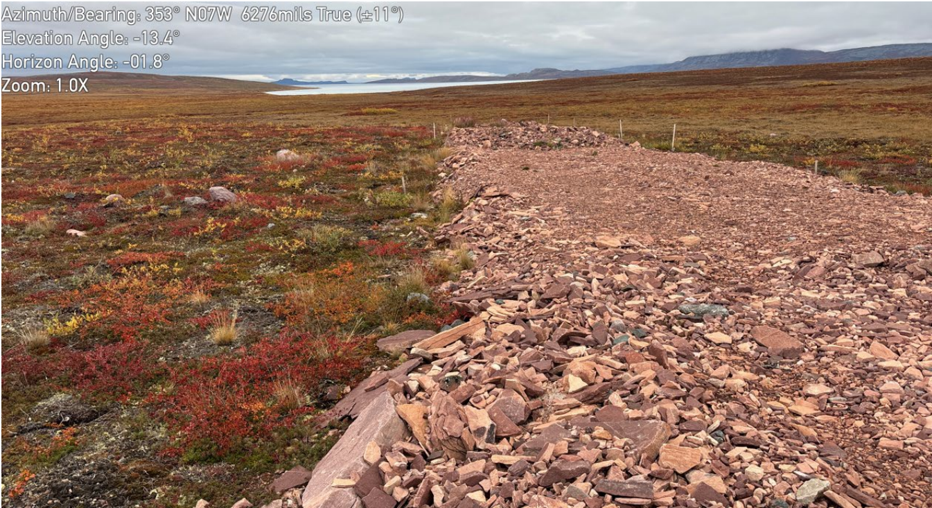
M-83: NW end of the former explosives storage access road – Note fill is too thin
