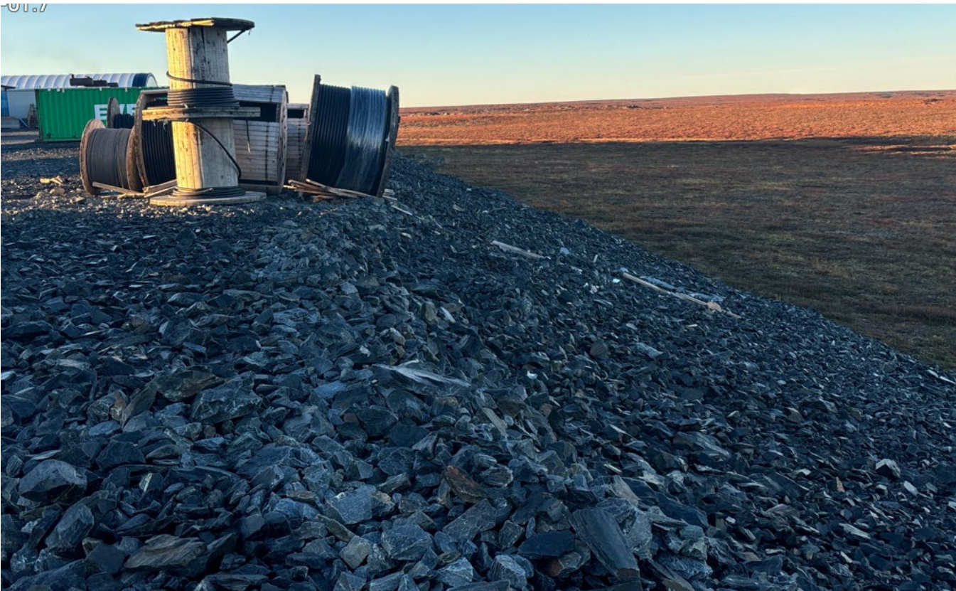
G-185: Western side of pad – Note coils to close to edge
