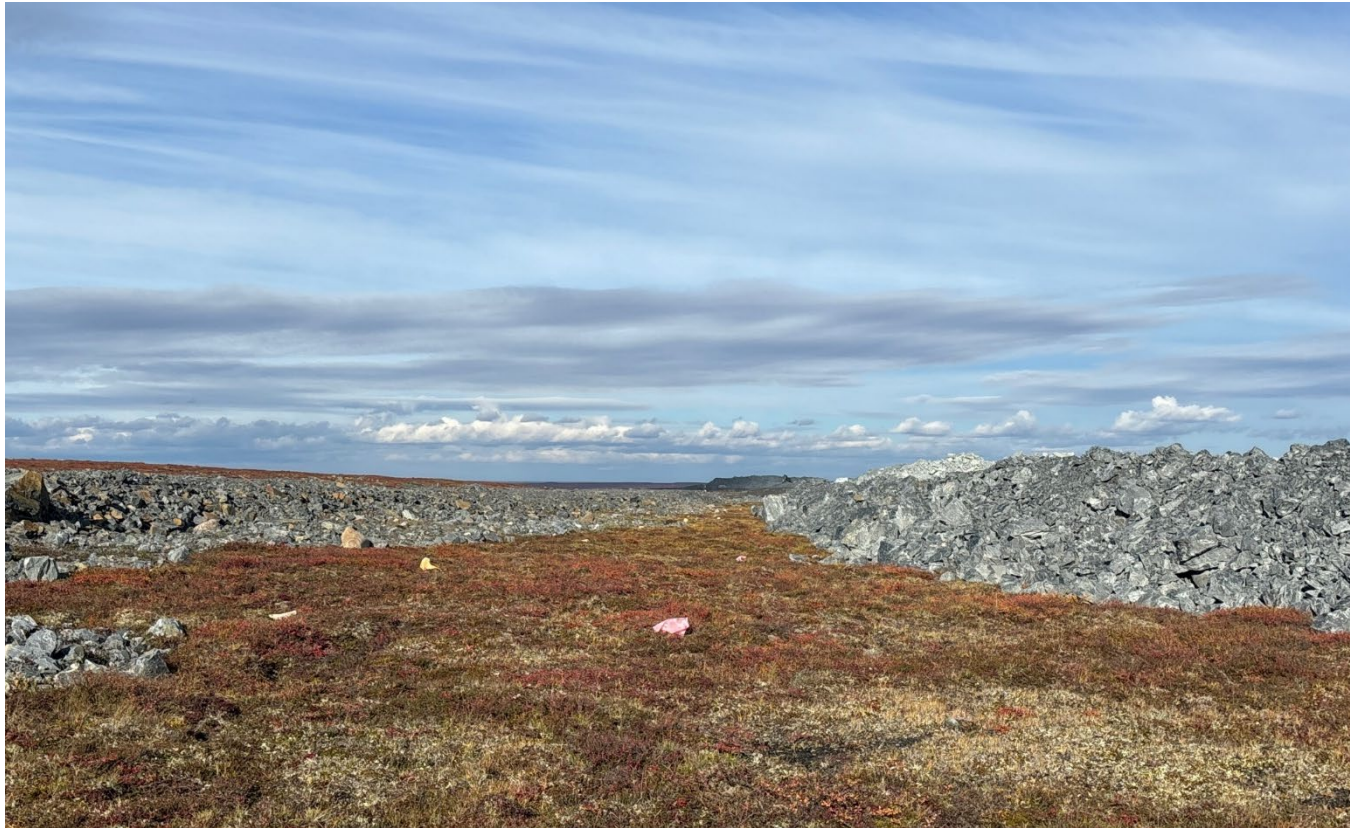
G-103: Diversion berm (left), WRSA (right), facing NE – Note WRSA too close to diversion berm
