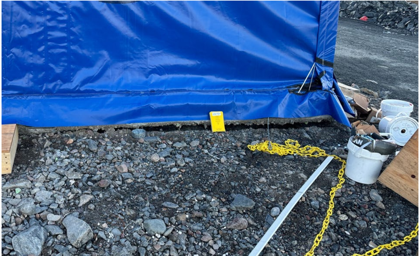
G-186: Tent foundation – Note 7cm gap between tent and foundation
