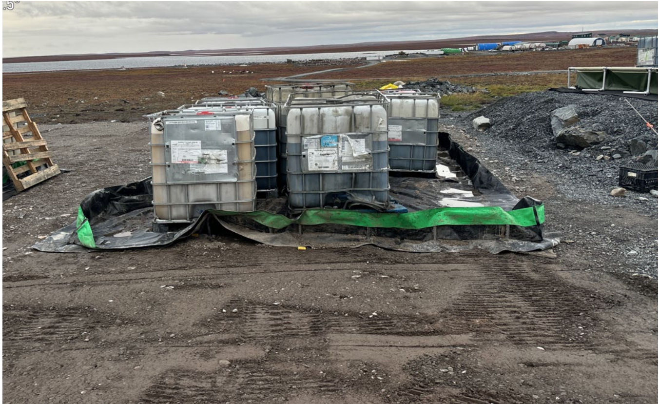
G-56: Containment berm is damaged
