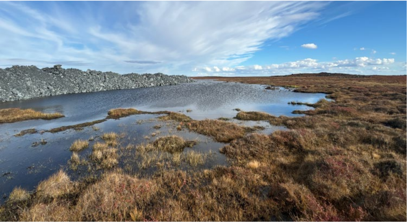
G-100: Southern end of WRSA, facing east – Note waste rock dumping in lake pond
