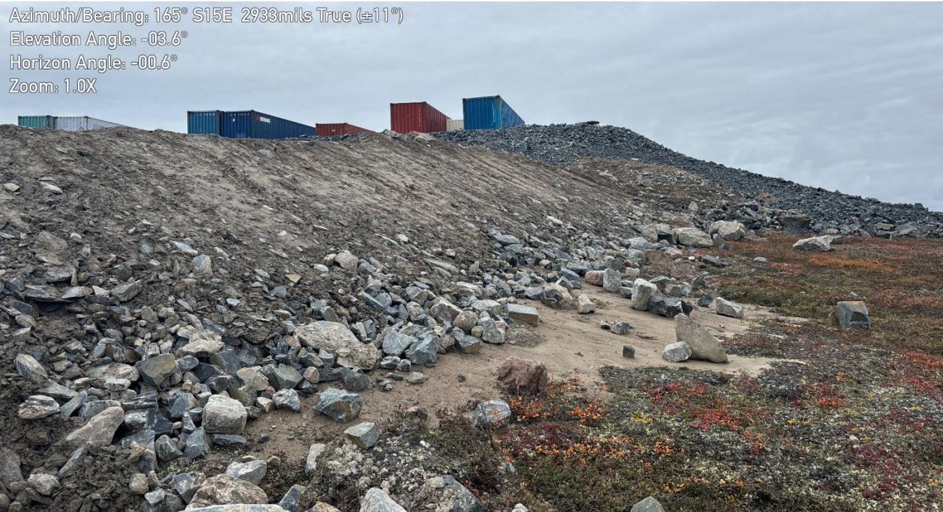
G-194: Camp Pad. Western slope – Note oversteepened slopes
