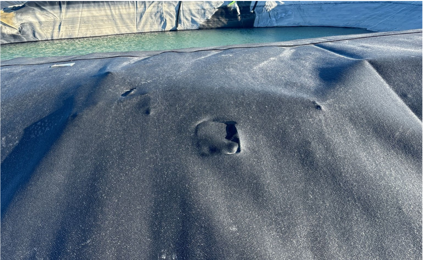
G-95: Liner damage
