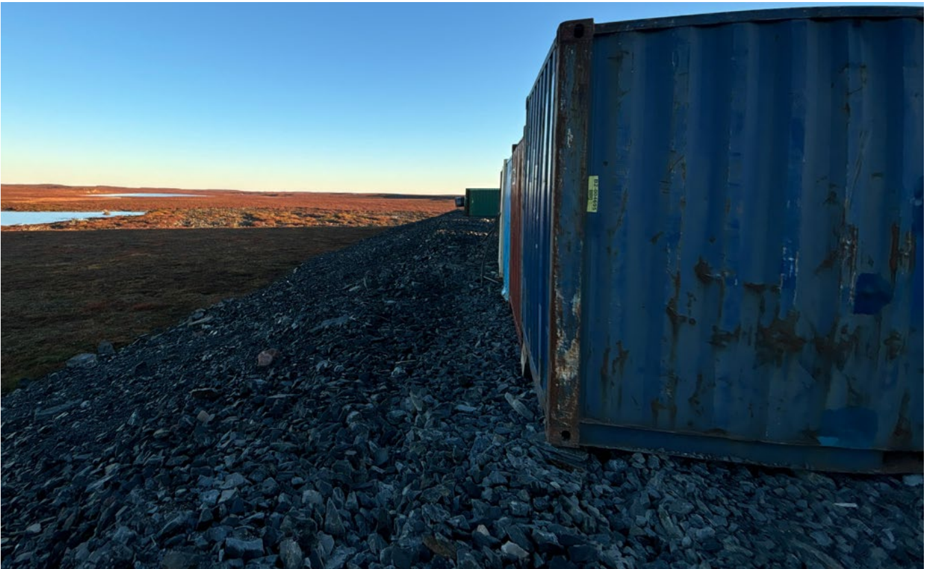
G-188: Western slope – Note seacans close to edge
