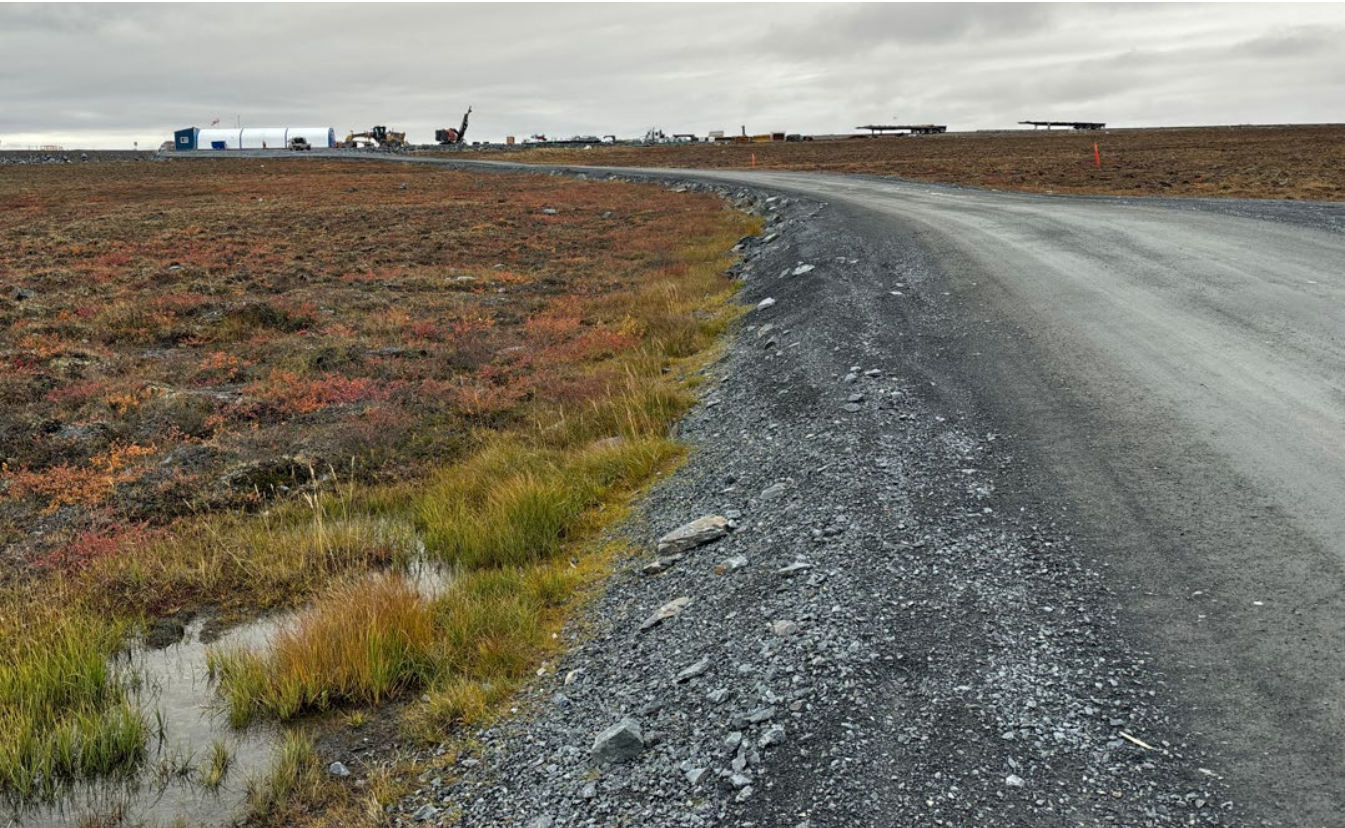
G-60: Ponding water at the toe of the access road, facing exploration camp
