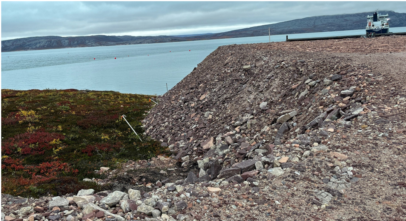
M-58: South pad facing east – Note steep slope
