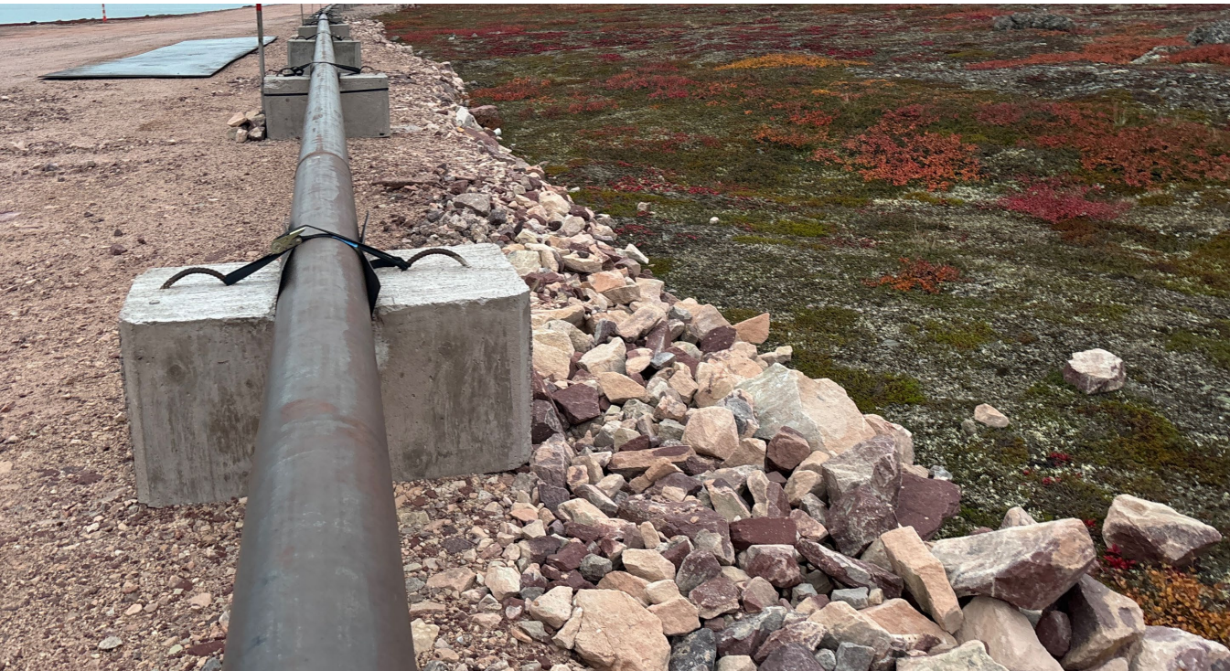
M-67: Note short distance between concrete block and edge and slope edge.
