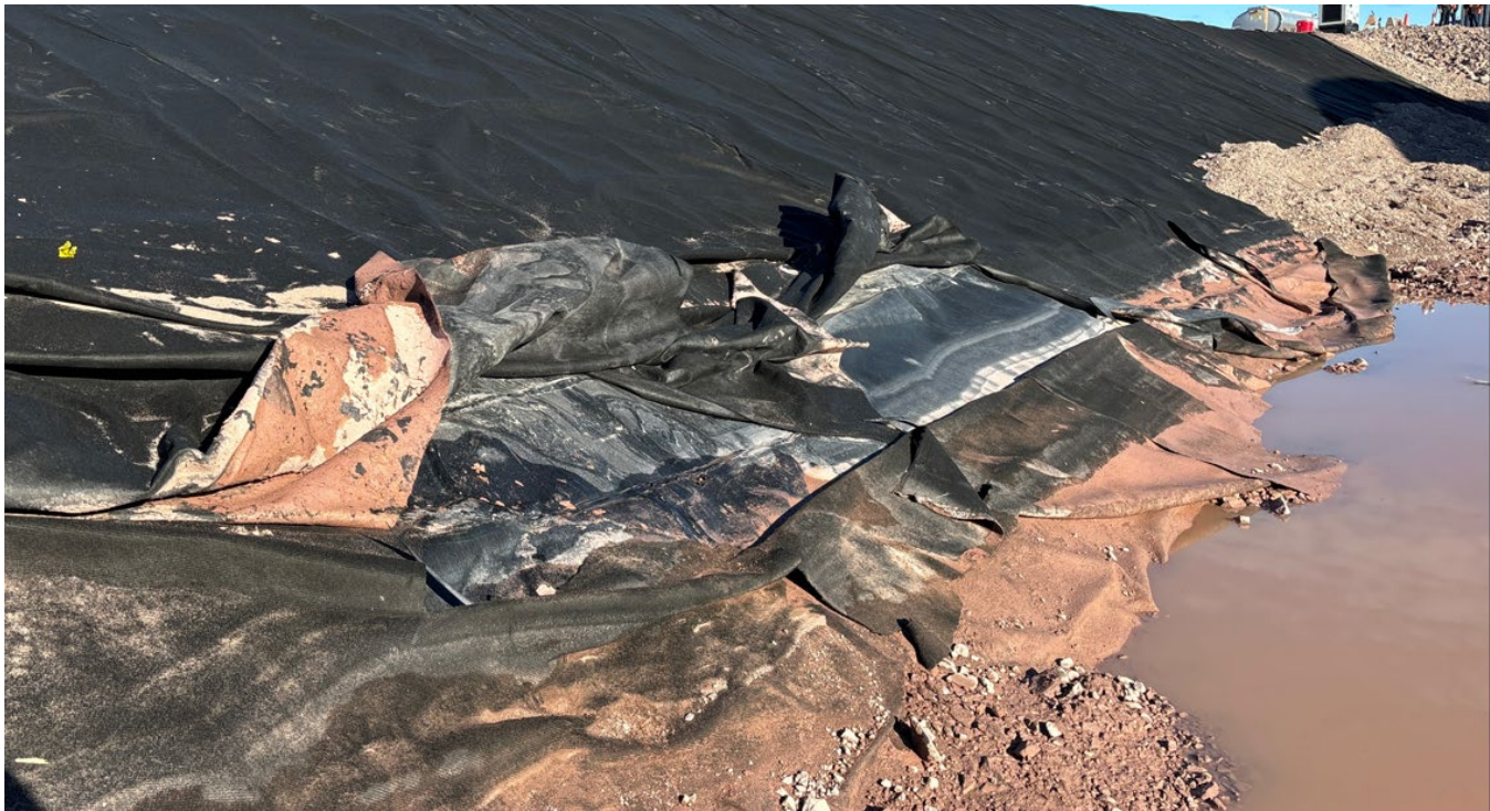
M-34: Liner damage
