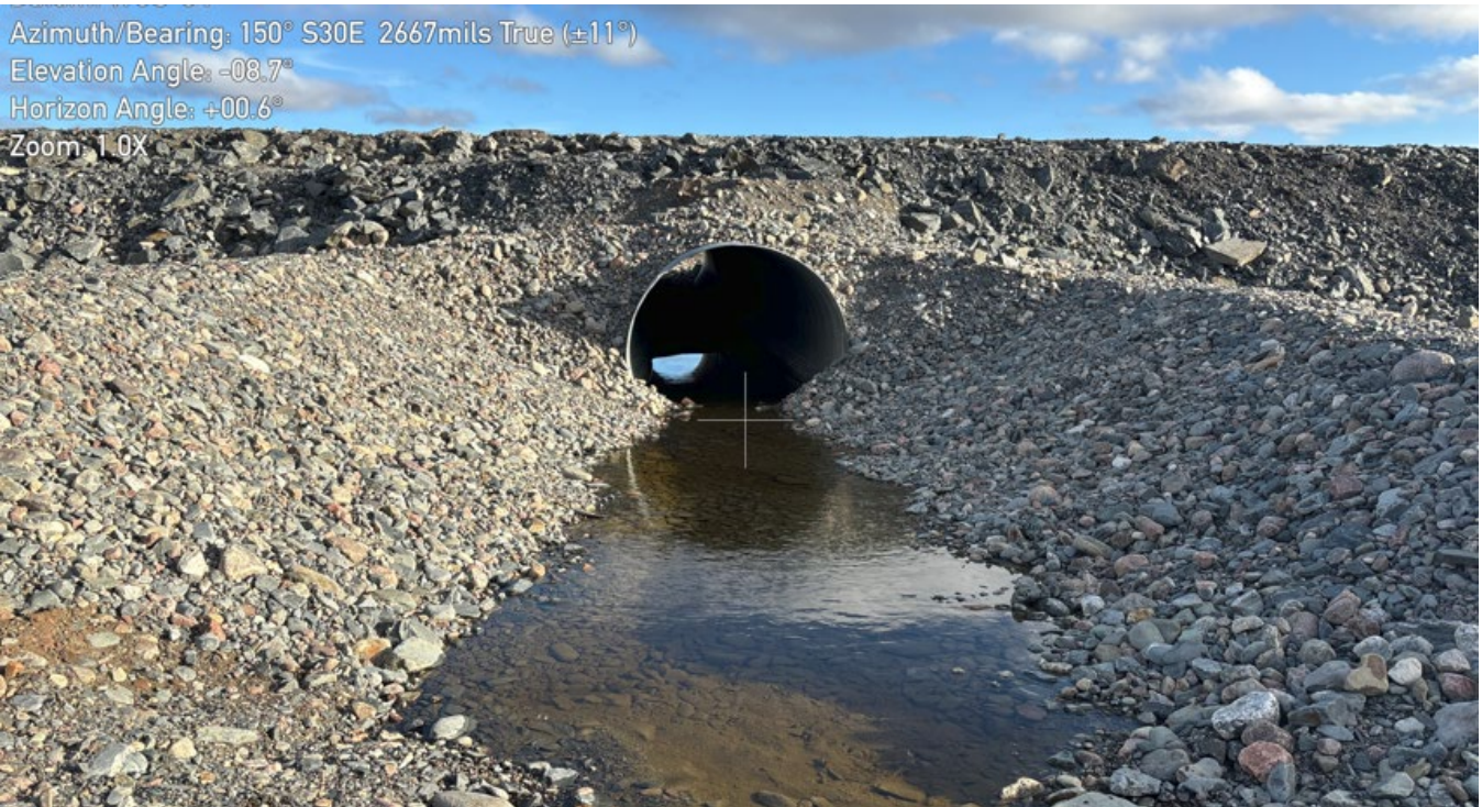
G-121: Gander Crossing Small Culvert, facing south– Note circular damage from installation. Ponding Water
