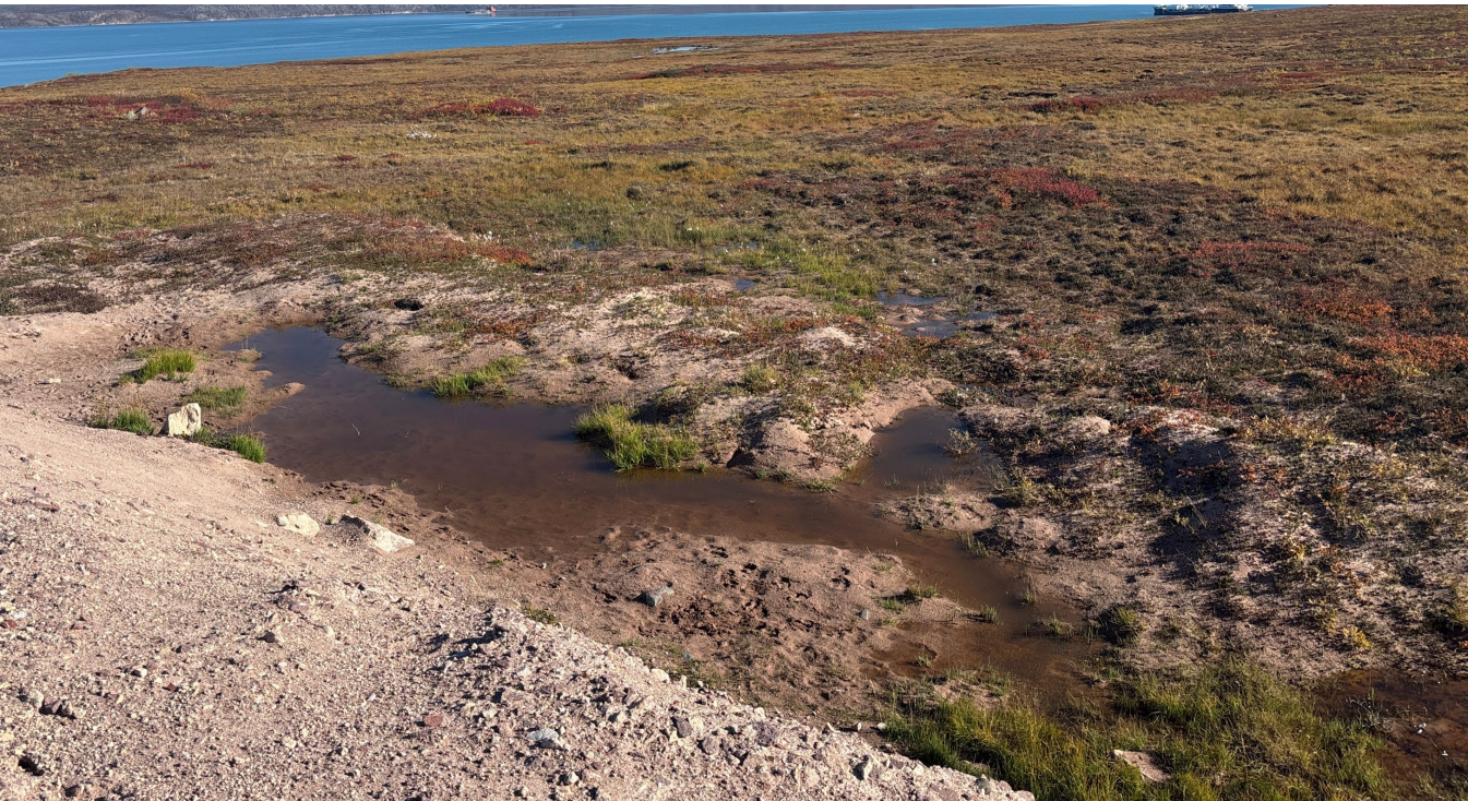
M-27: South end – Note ponding water at the toe of the embankment
