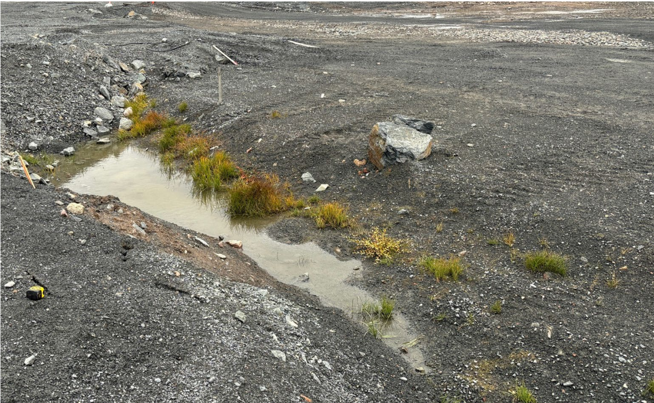
G-48: Beginning of apron, facing NW – Note ponding water
