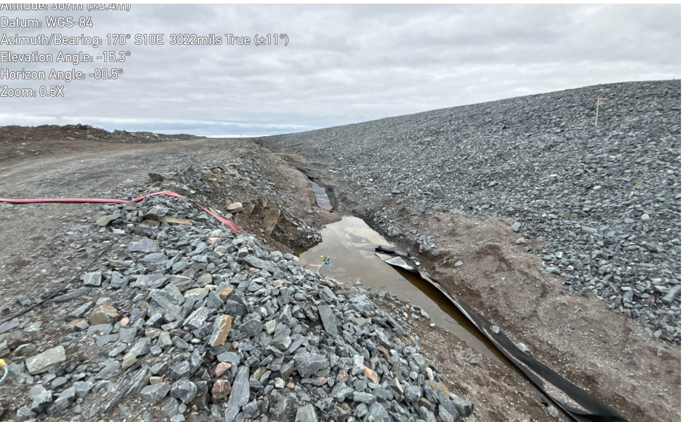
G-228: ponding water over liner at toe (between Sta 0+400 and Sta 0+450)
