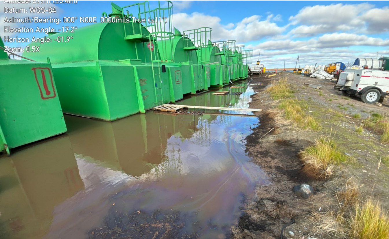
G-10: Fuel tank containment. Ponding Water
