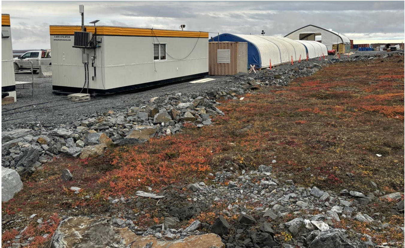
G-169: Typical pad thickness
