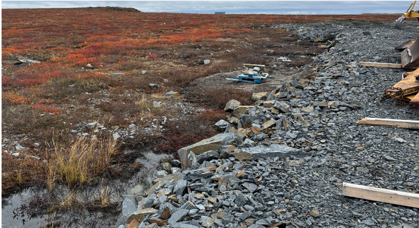
G-257: Edge of camp pad – Note ponding water
