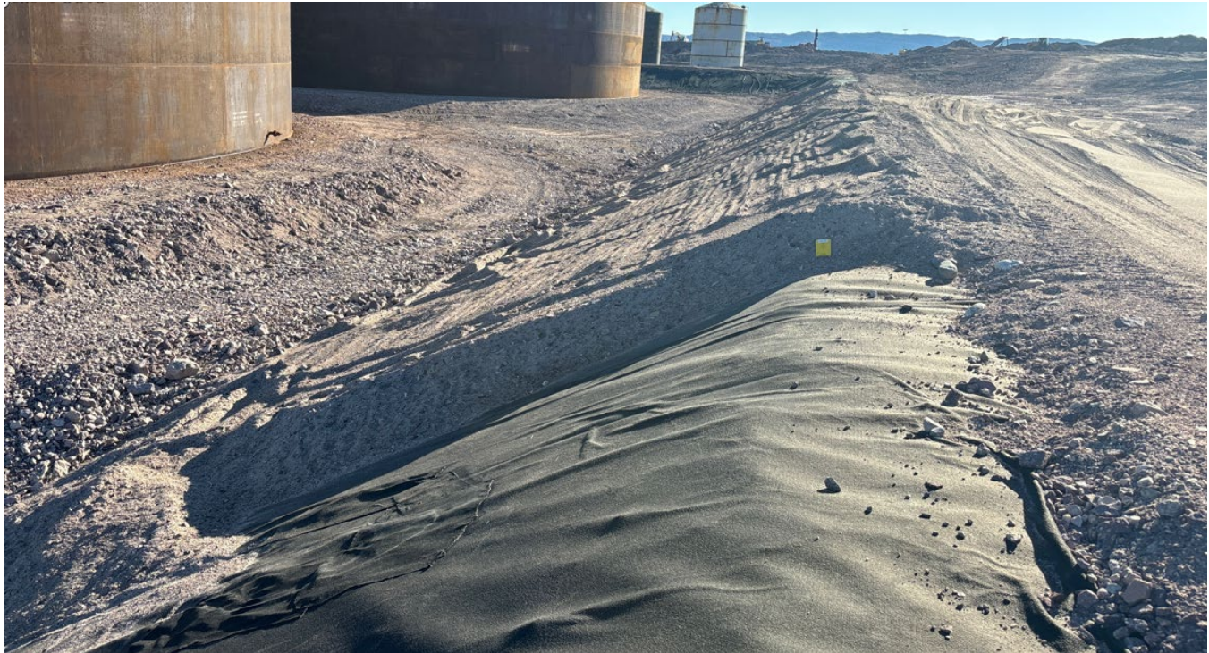
M-28: Liner fill is too thin, to allow equipment on the berm min 0.6 m of fill is required
