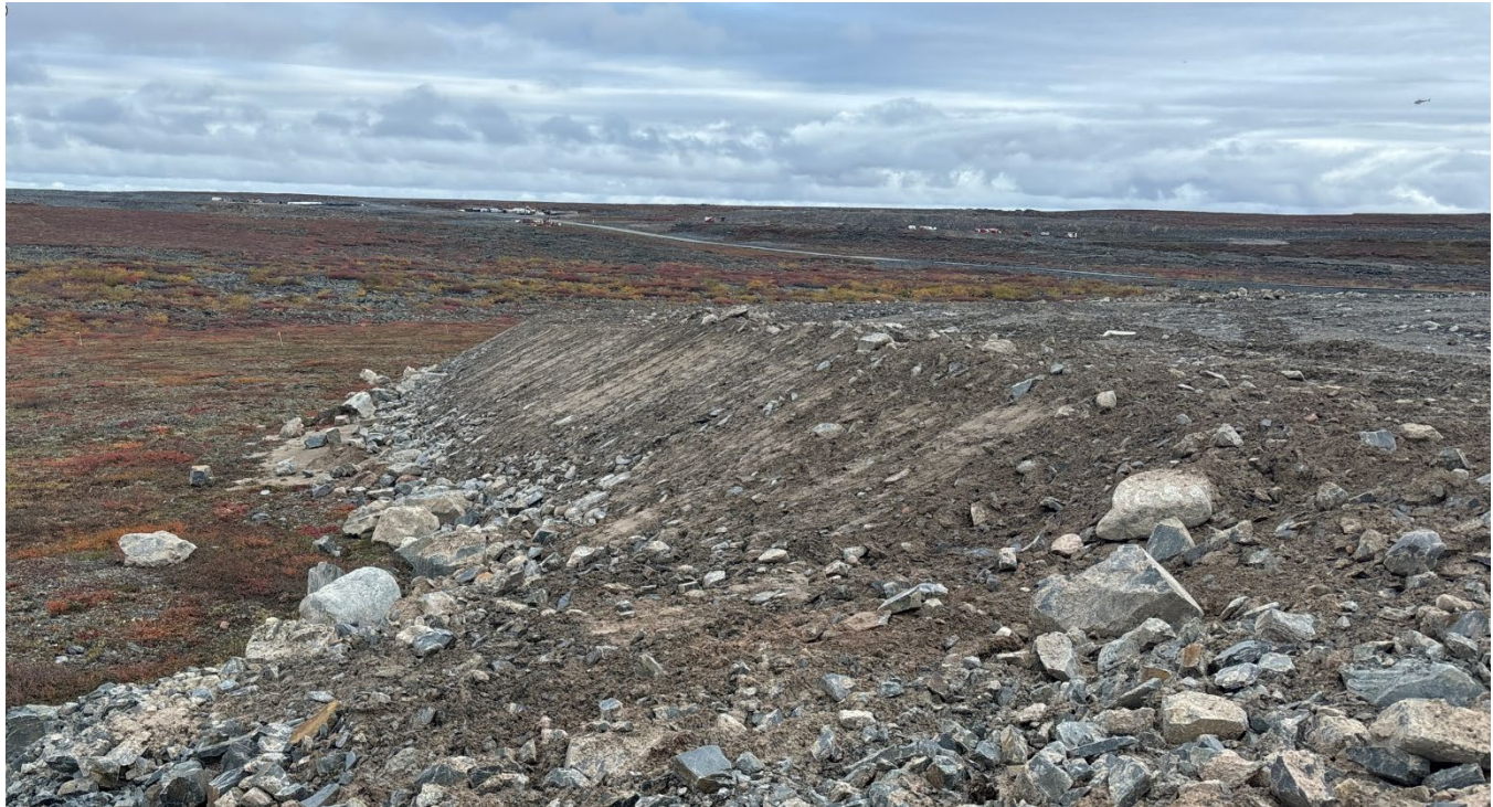
G-193: Western end of extension – Note slopes are prone to significant settlement. Looking north
