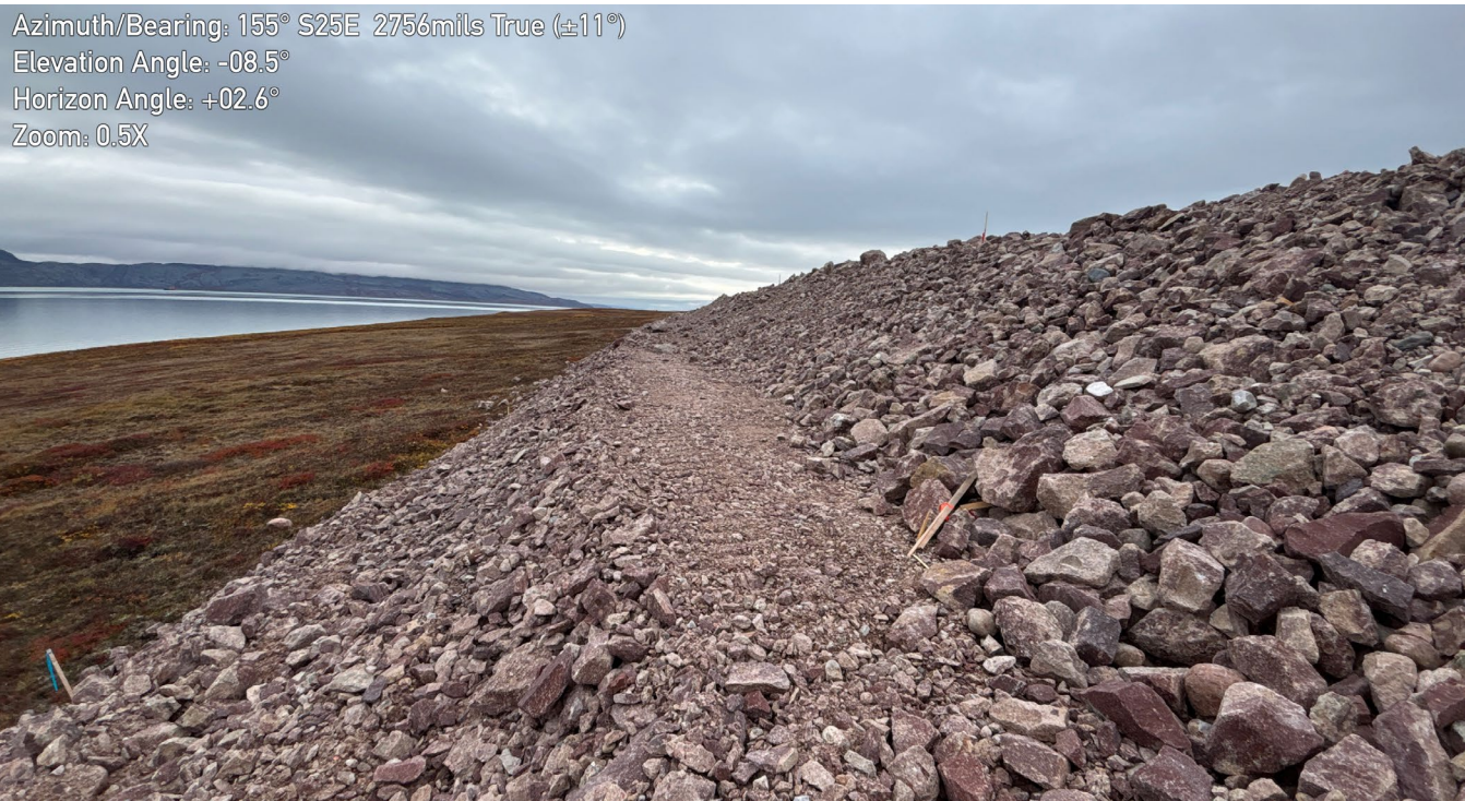
M-3: NE slope bench – Note fill material is placed in lifts
