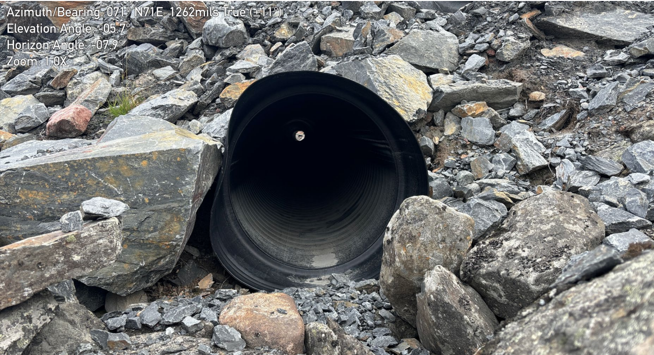
G-230: Toe of Crossing looking East – Note location of culverts do not match design location. Sizing insufficient for storm event (additional Culverts required)
