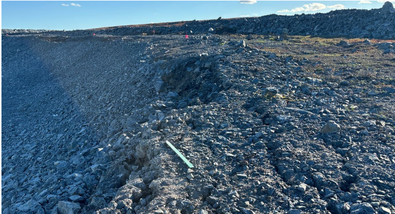
G-85: Crest of western wall, facing south – Note tension cracks
