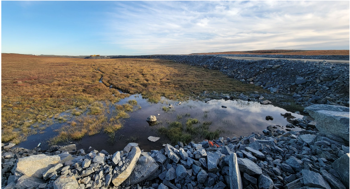
G-141: Echo haul road. Eastern side, facing south – Note ponding water
