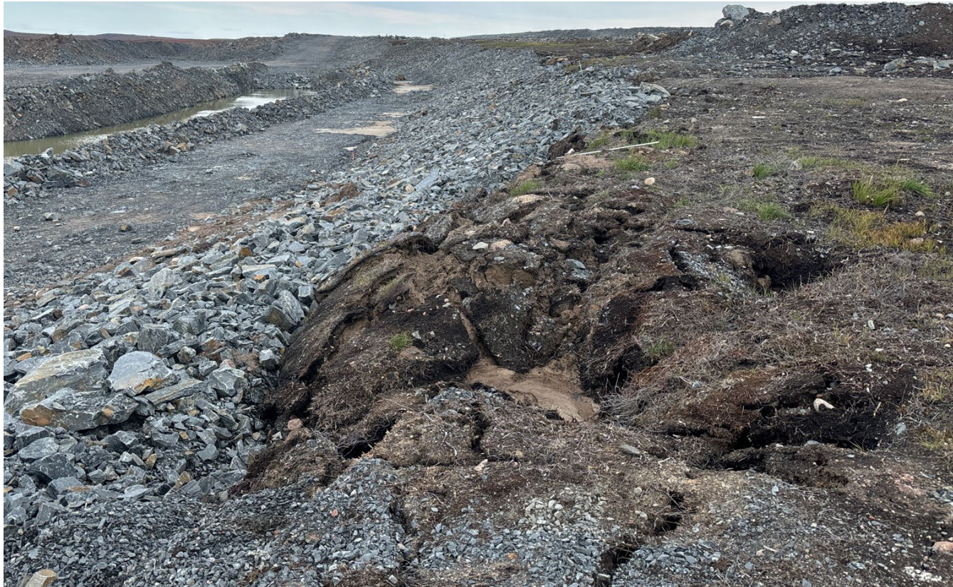
G-210: South end of slope, facing NW – Note thermal erosion due to lack of rockfill layer
