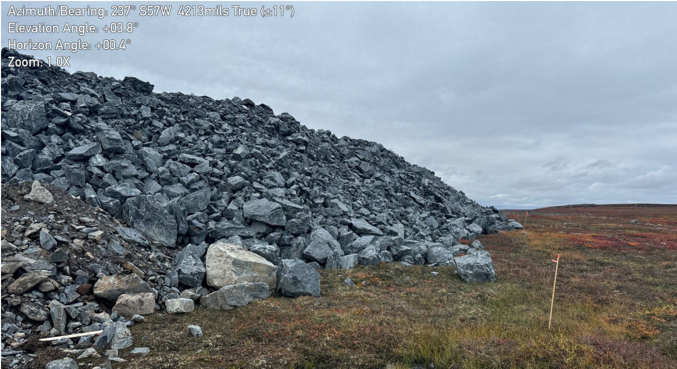
G-197: Pad extension looking west – Note oversteepened slopes
