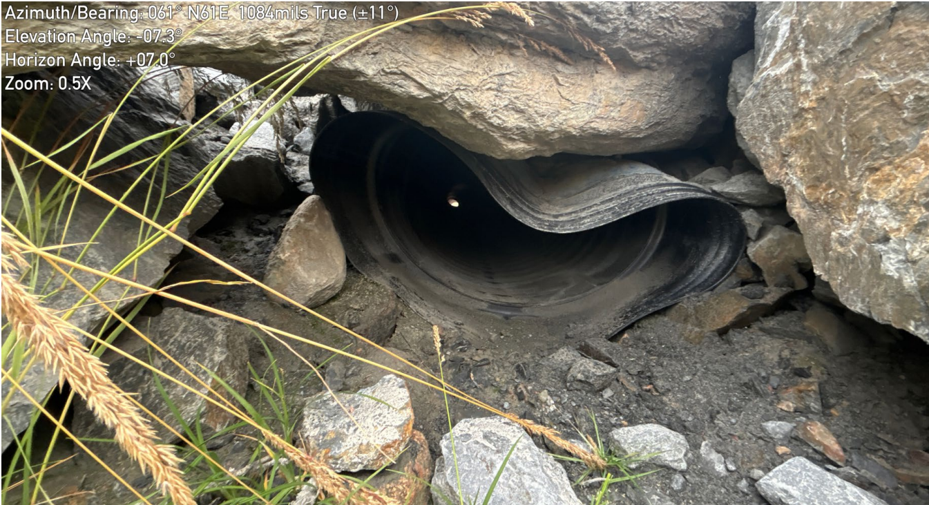
G-229: Goose Neck Crossing Culvert – Note No Fine Material around Culvert
