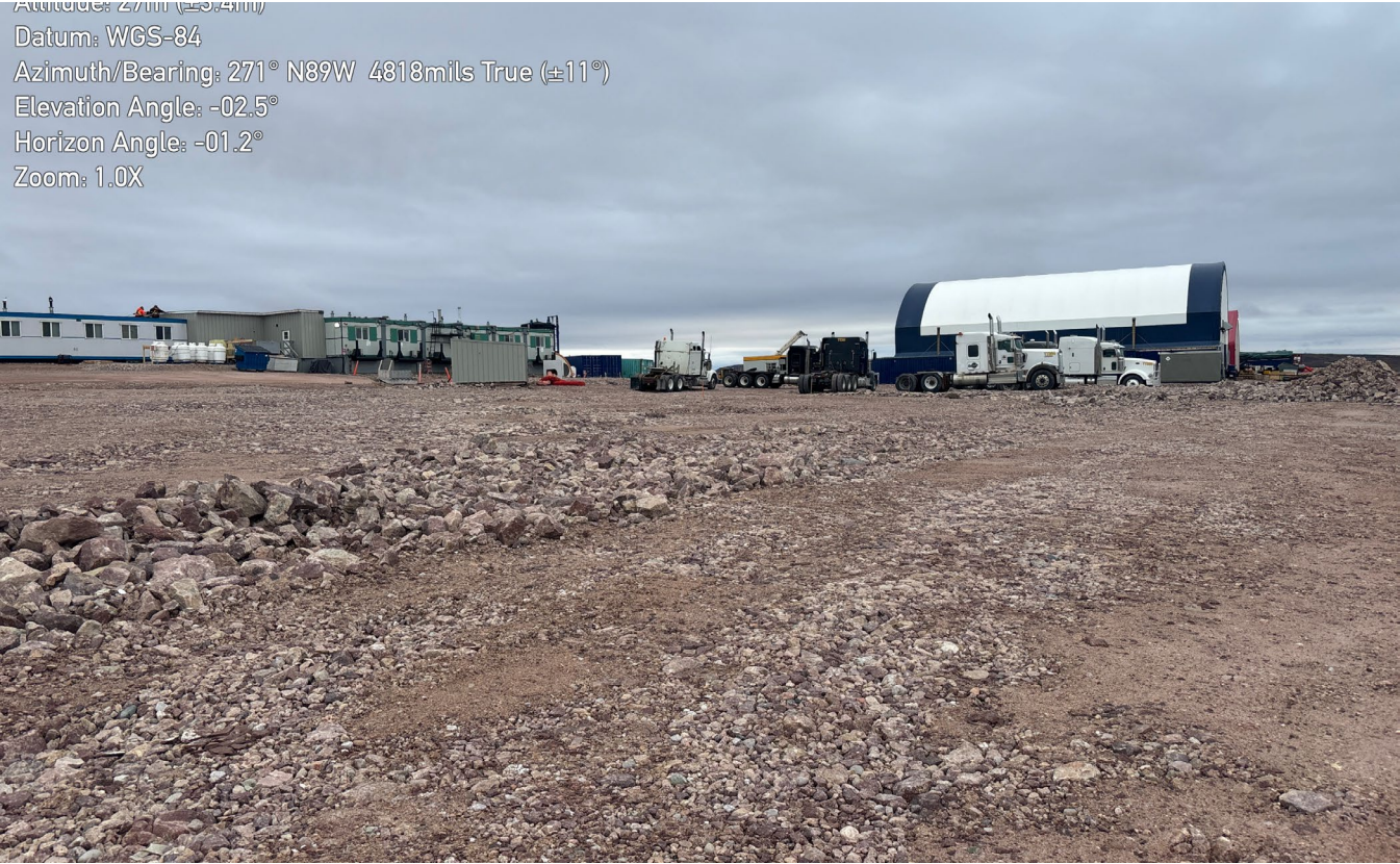
M-10: West side of extension - Note that fill material lacks proper compaction
