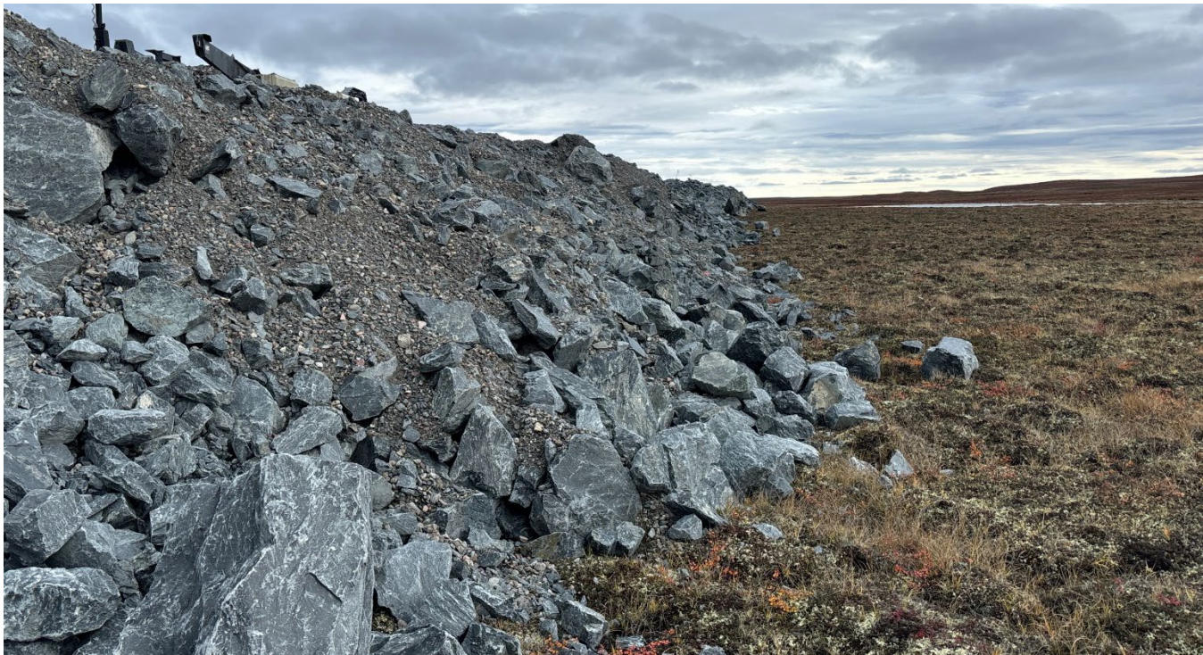
G-33: NW apron northern slope, facing SE – Note oversteepend slope
