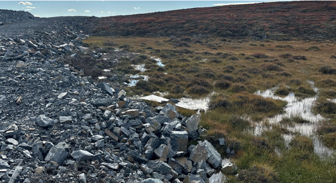
G-72: Diversion, facing west – Note thickness less than 1m
