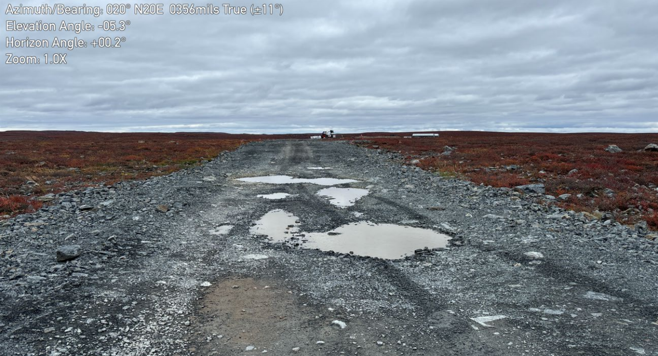
G-253: Access road, facing NE – Note road is underbuilt, and foundation is degraded
