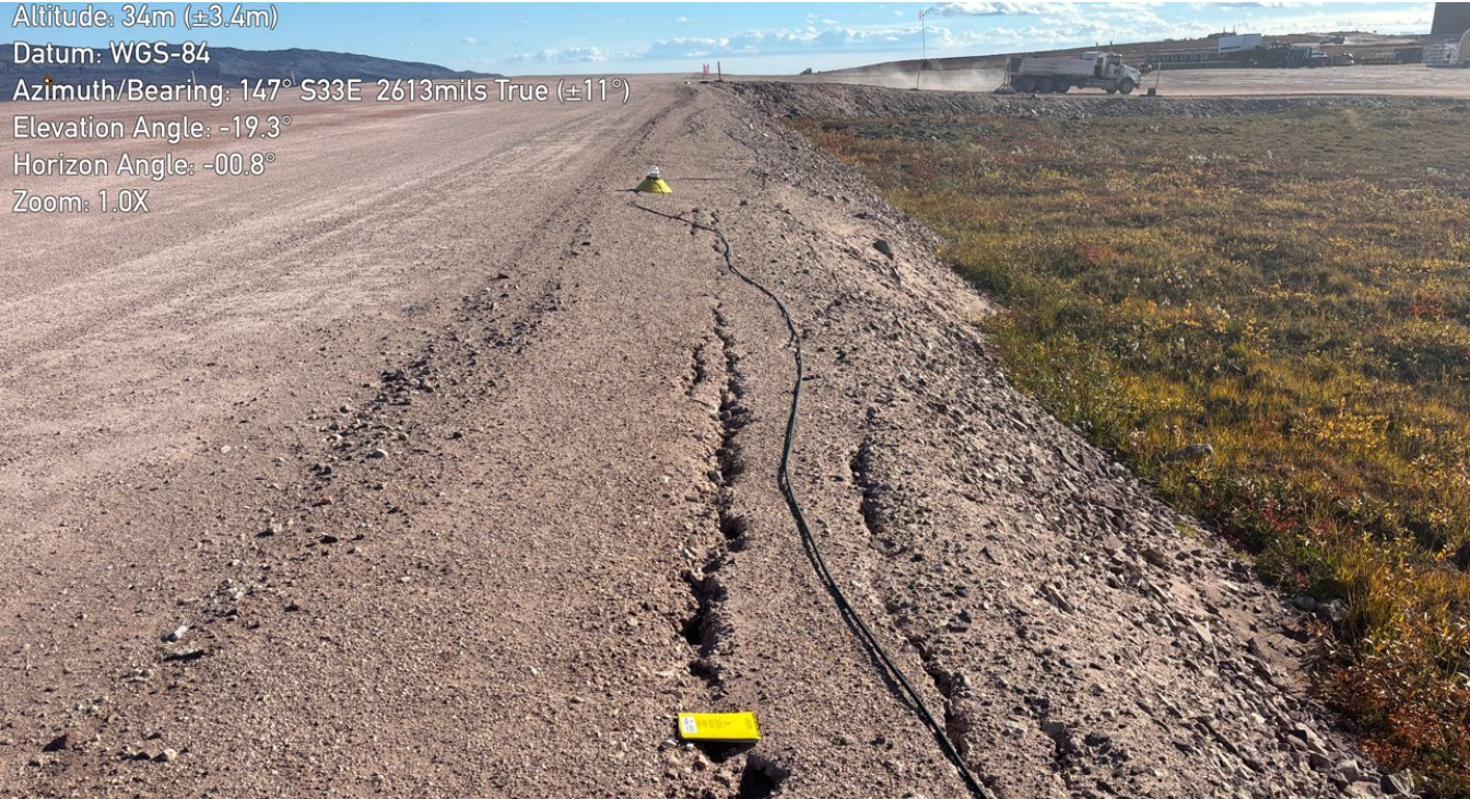
M-13: Airstrip, western side, facing SW – Cracks at the embankment crest – offset the lightening system off the crest
