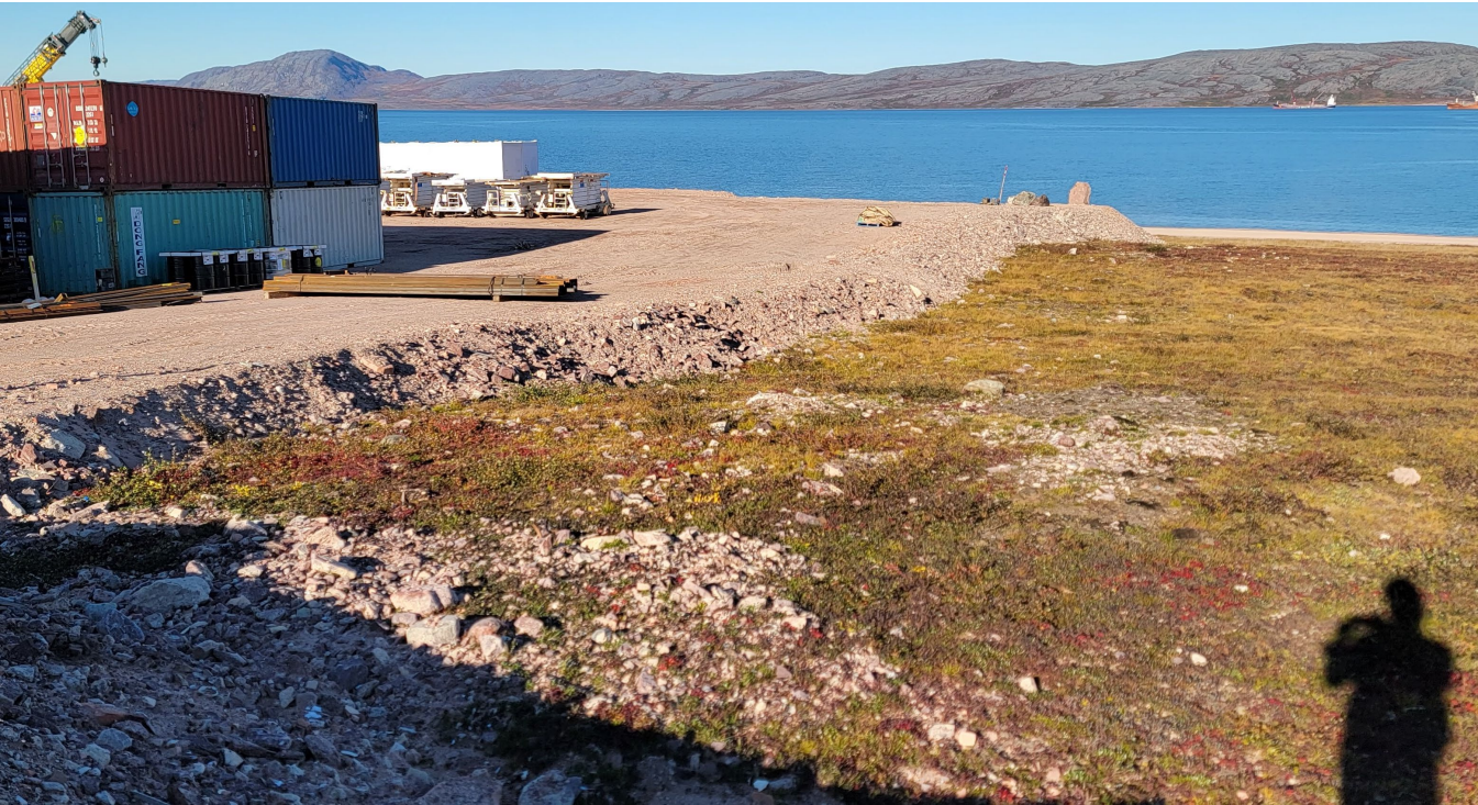
M-6: Typical Laydown pad thickness, facing NE
