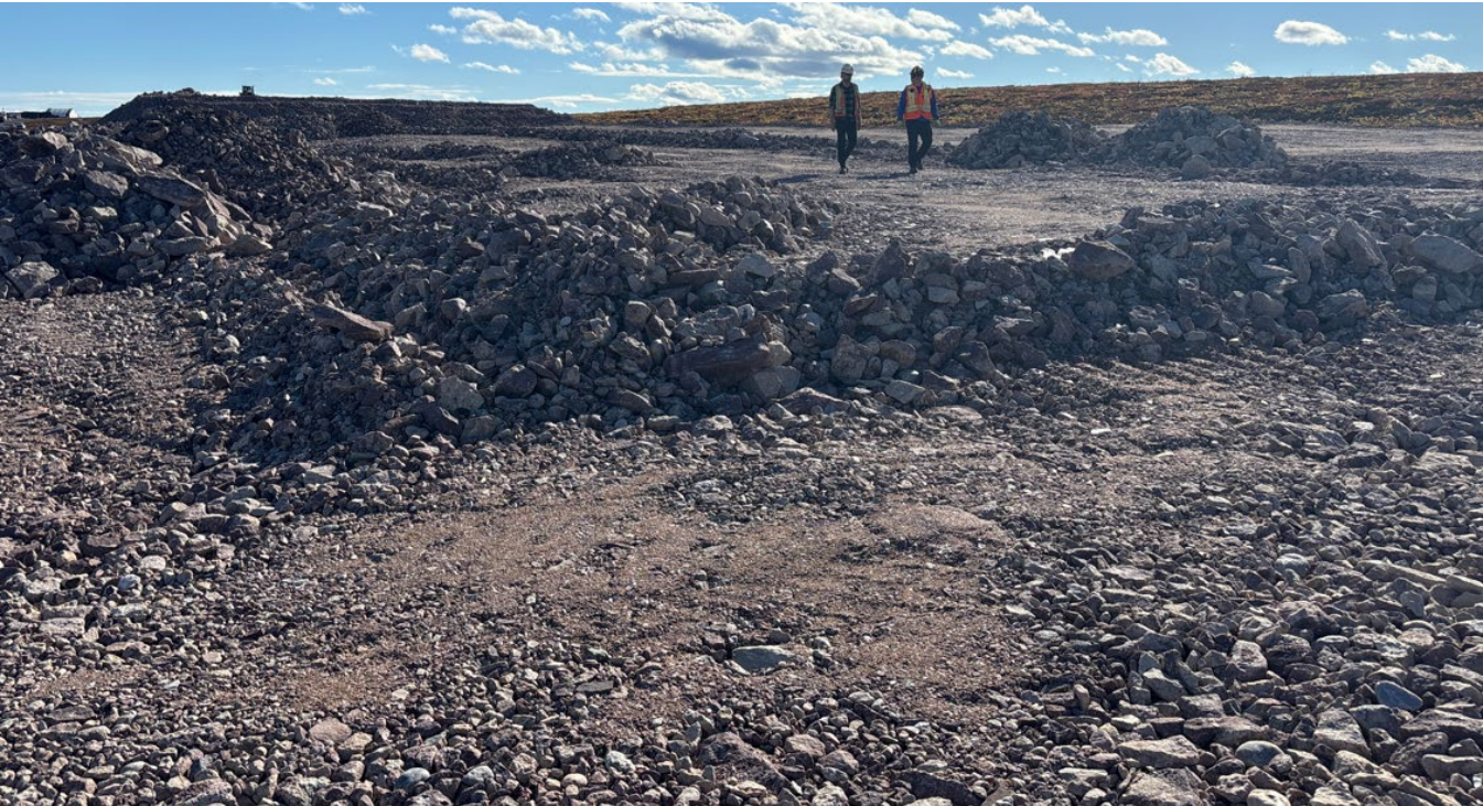
M-17: Airstrip extension, northern end – fill material is placed in 0.8m lifts
