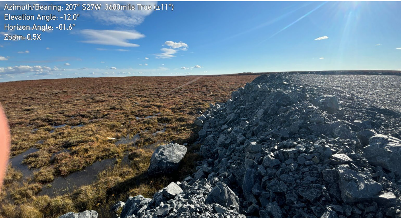
G-102: General view, southern slope, facing SW – Note lack of safety berm and irregular slope face
