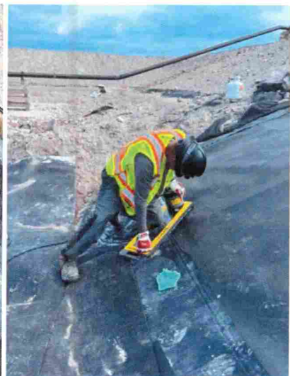
Final vac box testing at ramp area
