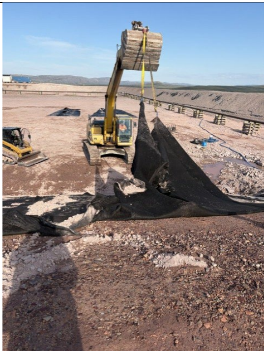
Photo 3: Removing Damaged Liner
