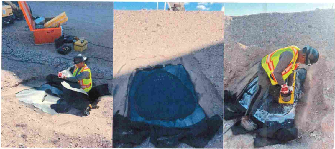
Removing damaged liner and geotextile
