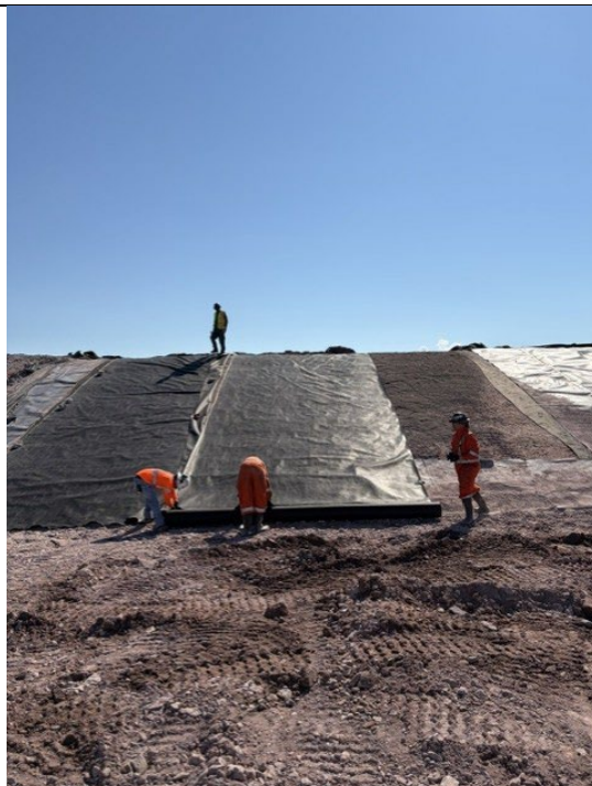
Photo 4 Replacing Geotextile
