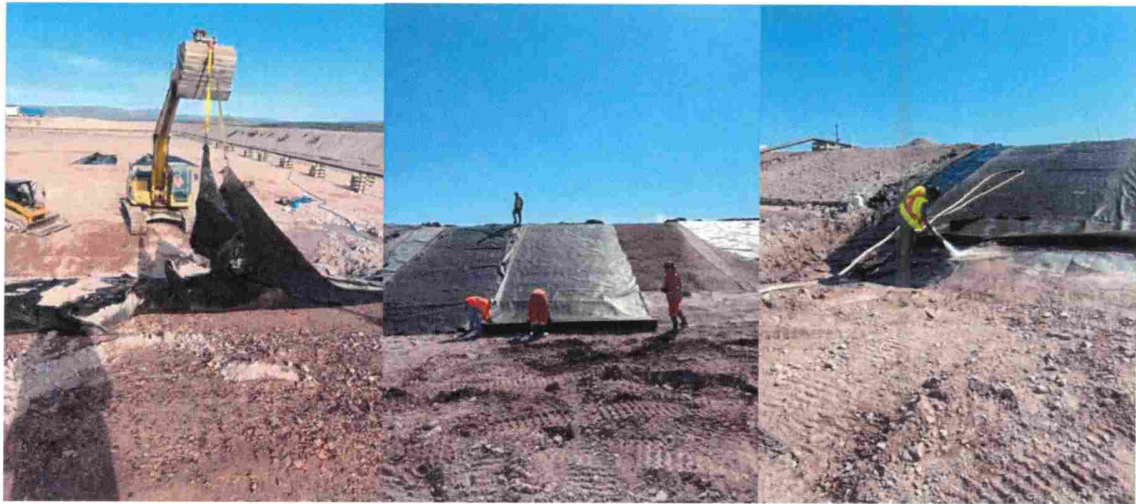
Replacing the geotextile
