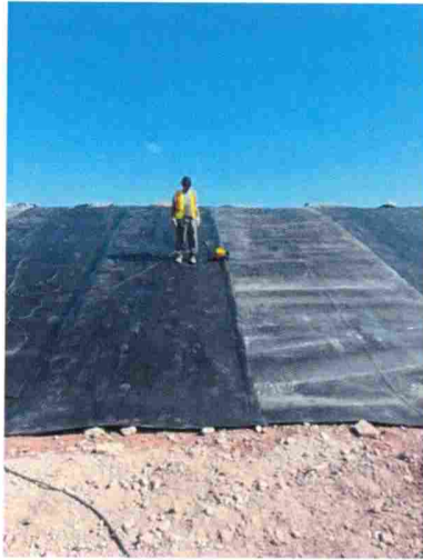
Wedge welding new liner
