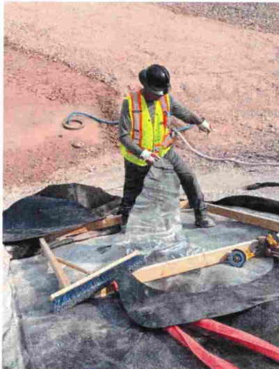
Damage by NW sump
