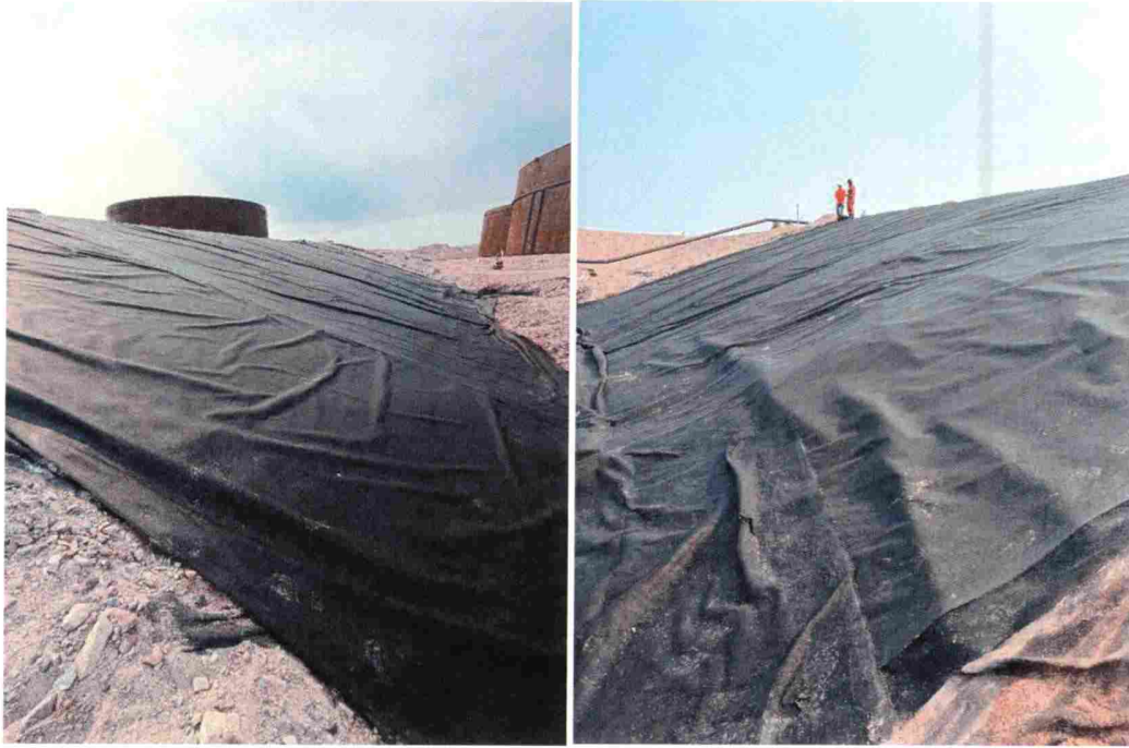
Geotextile cover over HDPE liner overlapping onto exposed floor geotextile.
