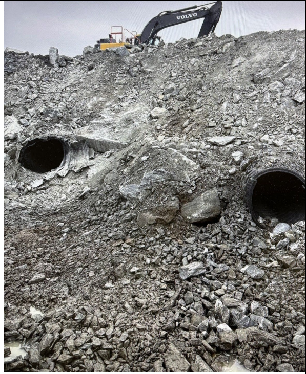
Photo 2 (August 07, 2026) – Echo Haul Road Inspection SE
