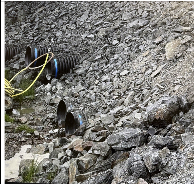
Photo 3 (August 07, 2026) – Echo Haul Road Inspection SW
