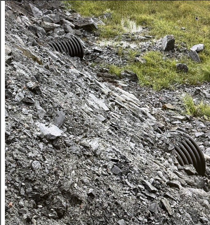
Photo 1 (August 07, 2026) – Echo Haul Road Inspection – N
