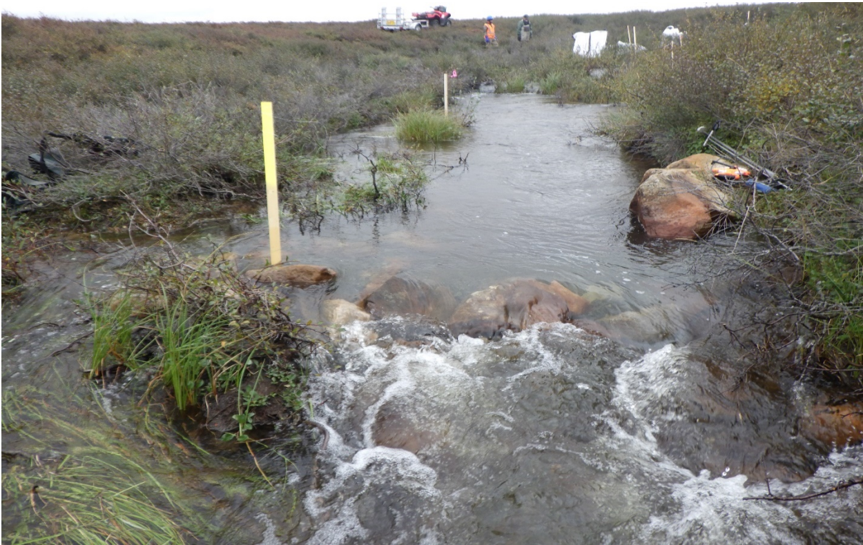
Figure 5. Constructing Instream Velocity Mitigation (Rock Weirs) in Rascal Stream West (September 2020).
