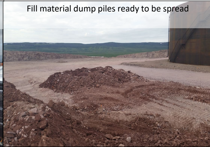
Containment floor being raised in lifts
