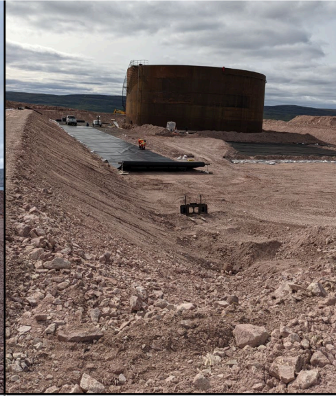
Top of NE Berm packed and keyed
