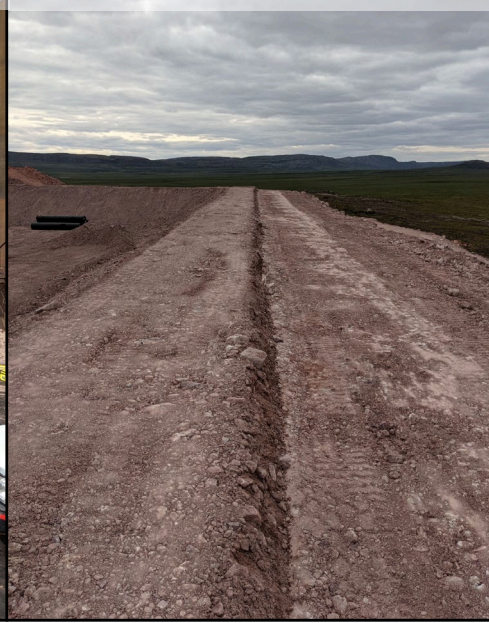
Top of NE Berm packed and keyed
