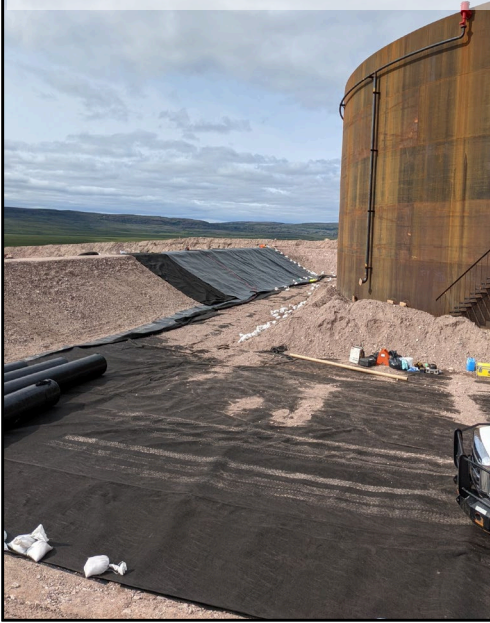
Geo and liner on SW berm
