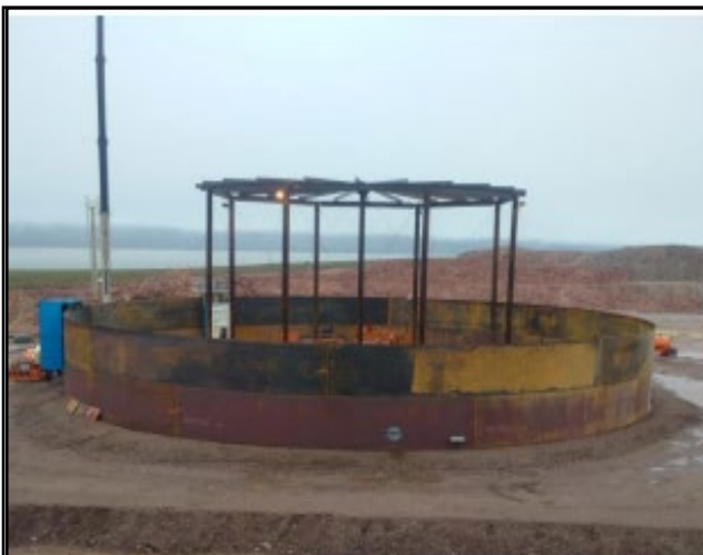
Elevation view : Tank Plates being installed
