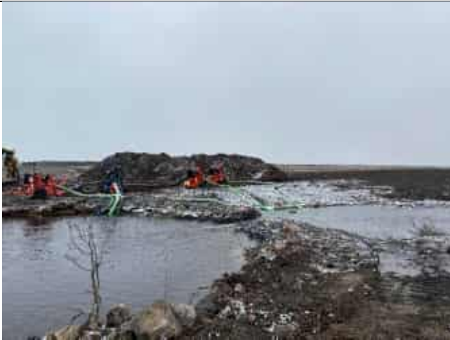
Photo 1: Dewatering pumps in upper pond and lower pond upstream of twin multiplate culvert excavation.
