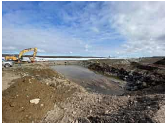
Photo 4: Twin multiplate culvert excavation at 9:53.
