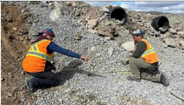
Photo 5: The excavated area extends 2.7 m from edge of the culvert on the west side
