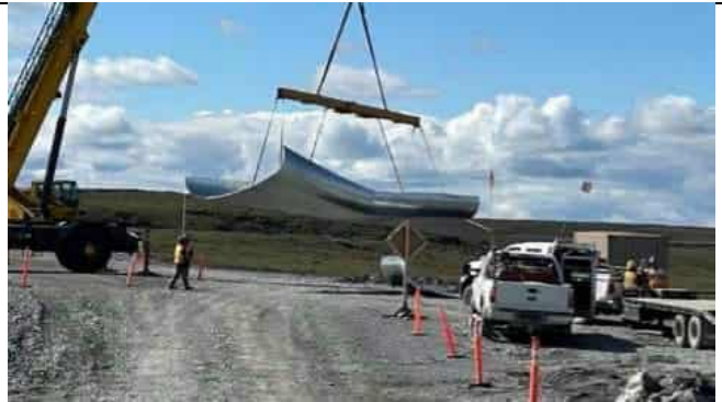
Photo 4: Culvert bottom plate of the downstream segment on the east side (right downstream) was deformed when being lifted
