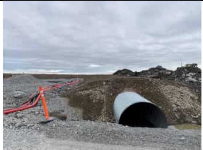
Photo 2: Secondary culvert raw esker backfill 0.6 m above culvert crest looking upstream at 14:38.
