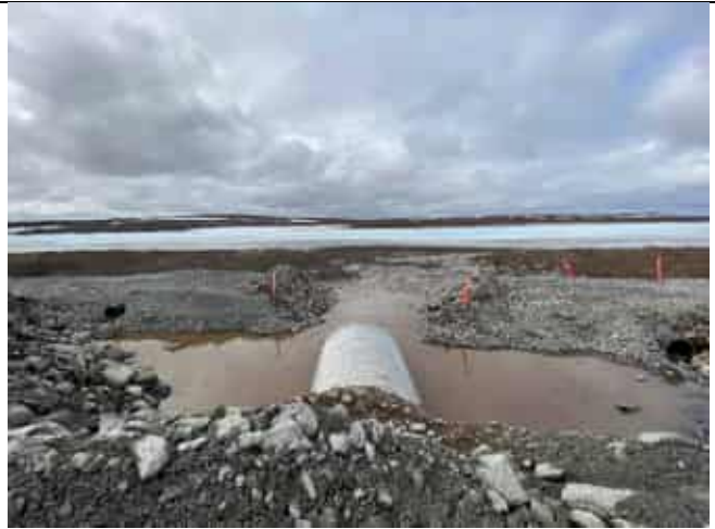
Photo 2: Secondary culvert discharging RSW over temporary riprap apron looking downstream at 14:11.
