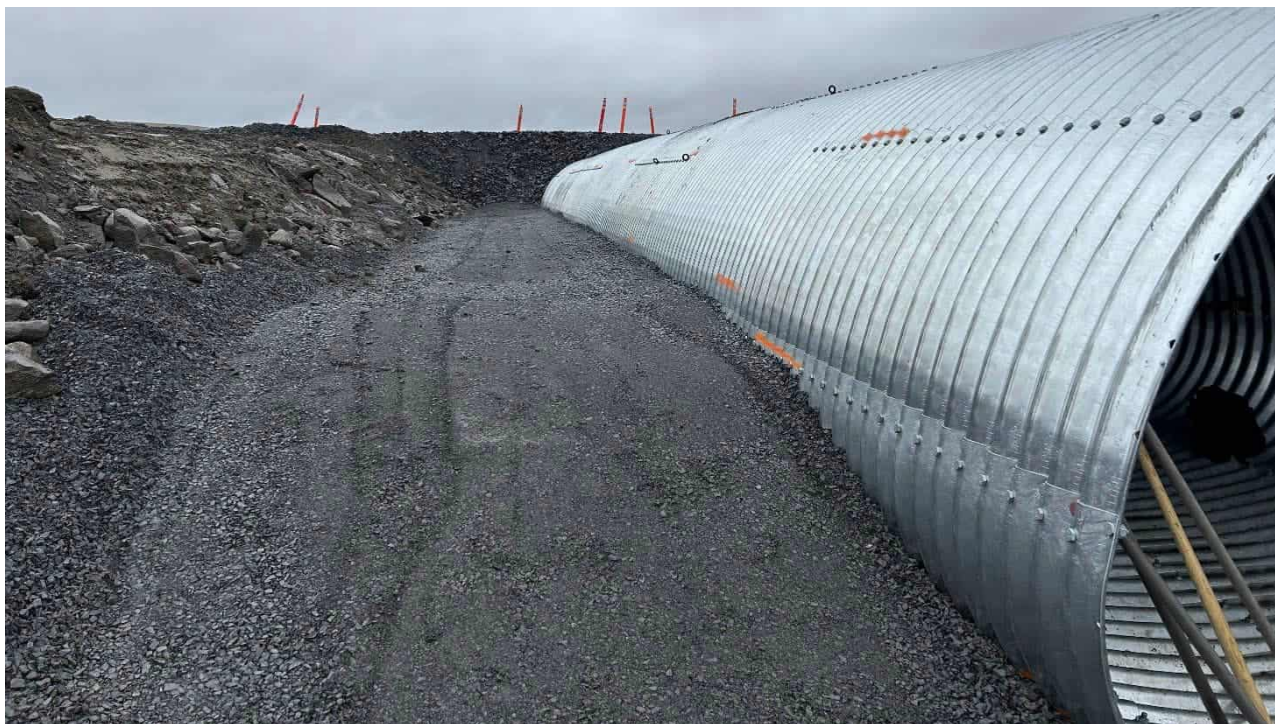
Photograph 9: Main Channel Culvert Left Barrel Backfill Placement and Compaction to Approximately 900 mm. Taken August 22, 2023 (Provided by B2Gold).
