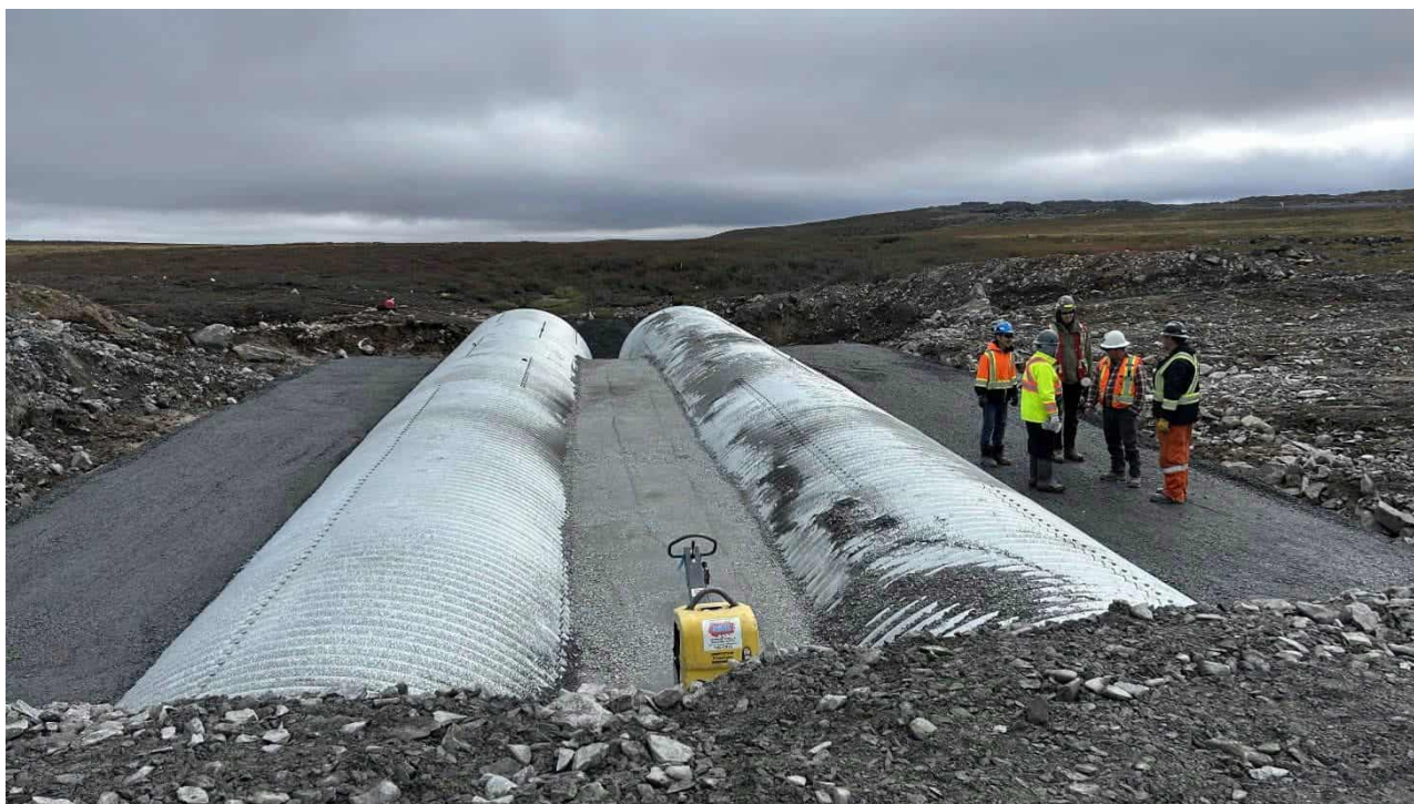
Photograph 12: Main Channel Culverts Backfill Placement and Compaction to Approximately 2400 mm Looking Upstream. Taken August 24, 2023 (Provided by B2Gold).
