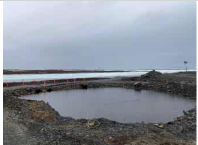
Photo 4: Twin multiplate culvert excavation at 16:15.
