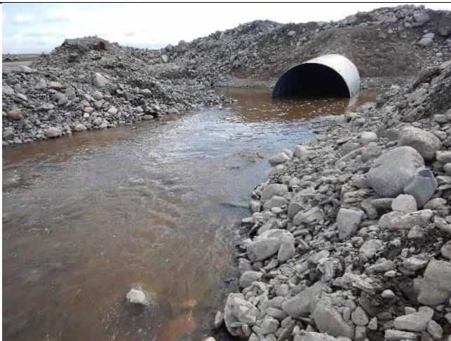
Photo 3: Secondary culvert discharging diverted RSW main channel over temporary outlet riprap apron looking upstream at 12:05.
