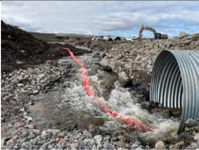
Photo 1: Secondary culvert receiving diverted flow from RSW main channel looking from RDB to LDB at 10:50.
