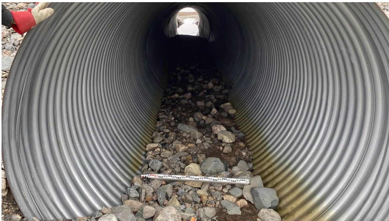
Photograph 25: Secondary Channel Culvert Substrate and Embedment Material Looking Downstream from Culvert Inlet, Taken September 17, 2023
