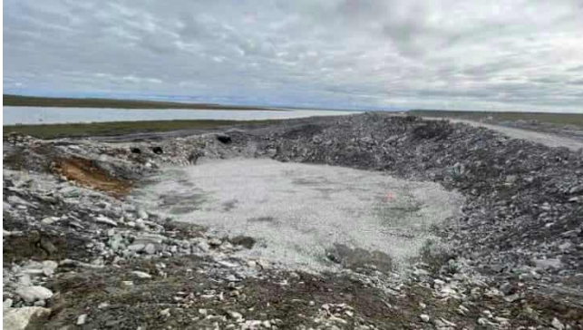
Photo 3: Prepared Segment of The Culvert Bedding at 08:40.
