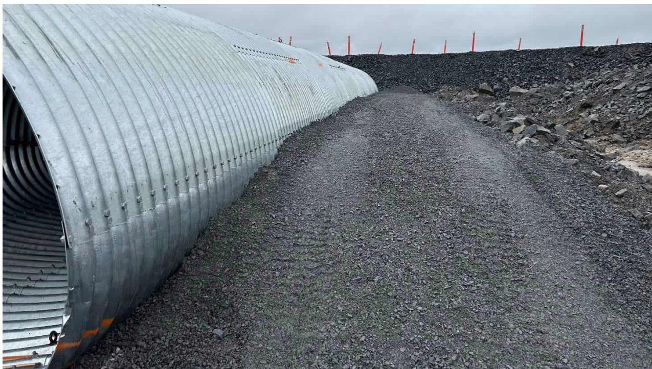
Photograph 10: Main Channel Culvert Right Barrel Backfill Placement and Compaction to Approximately 900 mm. Taken August 22, 2023 (Provided by B2Gold).
