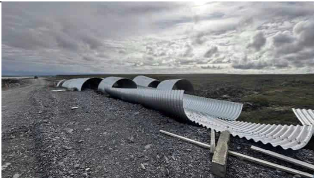
Photo 5: Partially Assembled Culvert Plates
