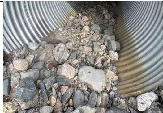
Photo 6: Minimal channel substrate was identified inside the secondary culvert
