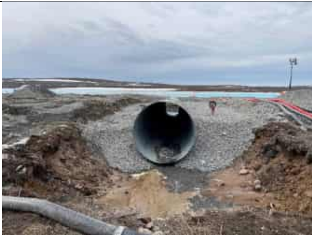
Photo 3: Secondary culvert inlet section raised without bedding underneath looking downstream at 16:52.
