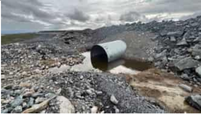
Photo 7: Outlet of the secondary culvert was partially submerged under low-flow condition
