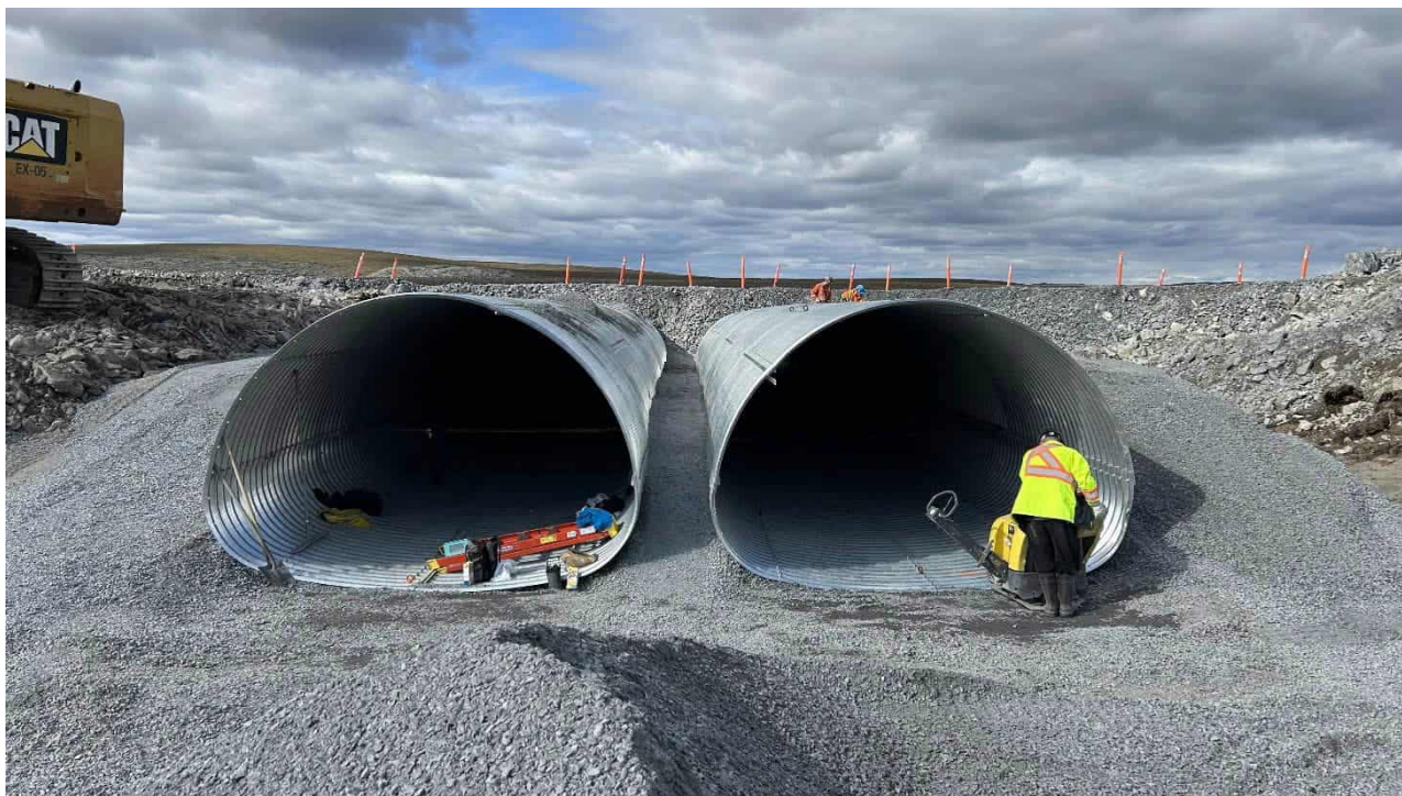
Photograph 11: Main Channel Culverts Inlets and Backfill Placement and Compaction. Taken August 23, 2023 (Provided by B2Gold).
