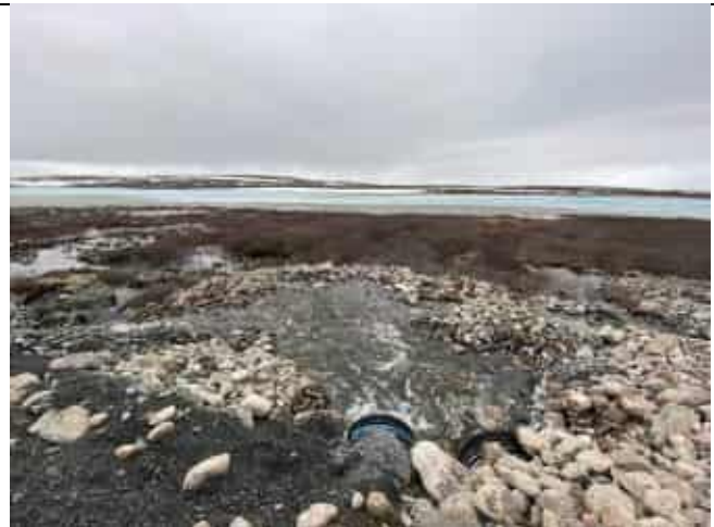
Photo 4: Temporary culverts discharging twin multiplate culvert excavation
