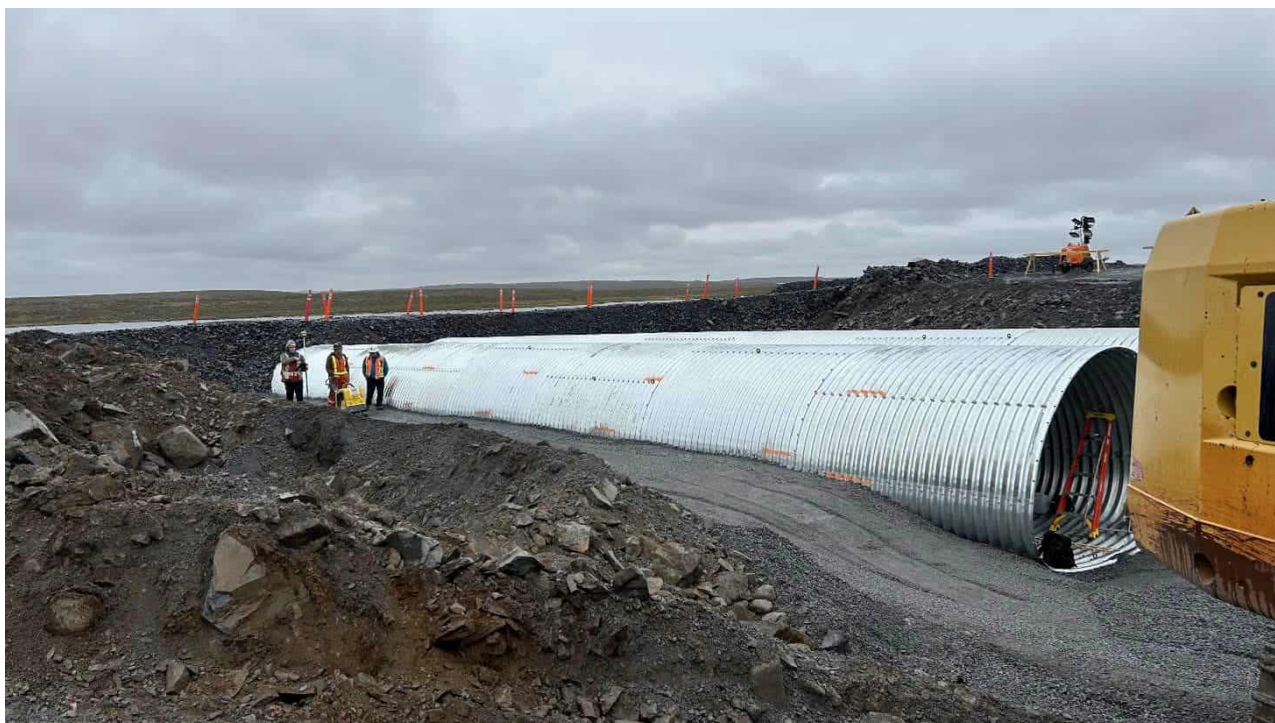
Photograph 7: Main Channel Culverts Backfill Placement and Compaction to Approximately 900 mm Above Culvert Invert. Taken August 22, 2023 (Provided by B2Gold)
