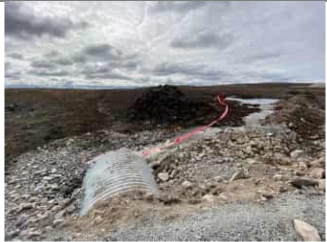
Photo 2: Secondary culvert receiving diverted flow from RSW main channel looking upstream at 10:49.
