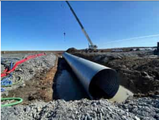
Photo 3: Secondary culvert placement with 4 sections looking upstream at 16:09.
