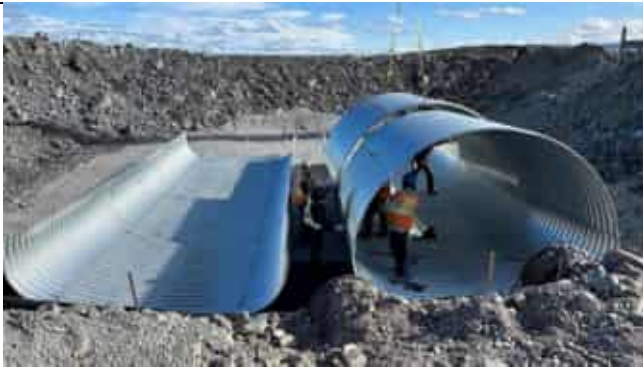
Photo 3: Top plate assembly began prior to placement of embankment material and boulder cluster
