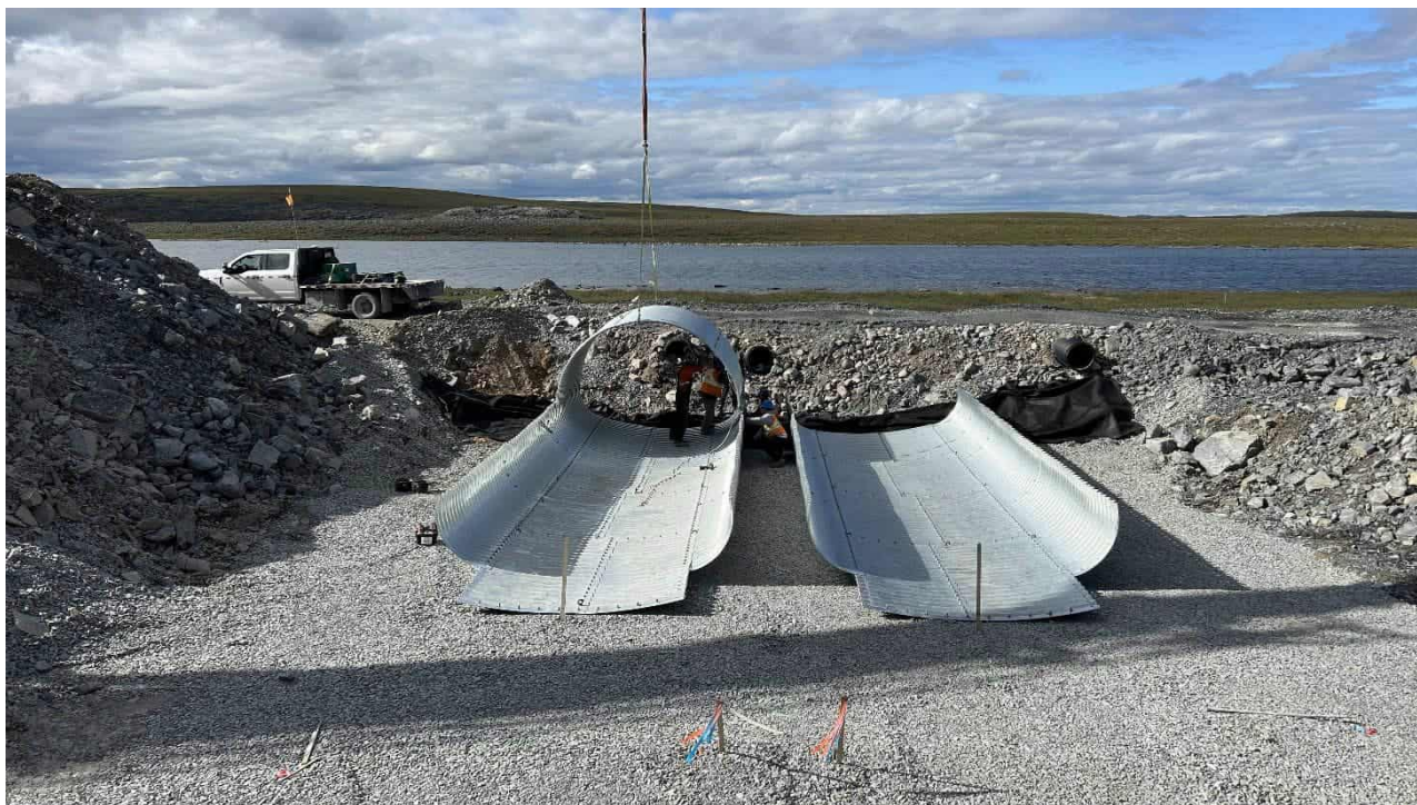
Photograph 3: Main Channel Culverts Assembly on Bedding Layer Looking Downstream. Taken August 6, 2023
