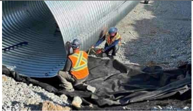
Photo 2: Non-woven geotextile extends 2 m beneath culvert
