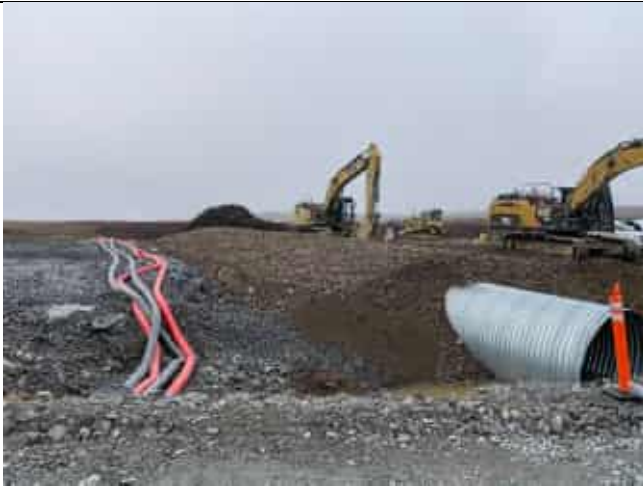
Photo 1: Secondary culvert raw esker backfill 0.3 m above culvert crest looking upstream at 8:59.
