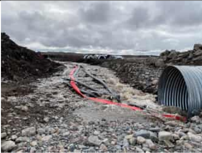
Photo 1: Secondary culvert receiving diverted flow from RSW main channel looking from RDB to LDB at 15:58.
