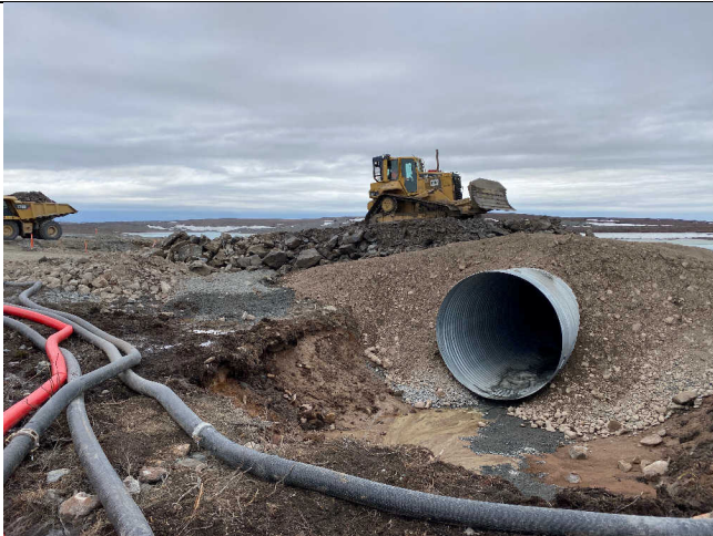
Photo 3: RoQ placement above raw esker backfill looking downstream at 16:52.
