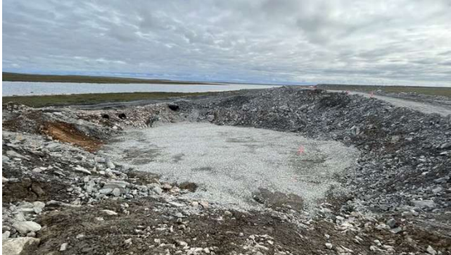
Photo 3: Prepared Segment of The Culvert Bedding at 08:40.
