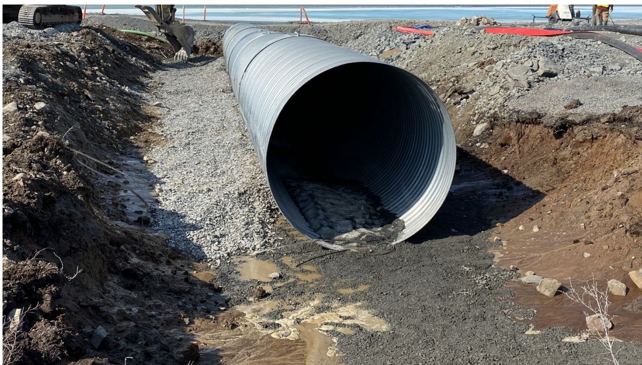
Photograph 20: Secondary Channel Culvert Inlet Placement on Bedding Material, Taken May 11, 2023
