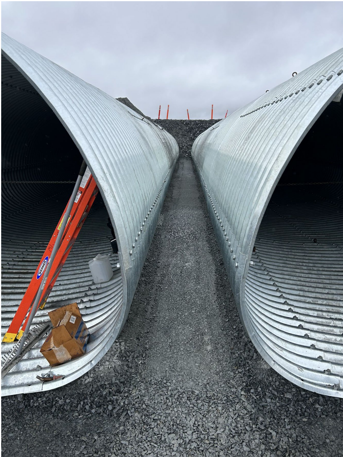
Photograph 8: Backfill Placement and Compaction Between the Main Channel Culverts. Taken August 22, 2023 (Provided by B2Gold).
