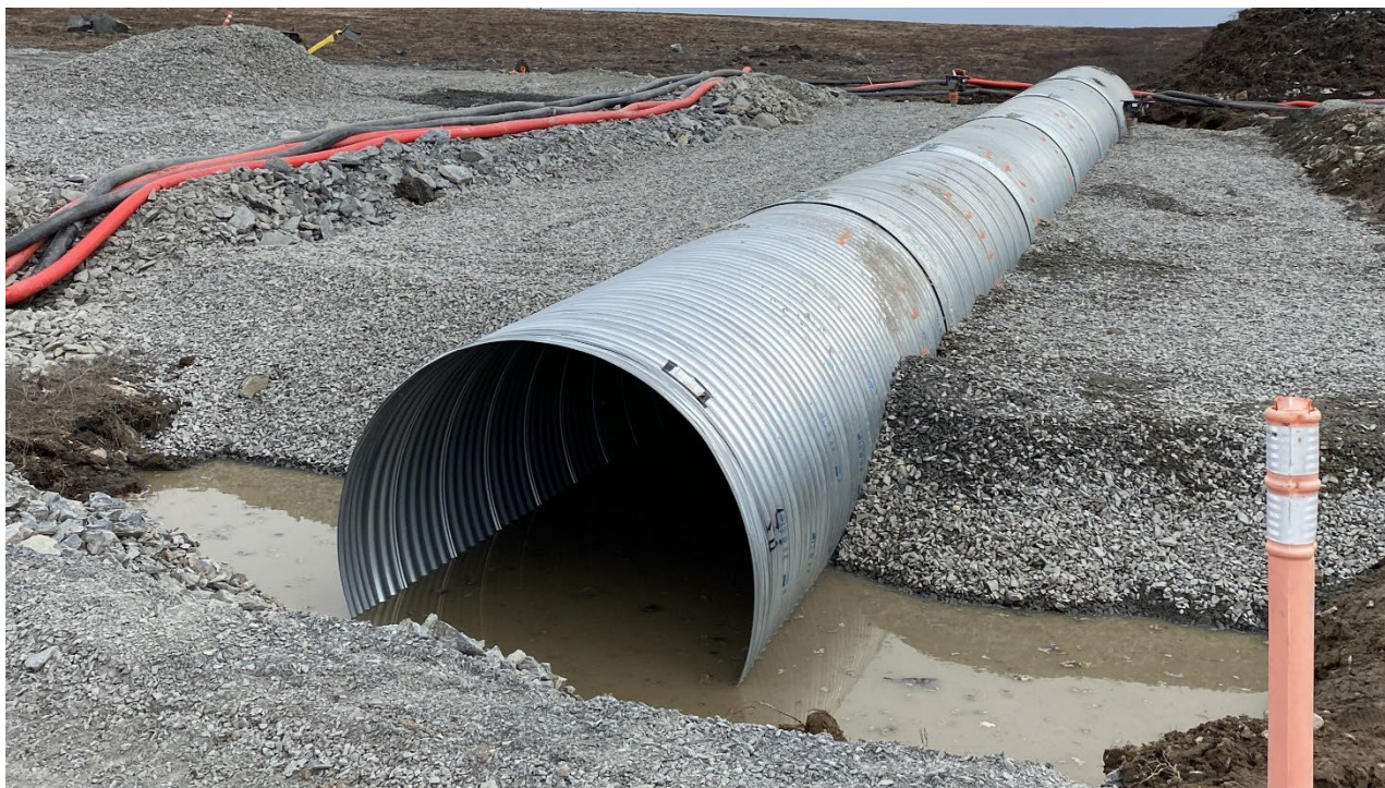
Photograph 21: Secondary Channel Culvert Backfill Placement with Approximately 900 mm on Left Downstream Wall From Outlet at Left Downstream Bank, Taken May 13, 2023
