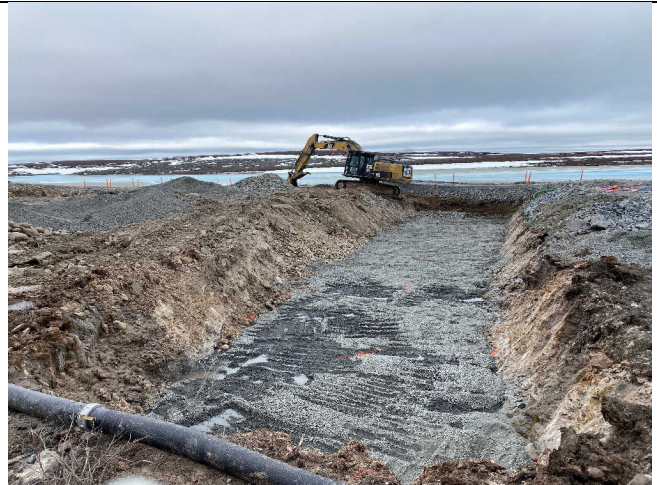
Photo 2: Secondary culvert excavation with bedding placed looking downstream at 8:24.
