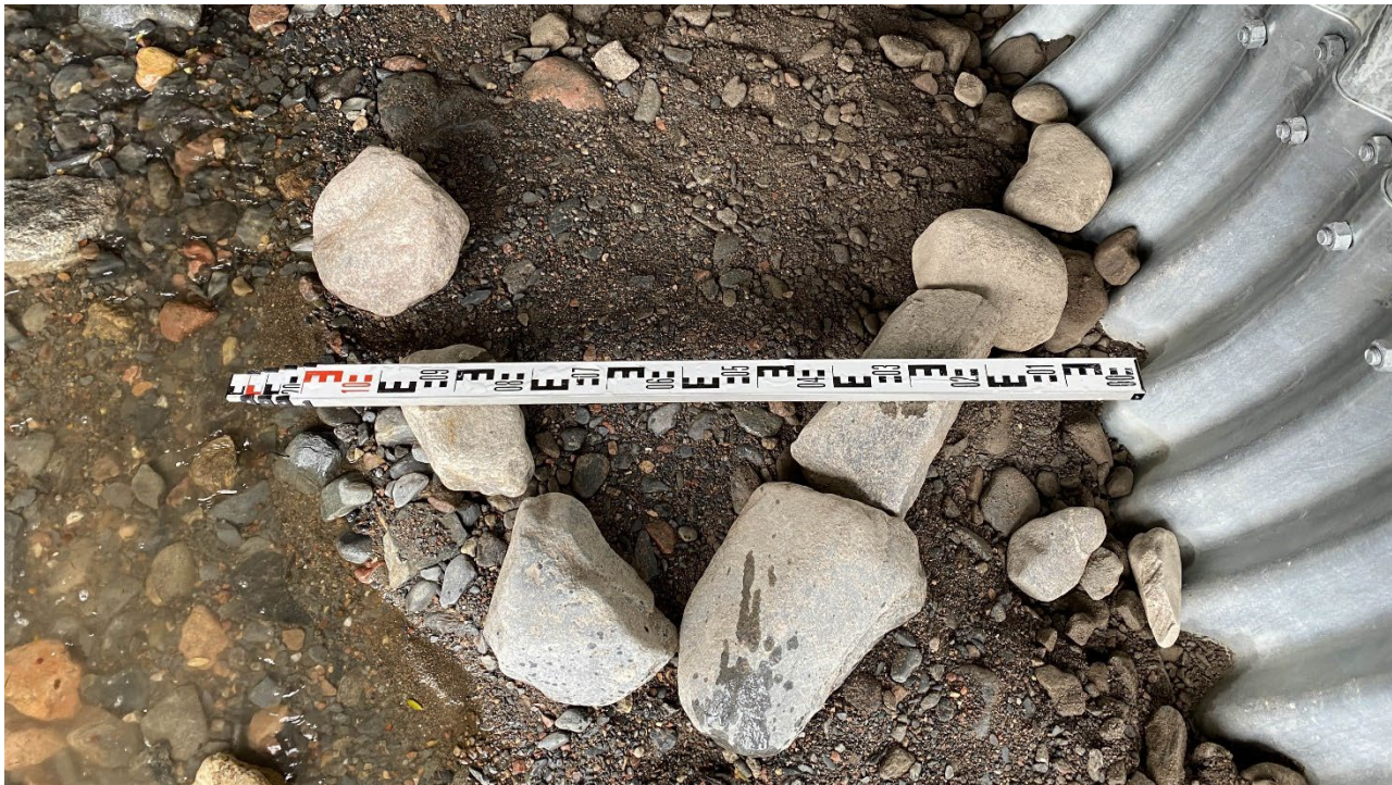
Photograph 17: Main Channel Culverts Typical Boulder Cluster and 1 m Scale Bar, Taken September 17, 2023
