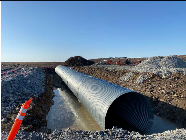
Photo 1: Secondary culvert placement with 6 sections looking upstream at 7:32.
