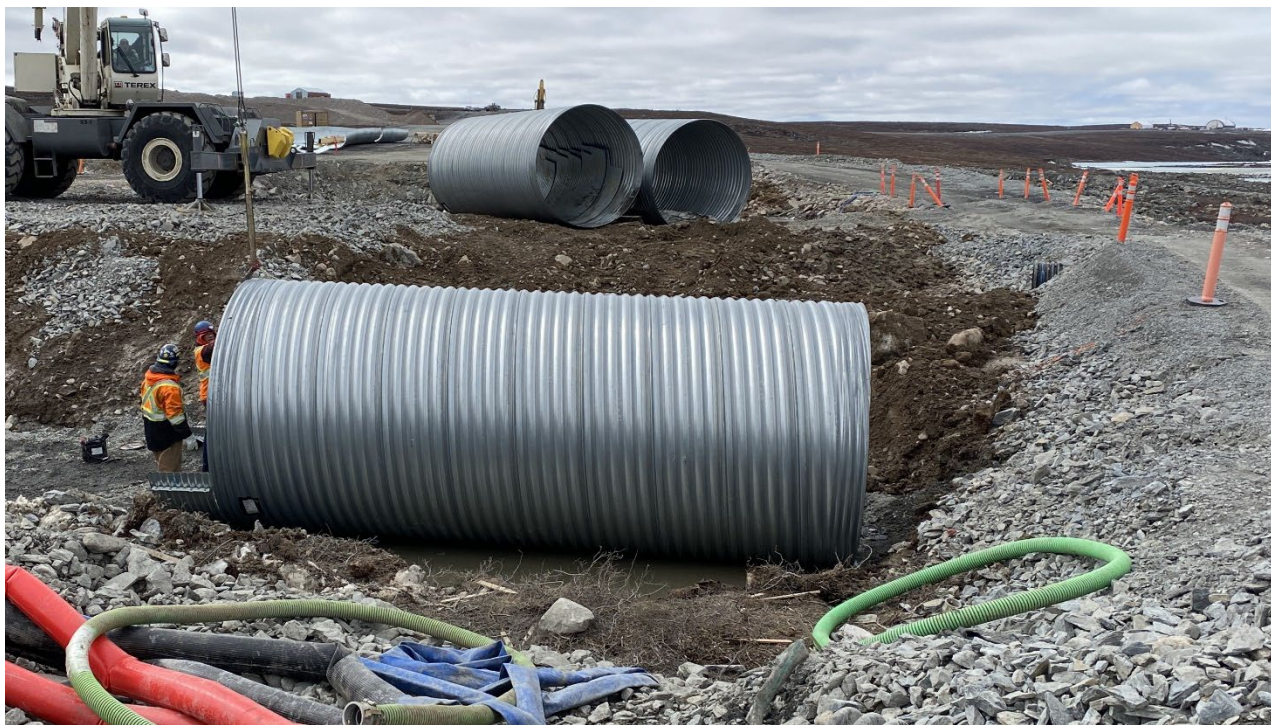
Photograph 19: Secondary Channel Culvert Outlet Placement on Bedding Material, Taken May 11, 2023
