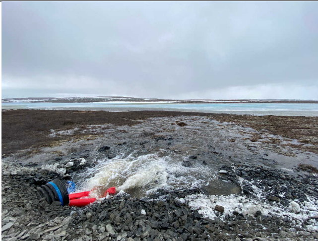
Photo 3: Dewatering pump discharge downstream of secondary culvert excavation
