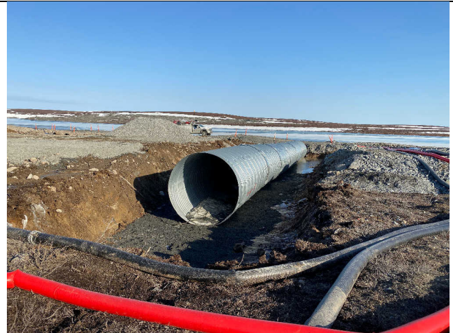
Photo 2: Secondary culvert placement with 6 sections looking downstream at 7:28.
