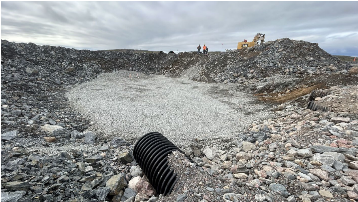
Photograph 1: Main Channel Excavation Extents and Bedding Layer Looking Upstream. Taken August 5, 2023
