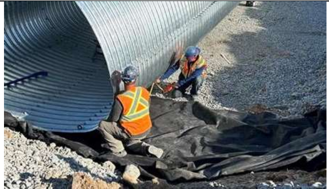
Photo 2: Non-woven geotextile extends 2 m beneath culvert
