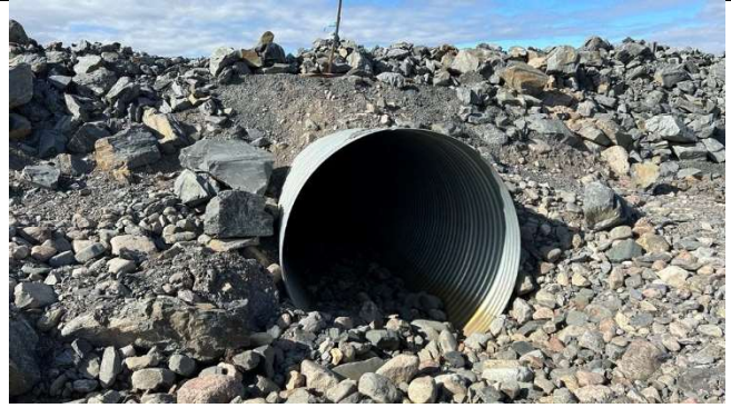
Photo 8: No non-woven geotextile was identified at the inlet and the outlet secondary culvert
