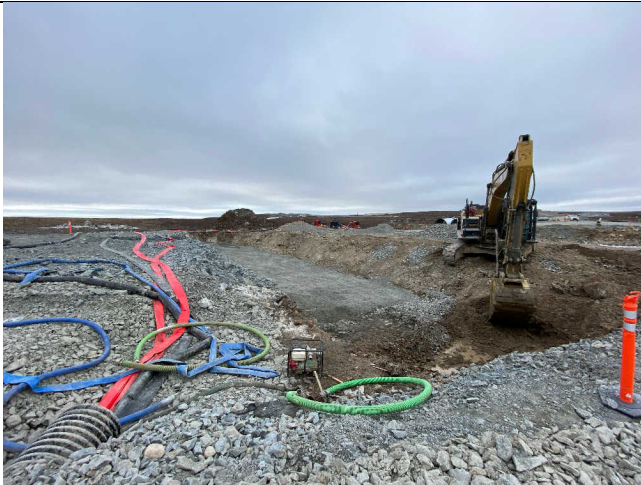
Photo 1: Secondary culvert excavation with bedding placed looking upstream at 8:23.
