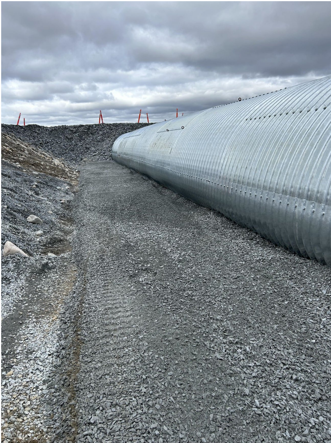
Photograph 5: Start of Backfill Placement for Main Channel Culverts. Taken August 21, 2023 (Provided by B2Gold)
