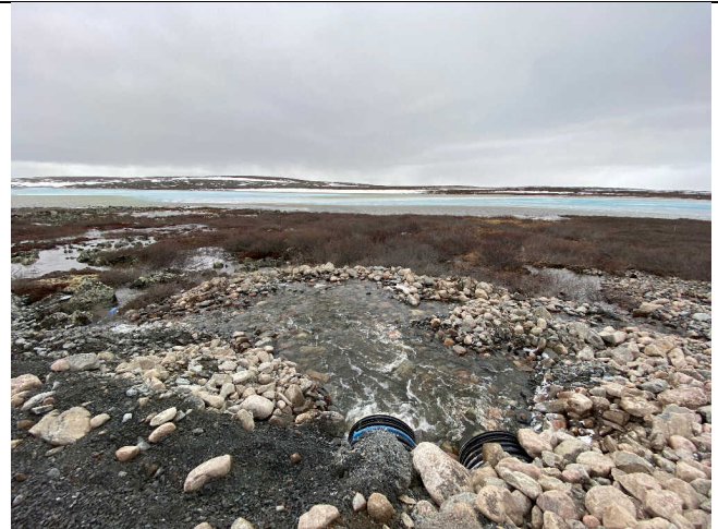
Photo 4: Temporary culverts discharging twin multiplate culvert excavation
