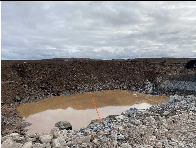
Photo 3: Temporary diversion dam isolating twin multiplate excavation looking upstream at 16:13.
