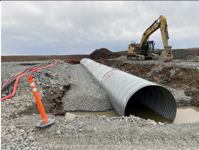
Photo 1: Secondary culvert placement with 6 sections looking upstream at 7:56.
