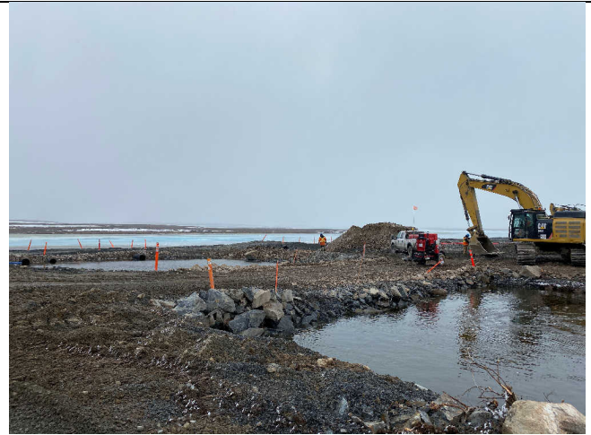
Photo 2: Lower pond seeping into twin multiplate excavation through temporary road.
