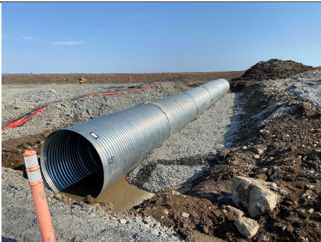
Photo 3: Secondary culvert backfill placement on left downstream bank looking upstream at 16:40.
