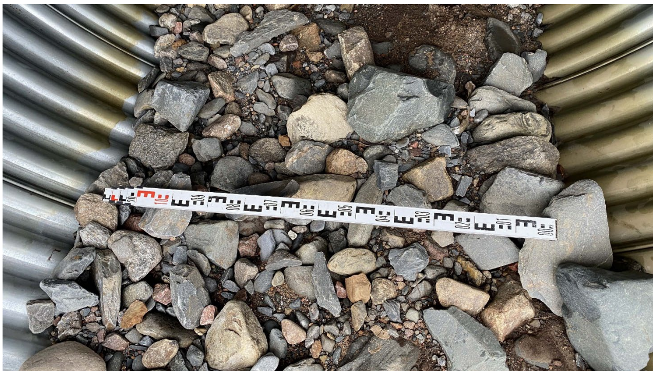
Photograph 26: Secondary Channel Culvert Substrate and 1 m Scale Bar at Inlet, Taken September 17, 2023
