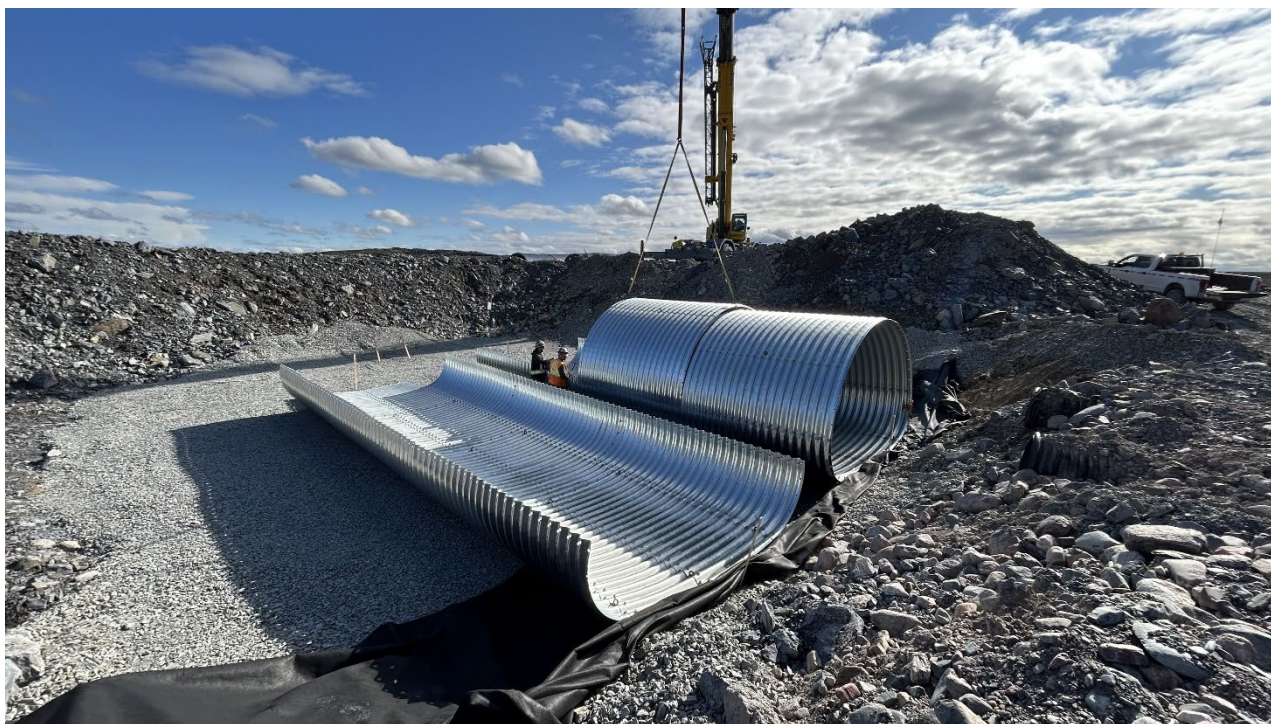
Photograph 4: Main Channel Culverts Assembly on Bedding Layer Looking Upstream. Taken August 6, 2023
