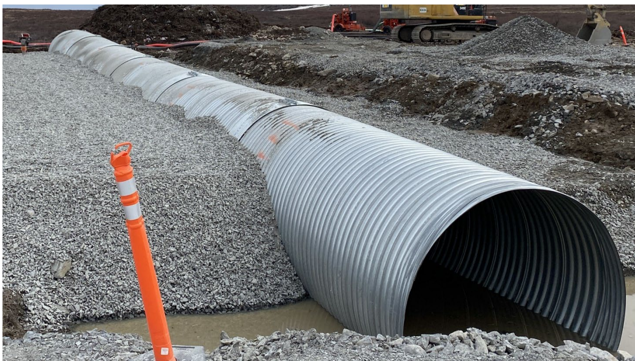
Photograph 22: Secondary Channel Culvert Backfill Placement with Approximately 1500 mm on Right Downstream Wall From Outlet at Right Downstream Bank, Taken May 13, 2023
