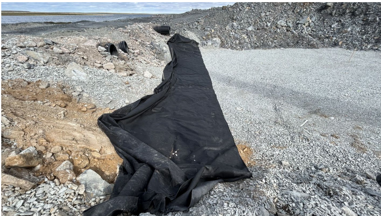
Photograph 2: Main Channel Geotextile Placement at Downstream End and Bedding Layer. Taken August 6, 2023
