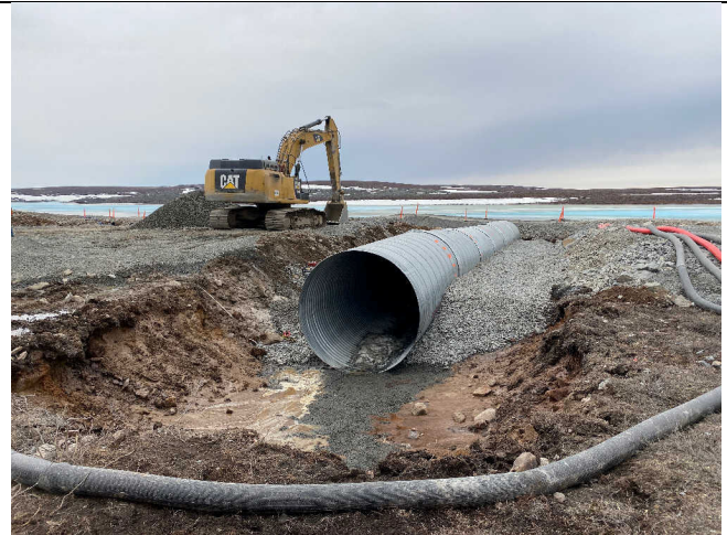
Photo 2: Secondary culvert placement with 6 sections looking downstream at 7:58.
