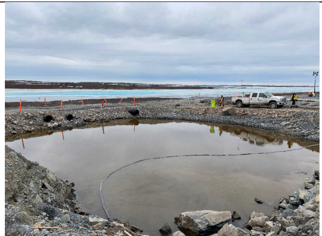
Photo 4: Twin multiplate culvert excavation at 16:40.
