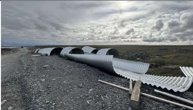
Photo 5: Partially Assembled Culvert Plates
