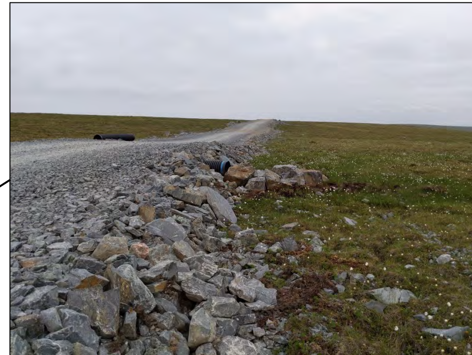
Photo 3 - Outlet, note rocks placed to dissipate water energy at culvert outlet. Cover above pipe may be insufficient/problematic when traversed by larger vehicles.
