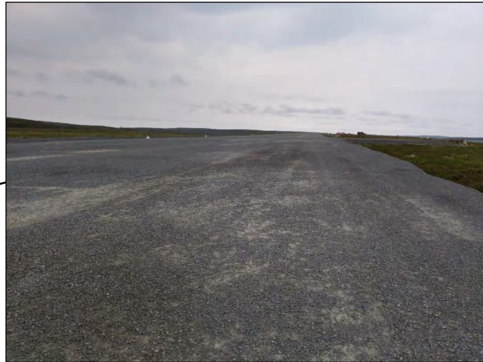
Photo 27 – View northerly direction of airstrip surface, no cracking observed despite lower fill thickness
