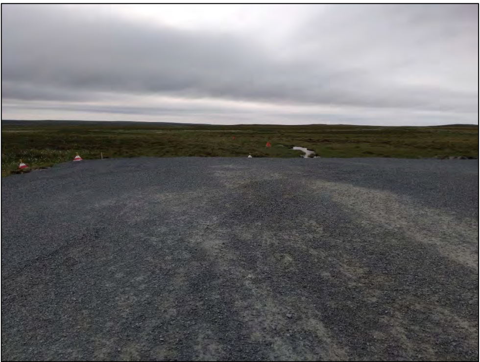
Photo 26 – Southern end of airstrip where thick fill note, no cracking or undulation observed
