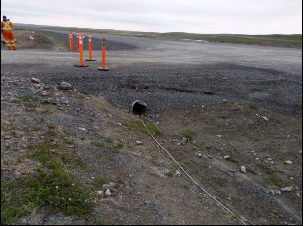
Photo 21 – Culvert along airstrip channel along northern edge
