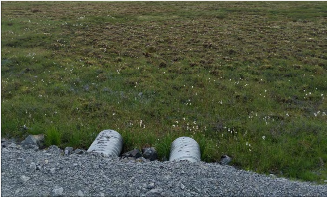
Photo 18 – Culvert invert at outlet below tundra surface
