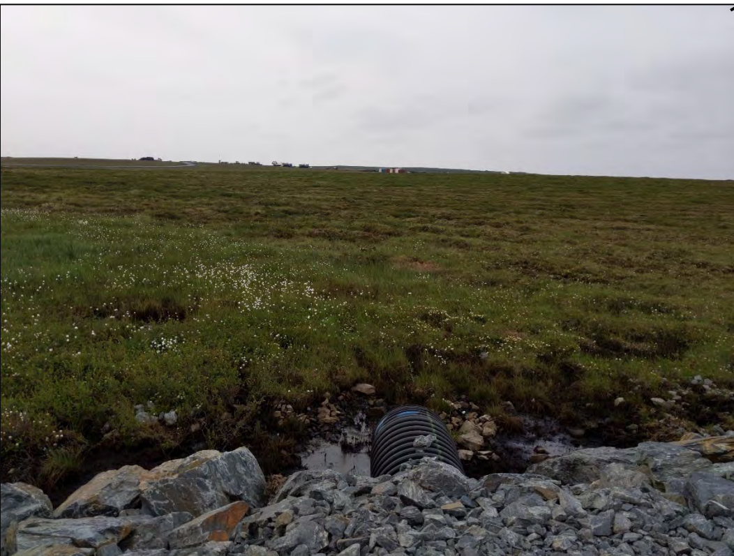
Photo 2 – Inlet, no ponding observed
