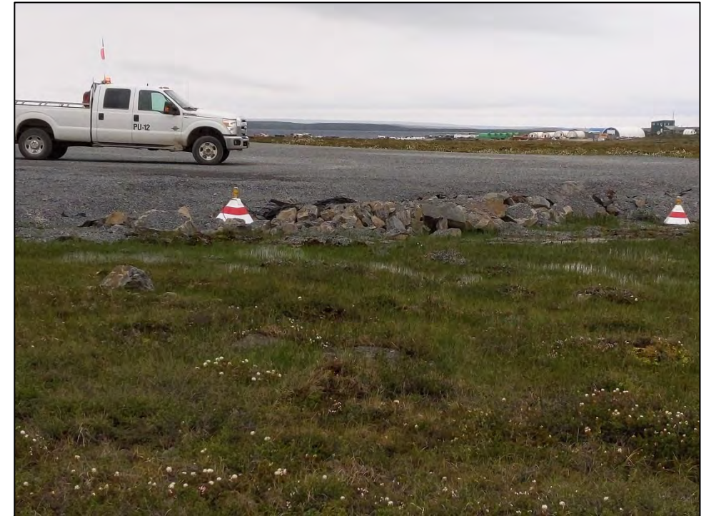
Photo 13 – Southern end of airstrip, note thin fill thickness
