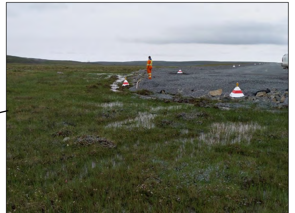
Photo 14 – Water ponding at southern point of airstrip, flow continues southeast
