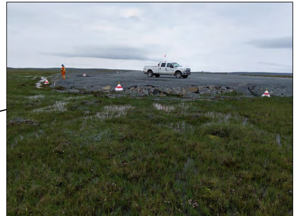
Photo 18 – water ponding at southern end of airstrip, also note think airstrip fill.
