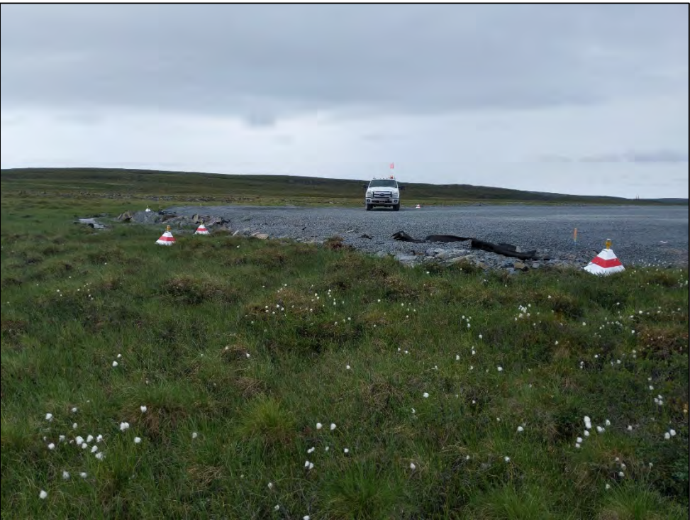
Photo 22 – southern end of airstrip, note thick airstrip fill thickness; geotextile exposed.
