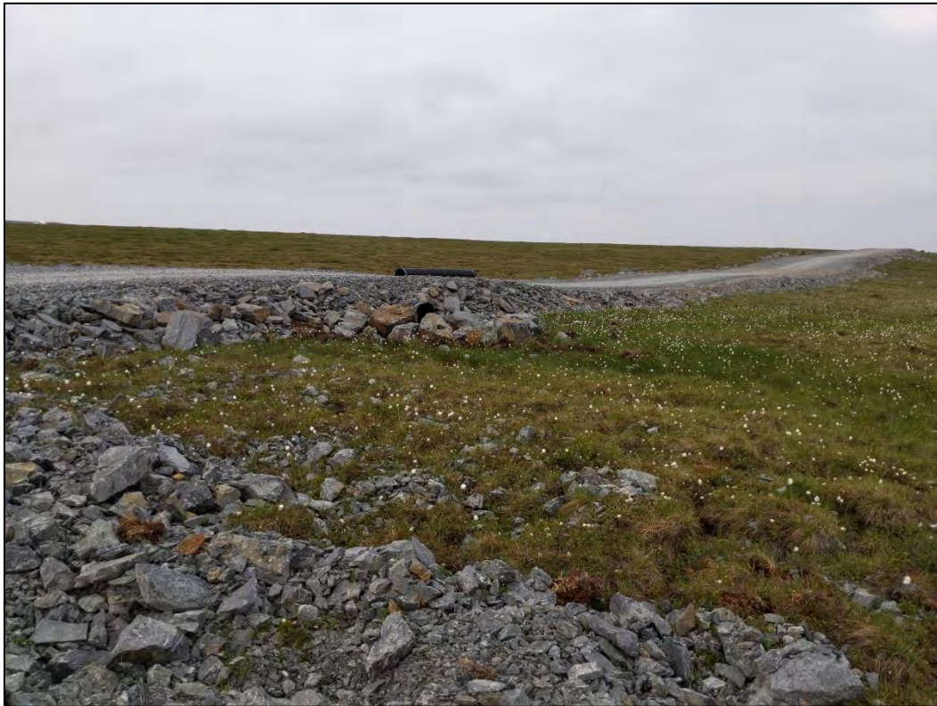
Photo 1 – Outlet, note rocks placed to dissipate water energy at culvert outlet.
