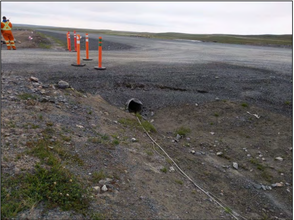
Photo 21 – Culvert along airstrip channel along northern edge
