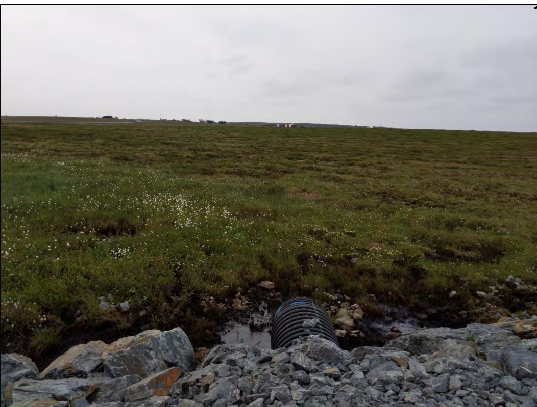
Photo 2 – Inlet, no ponding observed
