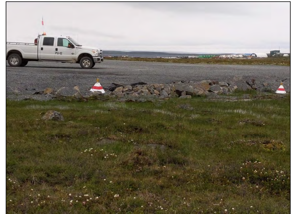
Photo 13 – Southern end of airstrip, note thin fill thickness
