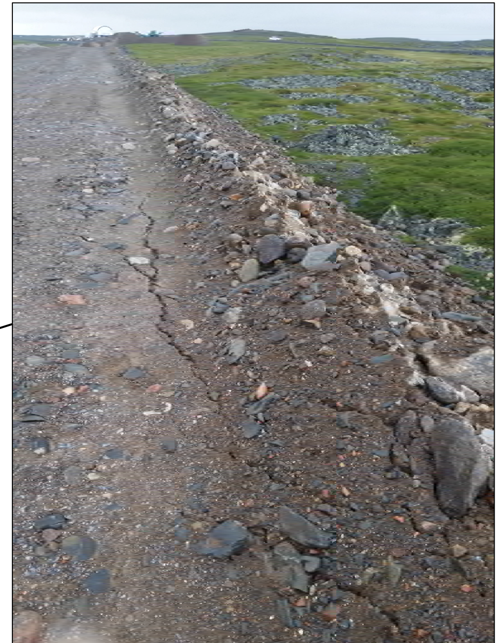
Photo 23 – Note cracks on roadway, road fill ~4 m above tundra
