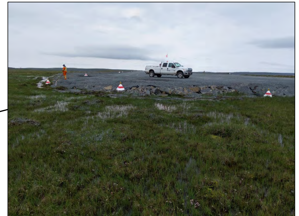
Photo 18 – water ponding at southern end of airstrip, also note think airstrip fill.
