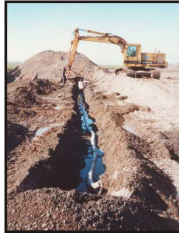
French drain and catch basin construction
