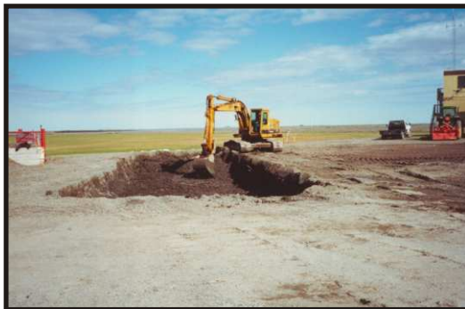
Benzene contaminated soil excavation
