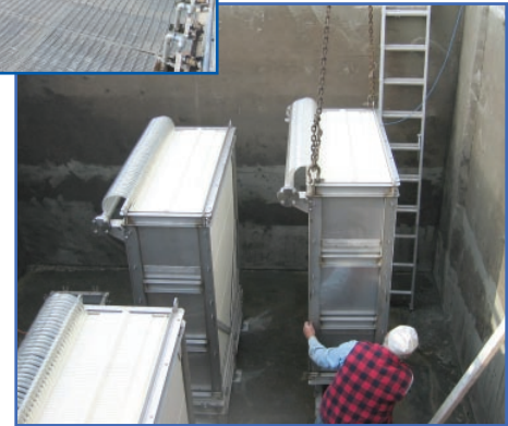
Installing the MBR units.
